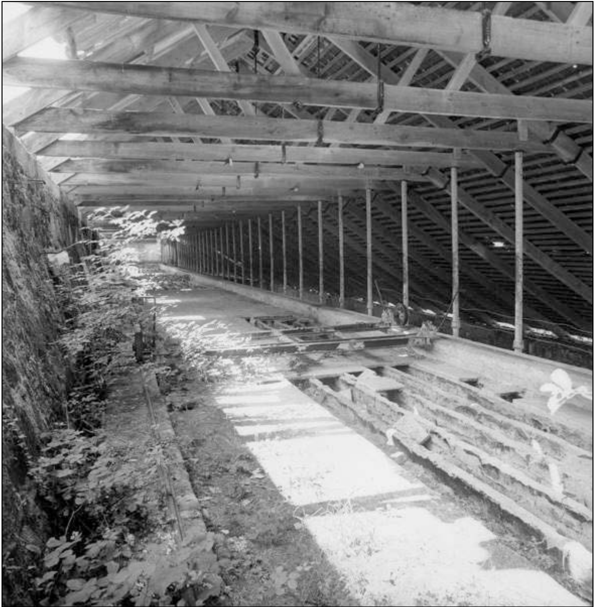
Figure 37 The drying floor and travelling bridge (used for distributing semi-liquid clay across the drying floor) at the derelict Carlyon Farm china-clay dry in the Trenance valley, near St Austell. It was completed in 1921 and was reputedly the largest pan kiln ever built. The photograph dates to between 1968 and 1984. (Photograph: ECC archive, held by the China Clay History Society.)
