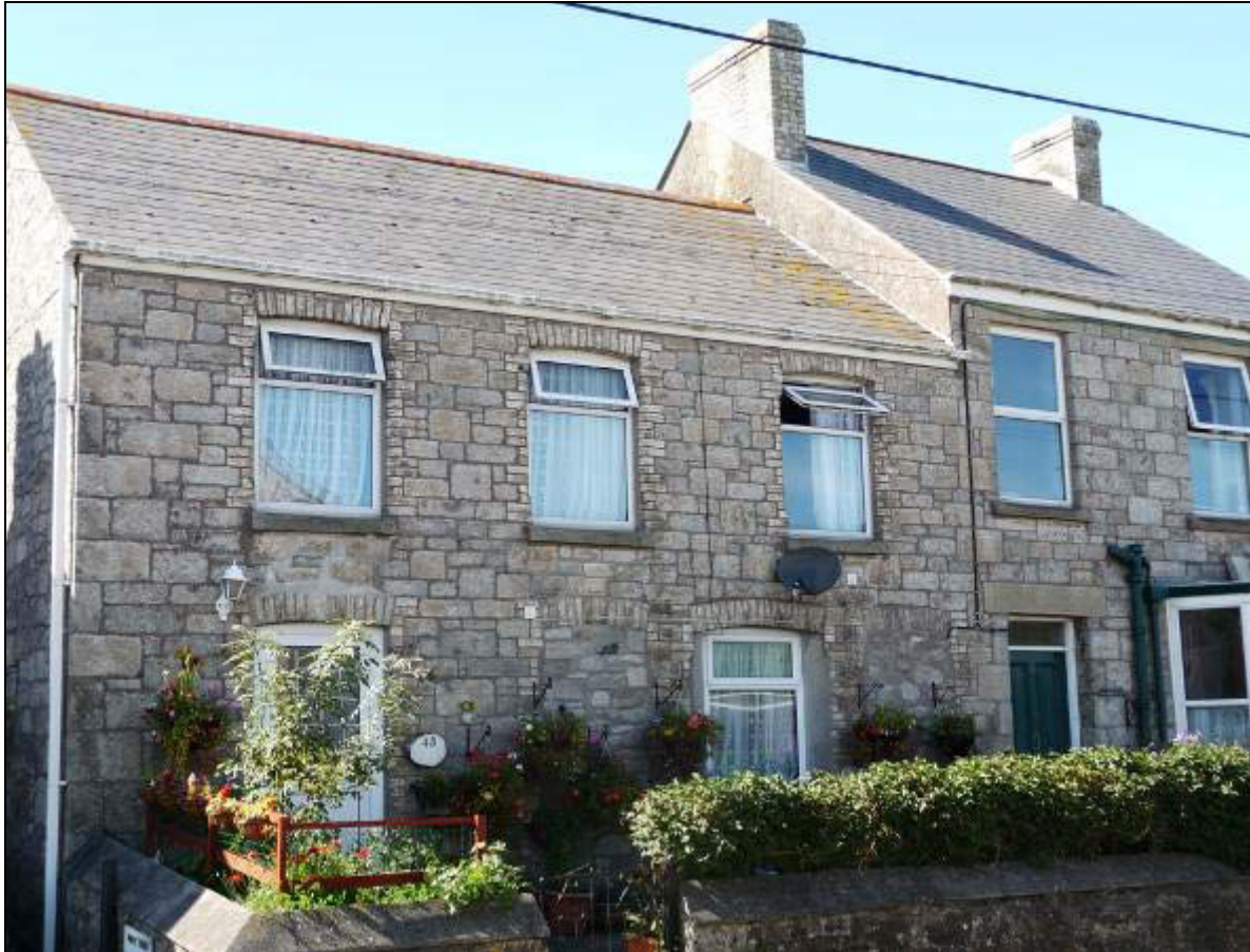
Figure 84 Granite and brick, the latter almost certainly from local brickworks, used on the elevations of late nineteenth-century houses in Fore Street, St Stephen-in-Brannel. (Photograph: Graeme Kirkham.)
