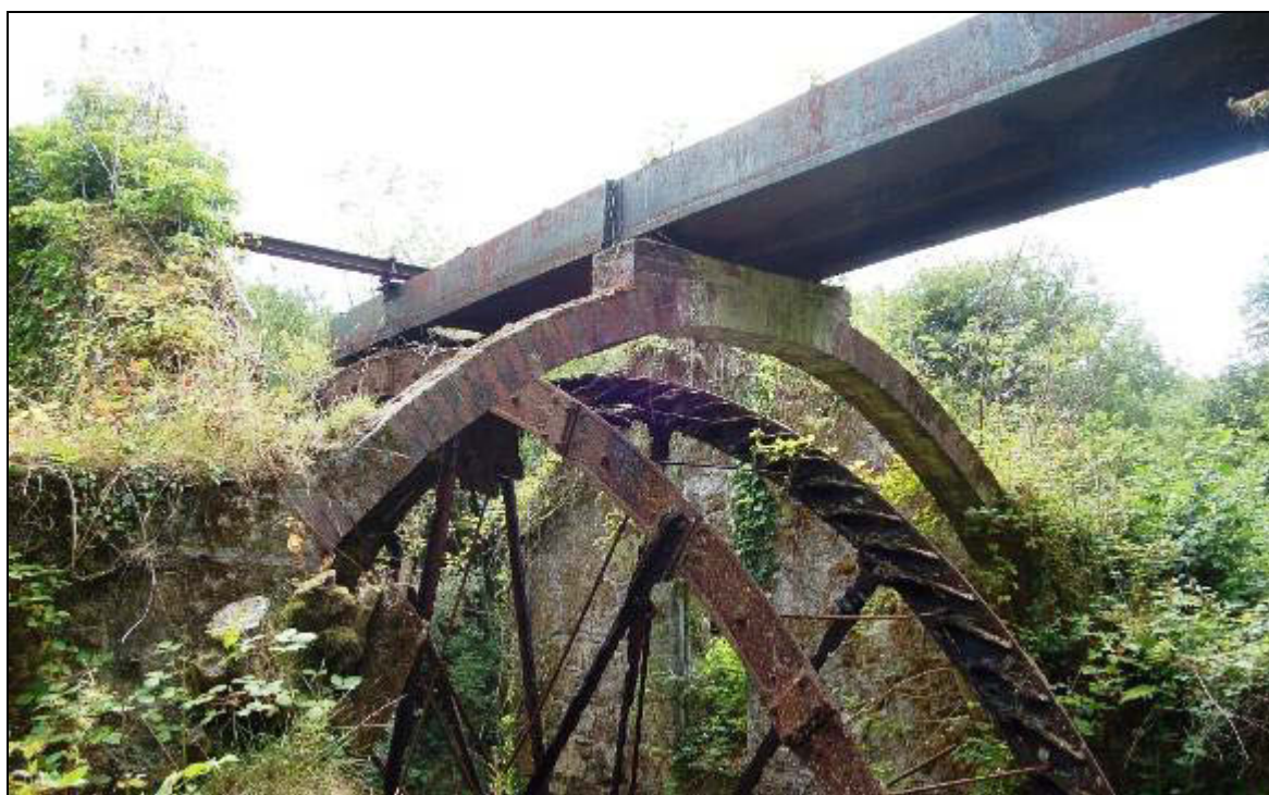
Figure 99 The remains of an overshot water wheel and launder at Big Wheel china stone mill in the Tregargus valley, photographed in 2006. The complex, built about 1898, is a Scheduled Monument and a Grade II Listed Building (Cole and Smith 2002). (Photograph: Historic Environment, Cornwall Council.)
