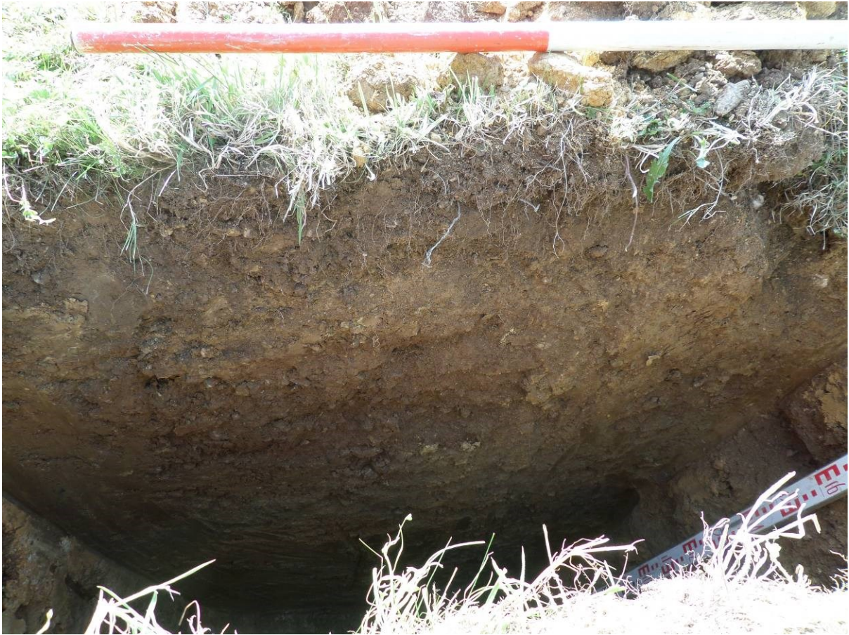
Figure 13: South facing section of Test pit 6 showing layer of possible degraded, re-deposited or older subsoil below a section of yellow clay subsoil and covering topsoil.
