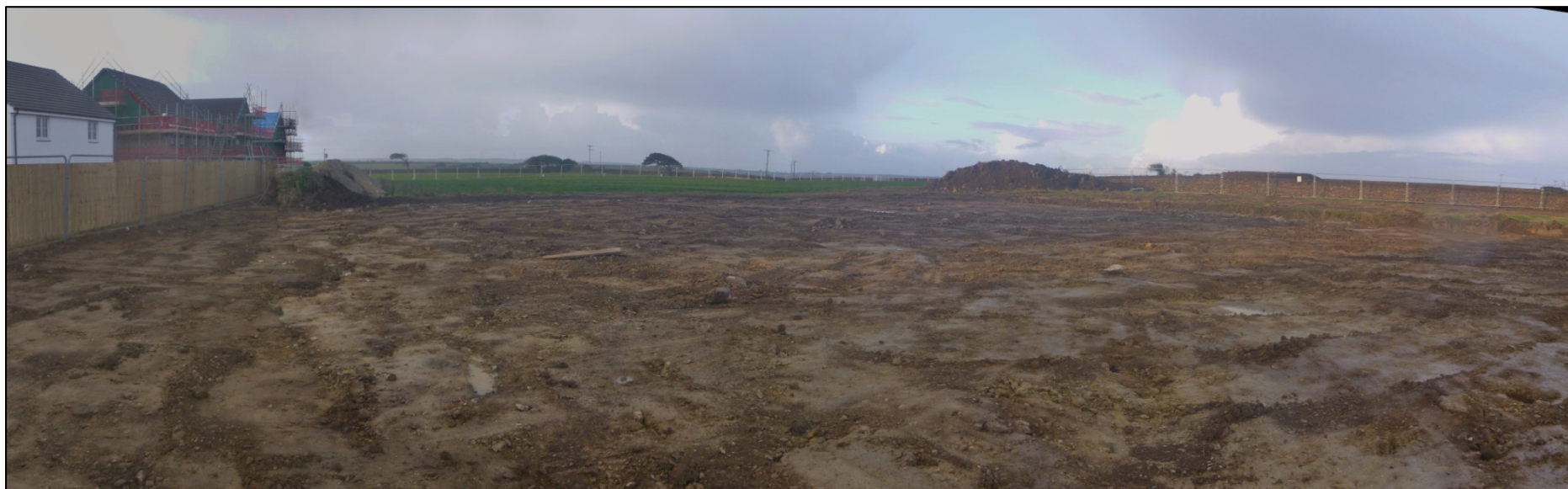
Figure 4: View of site post excavation looking south.
