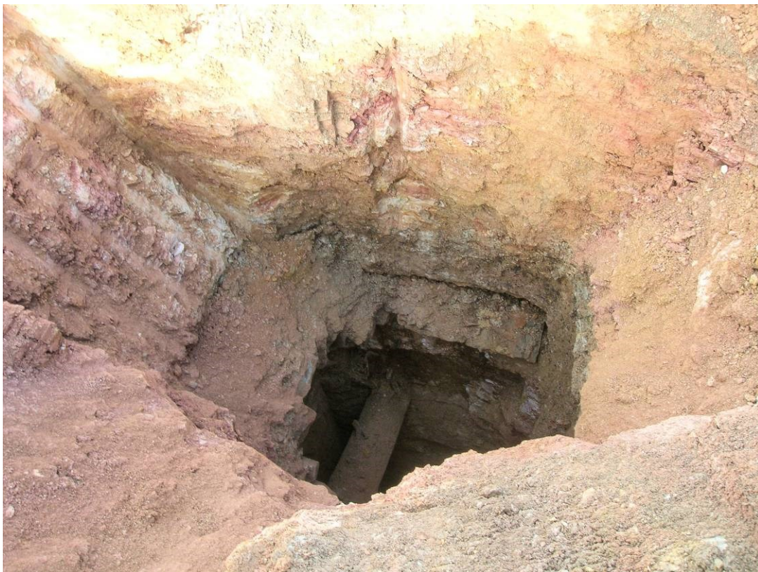
Figure 27. Hallenbeagle West. Shaft [236] showing rock cut ledge seating for blocking arch.
