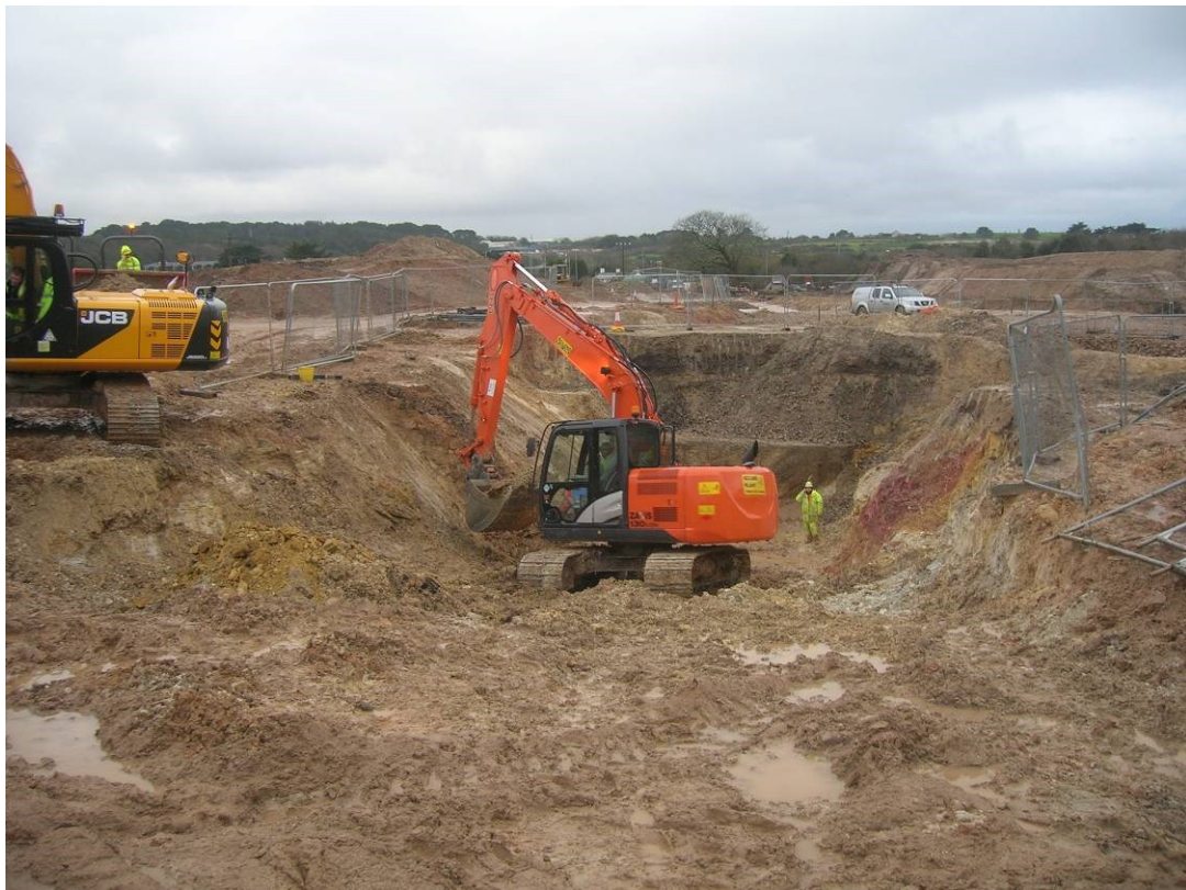
Figure 31. Hallenbeagle West Openwork [249]. Excavation of north-east terminal.
