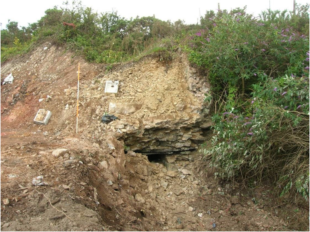
Figure 23. Hallenbeagle East. Area 1. Remnants of engine house [107] possibly that for an engine built by James Watt. Scale bar = 2.0m.
