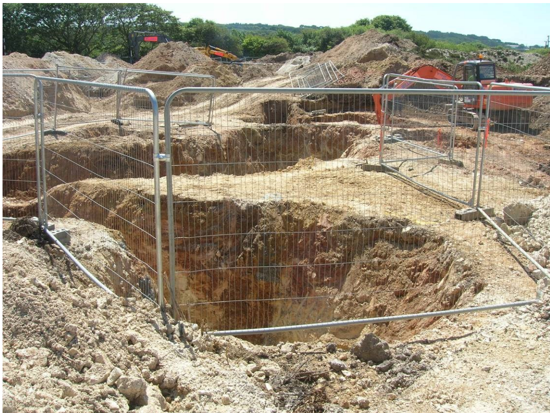
Figure 18. Hallenbeagle East. Outcrop shafts [35], [66], [67], [68] and [70]. Looking south-west.
