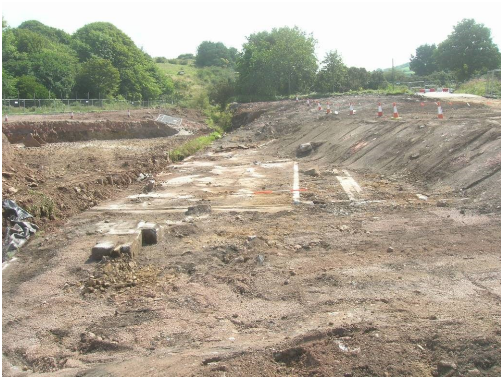
Figure 19. Red River Valley. Photograph of the concrete flooring and settling tanks or rag frame bases [84], part of the tailing works within the valley looking south-east.
