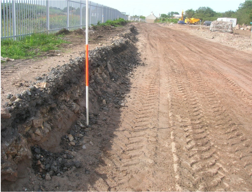
Figure 9. General view of Wilson Way showing spread of tailing sand over entire area.
