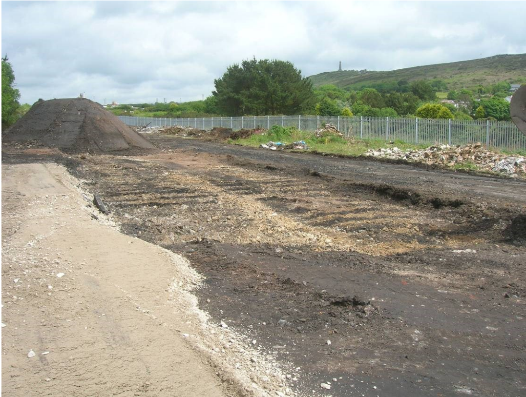
Figure 29. Photograph. Dudnance Lane to Wilson Way. Note the sleepers of the 1909 railway tracks preserved as 'ghosts' by the ballast material
