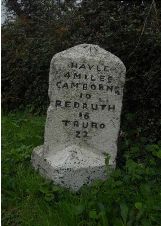
Figs 59 and 60. Sites 4 and 6. Cockwells and Canonstown turnpike milestones. Both show signs of impact damage, whilst the example at Canonstown has become part-buried in the tarmac pavement.
