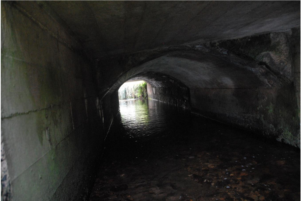
Fig 56. Site 2. The central section of the under-bridge at Crowlas retains its original twin arched stone structure, though the flanking modern sections are of concrete.
