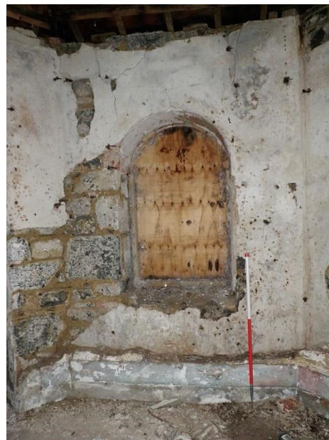
Fig 32 Blocked window in north-east wall of SE lodge.
