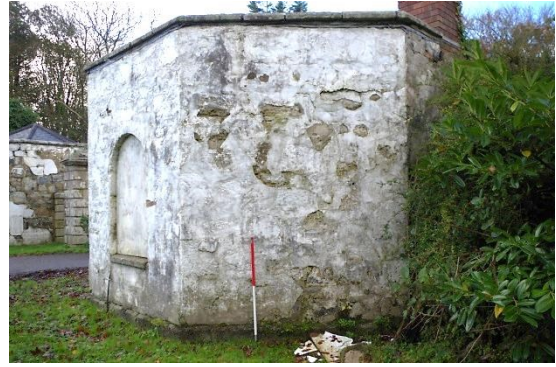
Fig 16 North elevation of NW lodge.
