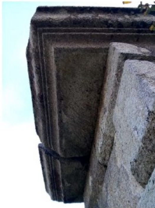
Plate 16: Extent of displacement of cap stones.
