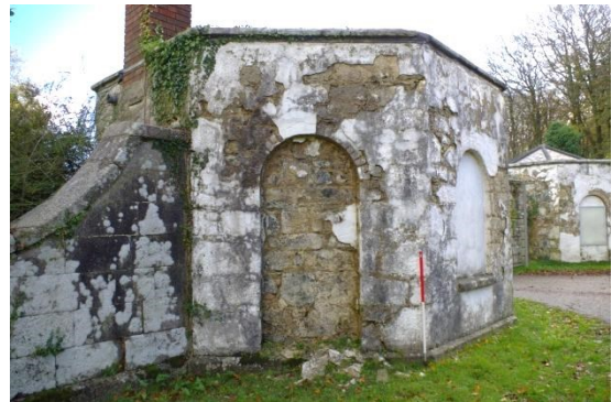
Fig 17 West elevation of NW lodge.
