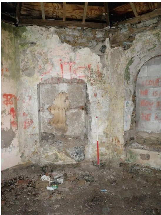
Fig 22 Cupboard behind blind doorway in south wall of NW lodge.
