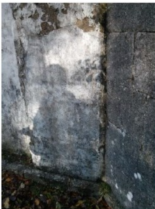
Plate 4: Granite plinth to base of wall, note junction with flanking wall.
