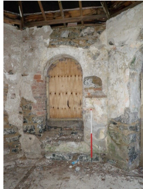
Fig 24 Blocked window in north-east wall of NW lodge.
