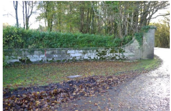
Fig 37 Front (west) elevation of SE flanking wall and pier.
