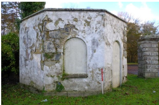
Fig 29 North-east elevation of SE lodge.
