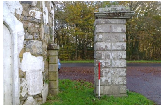
Fig 38 North-east elevation of free-standing gate pier.
