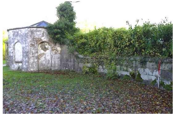
Fig 36 Front (west) elevation of SE flanking wall.
