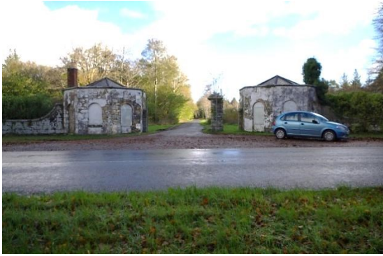
Fig 12 Lodges looking north-east from road.
