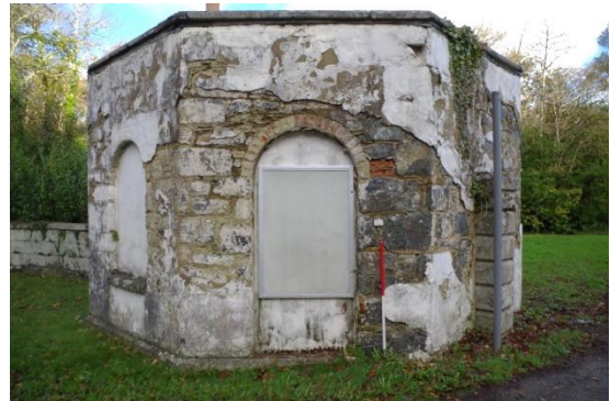
Fig 18 South-west elevation of NW lodge.
