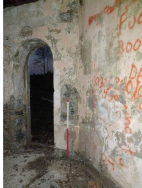
Fig 23 Door opening in east wall of NW lodge.
