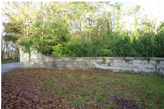
Fig 35 Front (south) elevation of NW flanking wall and pier.
