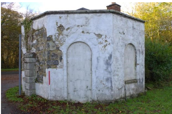
Fig 15 East elevation of NW lodge.
