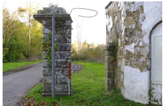
Fig 39 South-west elevation of free-standing gate pier.
