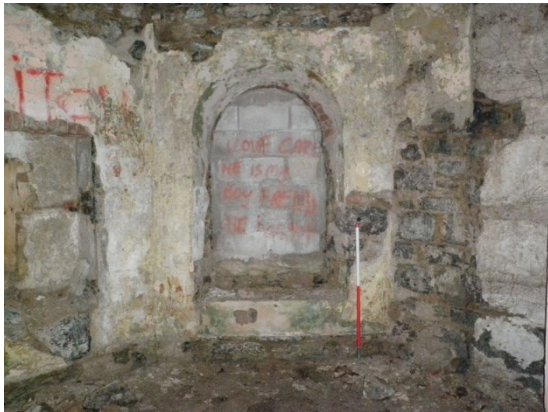
Fig 21 Blocked window in south-west wall of NW lodge.
