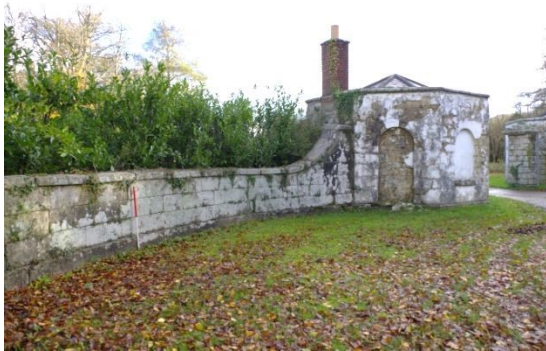
Fig 34 Front (south) elevation of NW flanking wall.
