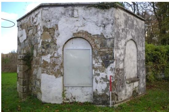
Fig 28 West elevation of SE lodge.
