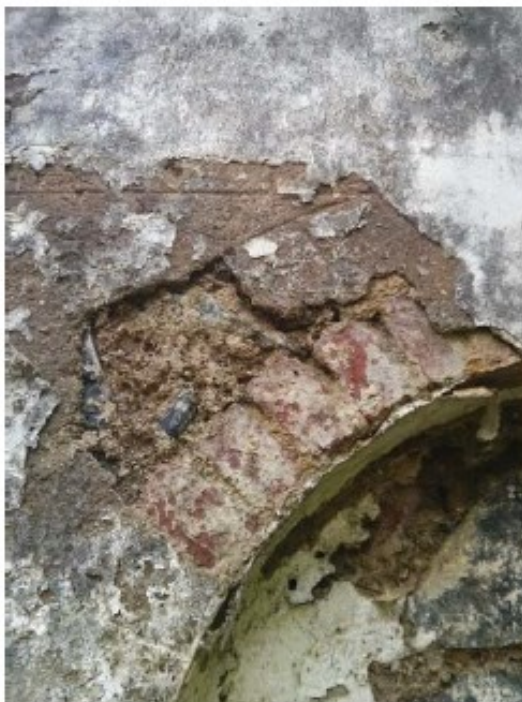
Plate 3: Exposed brickwork to arch, note incised lines in render.
