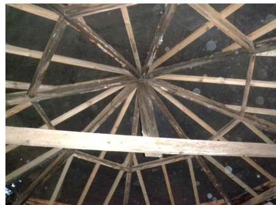
Fig 25 Roof structure in NW lodge.
