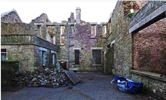
Fig 27 House rear from service yard.
