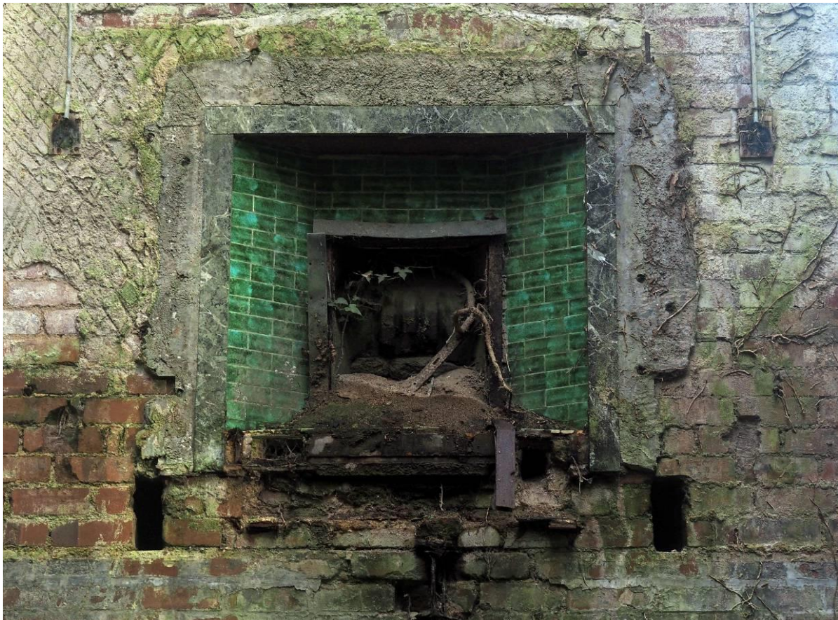
Fig 73 Fireplace within principal bedroom on first floor.
