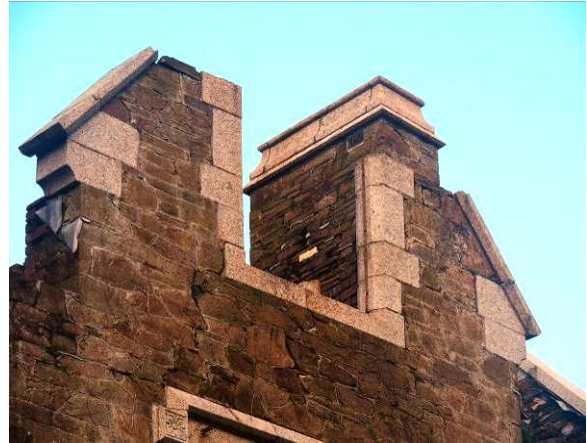
Fig 32 E stack beyond attic gable.
