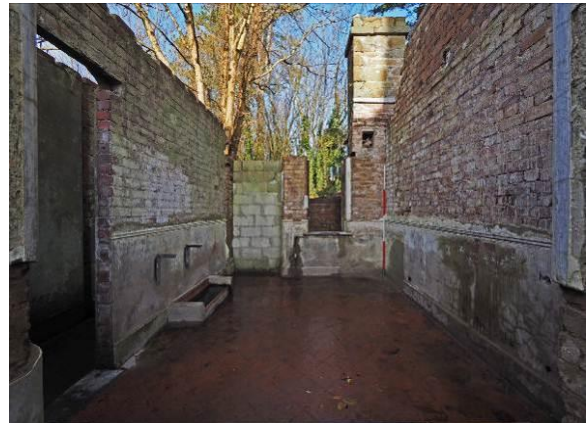
Fig 52 Wash-house from S.
