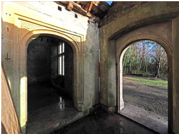
Fig 35 E porch doorways.
