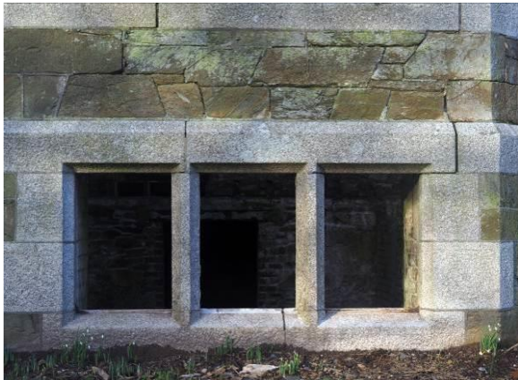
Fig 33 W basement window (iron frame remains).
