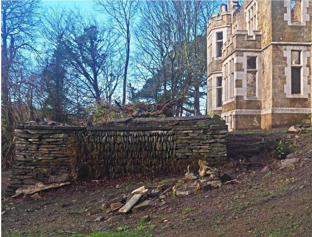
Fig 74 Terrace wall and steps SE of house.
