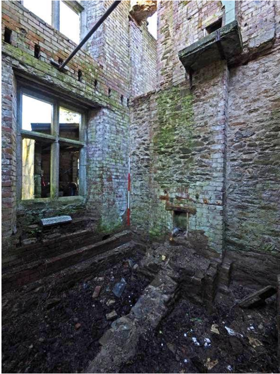
Fig 49 Servants' hall/'sitting room' and chamber above from SE.
