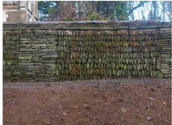
Fig 34 Terrace wall parallel to S elevation.
