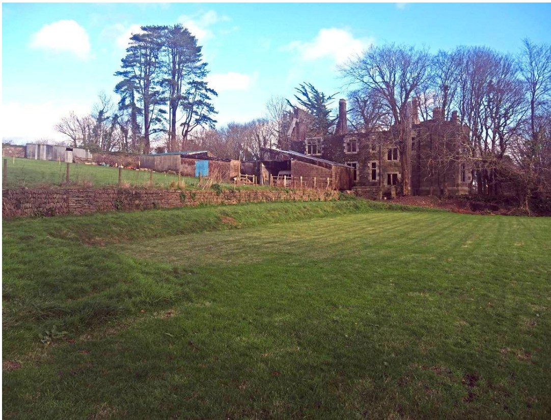
Fig 75 View of Penmadown House from the SW.
