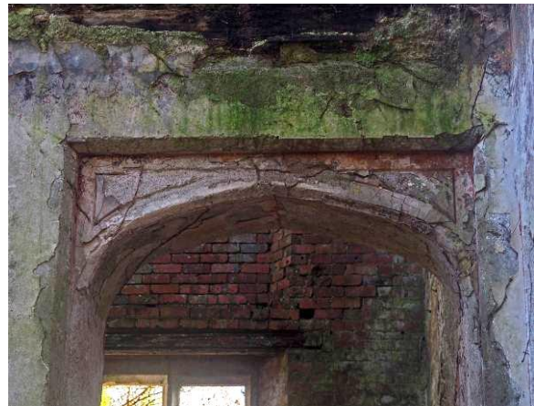
Fig 58 Stair hall E doorway arched head.
