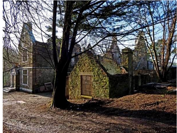
Fig 24 House from NE.
