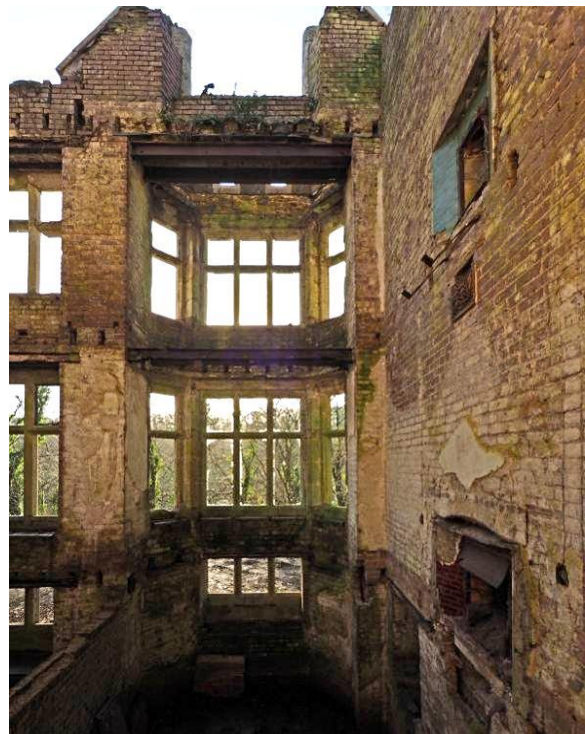
Fig 44 Dining room, chambers + basement to S.
