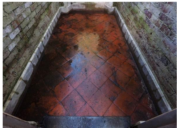
Fig 54 Dairy floor from S.
