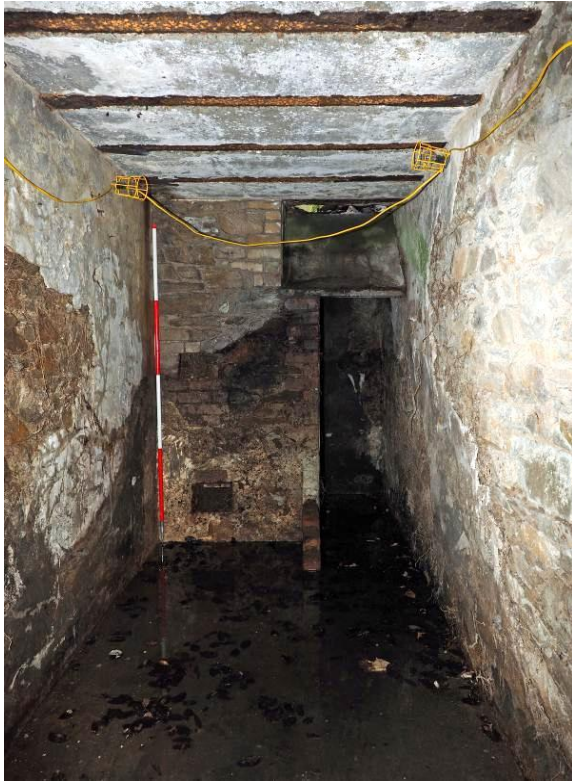
Fig 55 Coal cellar with 2 hatch levels.
