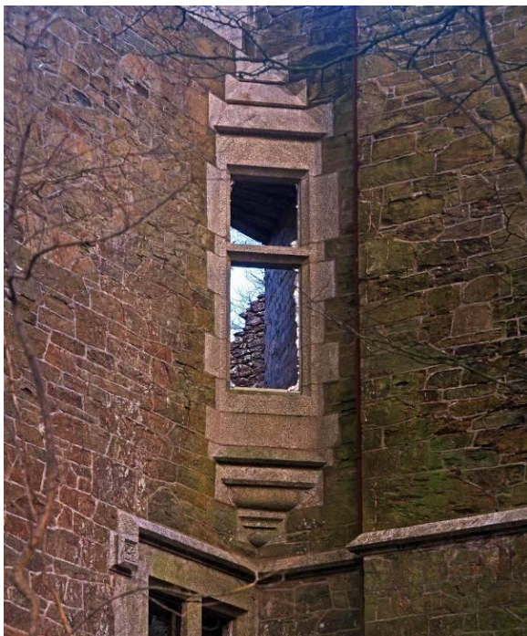
Fig 63 Squint window in SW corner.
