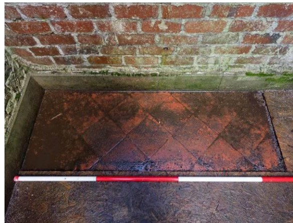
Fig 60 Diamond-pattern tile floor detail.
