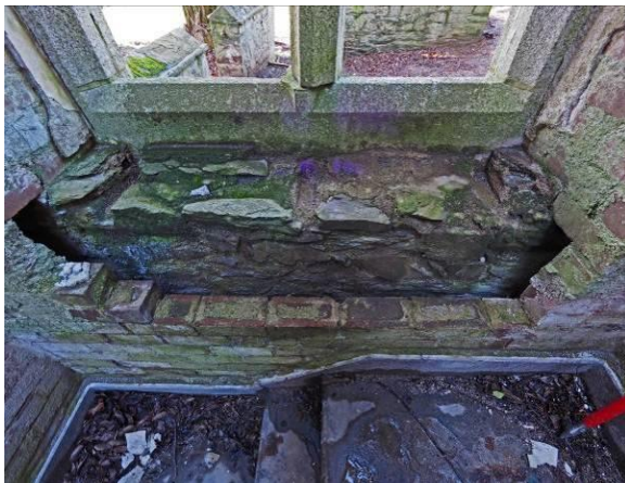
Fig 59 Back stair window and cavity wall.
