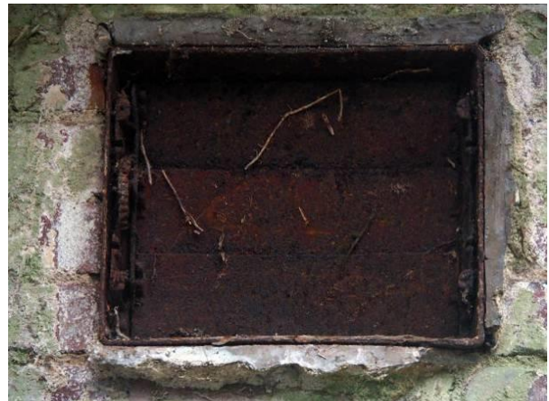
Fig 36 Hall chimney (adjustable flue vent).
