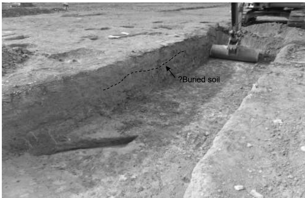
Figure 1. Machine excavation of the trench exposing the deposits, showing the putative buried soil
