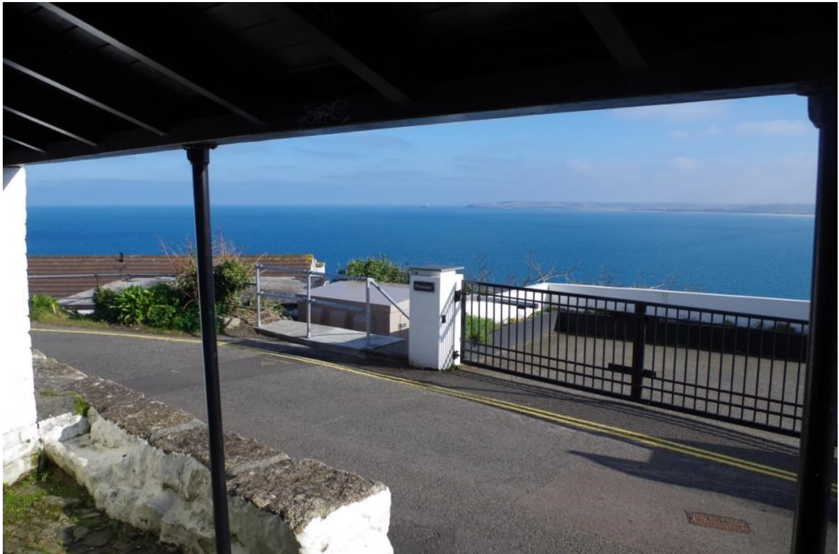
Figure 9: The view northeast across St Ives Bay to Godrevy lighthouse from the southern shelter of the baulking house now includes modern roofs and amenities.
