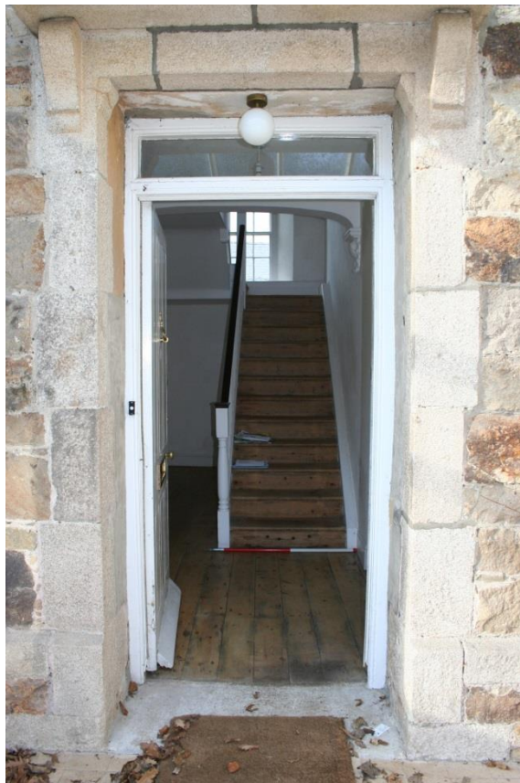
Fig 33 Doorway to the entrance hall and stairs of the Victorian south wing, with distinctive granite surround and good survival of original wood- and plasterwork
