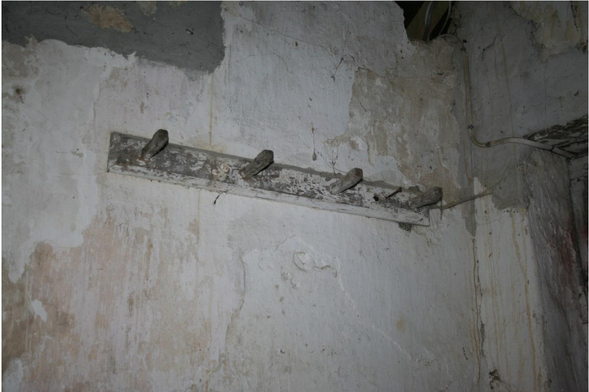
Fig 46 Wooden rack with pegs for horses' bridles or similar tack, fixed on the wall of the Stable passage behind the stalls, at the south (harness room) end of the east wall
