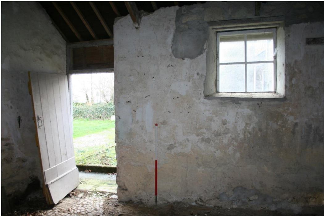
Fig 43 Door on east of Stable, possibly replacing a taller one, and passage with window and peg rack (far right) which gave access to stalls behind and harness room to right
