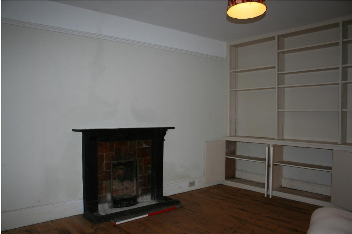
Fig 30 Fireplace, part altered, on the south in the main reception room of c1850. A second doorway probably lies behind the shelving on the west (out of shot)
