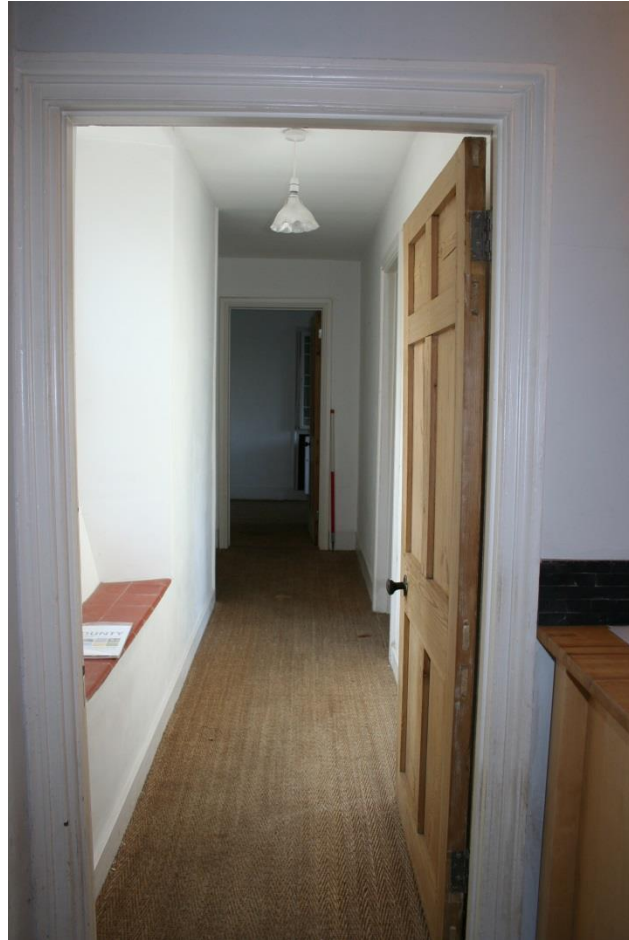
Fig 6 Service passage probably made c1850 inside south front of early house linking Kitchen (foreground) to south wing of that date (opening to left, opposite scale)
