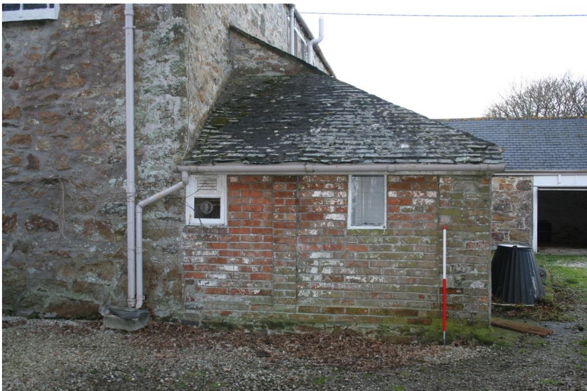
Fig 11 Lean-tos, east side, showing rebuilding in brick probably c1850 from the early Dairy (left of centre) and from the 'flesh house' previously extended around this A 19C window in the eastern bedchamber, probably replacing an early one, can be seen, top left. The Vicar's study, noted in 17C and 18C terriers as over the dairy, may have been so in the sense that it was in the corner of the chamber lit by the window
