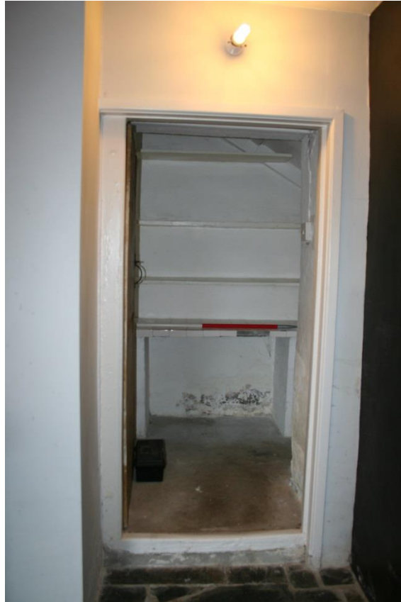
Fig 12 Interior of early Dairy on the north east of the Kitchen, with door and flooring probably of the Victorian phase, and shelving arrangements altered more recently
