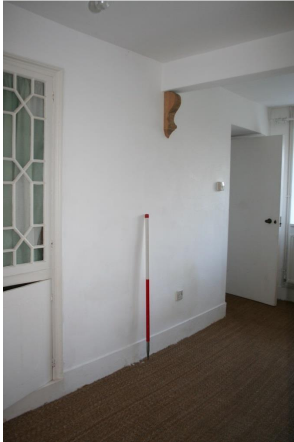
Fig 4 Probable site of a fireplace in the Parlour at the west end of the early house, between a cupboard with 19C glazing, and a modern, inserted doorway
