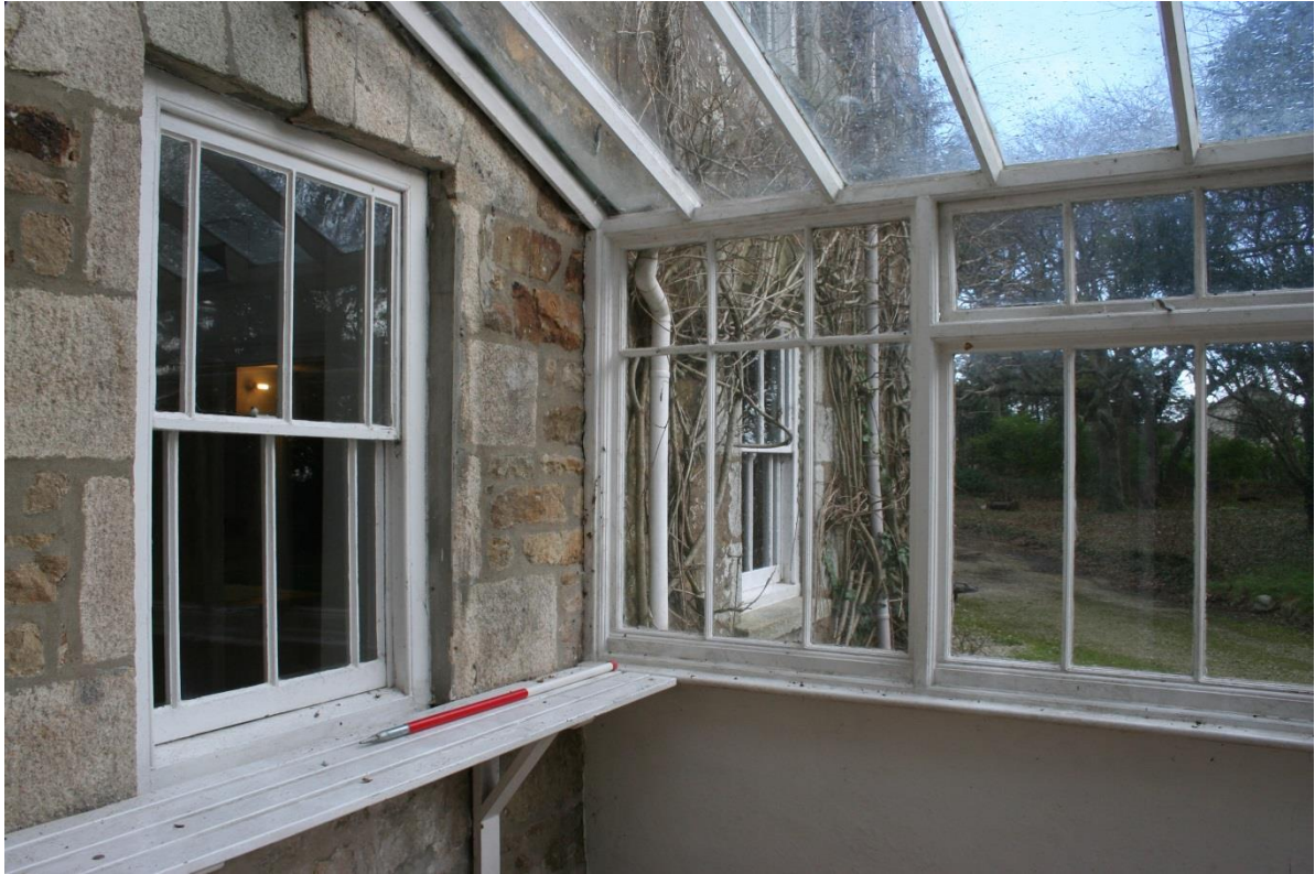
Fig 36 Interior of Conservatory, also showing detail of one of the mid-19C windows, this one lighting the service passage inserted within the south front of the early house
