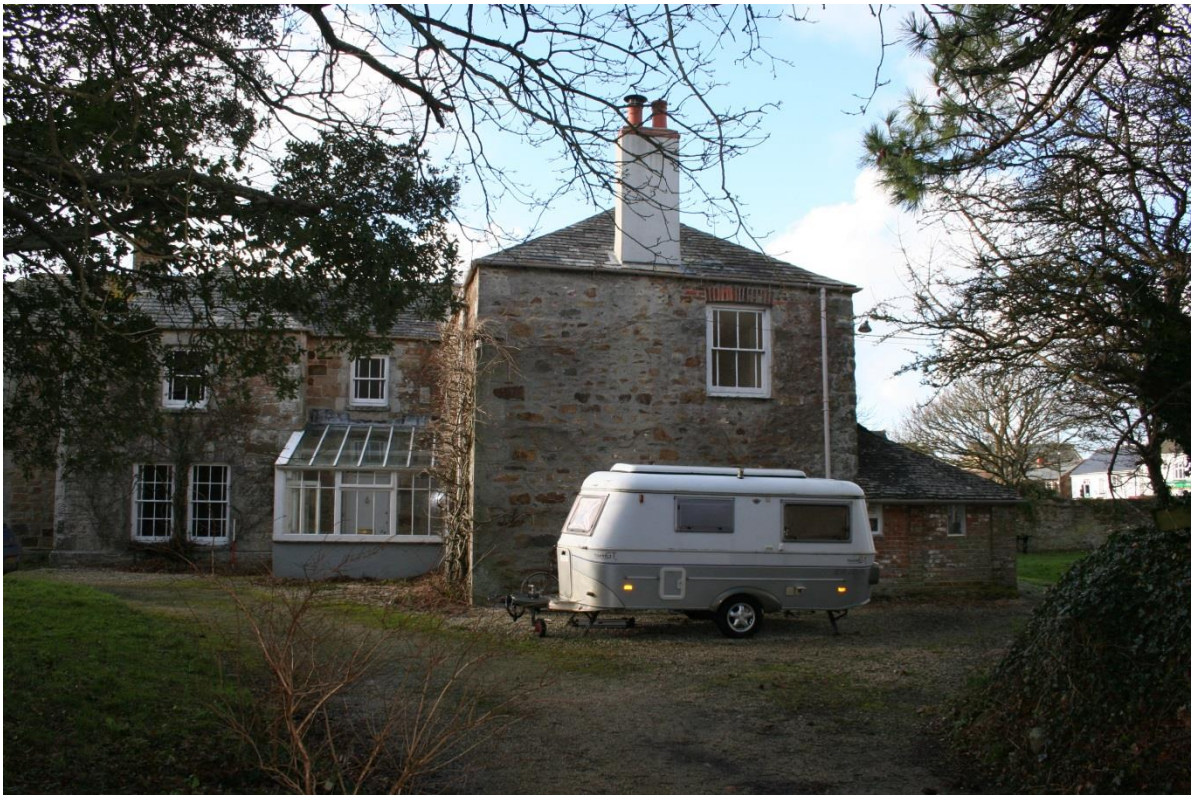
Fig 27 East side, showing how c1850 only some of the style used for the new front, left, and applied to the earlier south front (centre, facing left), was extended to the rear
