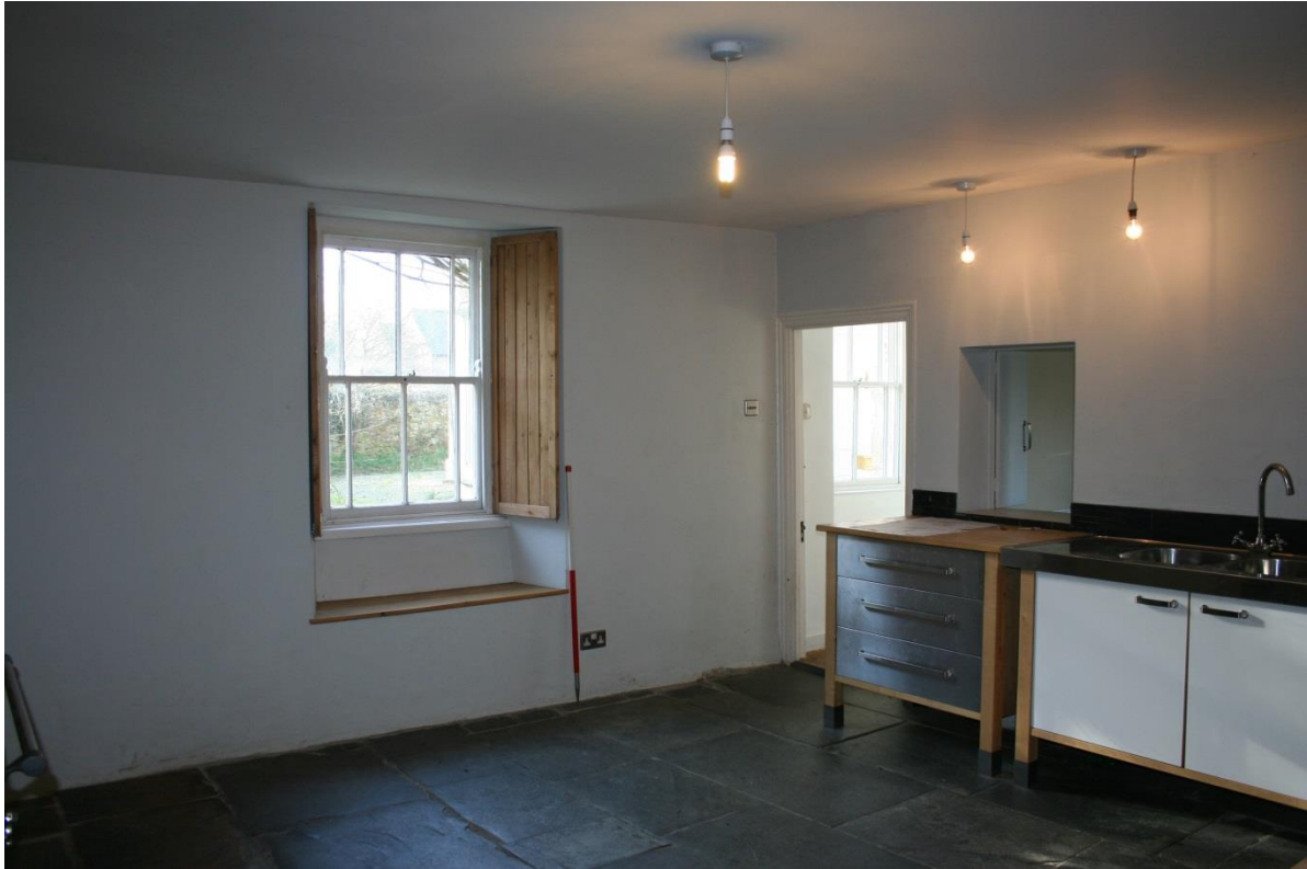
Fig 8 Early Kitchen, with service passage of c1850 beyond, showing south front with windows of c1850, slate floor probably of similar date, and 20C dining room hatch
