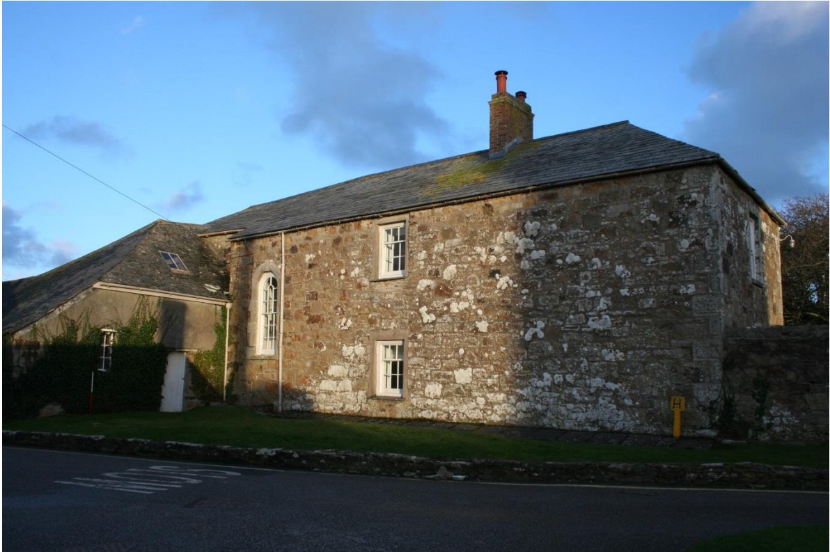
Fig 28 Plainer side of the Victorian wing, facing the churchtown on the west. The Vicar's bedroom was probably that to the south with a window facing the church (right)
