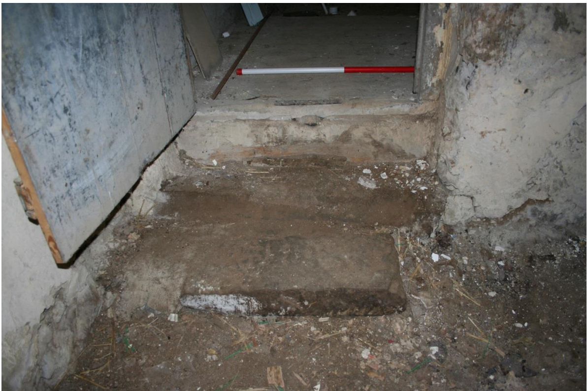
Fig 47 Steps of worked stone, the lower one oddly sized so perhaps re-used, linking the later Stable with the Store on its south, probably its harness room
