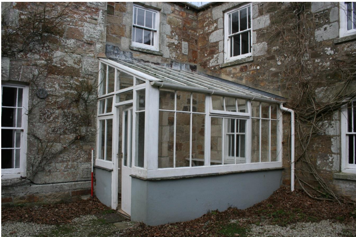
Fig 35 Conservatory at the main entrance, between the early house (right) and the wing of c1850 (left), with some early-mid 20C woodwork and a more recent roof
