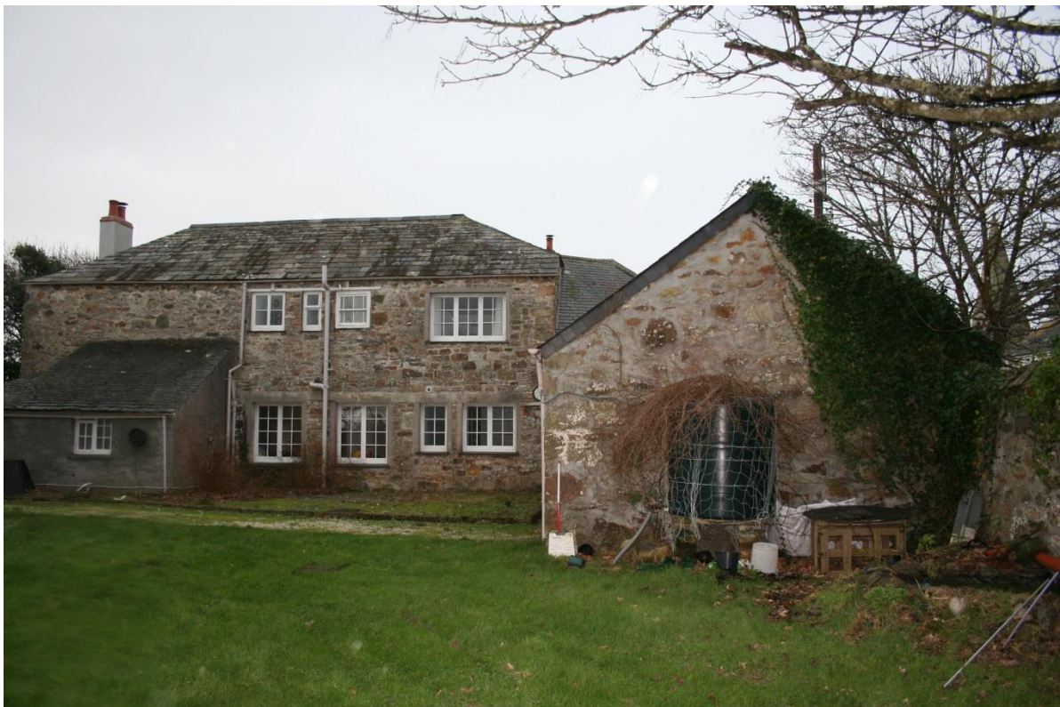
Fig 41 Carriage House and Stable wing and early, east-west range of the house, from the rear (north). Other buildings formerly stood north of the Carriage House (right)
