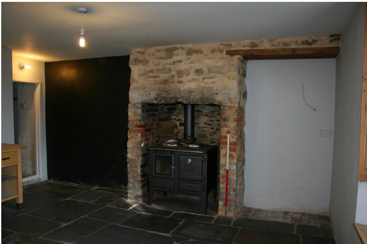
Fig 9 East end of Kitchen with doorway to dairy on north, and fireplace, rebuilt c1850, modified more recently by stripping of plaster and loss of wooden mantel shelf
