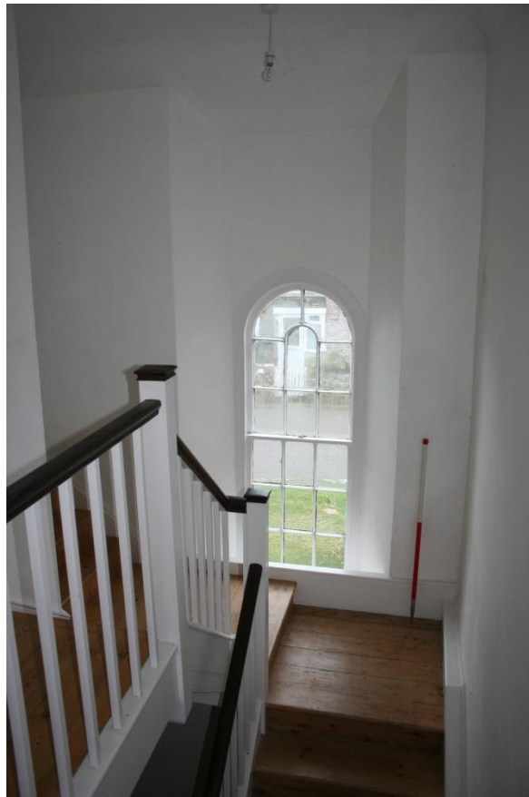
Fig 39 Spacious, well-lit stairway of c1850 rises against the west part of the south front of the early house (right), probably part cob and containing blocked window/s
