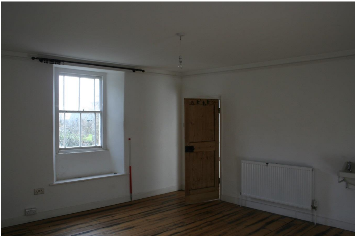
Fig 17 Larger, eastern early bedchamber, probably the Vicar's, showing the south wall rebuilt c1850 with window matching those of the south wing, and mid 20C basin
