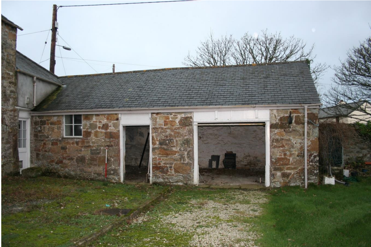
Fig 40 West front of Stable (left) and Carriage House (right) of c1850, with face of local stone resembling that of the contemporary south and east facades of the house
