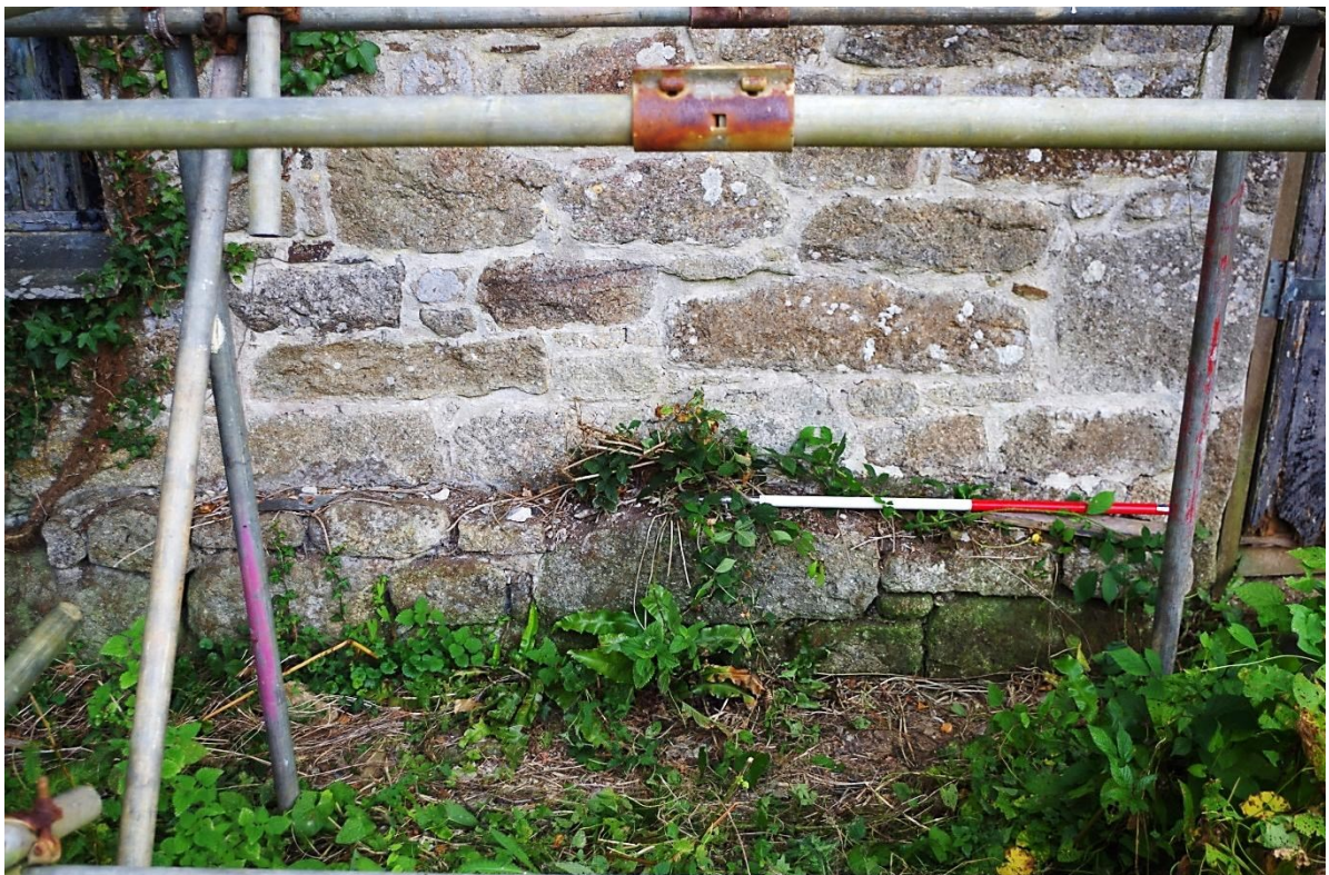
Fig 14 Protruding earlier (phase 1) walling at base of west (front) elevation
