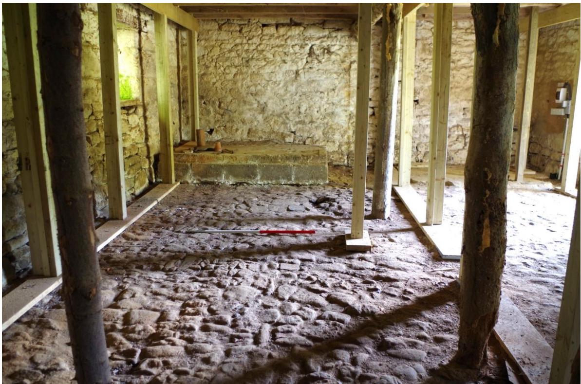
Fig 16 Interior ground floor looking south
