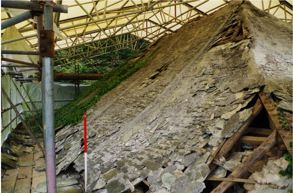
Fig 29 Exterior west side of roof looking north
