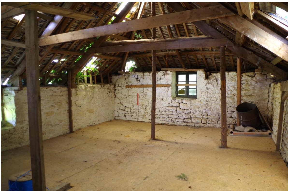
Fig 24 First floor looking north
