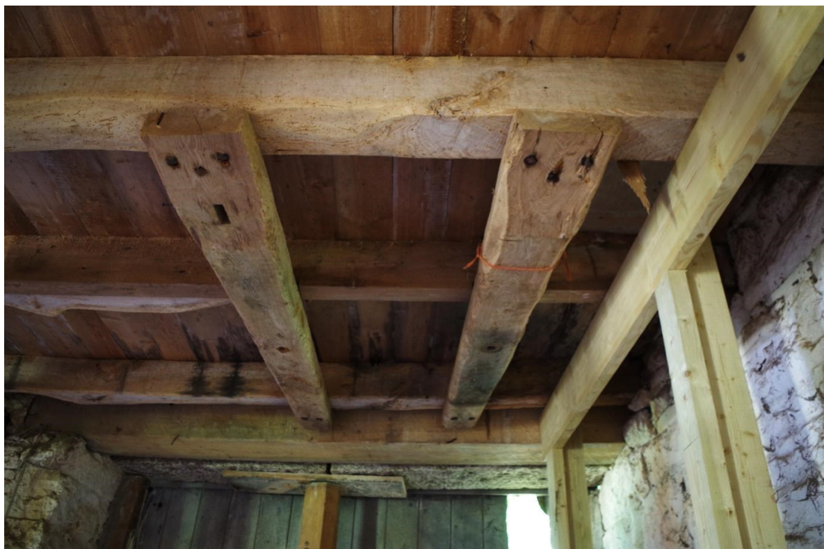
Fig 20 Cider press support timbers attached to joists in north-east corner of ground floor
