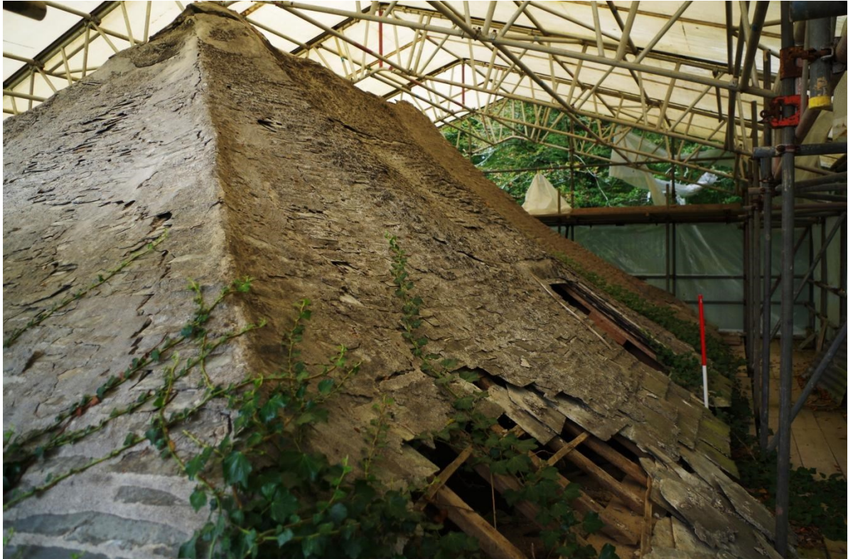
Fig 27 Exterior east side of roof looking north
