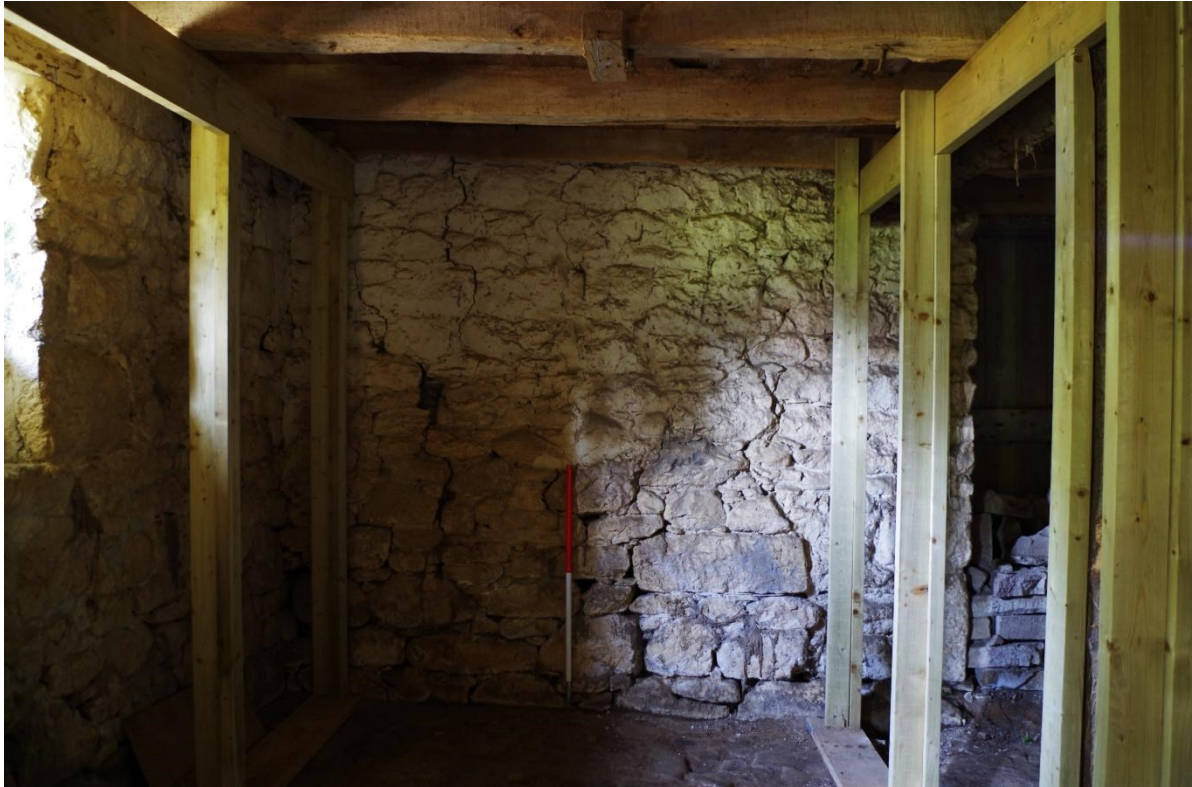
Fig 17 Interior ground floor north wall showing rebuilt door jamb
