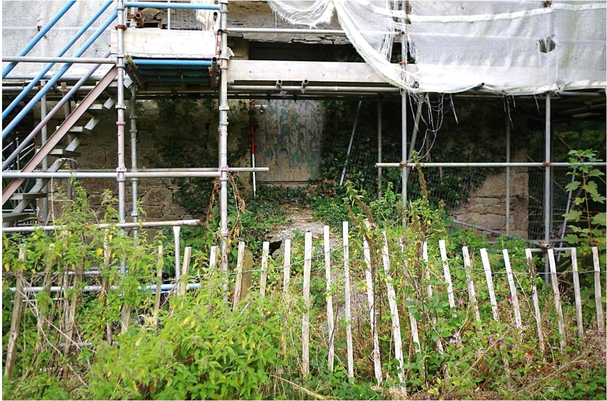
Fig 11 Exterior south elevation
