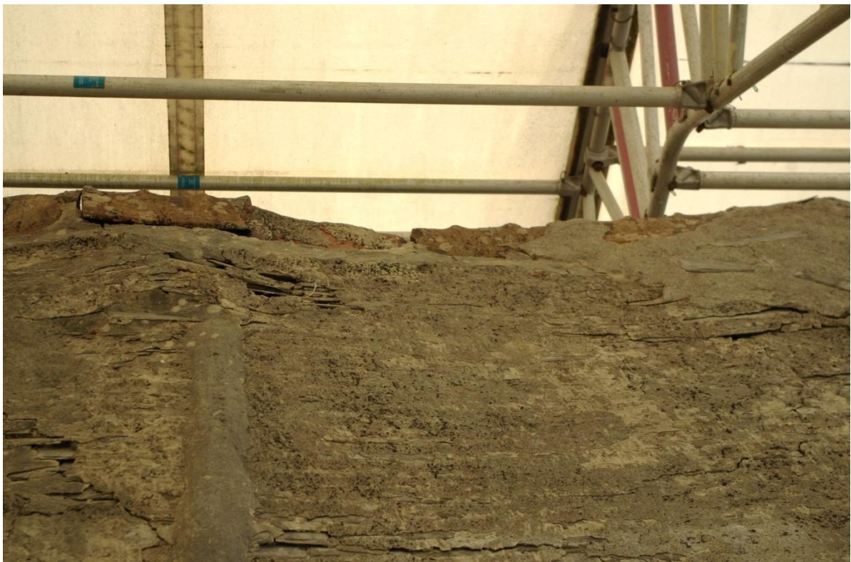
Fig 30 Crested ridge tiles viewed from west side of roof
