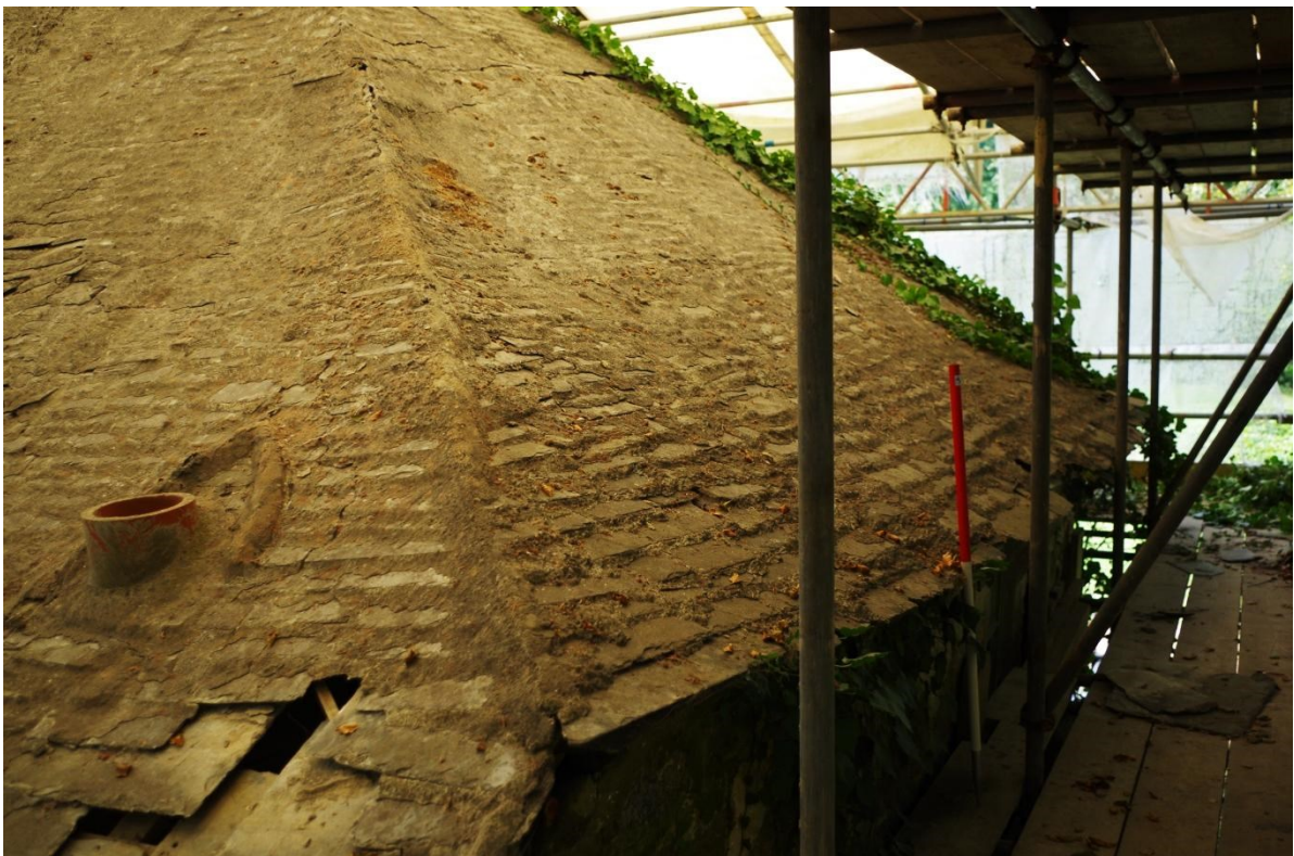
Fig 26 Exterior north end of roof looking west
