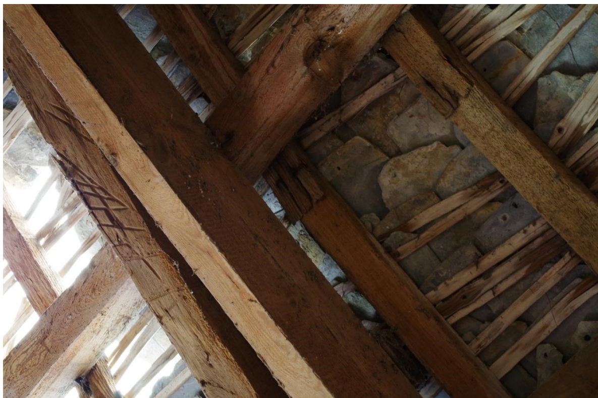
Fig 33 Carpenter's marks on early truss timber
