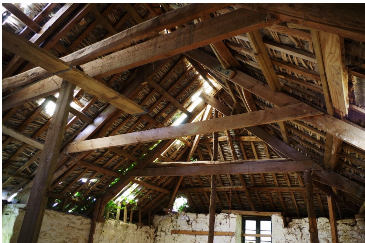
Fig 32 Roof structure looking north
