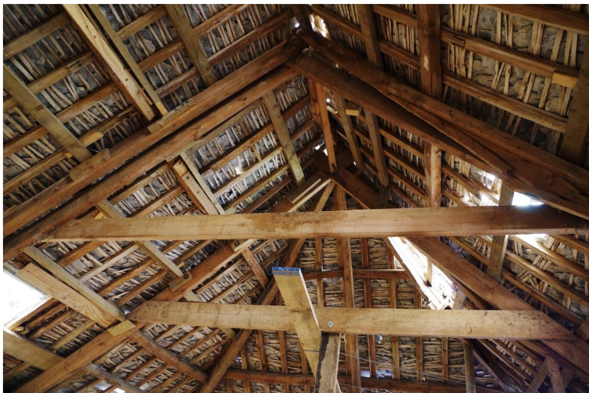
Fig 31 Roof structure looking south
