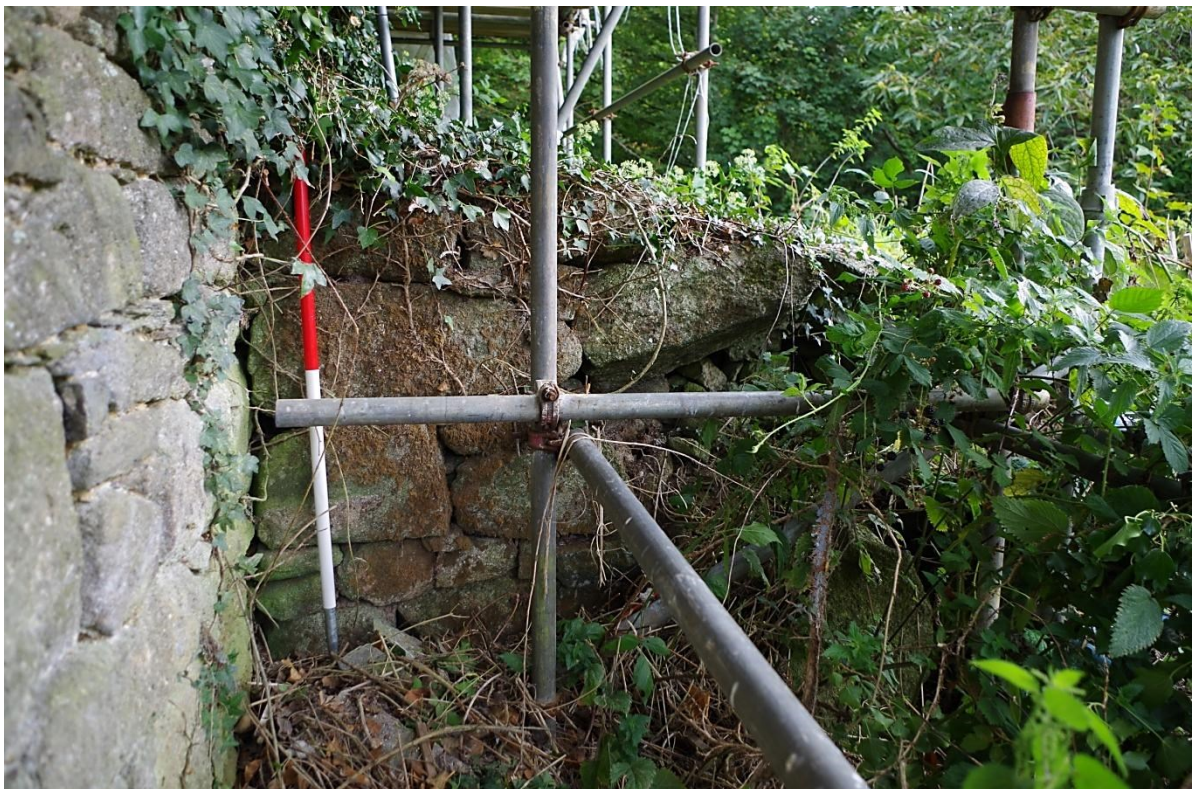
Fig 12 west elevation of ramp (former steps) on south side of building
