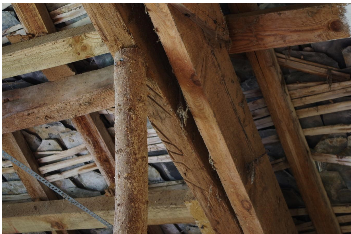
Fig 34 Carpenter's marks on early truss timber
