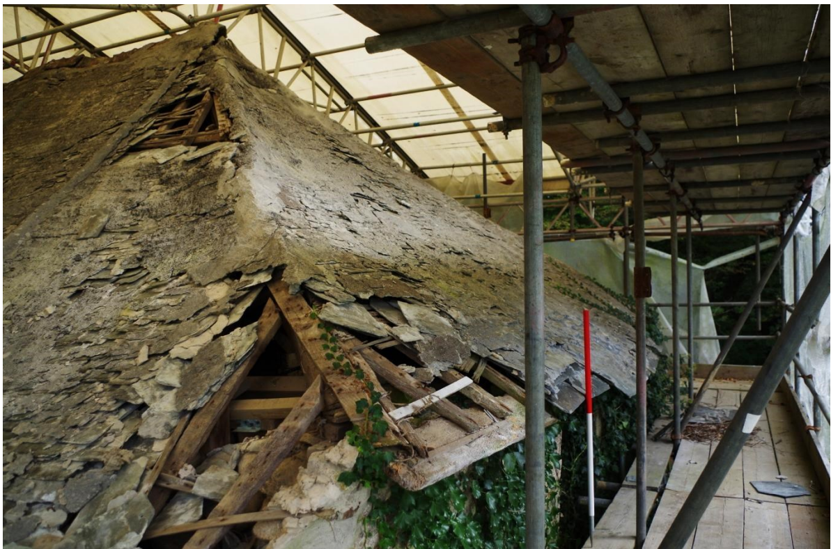
Fig 28 Exterior south end of roof looking east
