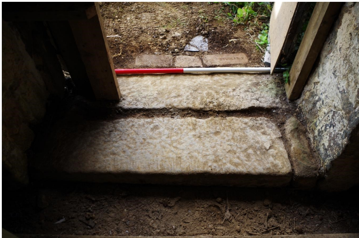
Fig 19 Granite threshold in west, ground floor door opening
