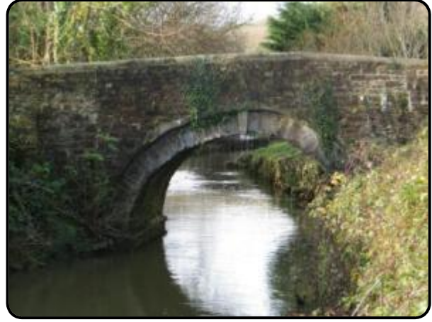
Canal bridge, Marhamchurch.
