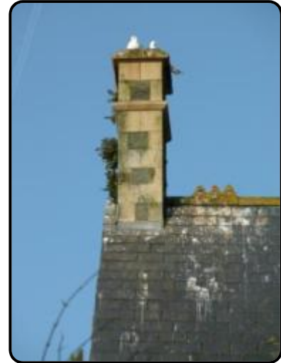
Figure 11 Vegetation and roosting seagulls on chimney.
