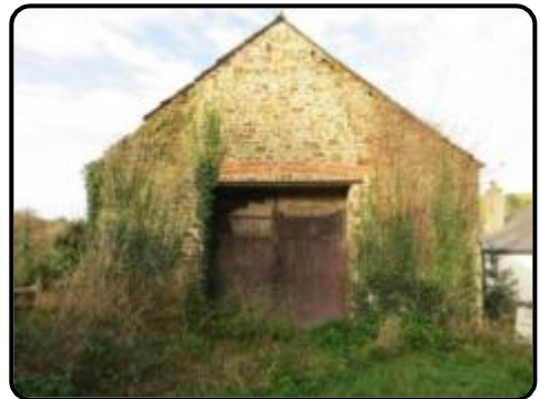
Former mid 19th century iron foundry, Marhamchurch.
