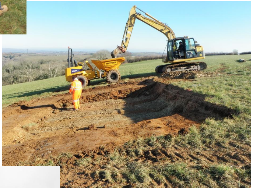
Fig10 (Right) The turbine footprint at the completion of topsoil stripping.
