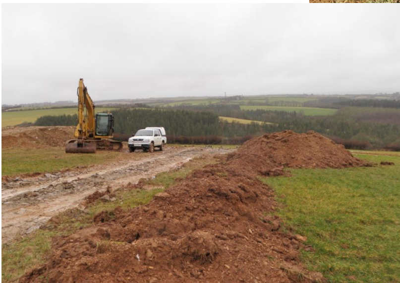
Fig 11 (Left) The temporary access track as it approached the turbine.
