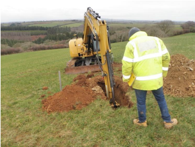
Fig 9 (Left) Geotechnical pit 1 being excavated.
