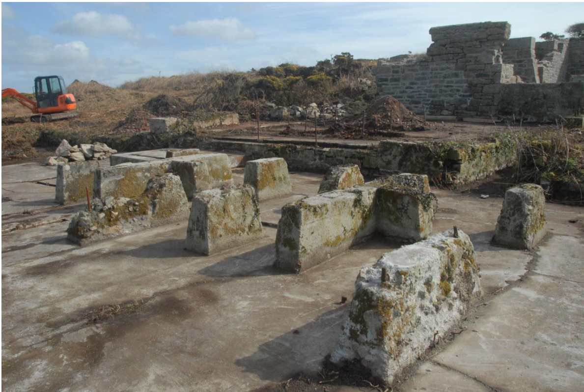
Fig 12. The Pinder Table floor in the mill. The poor condition of the concrete from which some of the plinths had been constructed is clearly evident.
