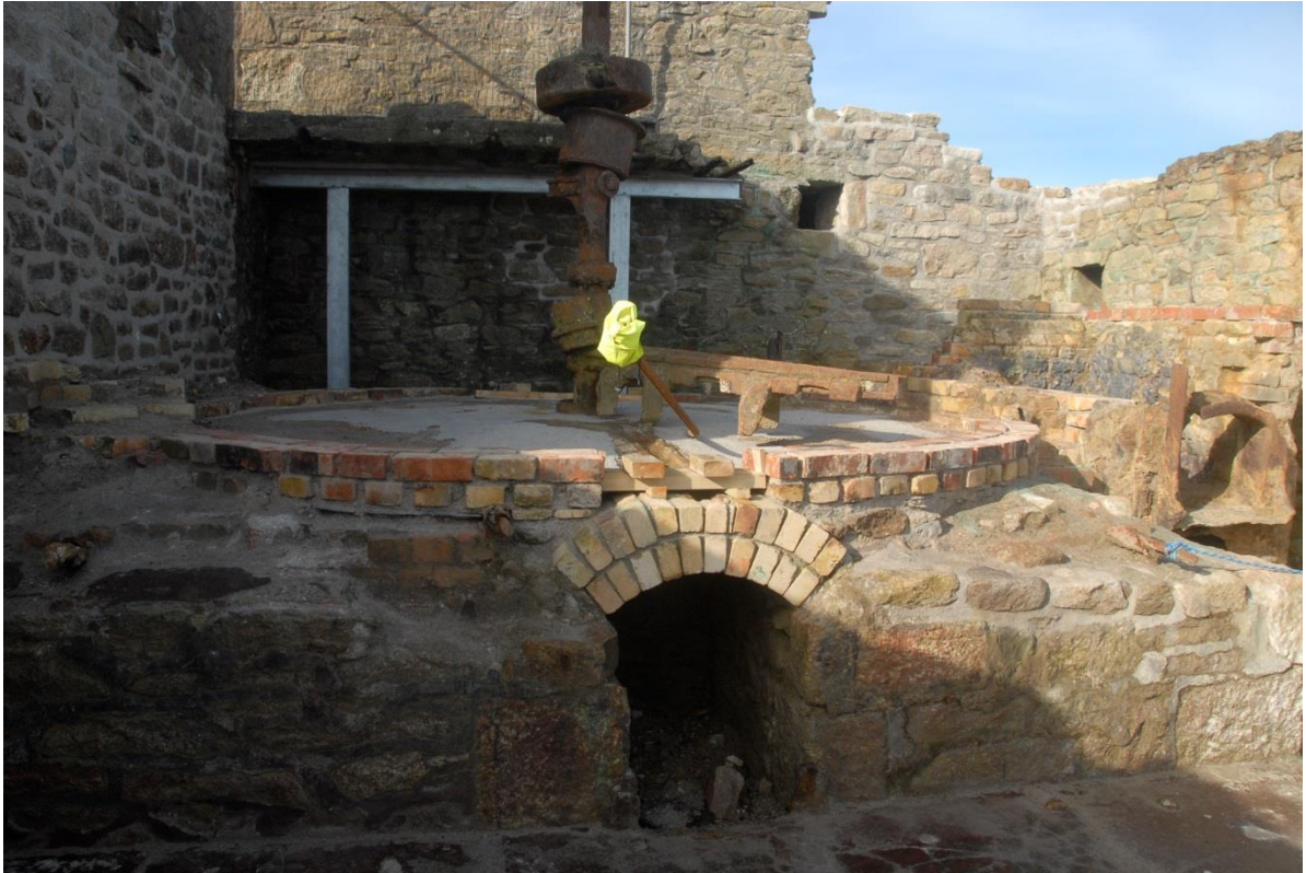
Fig 69. The reconstructed brickwork around the base of the calciner bed and over the discharge vault and (background) the replacement steelwork support to the walkway which formerly accessed the calciner feed hopper.
