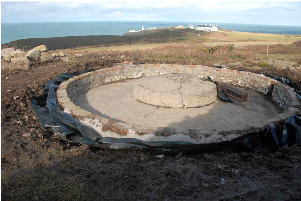
Fig 76. The geotextile root barrier in place in the trench around the northern buddle. This was subsequently backfilled with an inert gravelly material.
