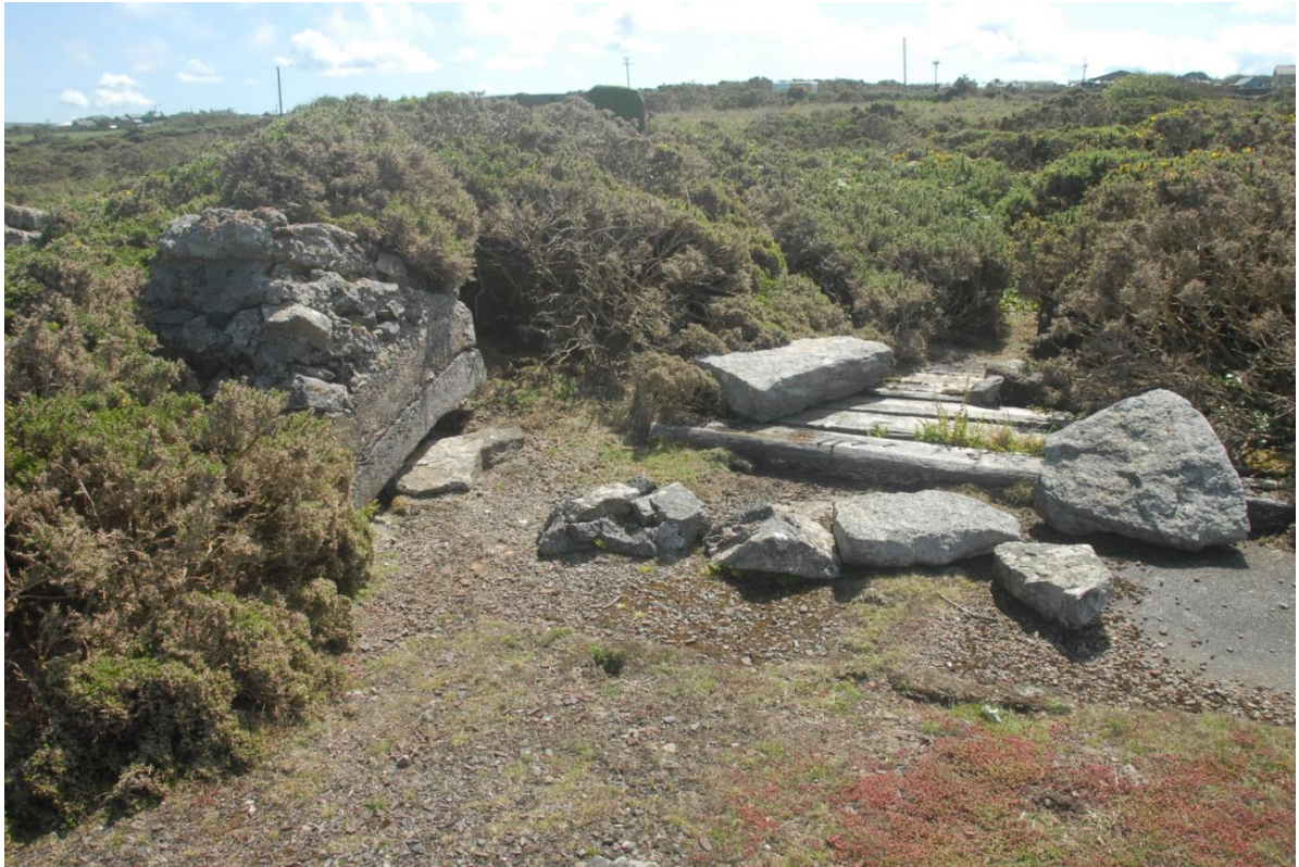
Fig 16. Trease Shaft prior to the clearance of the gorse which had encroached on it. The shaft is open to water at a depth of about 10m under the timber sleepers.
