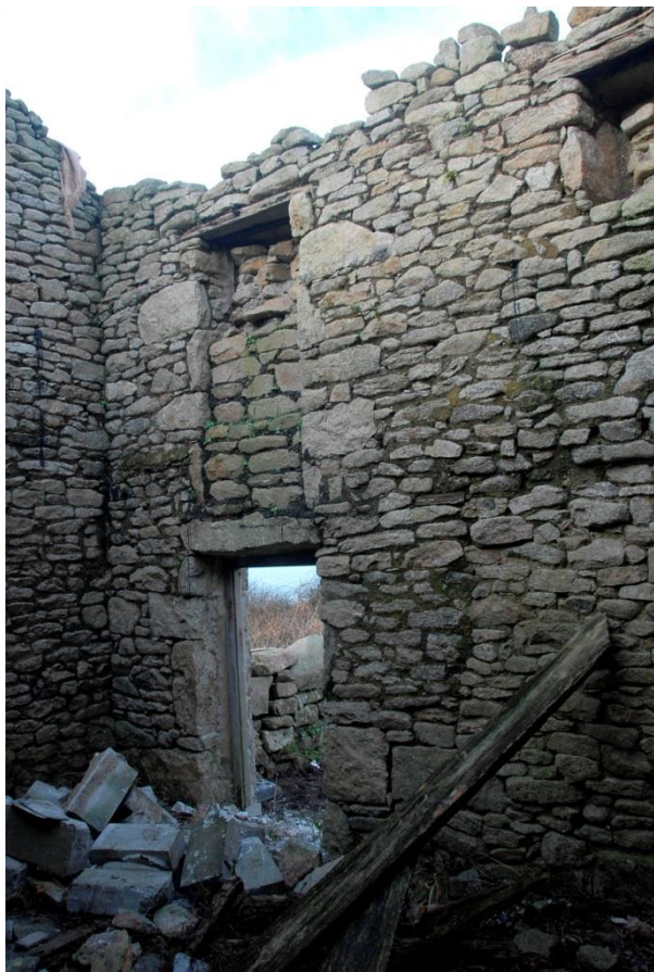
Fig 28. An early stage in the conservation works to the field barn.
