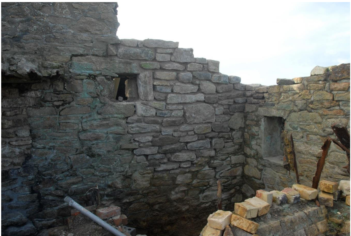
Fig 55. The reinstated masonry forming the eastern wall of the northern dust chamber, incorporating the reconstructed flue opening.
