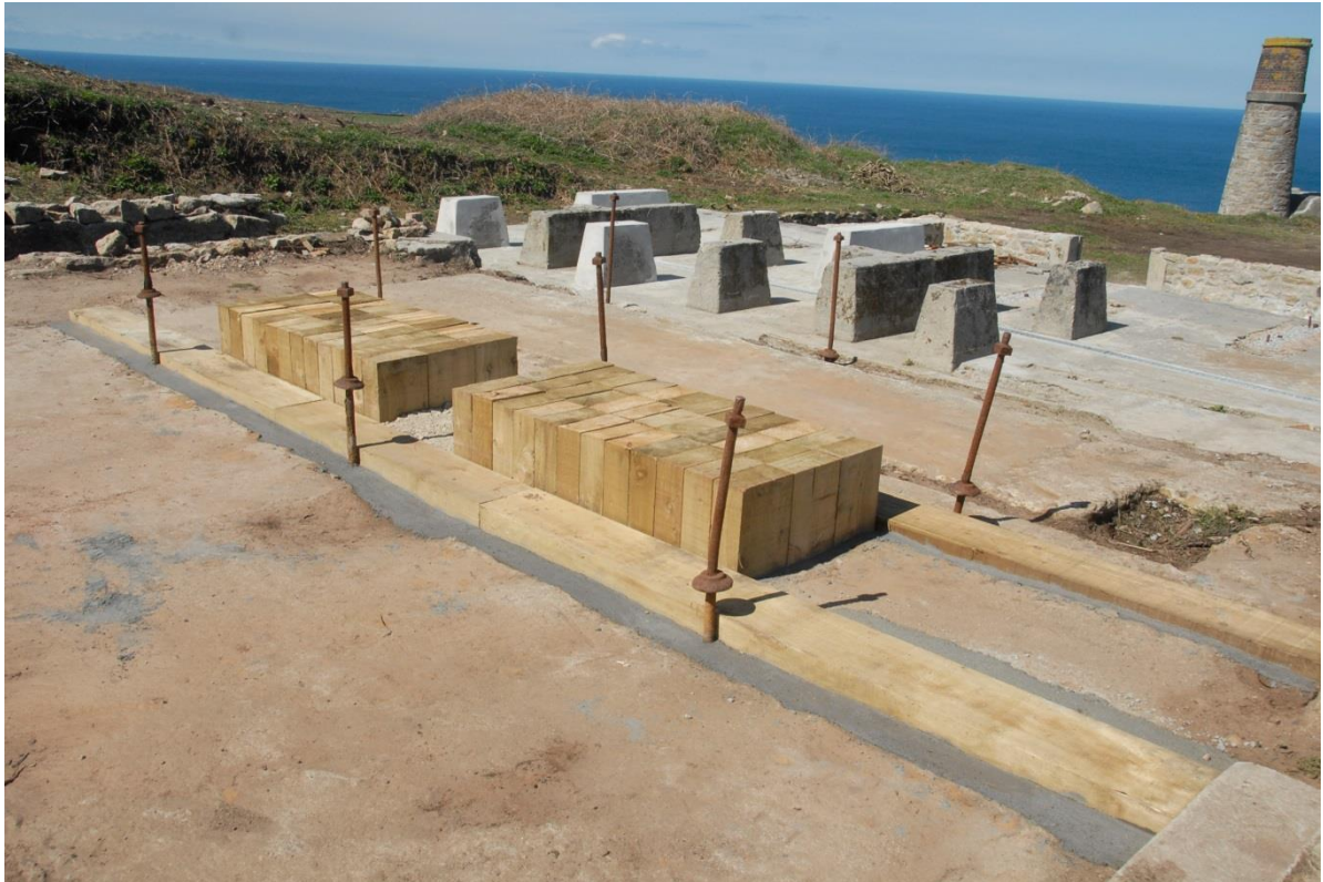
Fig 50. The completed reproduction anvil support timbers and mud cills. The infill concrete next to the mud cills is deliberately darker than the original to distinguish the new work from the old.
