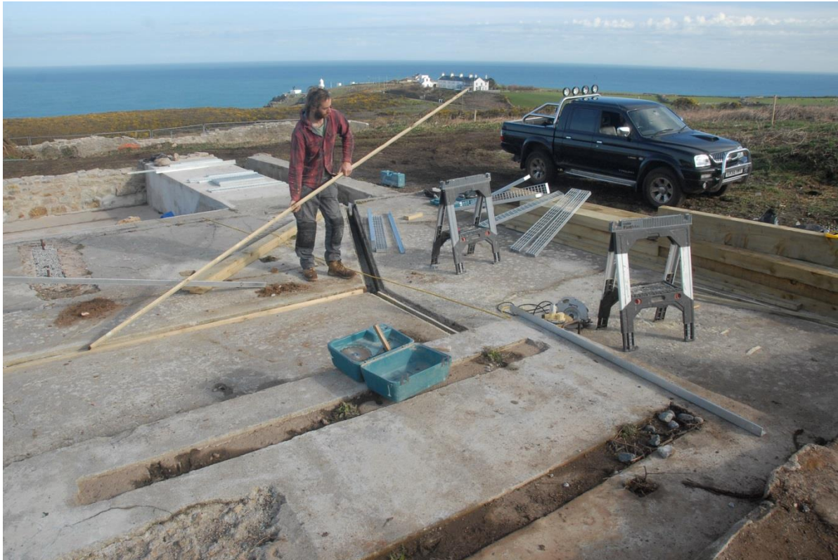
Fig 46. Preparing the timber linings to support the grilles over the mill floor drains.
