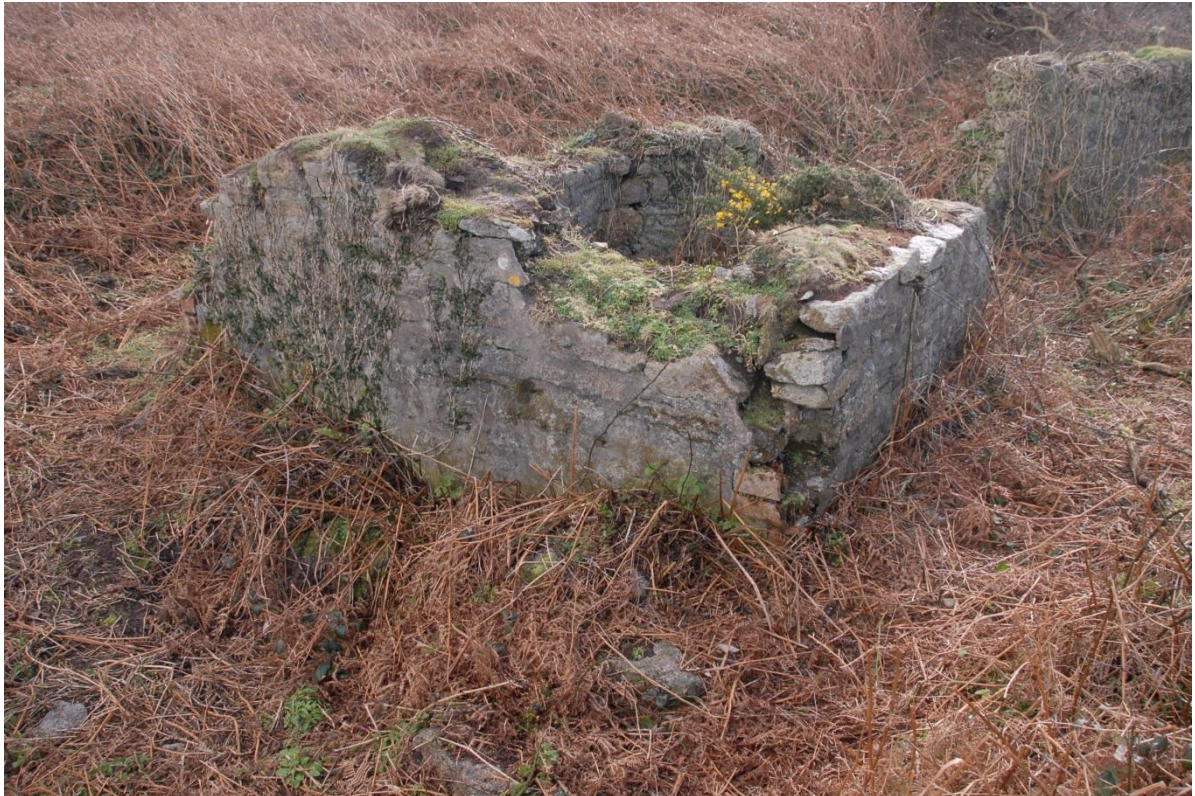
Fig 79. The probable powder house from the north east prior to works, showing the poor state of its masonry at this time.
