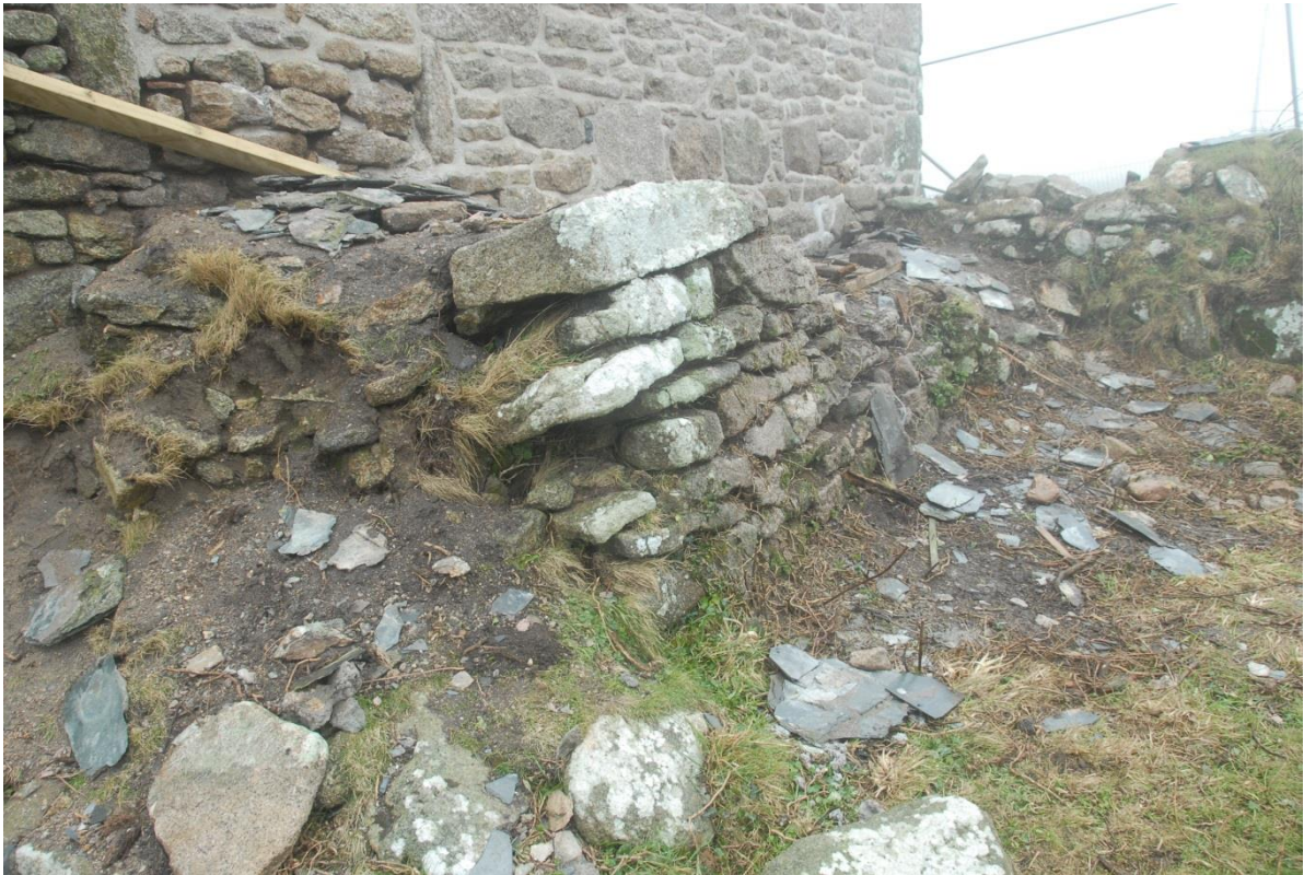
Fig 30. The poor condition of the ramp which formerly gave access to the upper floor of the field barn.
