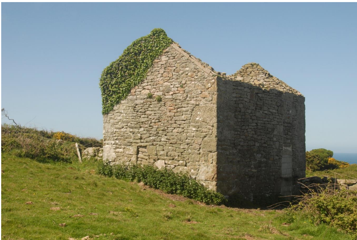
Fig 15. Trease field barn from the north-east, showing the blocked windows and door in these elevations.
