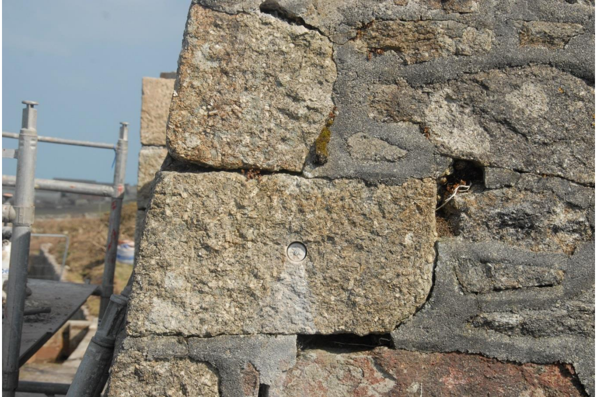
Fig 64. The only visible evidence for the Cintec reinforcing bars installed into the northern dust chamber wall (centre).
