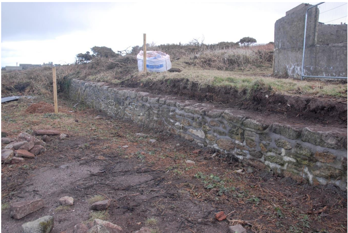
Fig 78. Completed works to the revetment wall linking the tin floors to the probable powder house.
