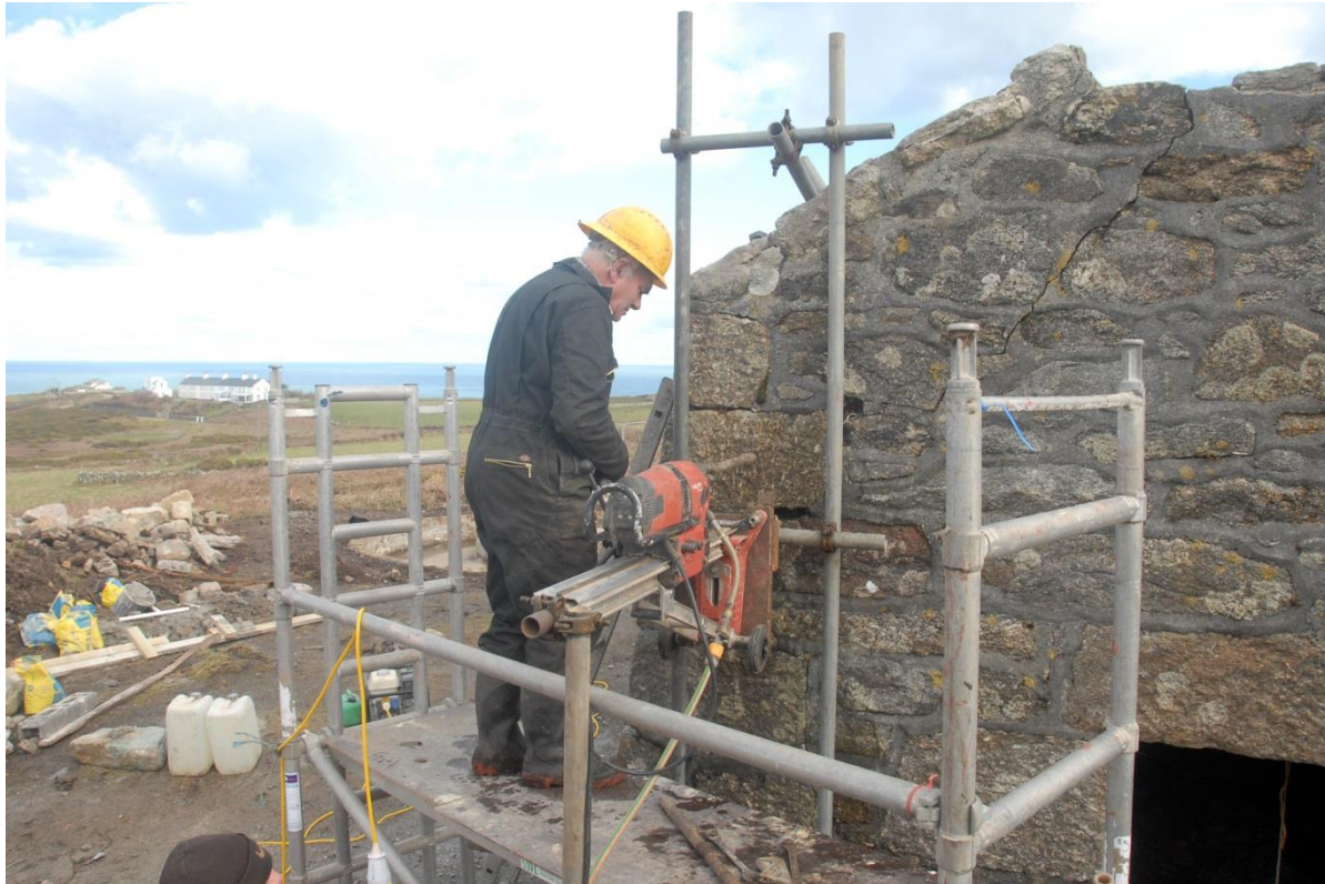
Fig 62. Drilling the five metre horizontal hole near the head of the dust chamber northern wall which would take one of the Cintec reinforcing bars.
