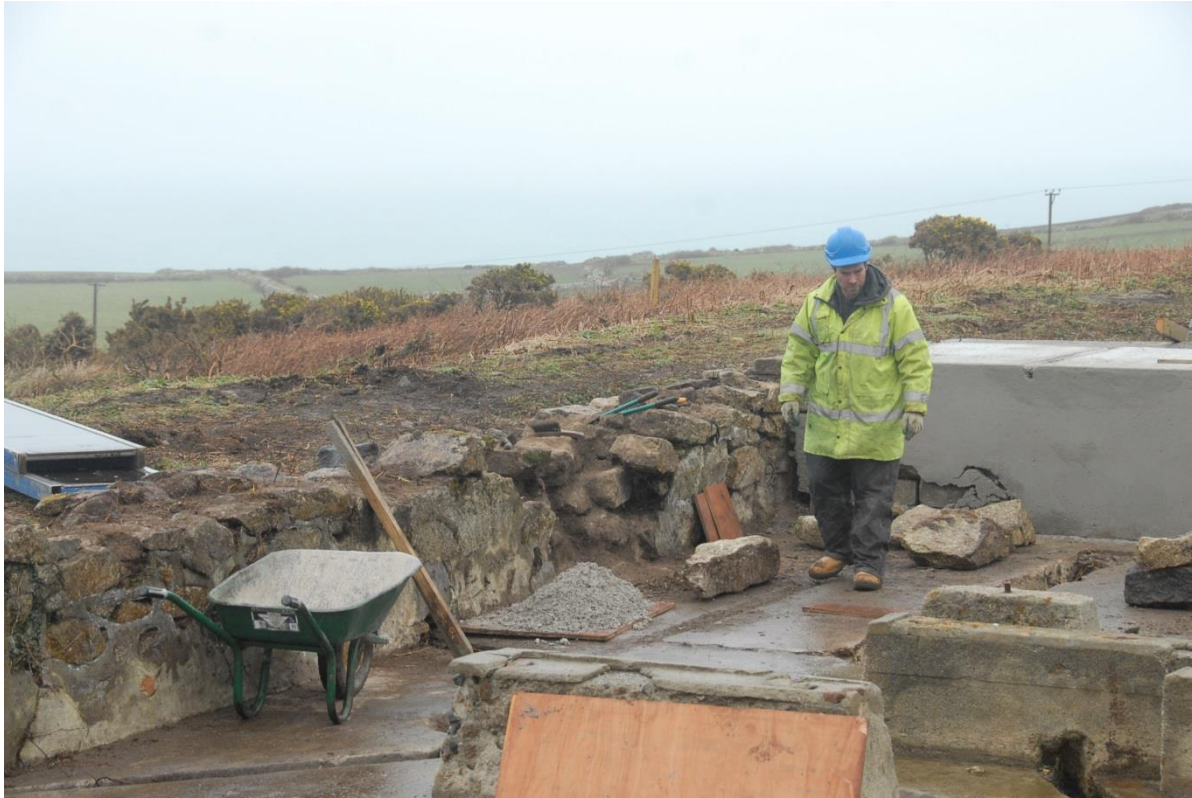
Fig 44. Work in progress during the repair of the walling around the lower mill floor.
