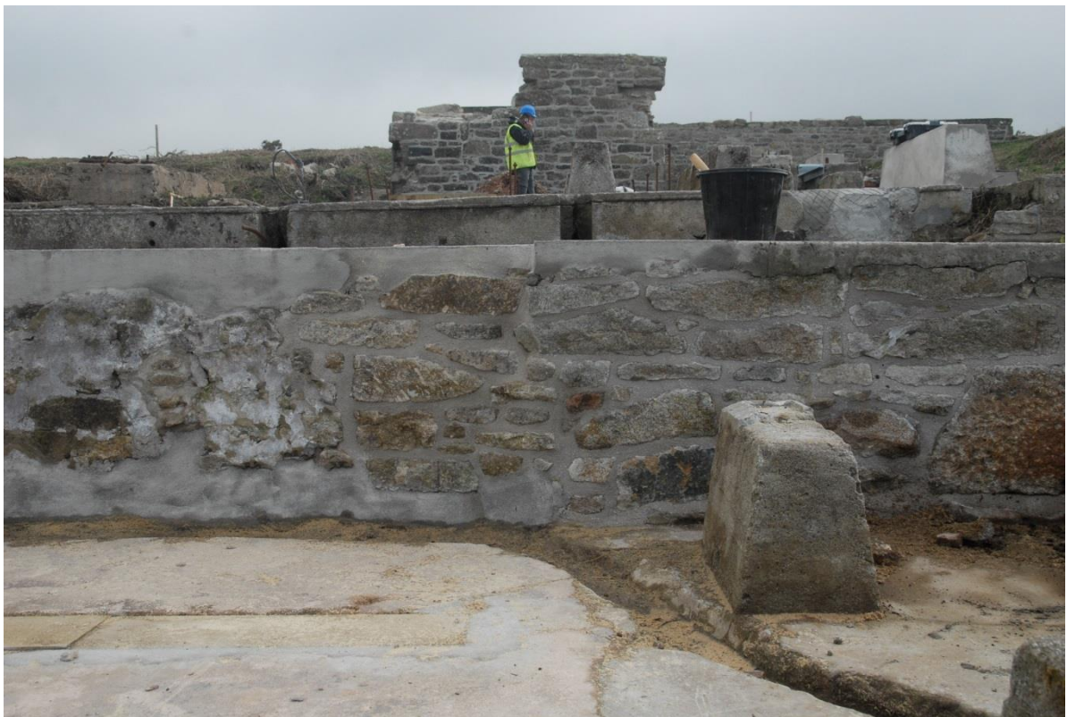
Fig 39. The completed repair works to the mill walling.
