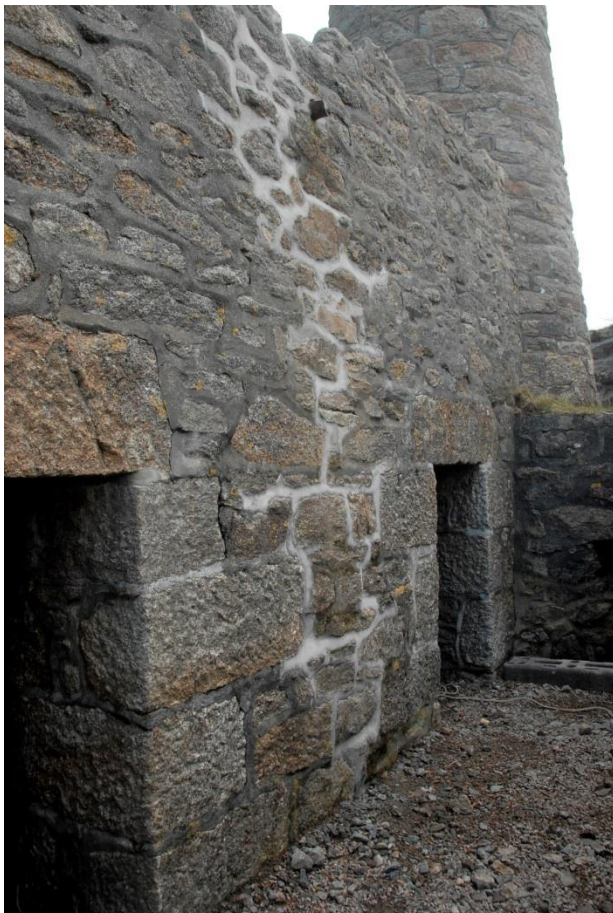
Fig 56. Repointing the lower section of the southern wall of the calciner enclosure in lime mortar. The upper section of the wall, which includes the location of the end of a feed hopper (top centre), was repointed in a cement mix to match the surrounding mortar.
