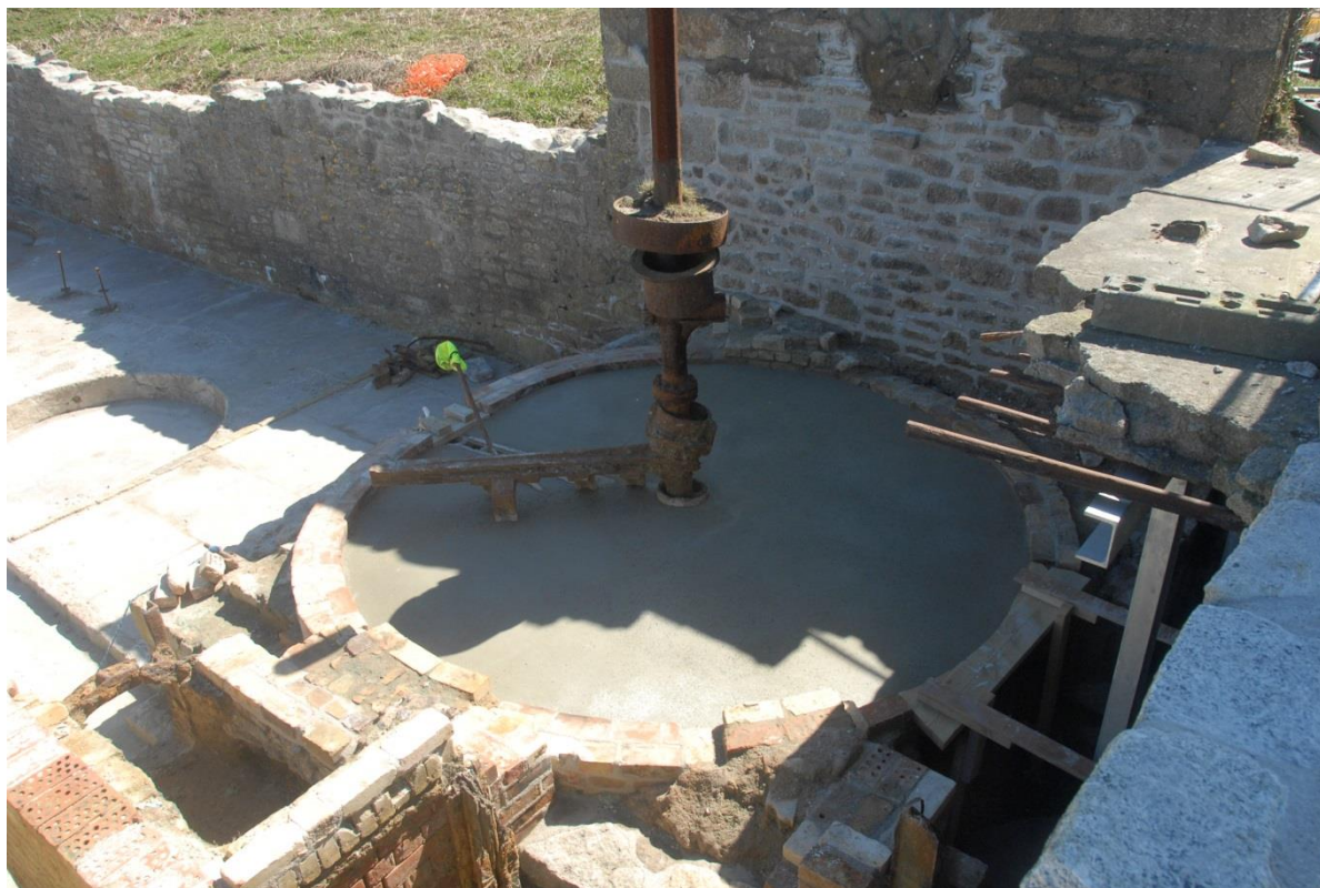
Fig 73. The completed Paverok screed to the calciner bed.
