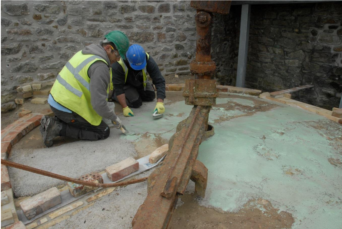
Fig 71. Applying the Nitocote bonding primer to the calciner bed.
