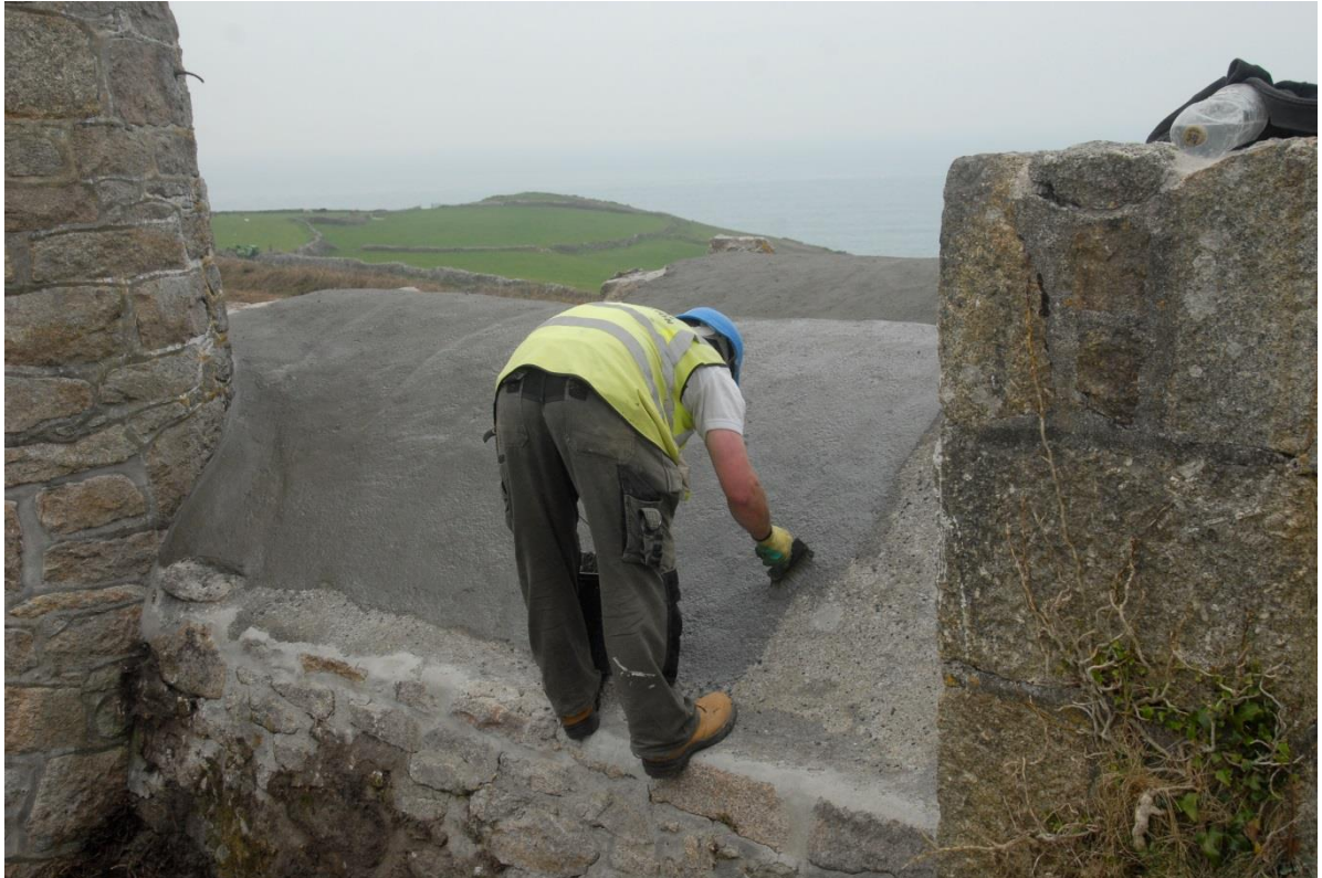
Fig 61. Applying the Fosrok Brushbond to the dust chamber roofs.
