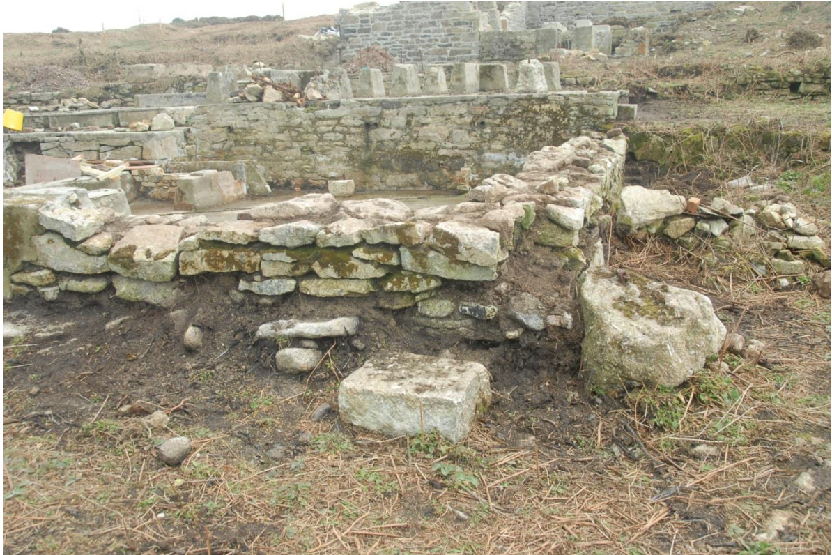
Fig 42. The very poor state of the walling which supported the lower section of the Trease mill building prior to works.
