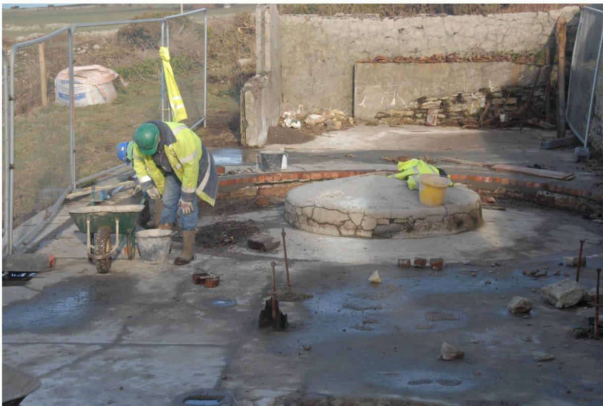
Fig 53. Work in progress during the repair works to the buddle on the tin floors.
