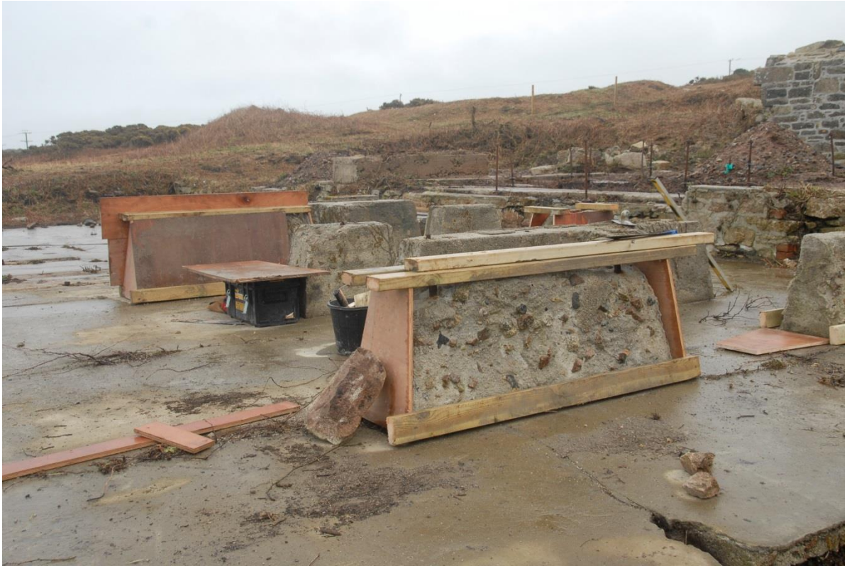
Fig 34. Formwork in place around the most decayed of the Pinder Table mountings on the middle mill floor.
