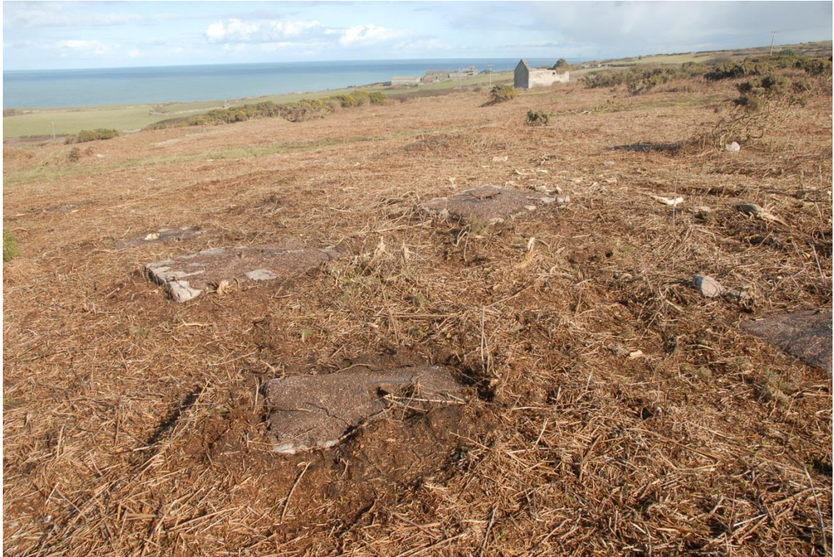
Fig 20. The concrete pads for the tramway from Trease Shaft to the mill exposed during site clearance.
