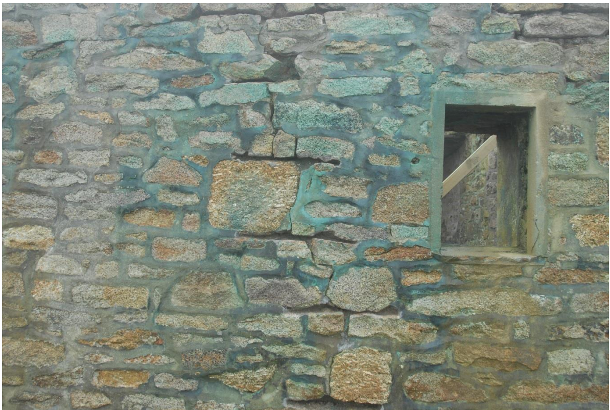
Fig 65. Joints crossing a vertical crack in the calciner enclosure northern wall cut out to receive helicoil bedjoint reinforcement.
