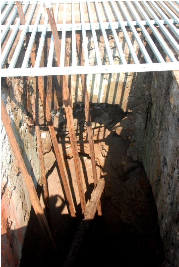
Fig 84. Manoeuvring the first section of the new steel grille onto Trease Shaft once the sleeper cap had been partly removed.
