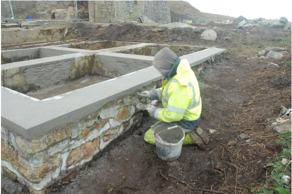
Fig 77. The completion of the works to the precipitation tanks to the north of the tin floors.
