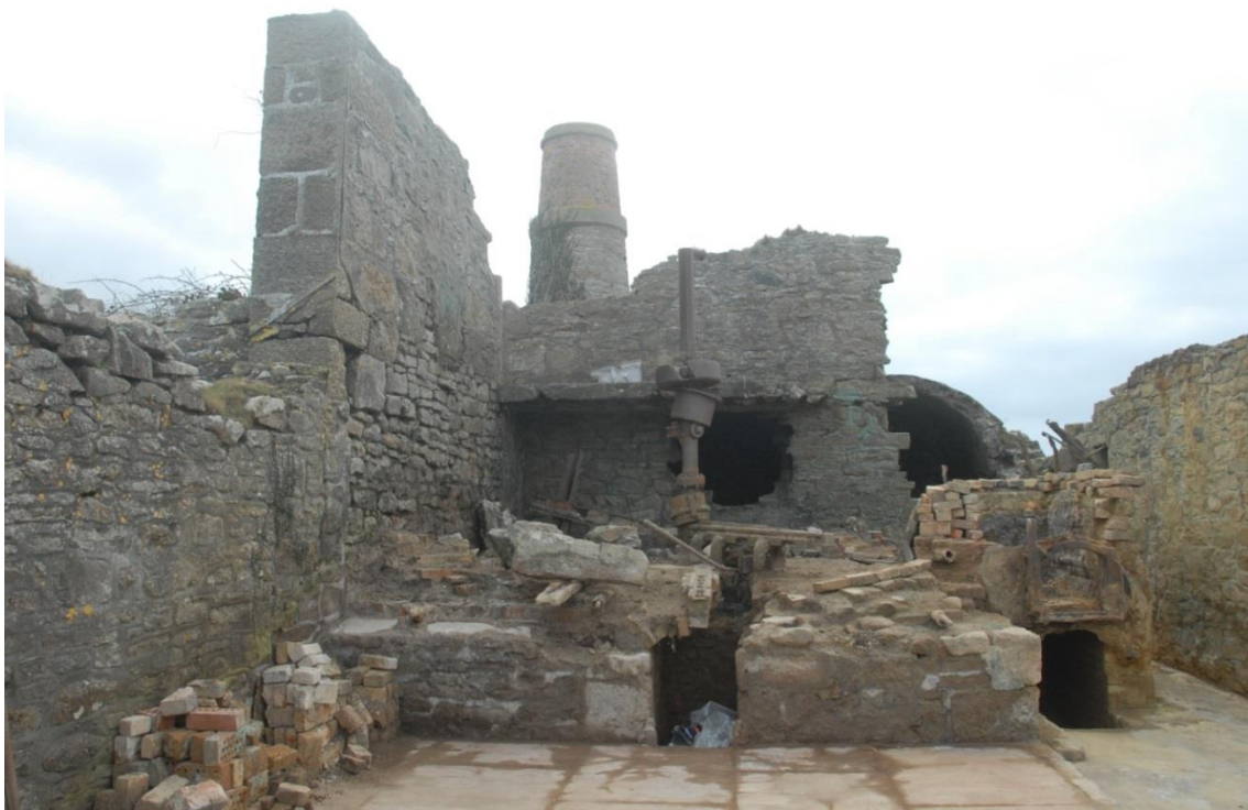
Fig 10. The calciner from the west following rubble clearance in 2015. The whole of its original brick superstructure of the calciner had been removed following the closure of the mine and the scrapping of its components.
