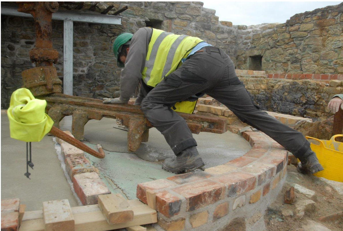
Fig 72. Laying the Paverok screed on the calciner bed.
