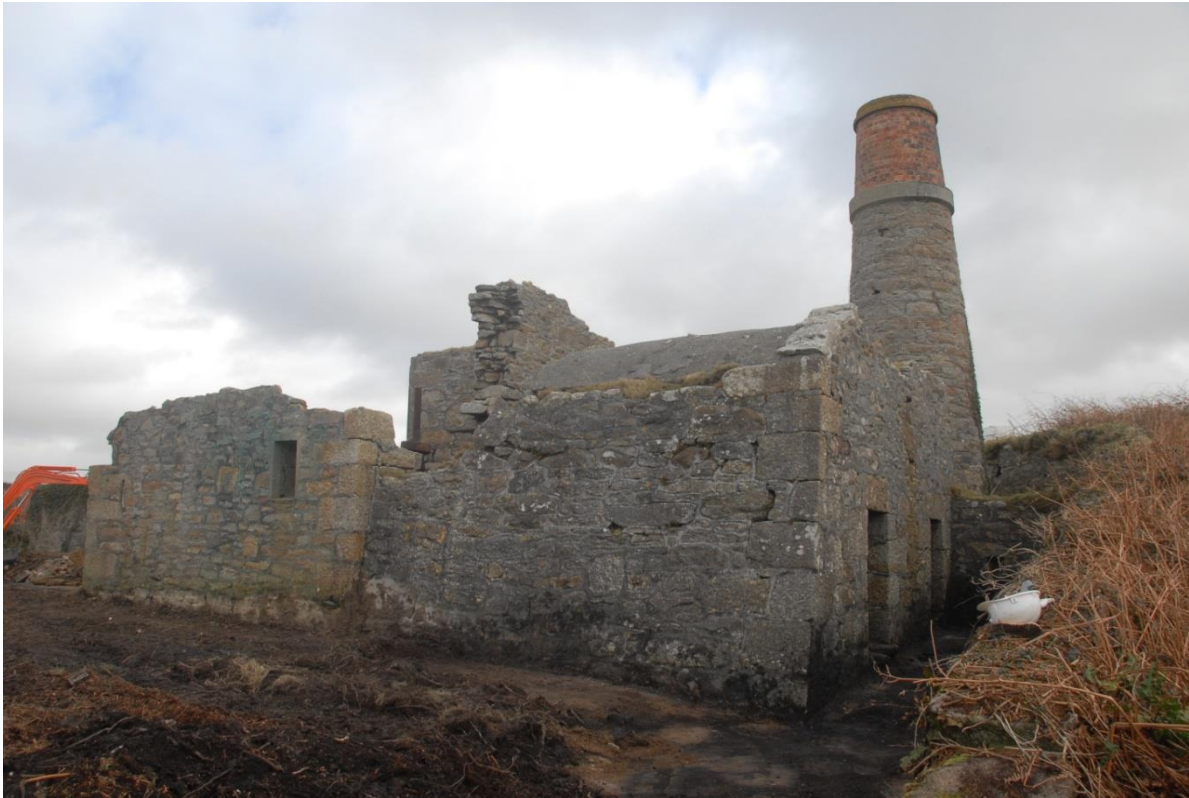
Fig 11. The calciner building (left) and dust chambers (right) showing the losses of original fabric from the western wall of the calciner and the eastern end of the northern dust chamber roof.
