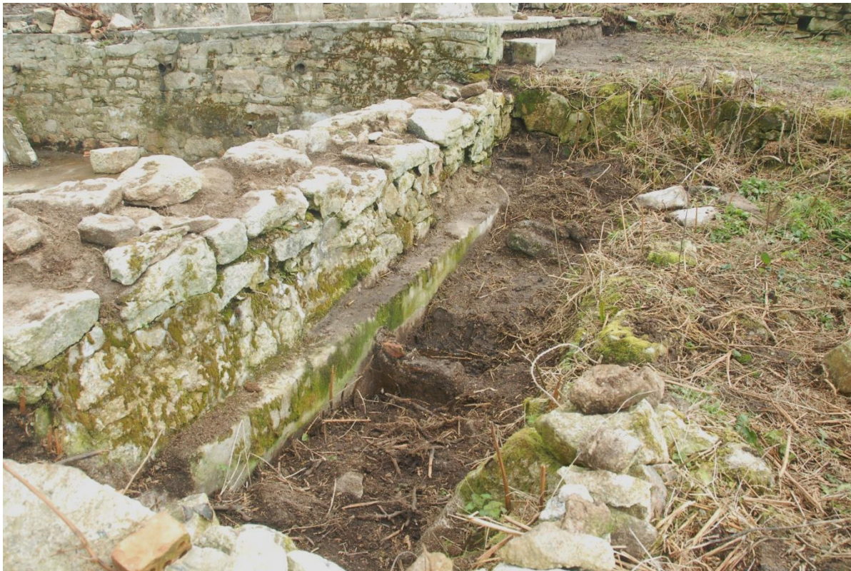
Fig 41. The small tanks external to the mill lower floor which would have collected run off from the nearby vanning tables.
