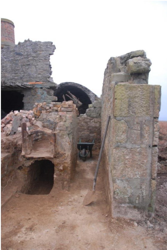
Figs 8 and 9. The eastern and western sides of the calciner furnace, showing the iron surround to the fire door (left) and the remains of the steel joists which had clamped the brickwork together to resist heat expansion forces (right).
