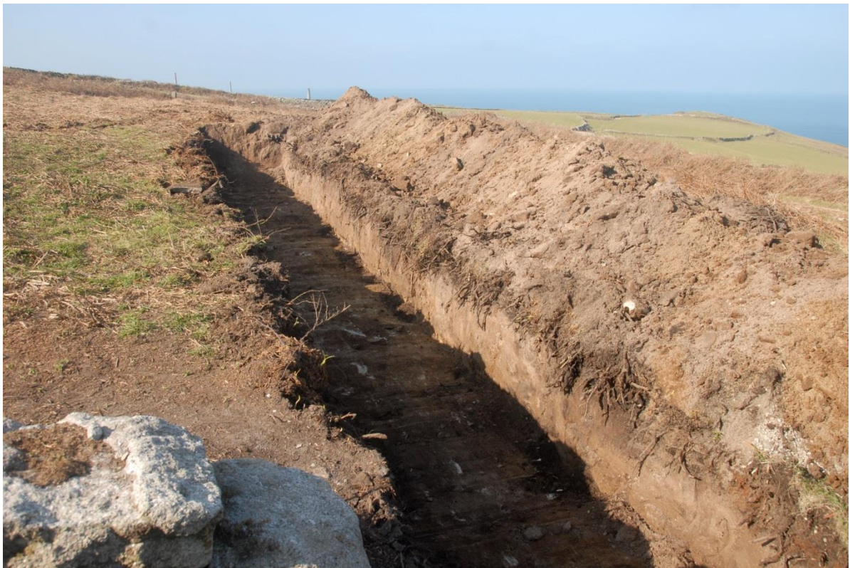
Fig 27. The 10m long trench to the west of the dust chambers excavated for the lightning conductor earth mats.
