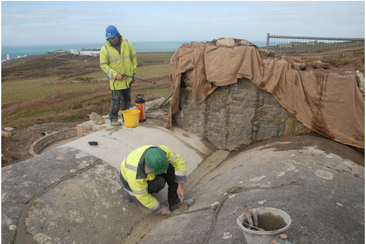
Fig 60. Grouting cracks in the roof of the dust chambers prior to the coating of the whole roof with Fosrok Brushbond to waterproof it.
