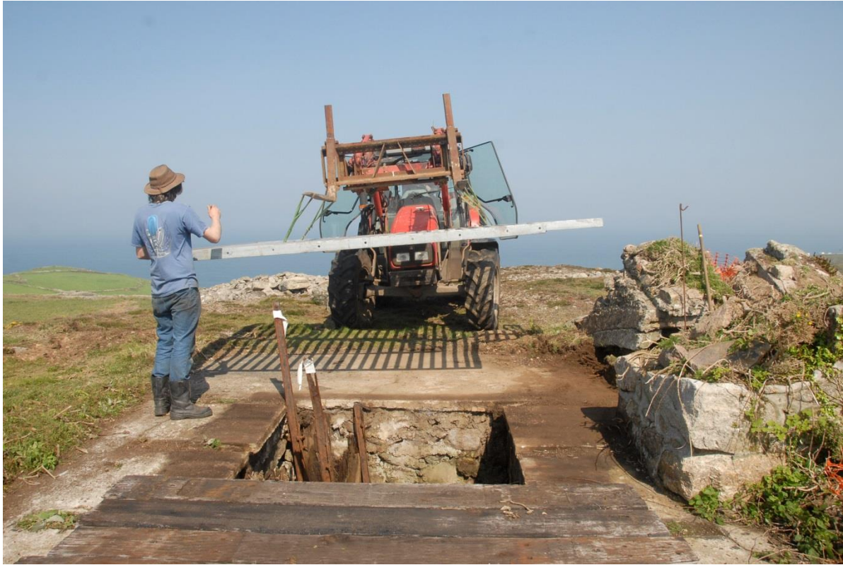
Fig 84. Manoeuvring the first section of the new steel grille onto Trease Shaft once the sleeper cap had been partly removed.
