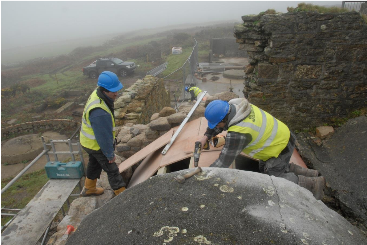
Fig 58. Making up the formwork on which the replacement section of the northern dust chamber roof would be cast.
