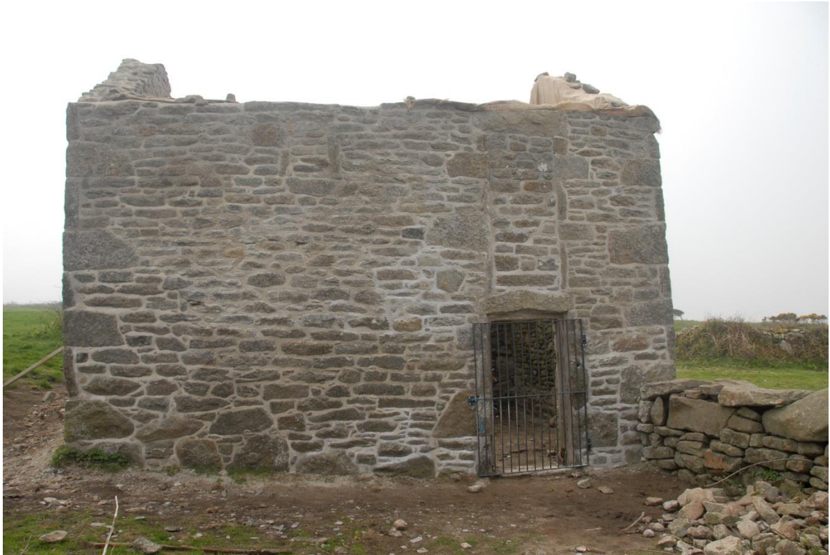
Fig 32. The completed northern face of the barn, showing the blocked upper floor doorway and windows and the lockable gate on the ground floor doorway.
