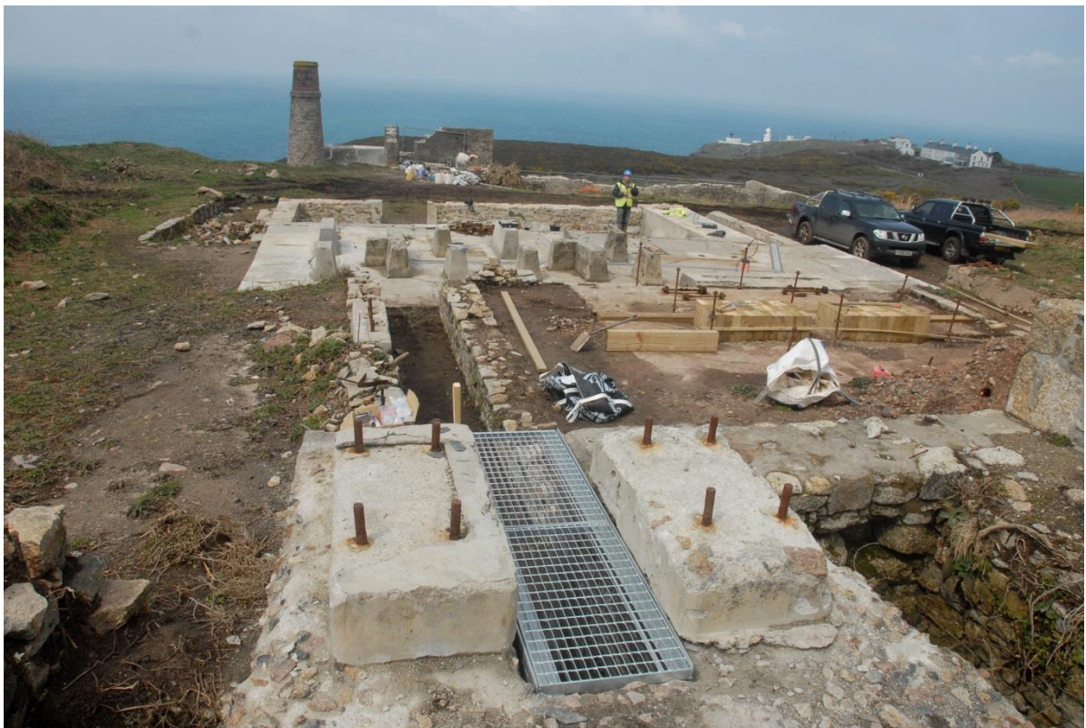
Fig 51. The grille set between the mill engine loadings.
