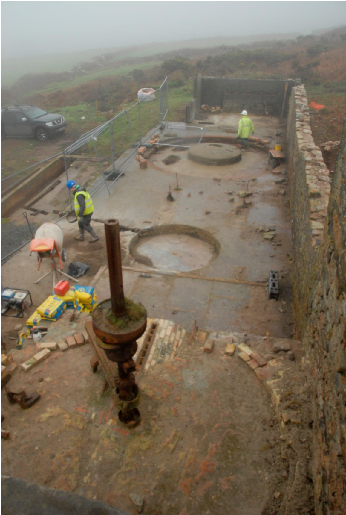
Fig 68. An overview of the tin floors at an early stage of the project showing (foreground) the calciner bed prior to reconstruction works.
