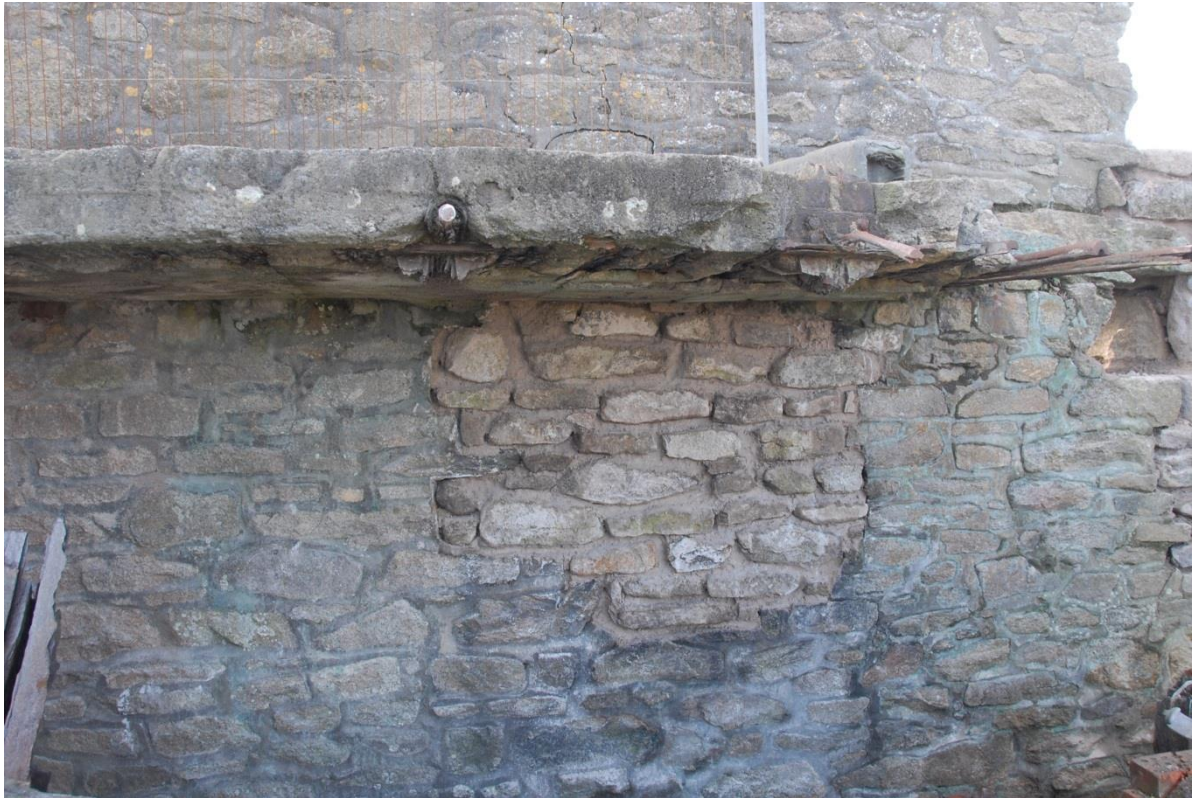
Fig 54. The rebuilt damaged section of the eastern wall of the southern dust chamber.
