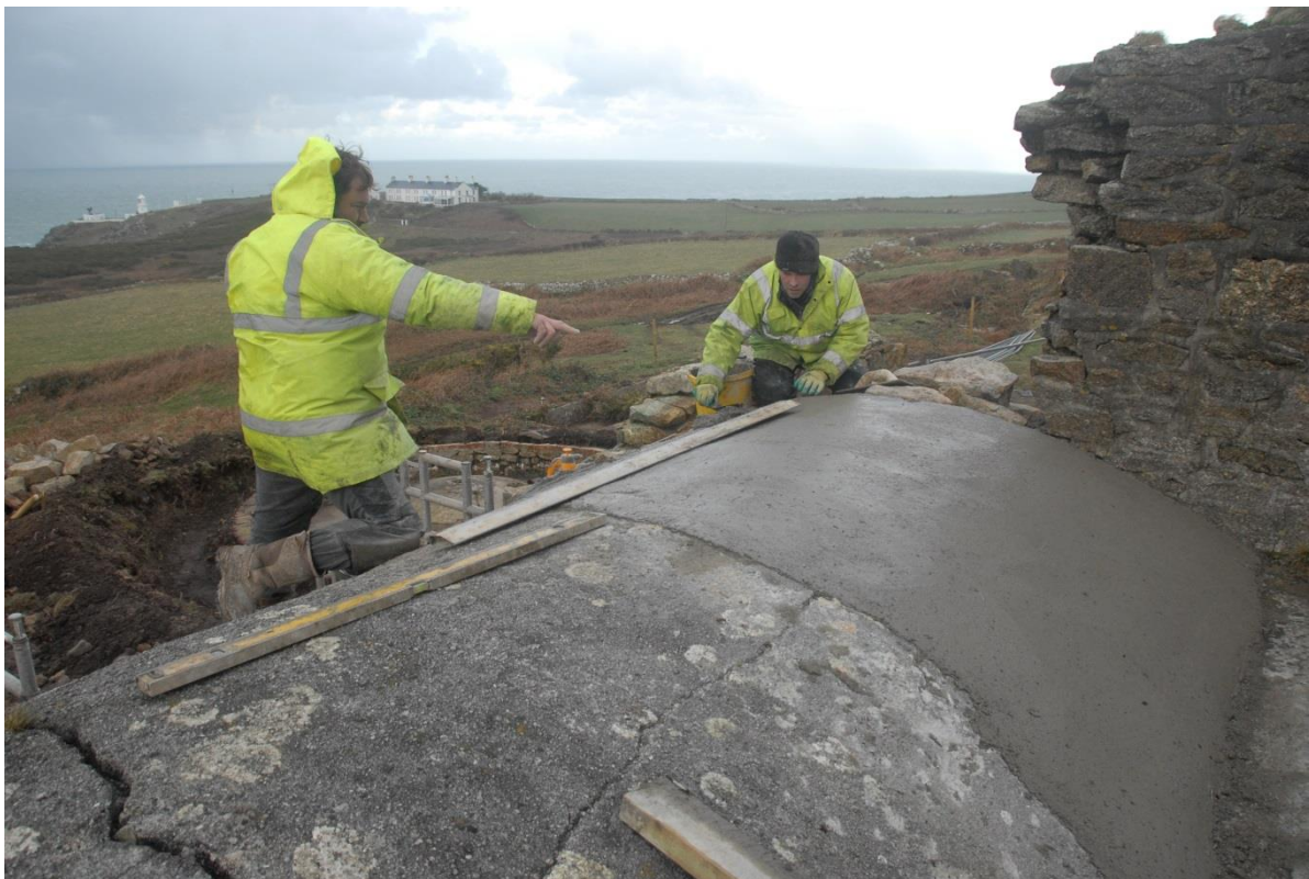
Fig 59. Forming the new section of concrete roof over the northern dust chamber.
