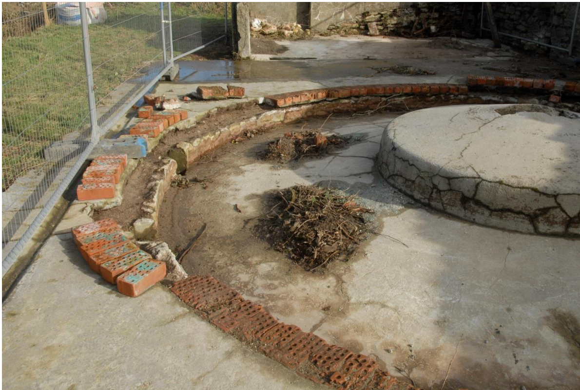
Fig 52. The buddle on the tin floors following the cutting out of its damaged brickwork. Salvaged bricks are being readied for the repair works.
