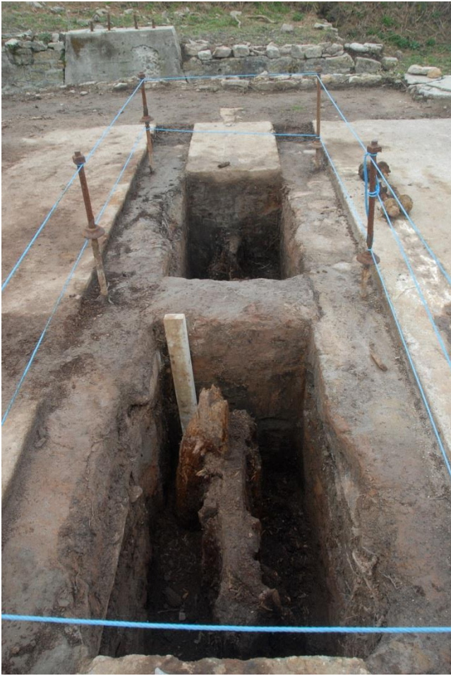
Fig 48. The excavated stamps anvil sockets, showing the remnant timberwork in their bases.
