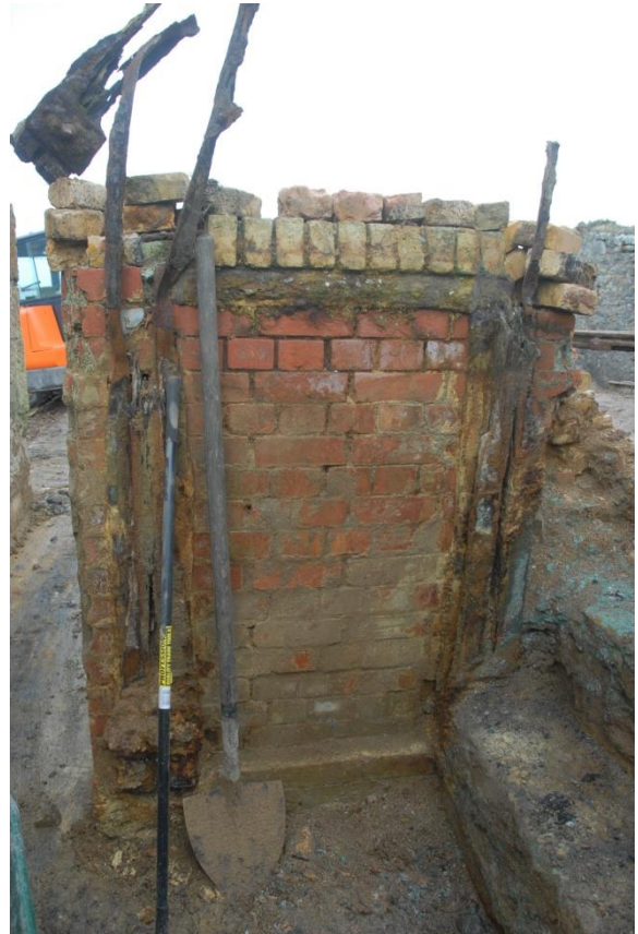
Figs 8 and 9. The eastern and western sides of the calciner furnace, showing the iron surround to the fire door (left) and the remains of the steel joists which had clamped the brickwork together to resist heat expansion forces (right).
