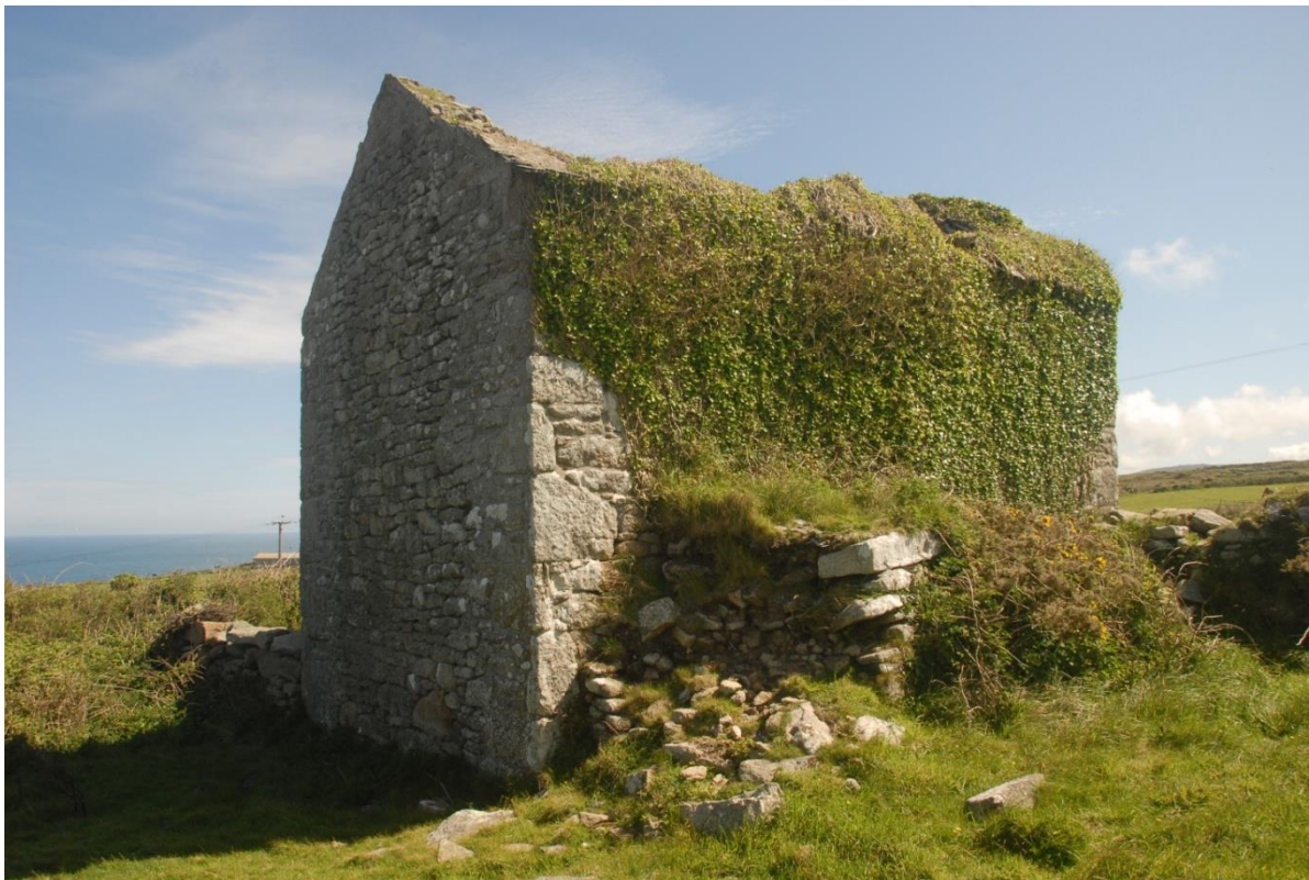
Fig 14. Trease field barn from the south-west, showing the remains of the ramp/steps to the first floor door and the ivy which covered the southern elevation of the building.
