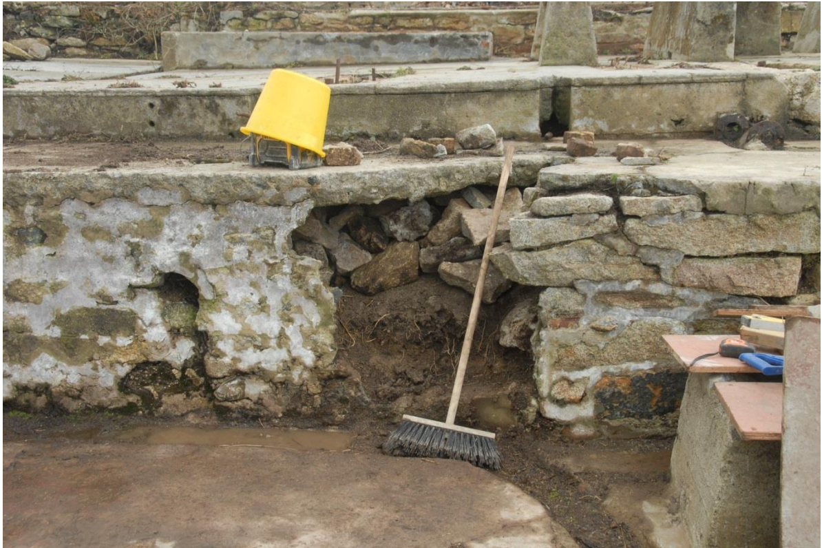
Fig 38. The significantly voided area at the rear of the lowest mill floor during its packing with loose stone and mortar to backfill it.
