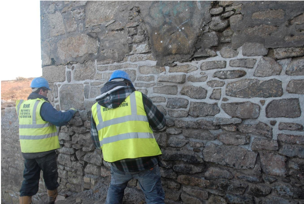
Fig 56. Repointing the lower section of the southern wall of the calciner enclosure in lime mortar. The upper section of the wall, which includes the location of the end of a feed hopper (top centre), was repointed in a cement mix to match the surrounding mortar.
