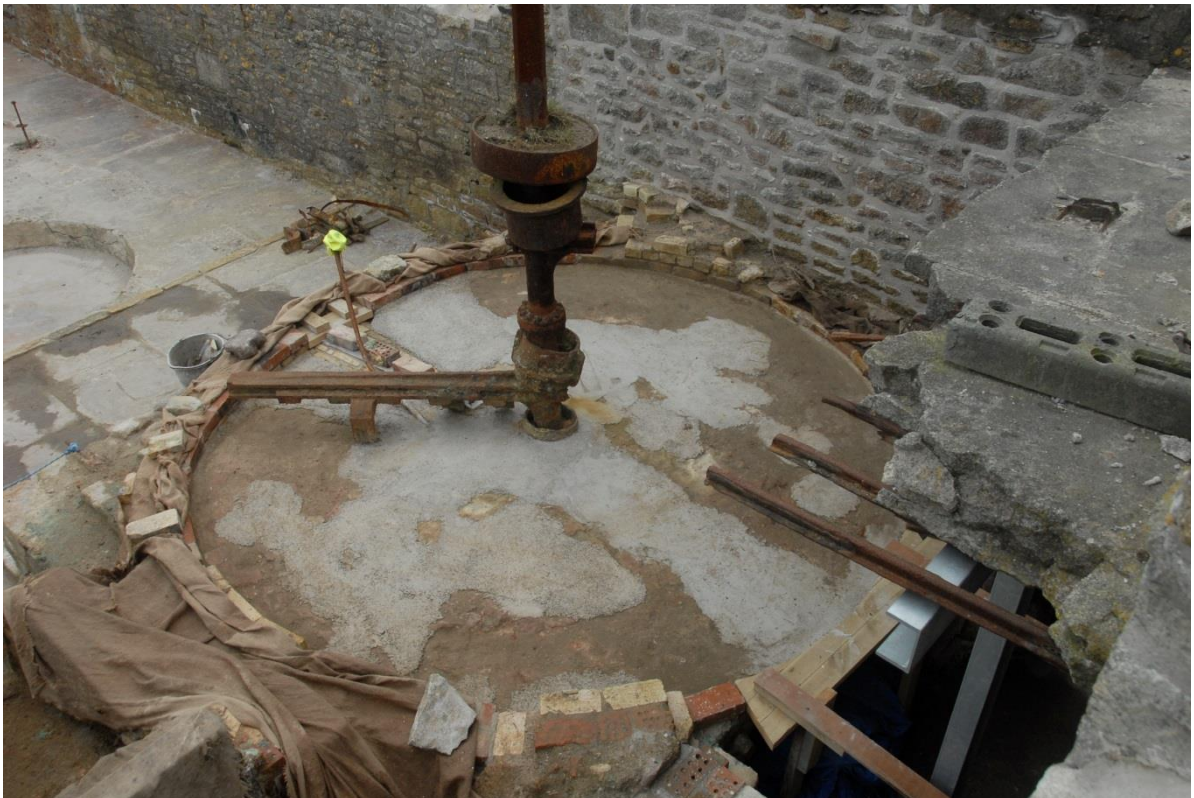
Fig 70. The calciner bed prepared for its re-screeding.
