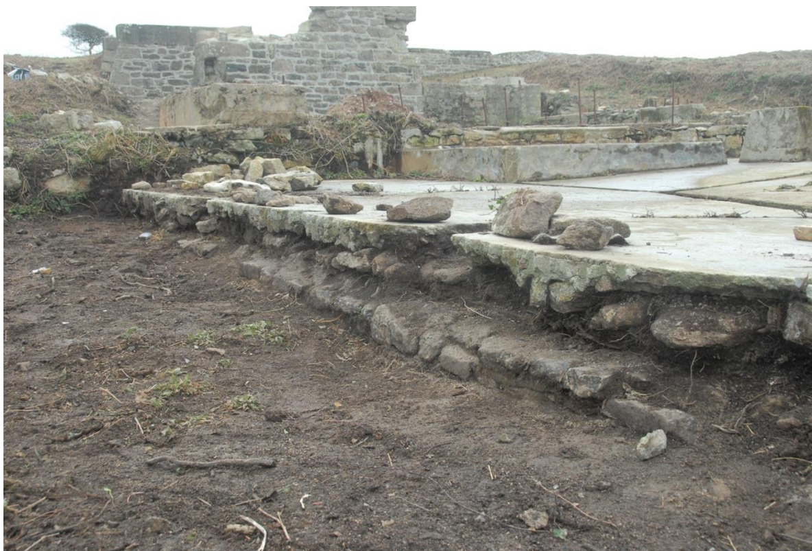
Fig 36. The badly undercut eastern edge of the middle mill floor prior to works.
