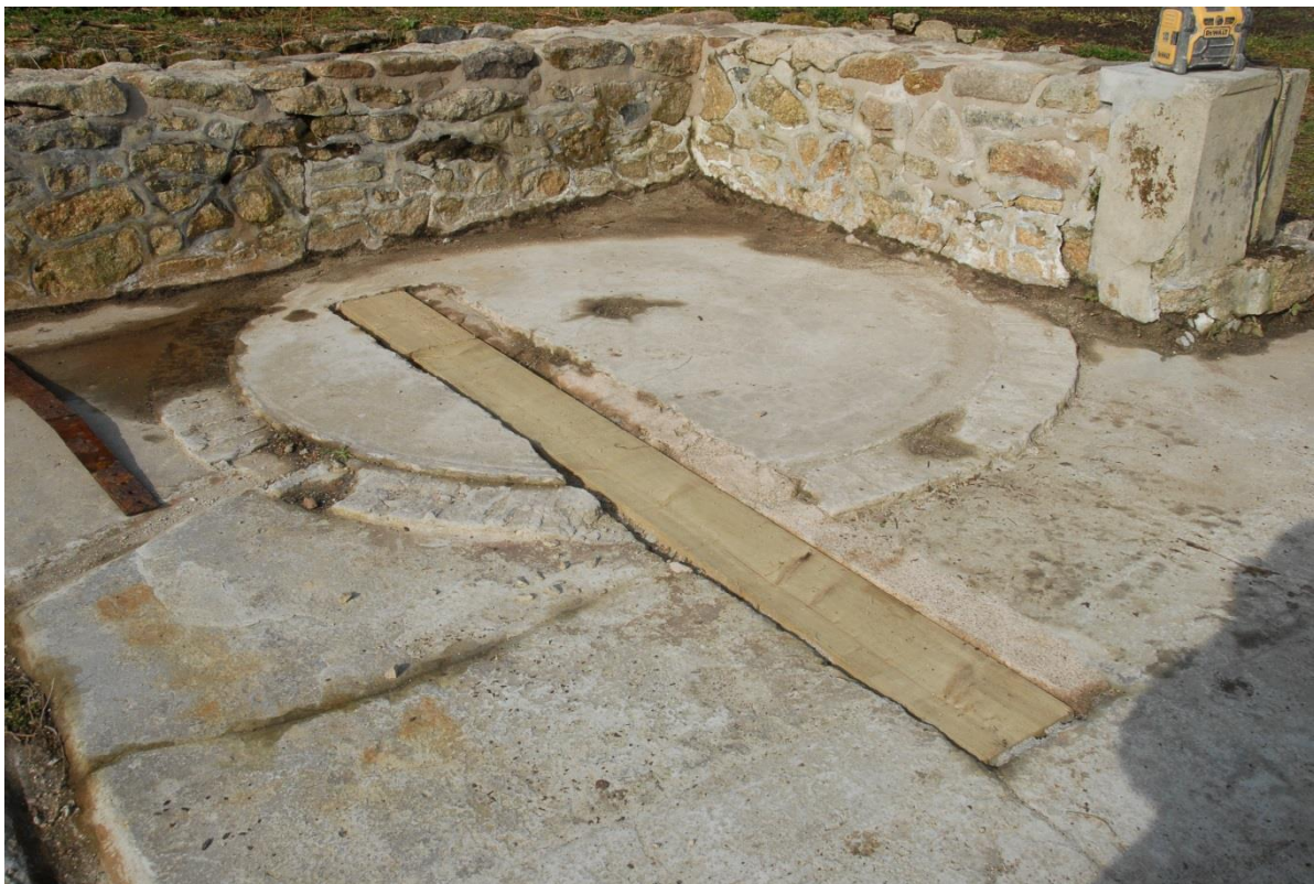
Fig 45. One of the replacement timbers set into the floor support sockets for one of the vanners, here crossing the buddle which it replaced.
