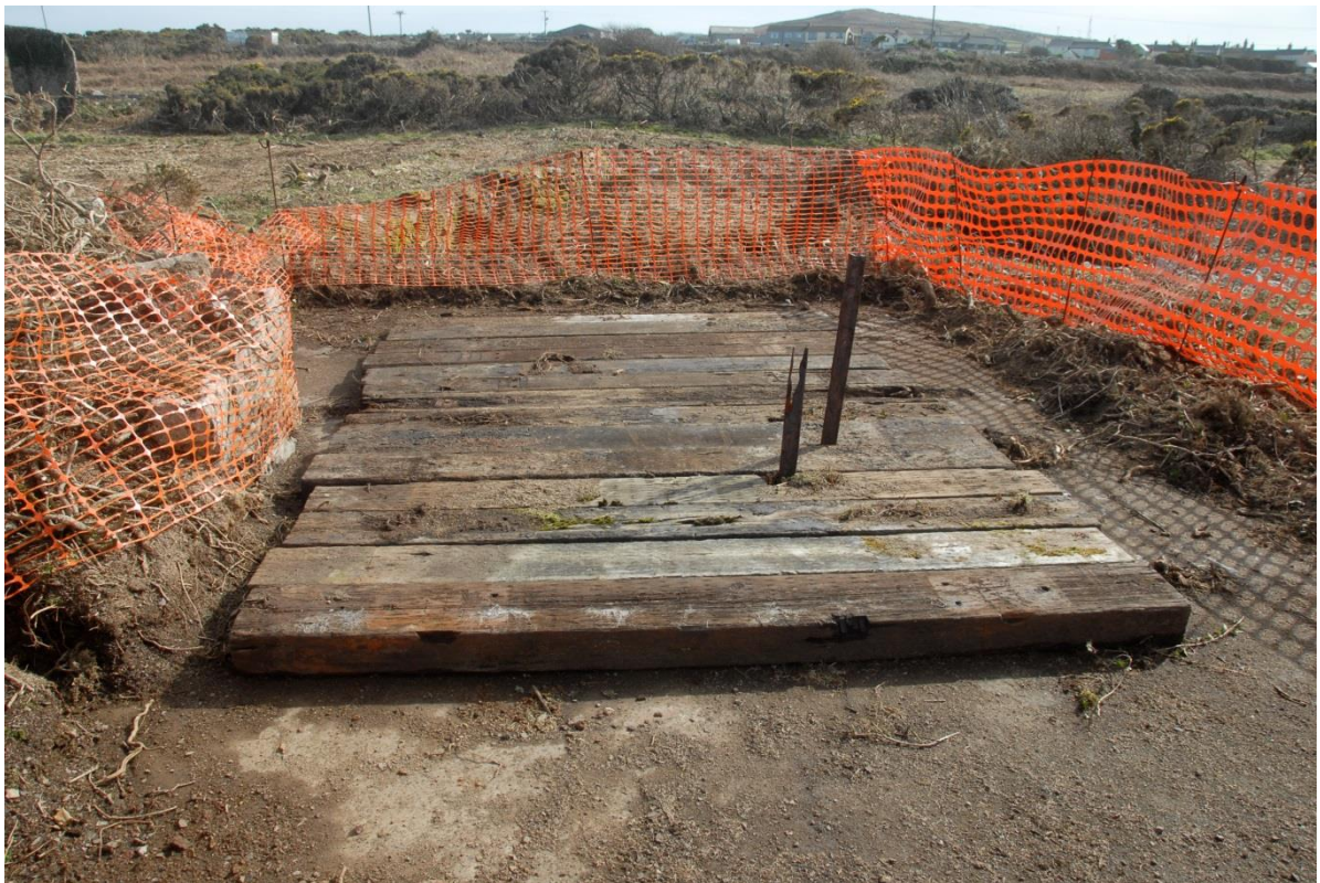
Fig 17. The Trease Shaft sleeper cover following the clearance of scrub vegetation. Paired tramway rails reused as shaft guides protrude through the cover. The sleepers were to be replaced by a galvanised steel grille (see Fig 86).
