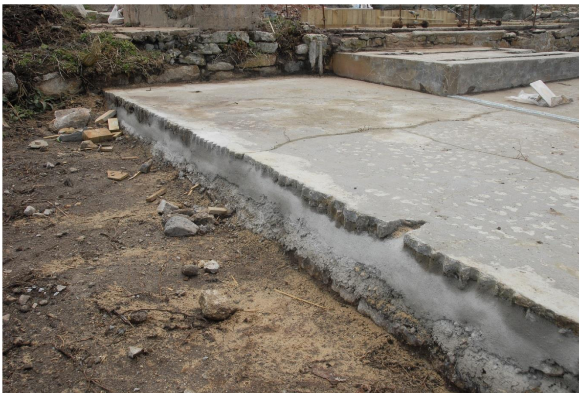
Fig 37. The concrete underpinning works to the edge of the mill floor.
