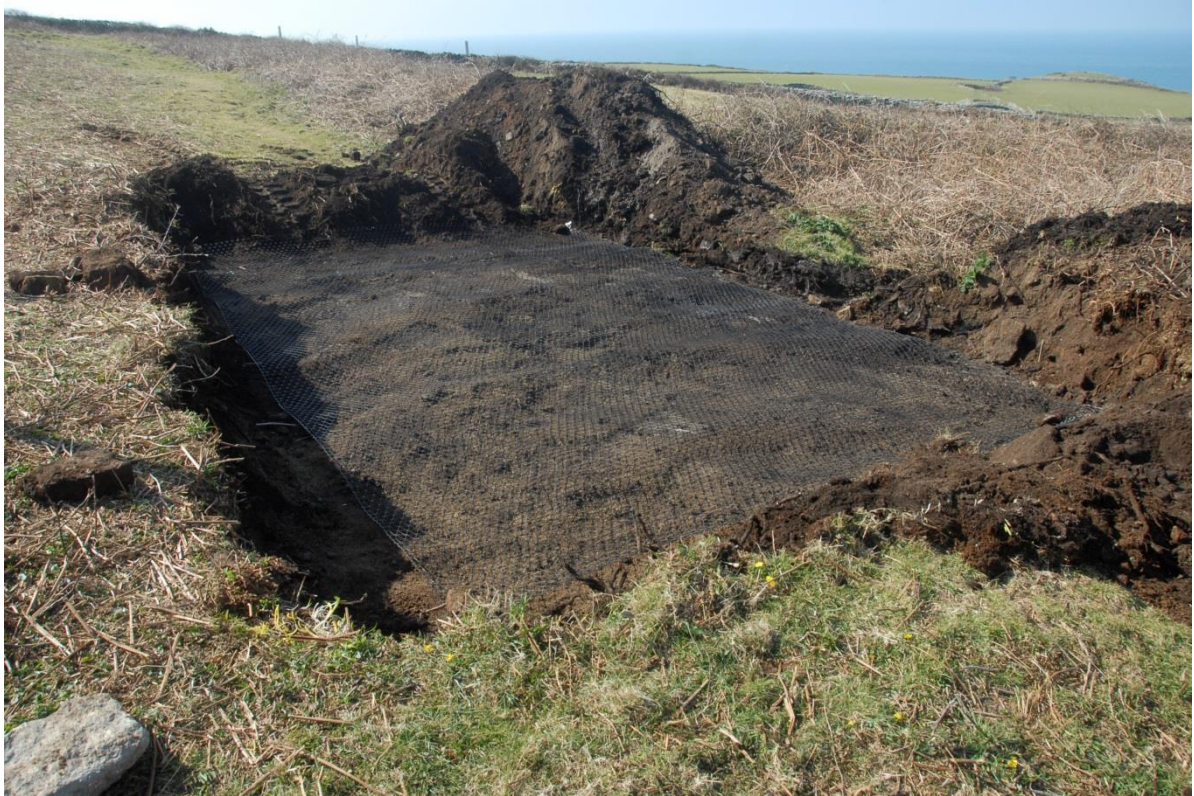
Fig 26. The geogrid reinforcement installed across the backfilled outcrop workings prior to the backfilling of this trench.
