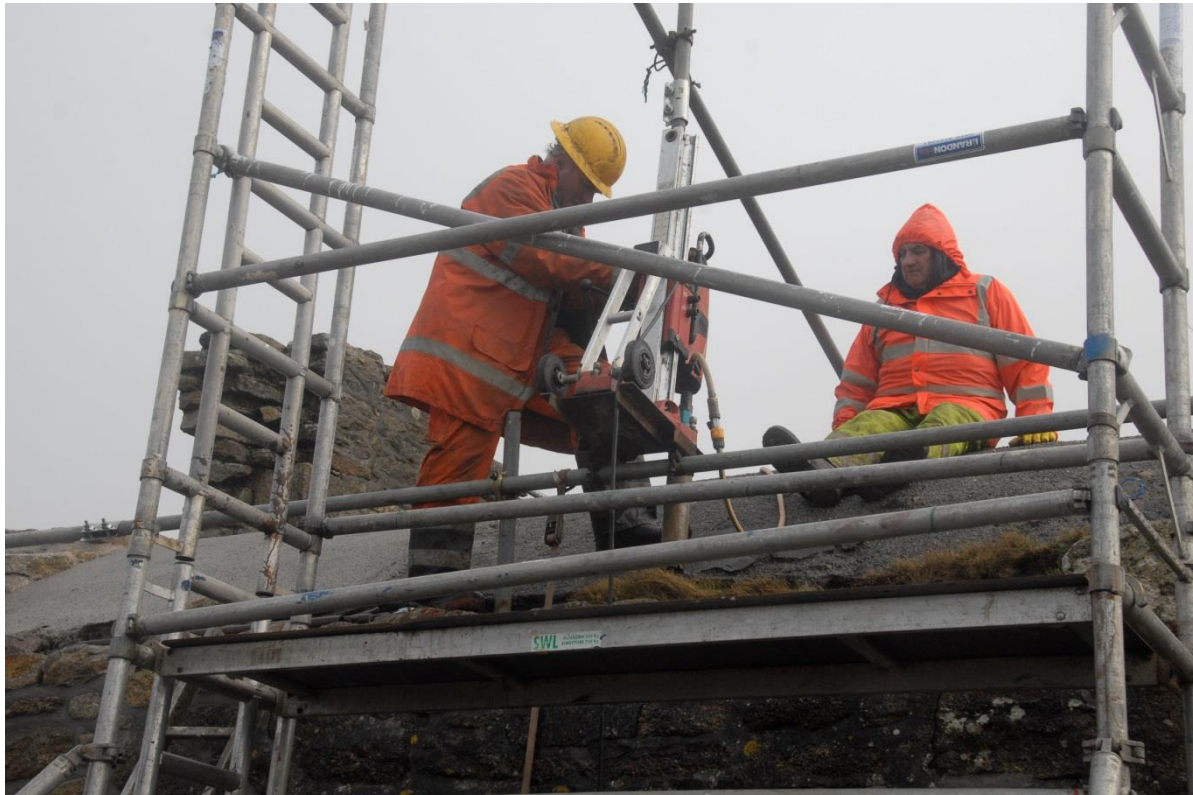
Fig 63. Drilling one of the vertical drill holes for the Cintec reinforcing bars to be installed within the northern wall of the dust chambers.
