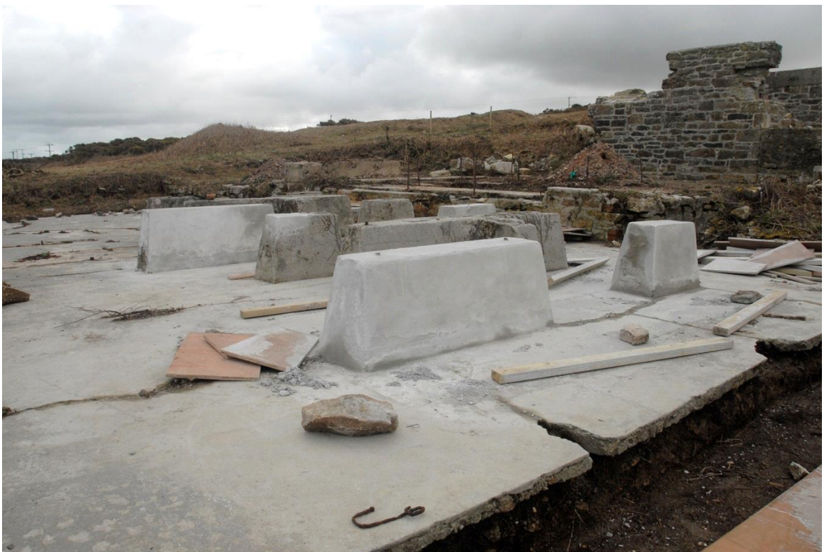
Fig 35. The re-formed Pinder Table mountings on the middle mill floor.
