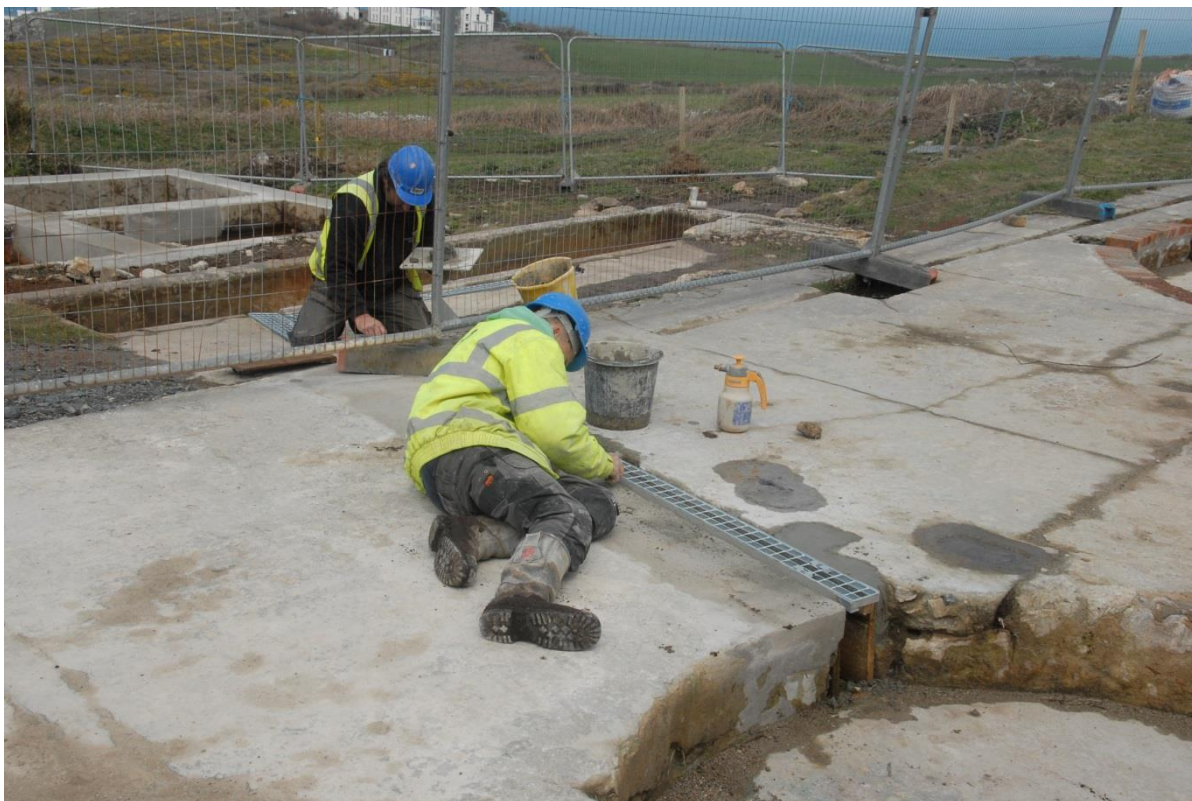
Fig 47. Installing grilles over drains on the tin floor.
