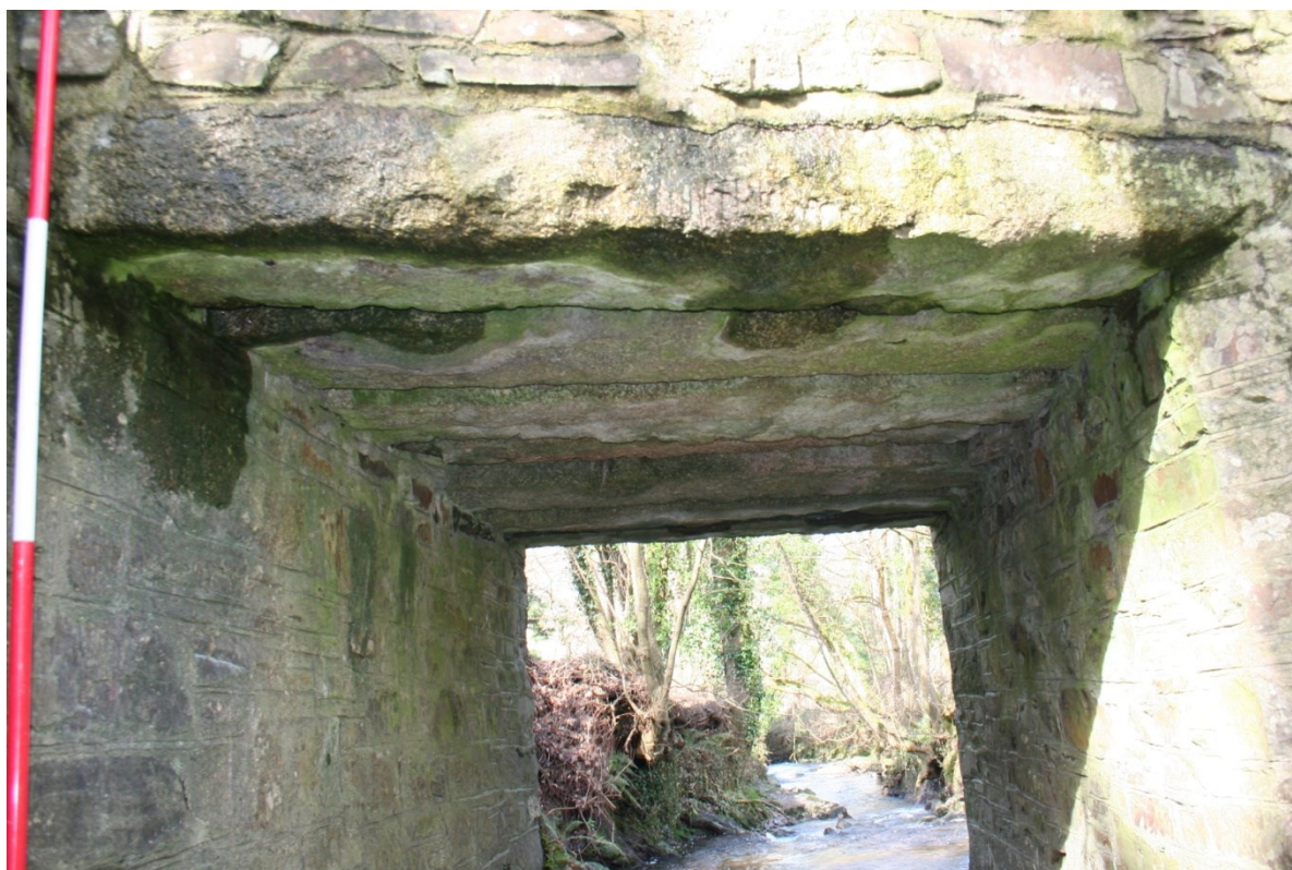
Fig 11 East (upstream) elevation showing span lintels
