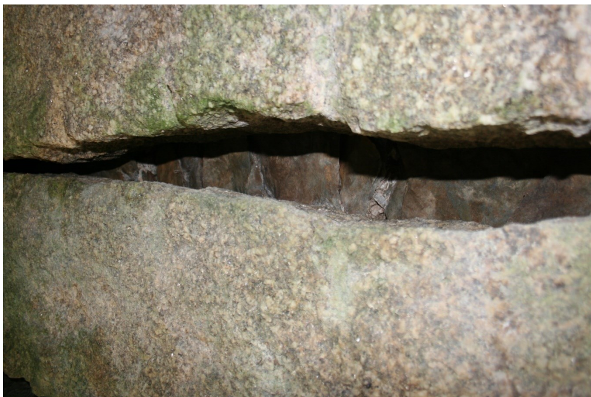
Fig 15 Detail of rubble core above span lintels
