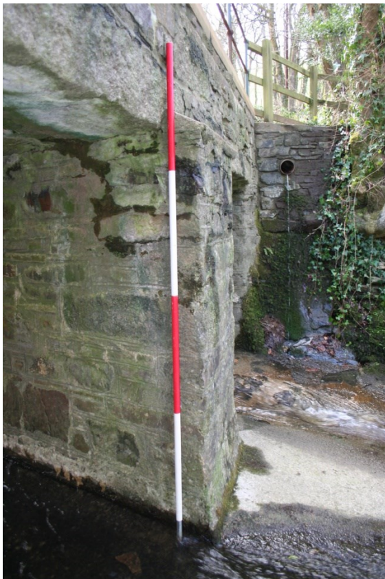
Fig 9 West (downstream) elevation showing square end of the cutwater pier
