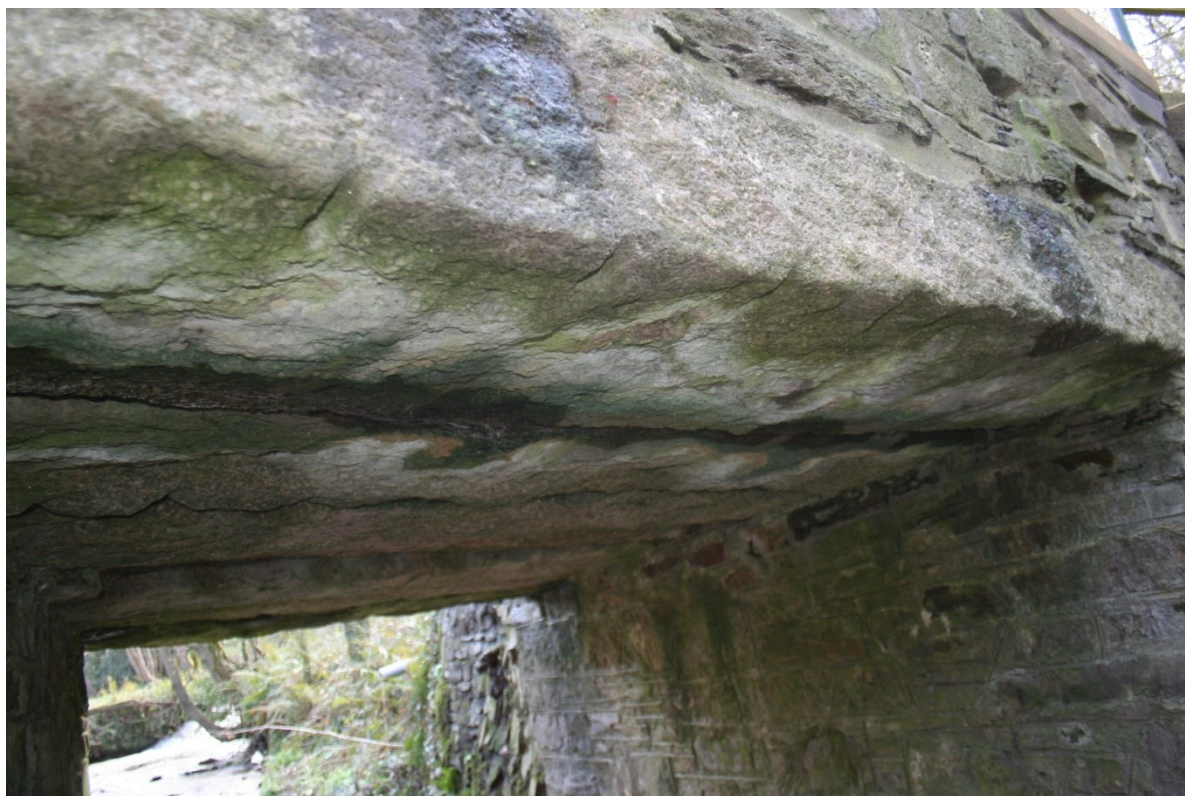
Fig 10 West (downstream) elevation showing span lintels with quarry drill marks
