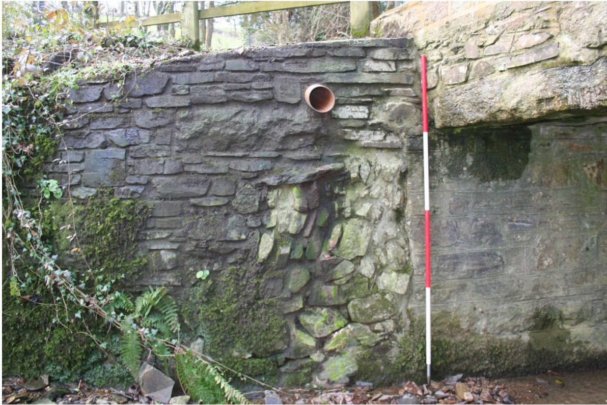
Fig 12 South abutment, upstream side showing evidence or earlier abutment walling
