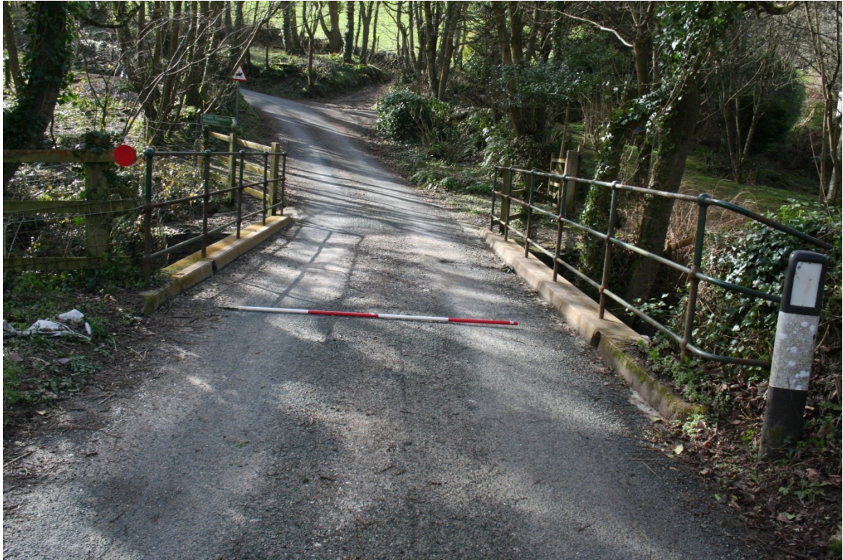
Fig 16 The bridge facing south
