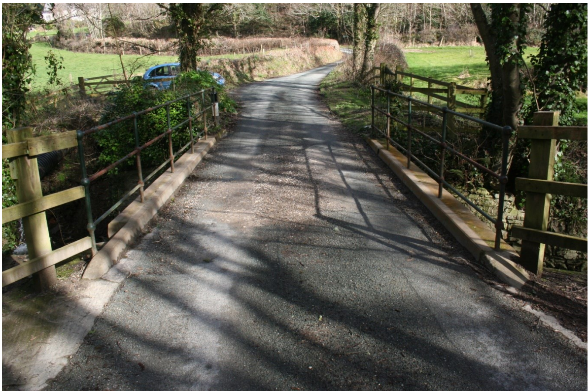
Fig 17 The bridge facing north
