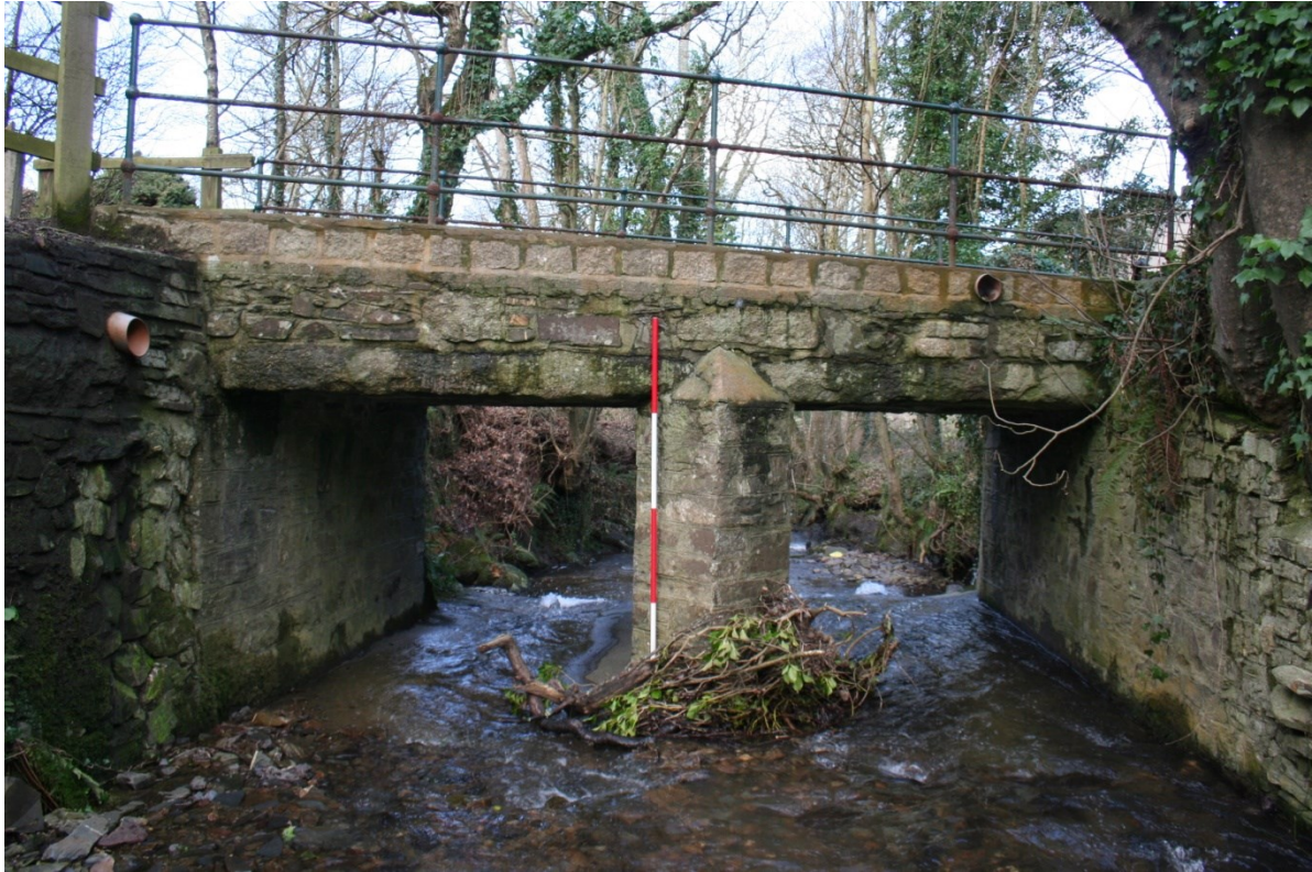
Fig 8 East (upstream) elevation
