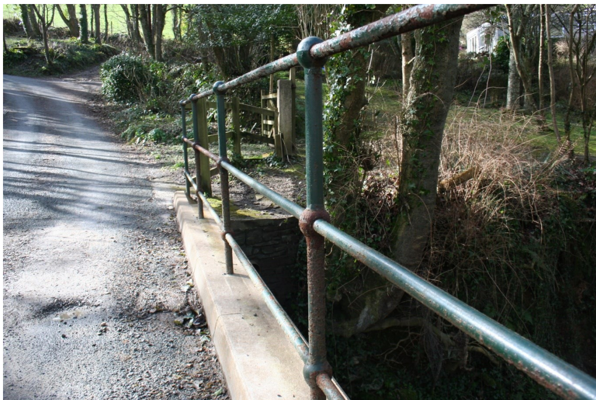
Fig 18 Detail of iron rails, downstream side
