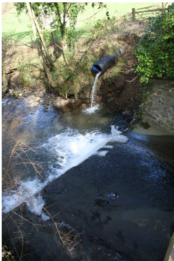
Fig 19 Weir and pipe, downstream
