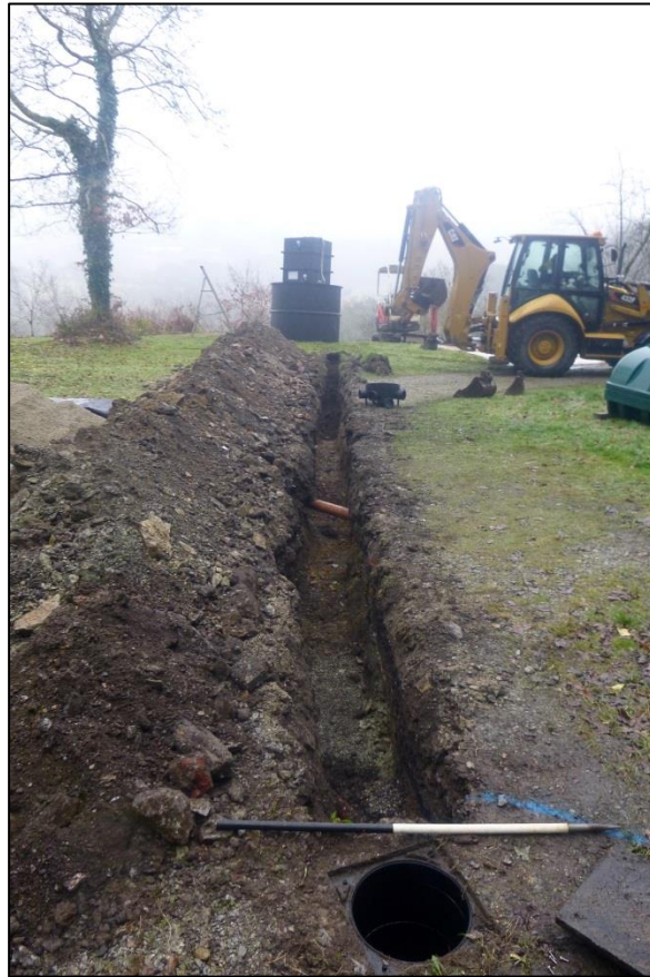
Figure 5: View of main sewer trench looking south (1m scale).
