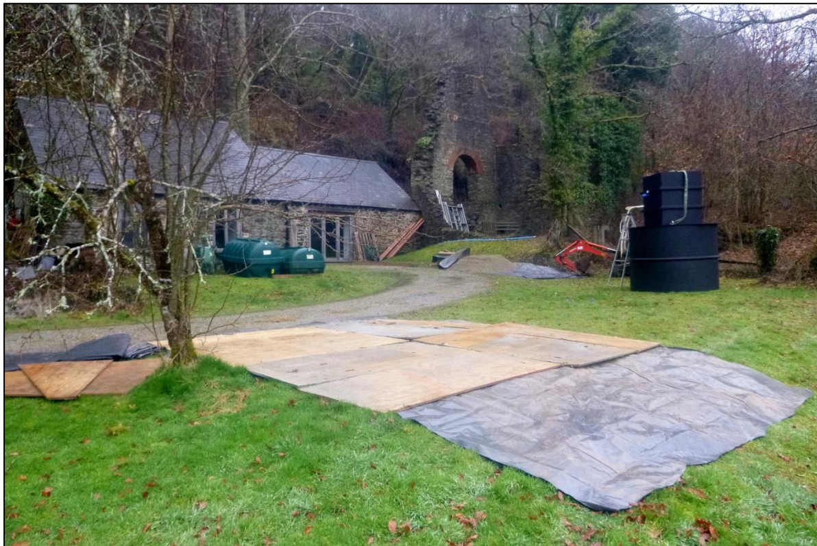
Figure 4: View looking north east of site prior to excavation.
