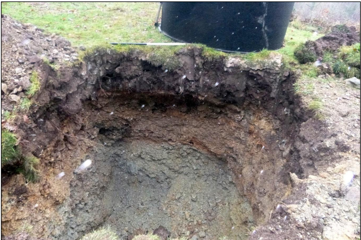
Figure 6: View of north facing section of main sewage plant pit (1m scale).
