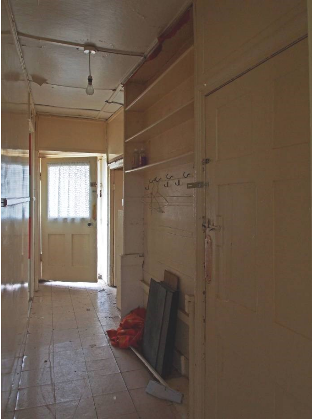
Fig 15 Rear hallway, showing the frame and shelving of the built-in dresser.
