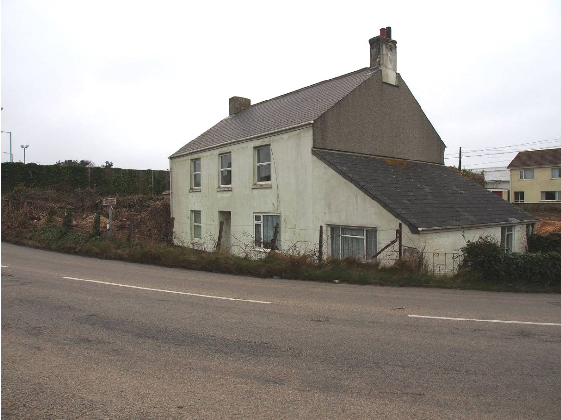
Fig 12 Penhellick, looking northwest.
