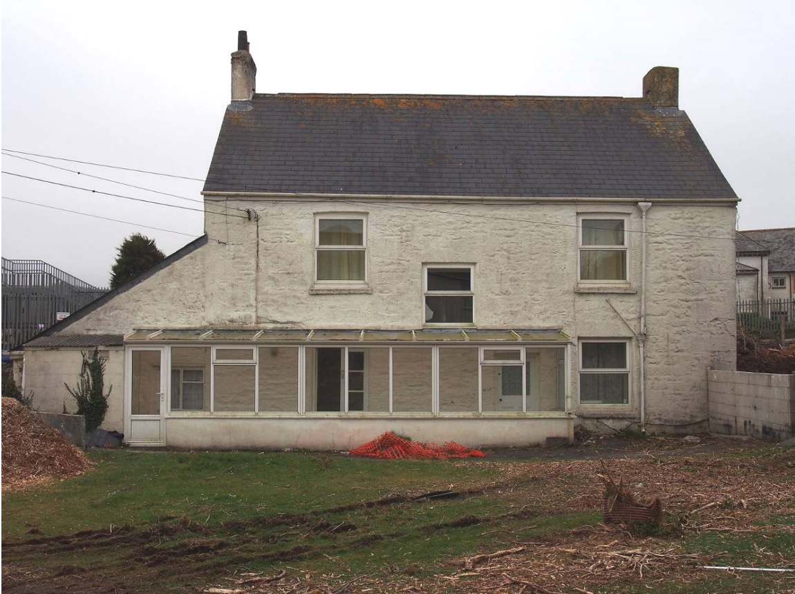
Fig 11 Rear (north) elevation of Penhellick.
