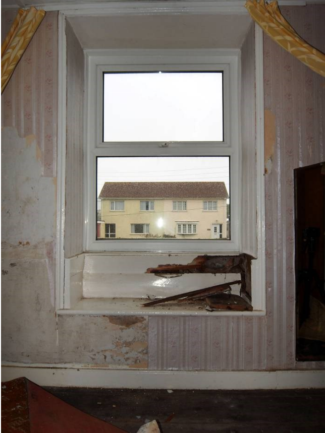
Fig 25 Original window seat and moulded architrave in window of Bedroom 1.
