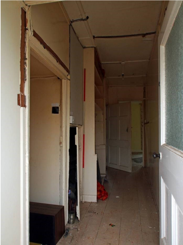
Fig 14 Rear hallway, with low doorway to former service room to left.
