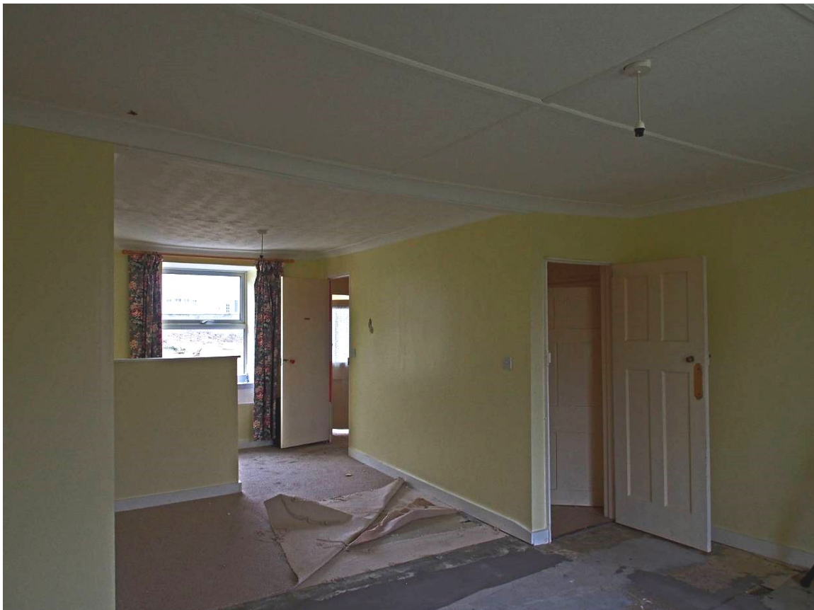
Fig 17 View into original kitchen space, now sub-divided by modern passageway partition.
