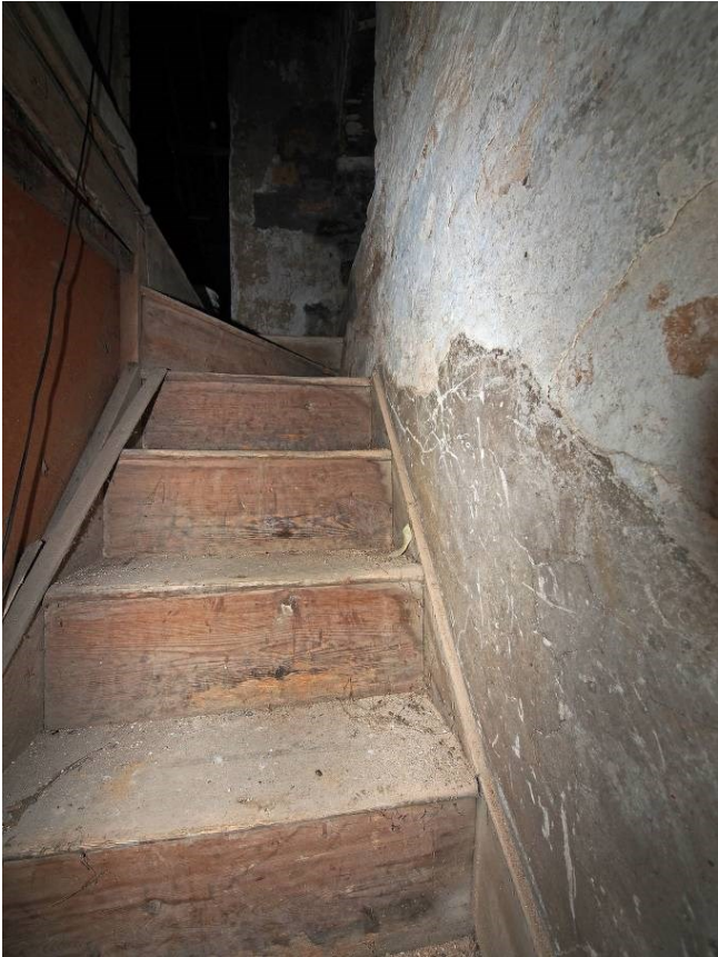
Fig 29 Service stairway to attic.
