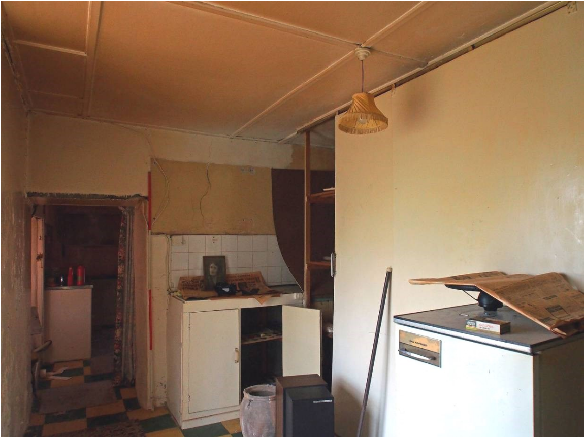
Fig 18 Rear service room.
