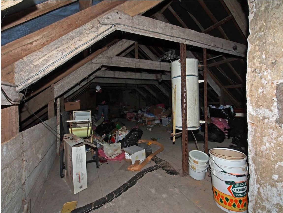
Fig 32 Attic level. The roof bays once formed divisions between service bedrooms.
