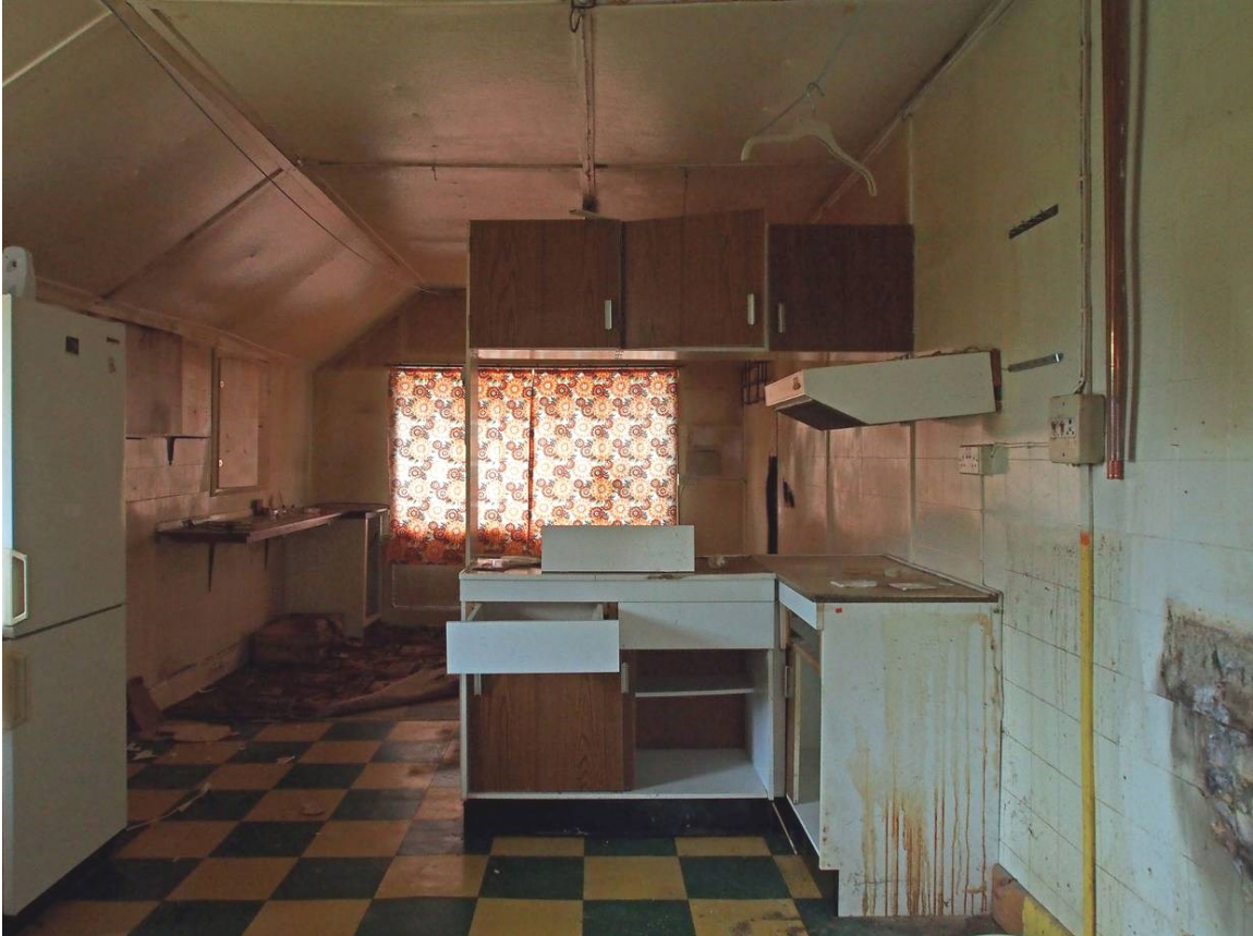
Fig 19 Replacement kitchen, built into extension.
