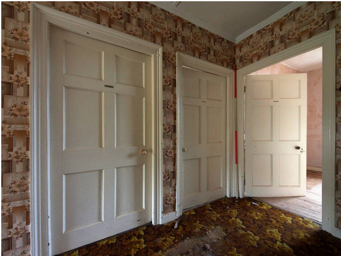
Fig 23 Original 18 th century 6-panel bedroom doors, viewed from the landing.
