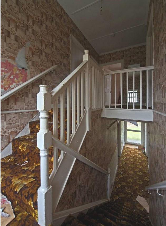
Fig 21 Stairs and landing.
