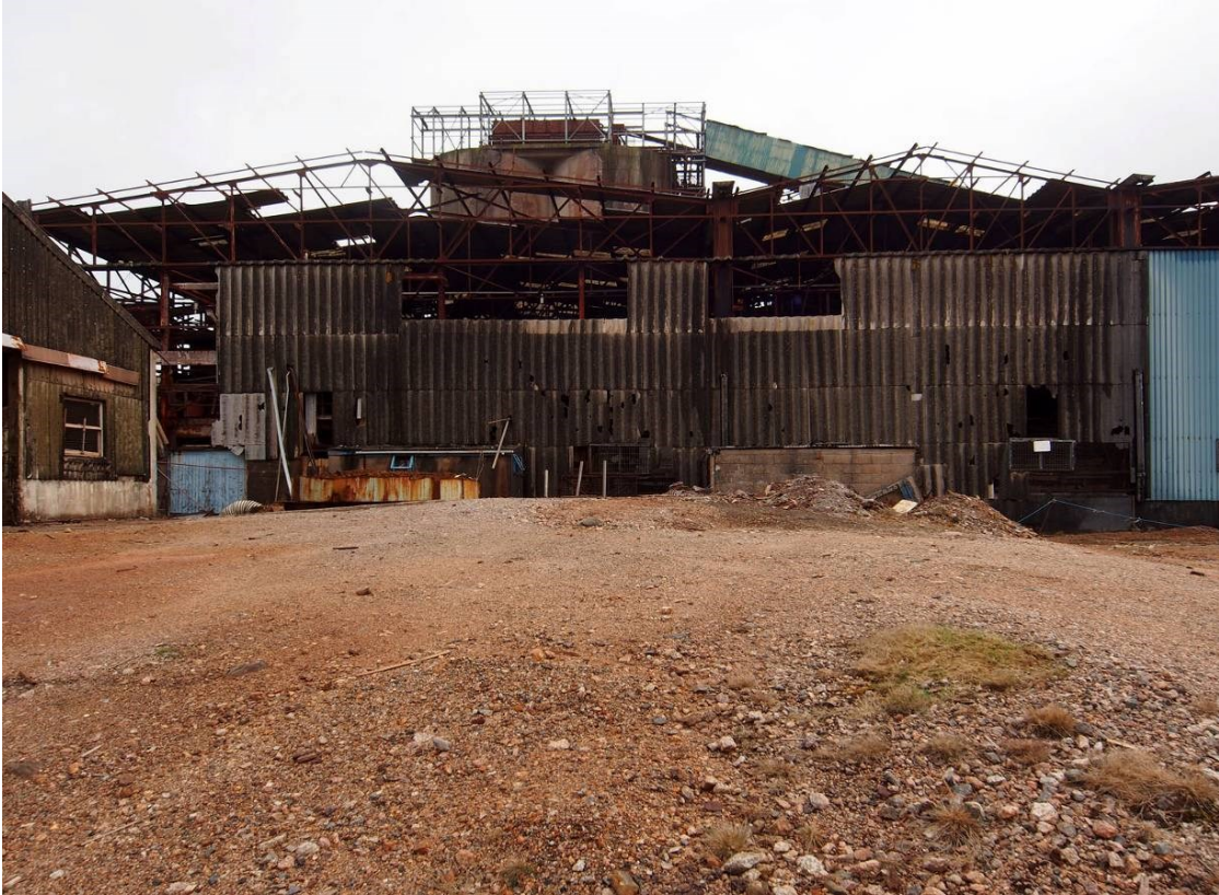
Fig 22. The table plant building viewed from the west.
