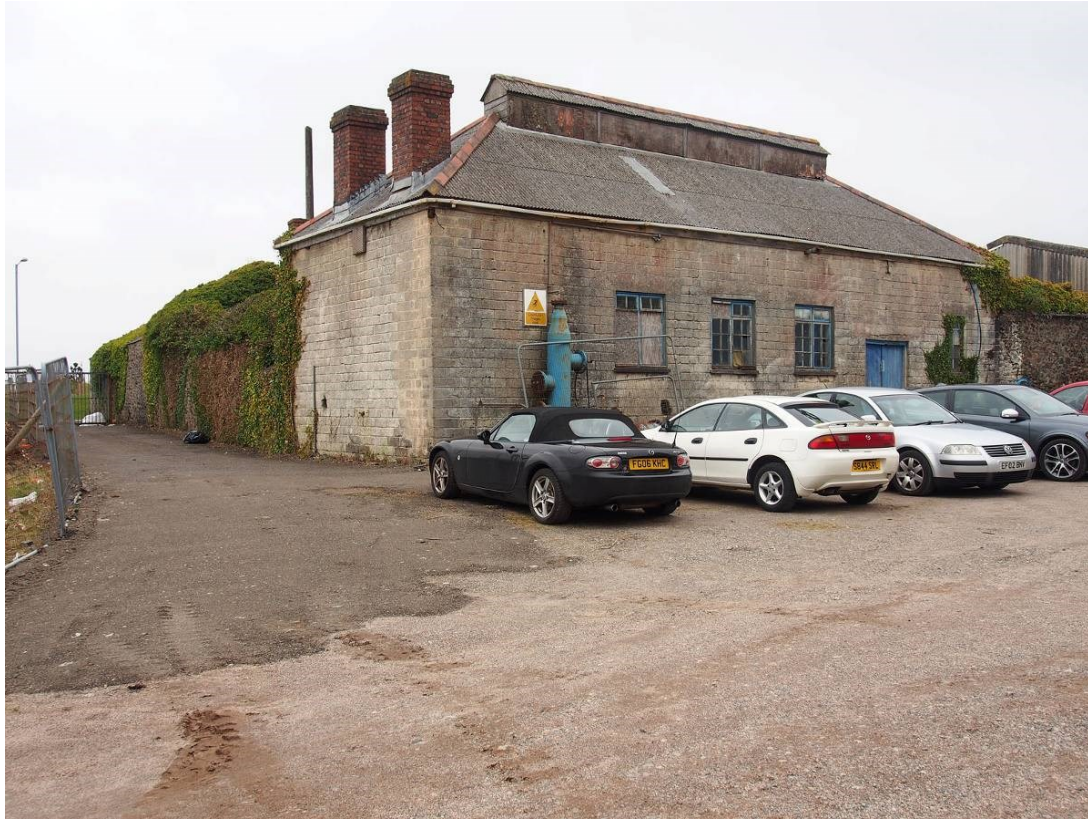
Fig 32. The South Crofty smithy building, constructed in the early 20 th century on the site of a smithy associated with Bartle's Foundry within the yard to its rear.
