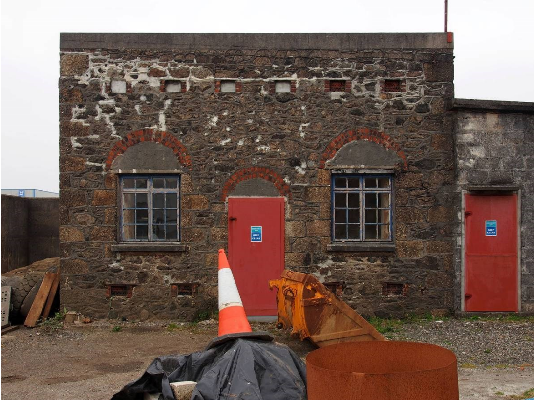
Fig 29. The early 20 th century sub-station building at South Crofty.
