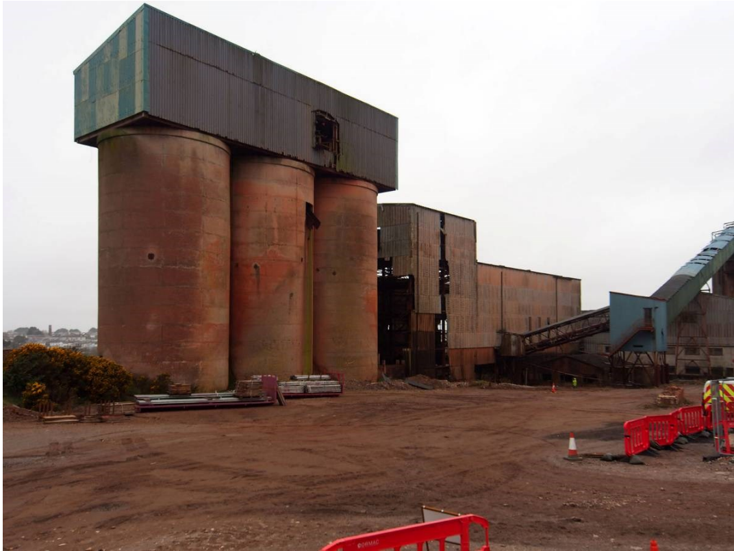
Fig 9. The primary ore bins (left), primary crusher house (centre) and the conveyor leading to the fine ore bins (right) viewed from the south east.
