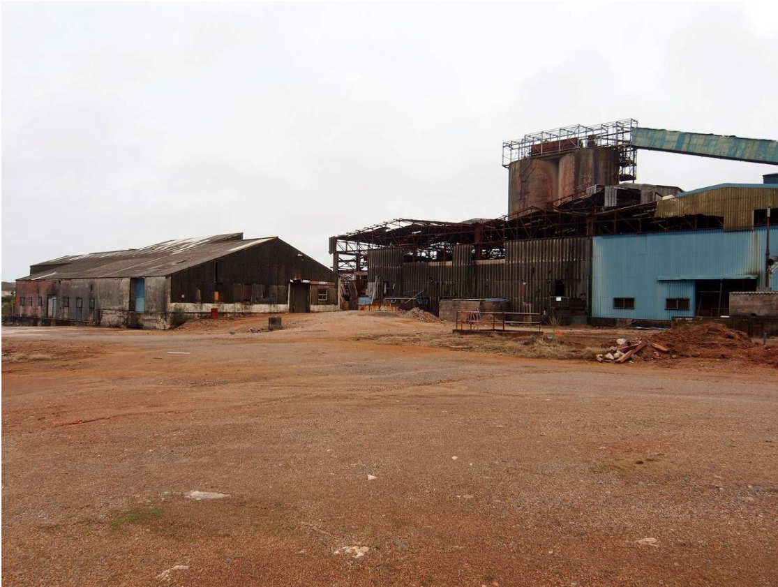
Fig 19. The northern end of the mill viewed from the south west. The roofless building in front of the fine ore bins sited the shaking tables and flotation plant.
