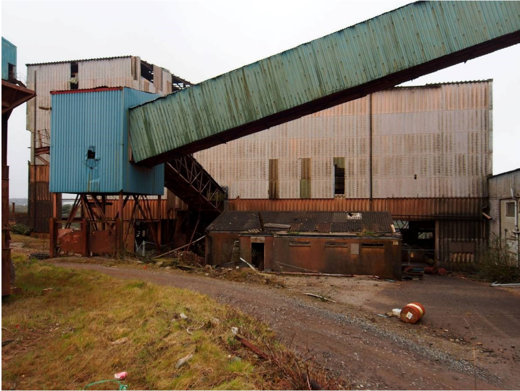
Fig 15. The primary crushing plant and ore conveyer from the east.
