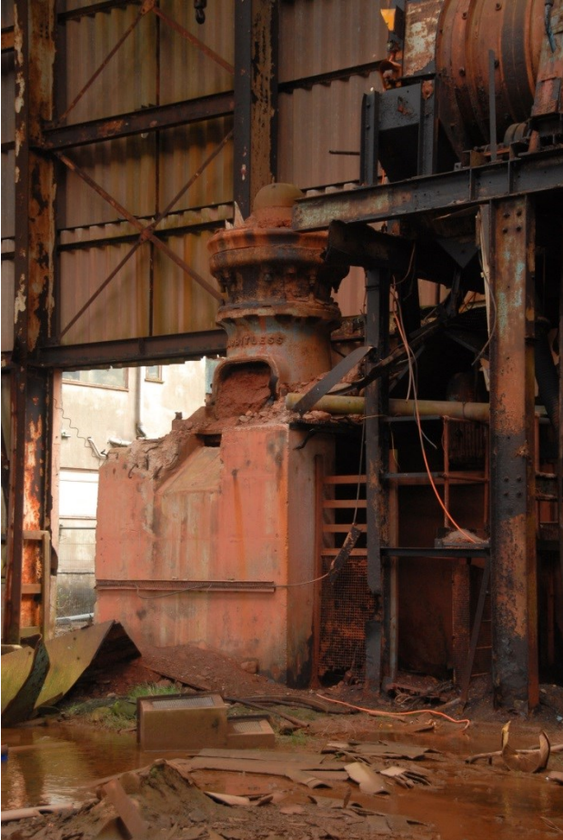
Fig 11. The large cone crusher in situ within the primary crusher building.
