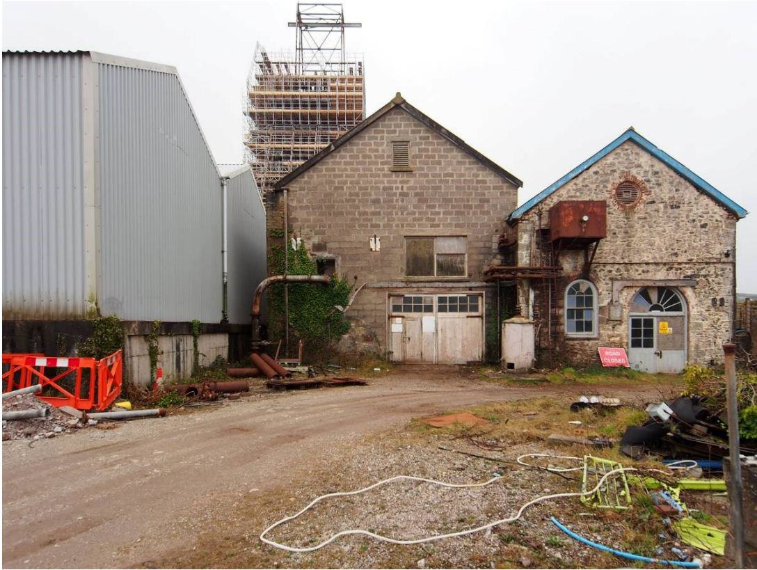
Fig 31. The original South Crofty air compressor houses.
