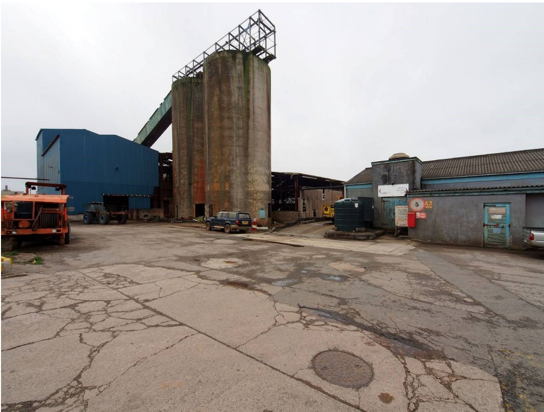
Fig 28. The north eastern corner of the mill, showing the Humphrey spiral building (left), fine ore bins and conveyor (centre) and maintenance workshop (right).
