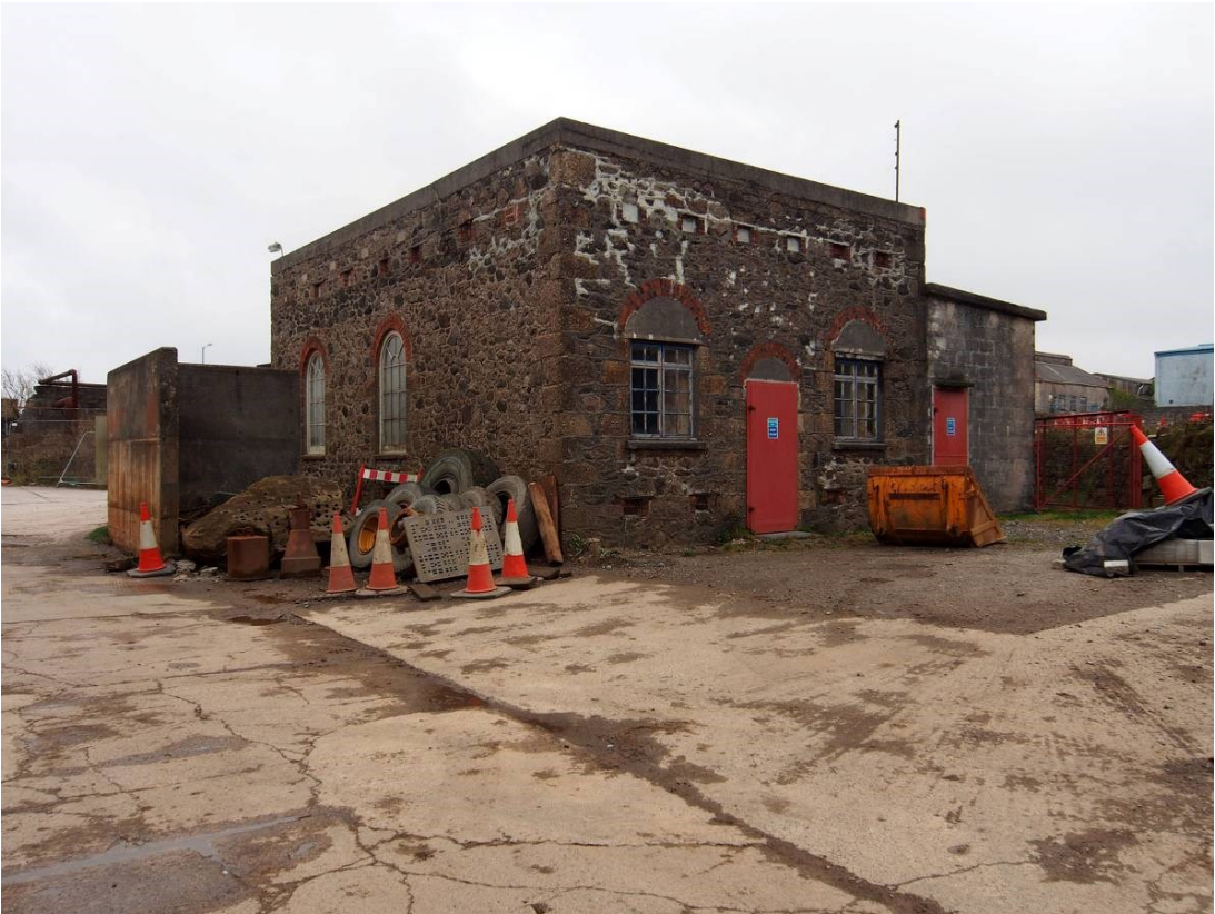
Fig 30. Another view of the South Crofty substation building adjacent to the former mine entrance road.
