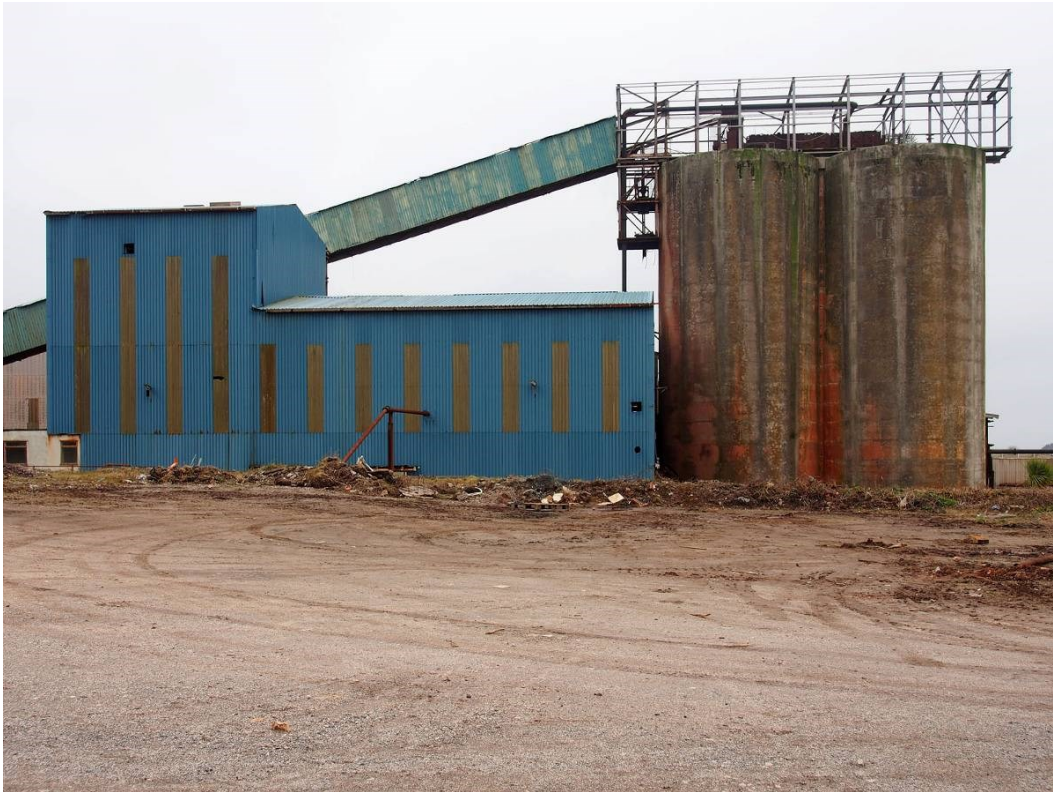
Fig 16. The Humphrey spirals building, ore conveyer and fine ore bins from the east.
