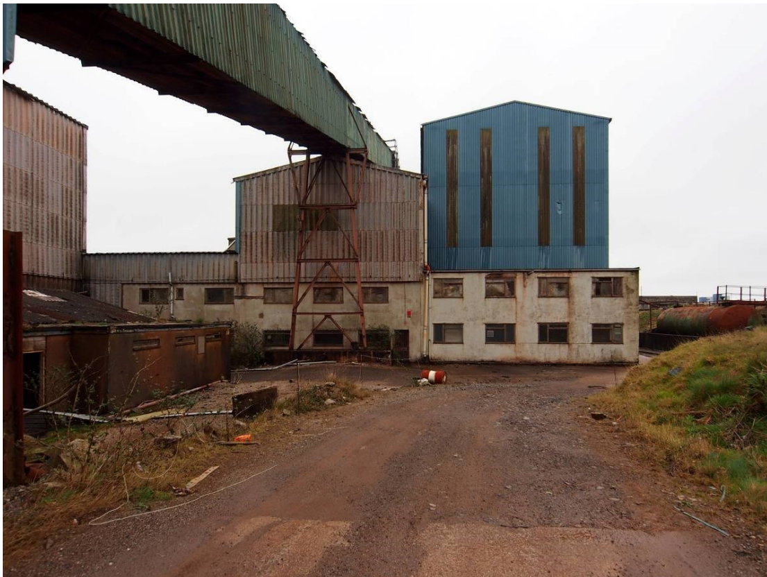
Fig 14. The north eastern section of the mill, showing the conveyor to the fine ore bins and the Humphrey spiral plant. The building to its left housed ball mills.
