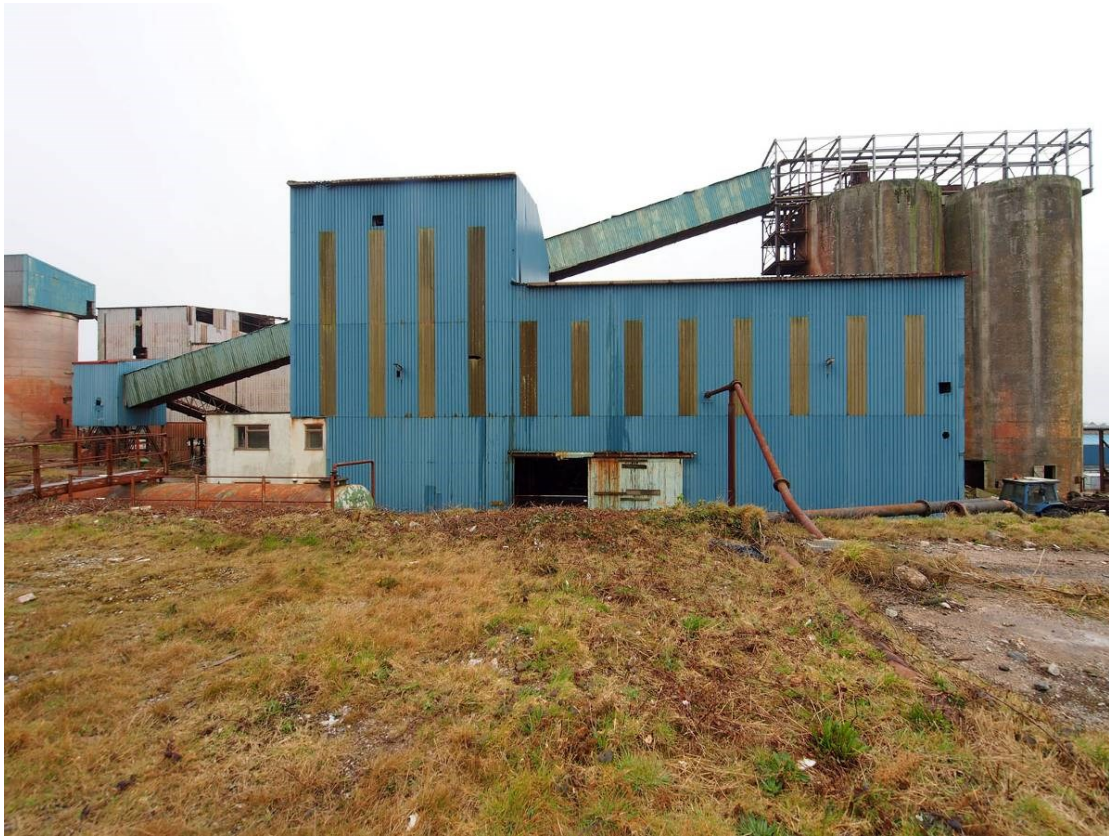
Fig 13. The north eastern part of the mill, showing the conveyor from the western section of the plant to the fine ore bins, as well as the building housing the Humphrey spirals.
