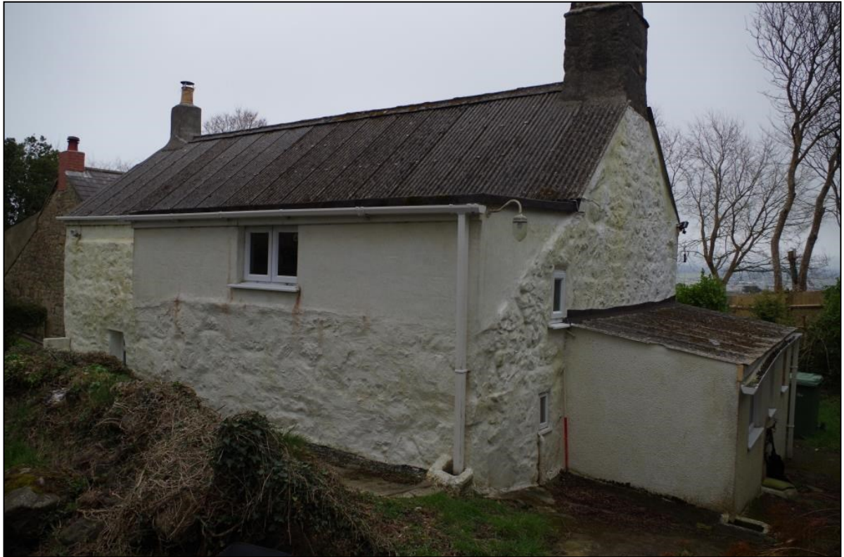
Figure 23: The west and south rear elevations of Building 4 with the modern bathroom extension to the south and partly historic west extension.
