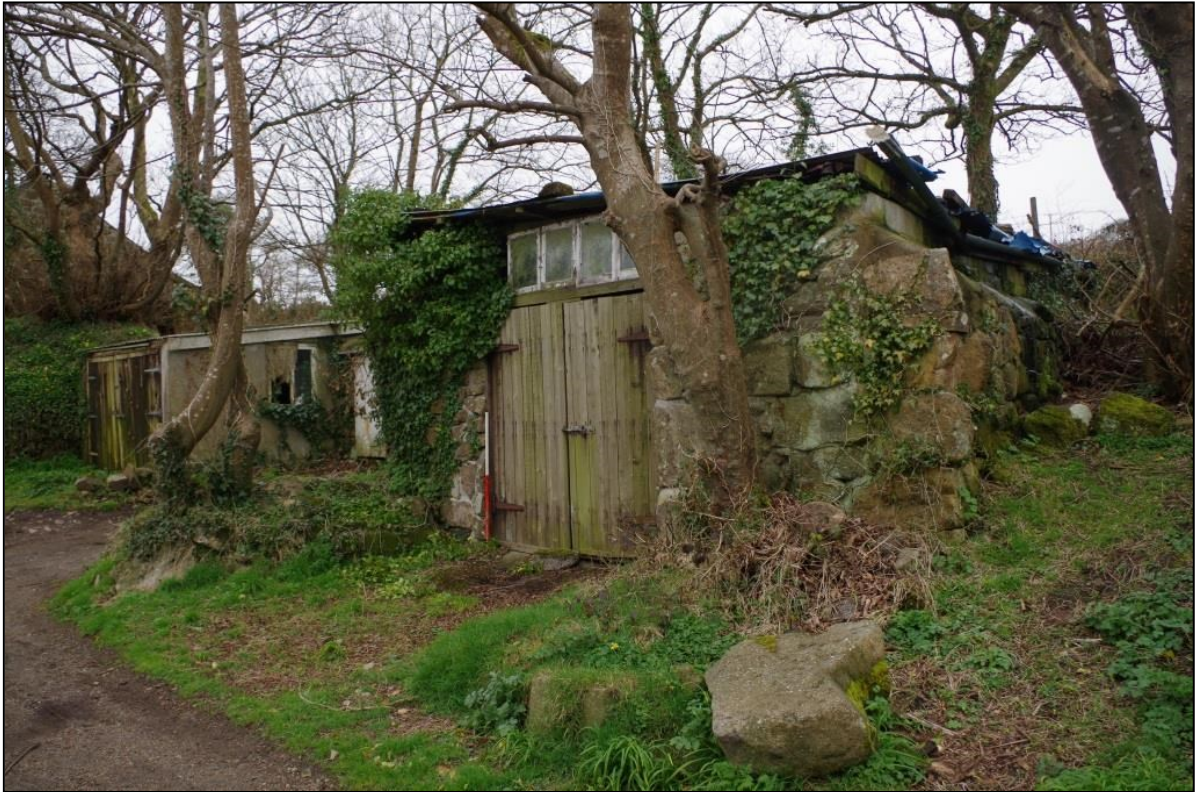
Figure 21: The east and north elevation of Building 2 with a modern doorway and additional walling on the north side.
