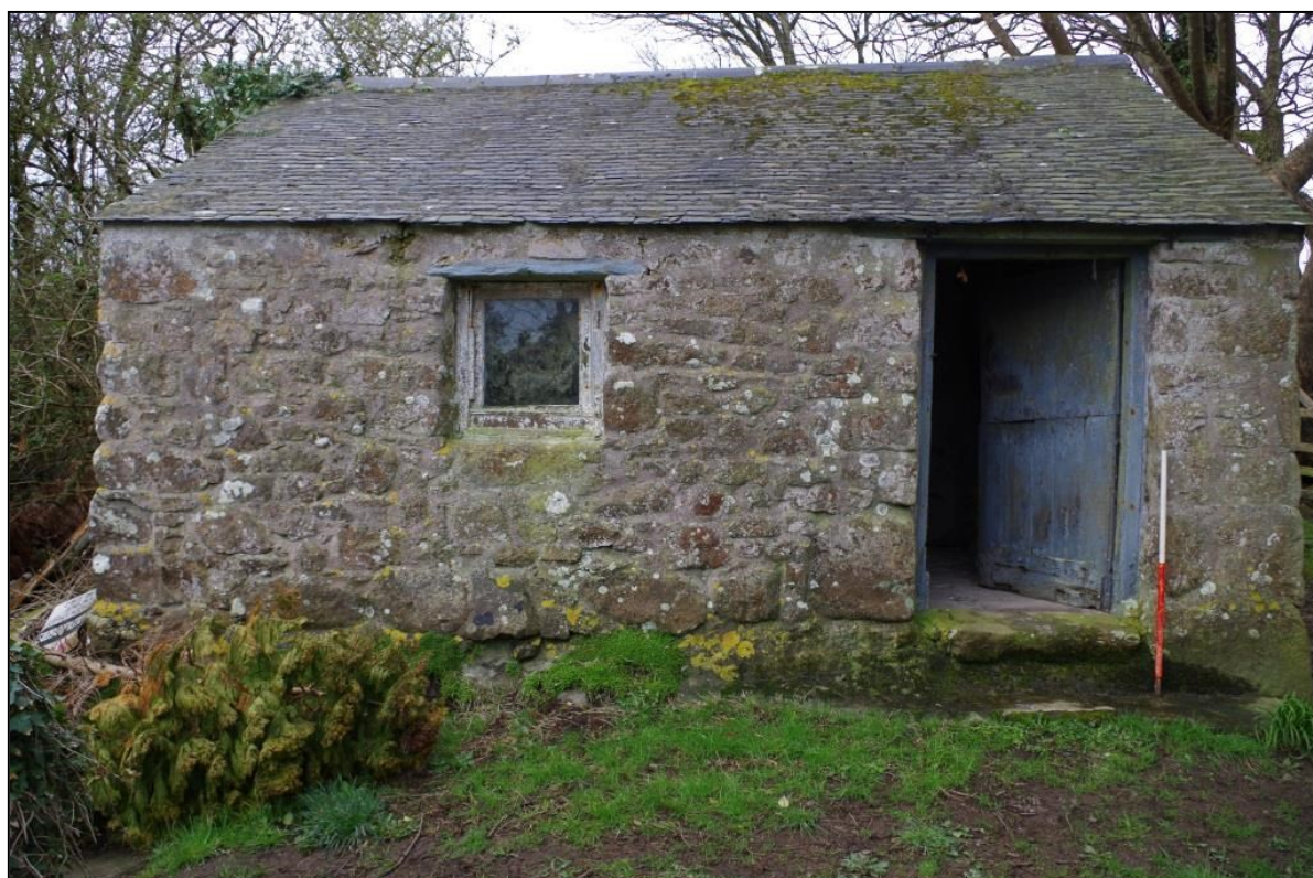
Figure 29: The north elevation of Building 6 with the high threshold step and slate roof.
