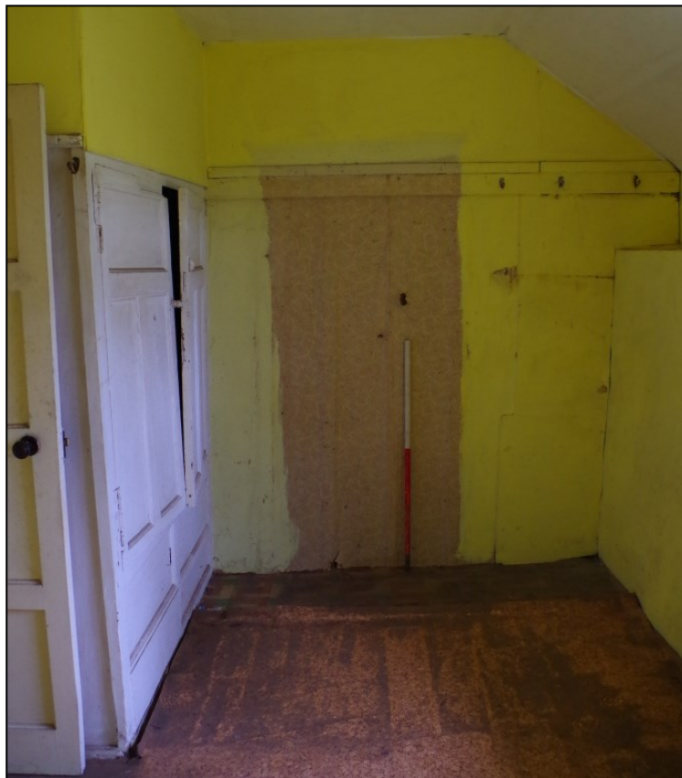
Figure 26: The first floor southern room of Building 4 looking north towards the dividing wall. The beige patch helpfully indicates a wood panel that may block a former doorway between the two upper storey rooms.
