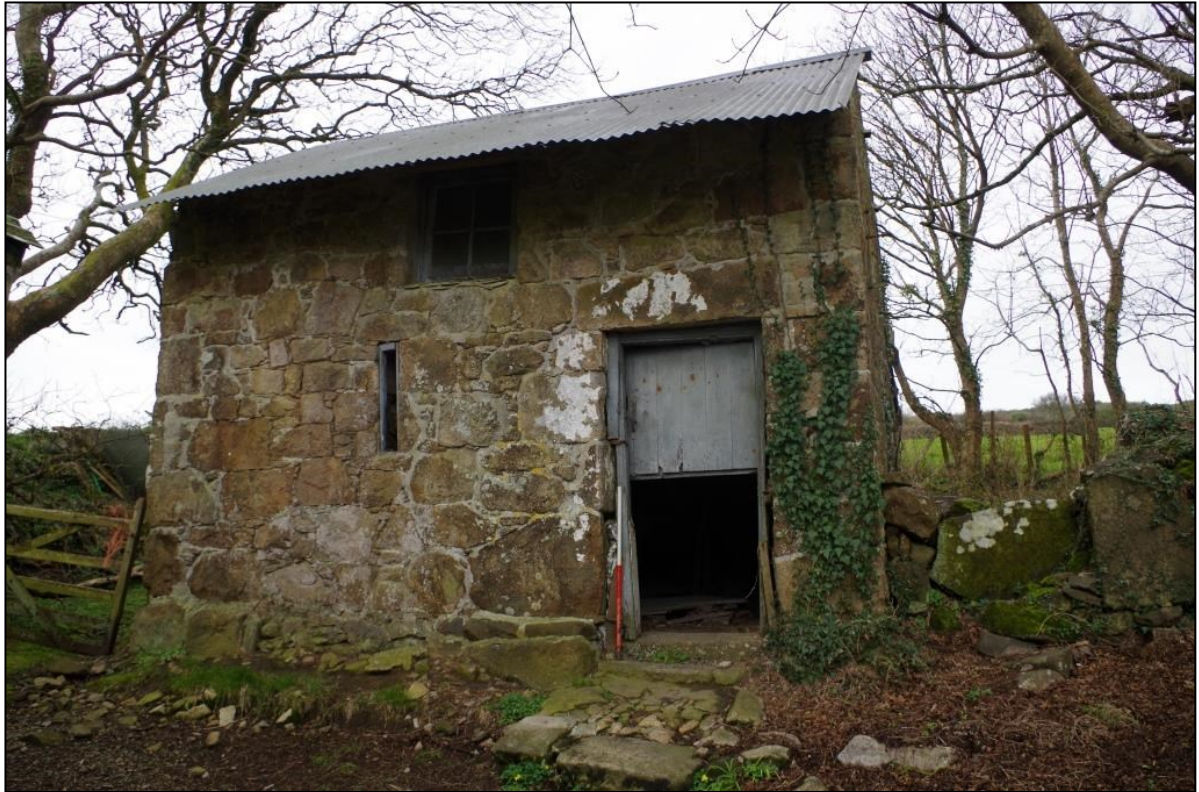
Figure 27: The eastern elevation of Building 5. Note the stable door with cobbled path, slit ventilation on the ground floor and larger window on the upper storey.
