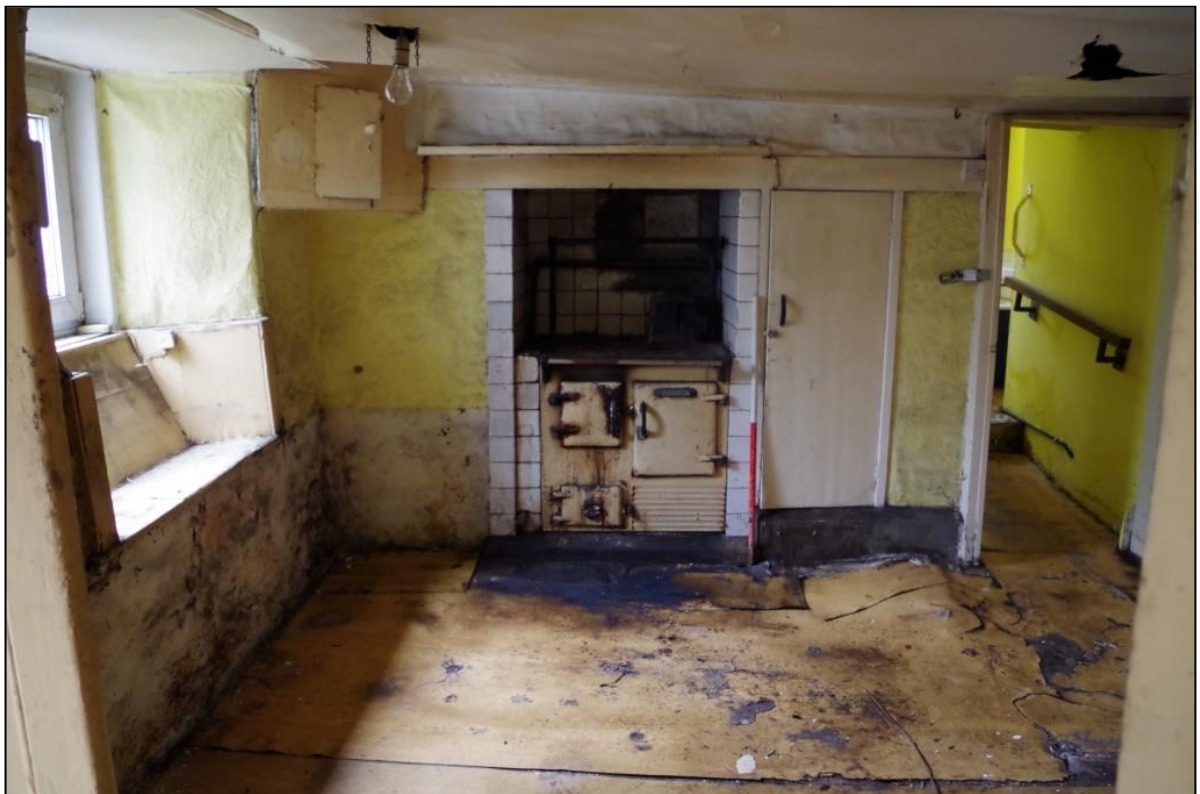
Figure 24: The southern ground floor room of Building 4 with the recessed cooking area. Note also the splayed window, passage to the bathroom and granite steps under the oven.
