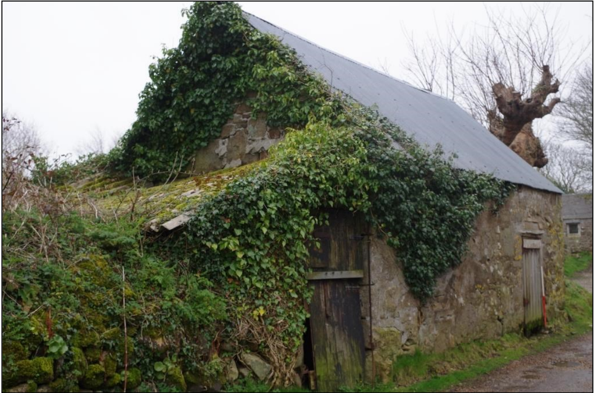
Figure 19: The north and west elevations of Building 1. Note the lean-to, steeply pitched roof and blocked opening obscured by ivy.
