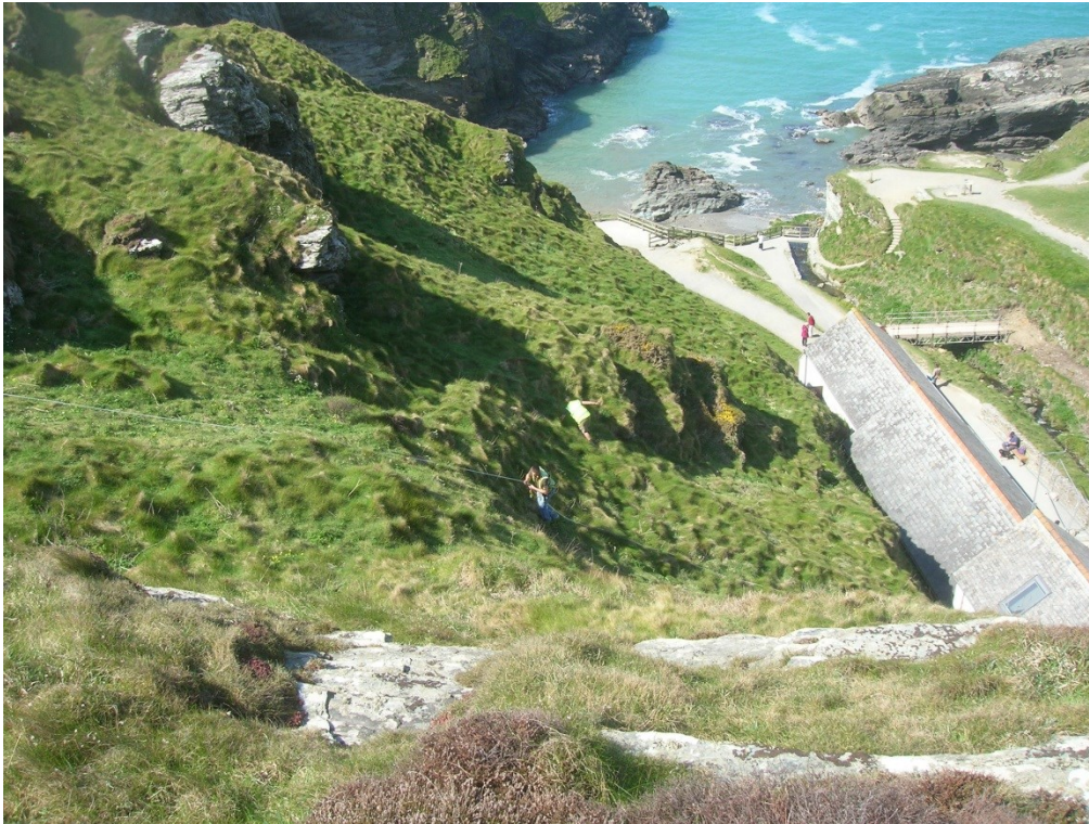
Figure 12. Photograph of the course of the service cable trench down the valley side, clearly showing one, possibly two terraces cut into the valley side.
