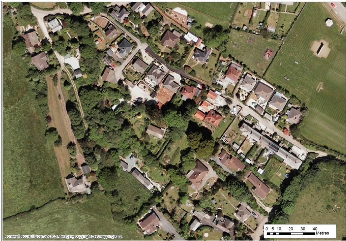
Figure 7. Aerial view of site taken in 2005 showing numerous trees within garden and on property boundaries.
