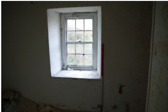
Fig 81 Interior bedroom 4 looking west with inserted 19 th century window opening
