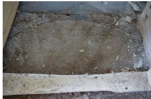
Fig 38 Half 19 th century millstone reused as threshold between wash house and kitchen
