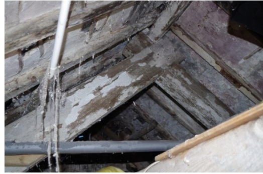
Fig 36 wash house roof structure looking west
