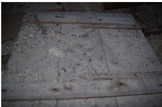
Fig 83 Interior loft hatch door (probably reused shutter)
