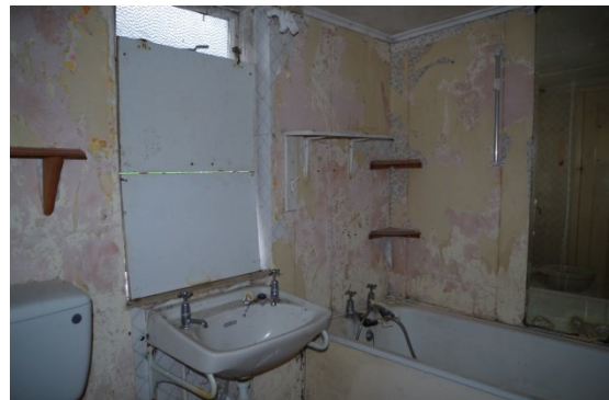
Fig 63 Interior bathroom looking south-west
