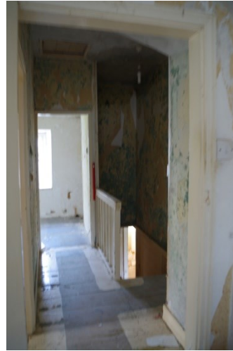
Fig 68 Interior landing looking west
