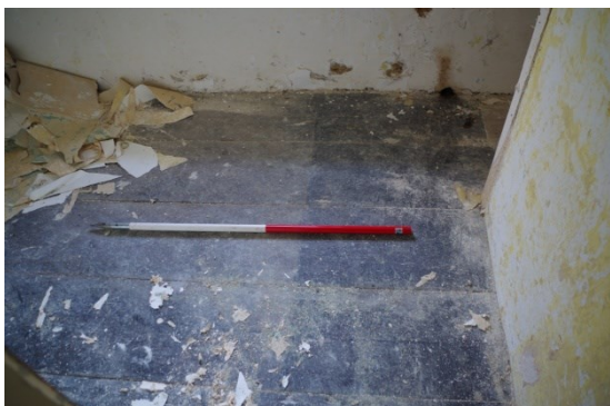
Fig 82 Interior bedroom 4 wide floorboards
