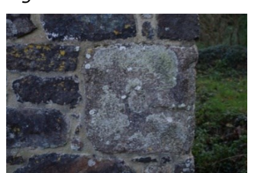
Fig 31 Reused centre of composite millstone
