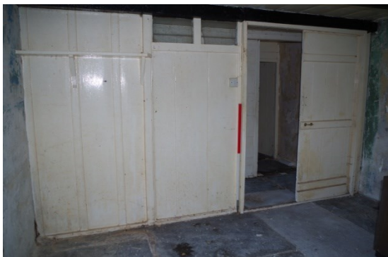
Fig 42 Interior kitchen looking south showing 18 th or early 19 th century planked wall
