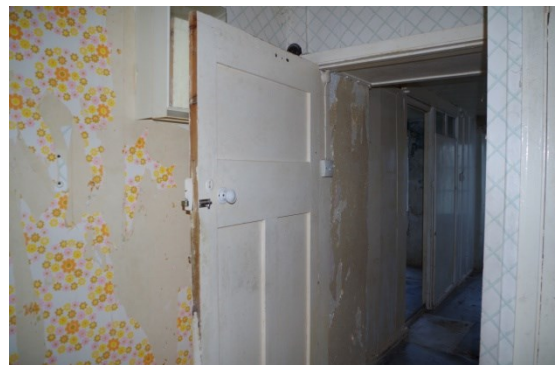
Fig 62 Interior bathroom looking east
