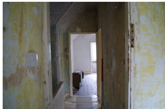
Fig 69 Interior landing looking east
