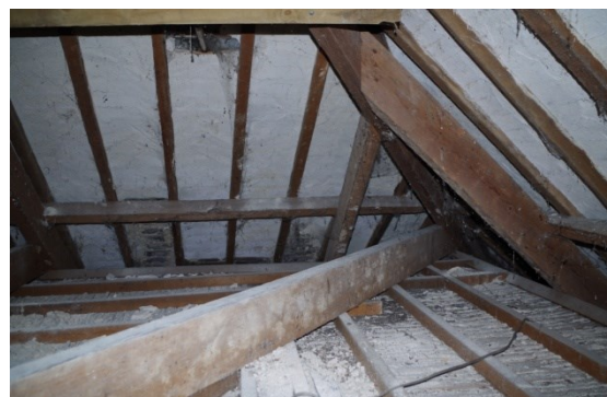
Fig 87 Roof timbers looking south at south-west corner
