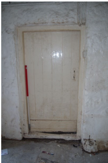
Fig 35 Former back door from kitchen showing differing wall widths either side
