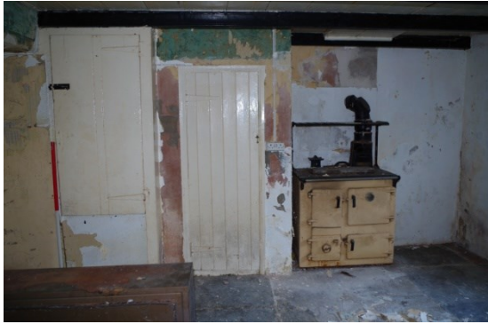
Fig 40 Interior kitchen looking north
