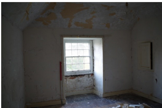
Fig 74 Interior bedroom 2 looking east
