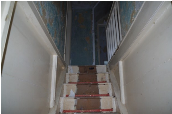
Fig 66 Interior staircase looking east
