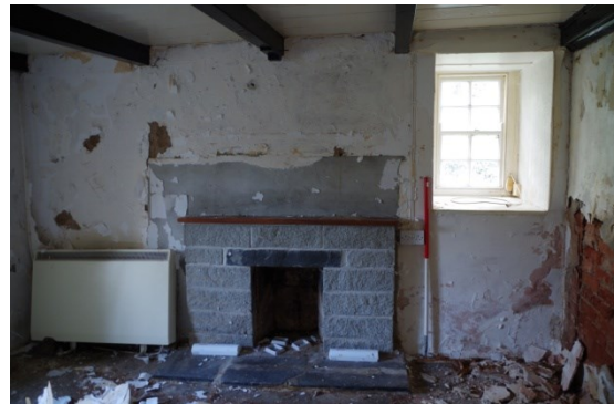
Fig 53 Interior living room looking south
