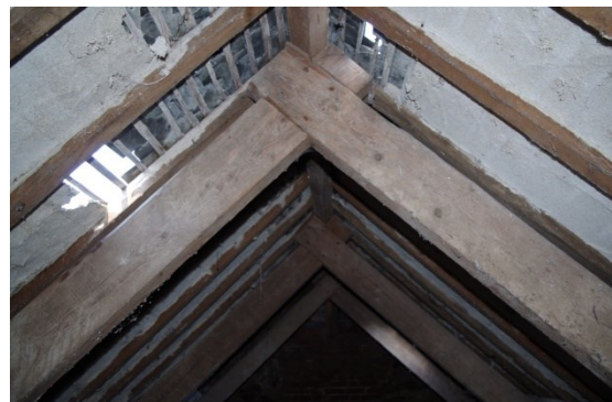
Fig 85 Roof timbers looking north
