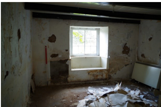
Fig 51 Interior living room looking east
