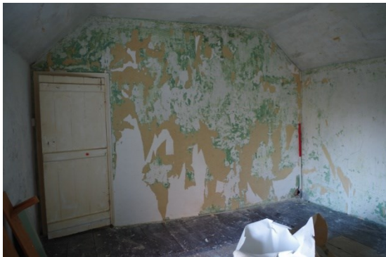
Fig 73 Interior bedroom 1 looking south-west
