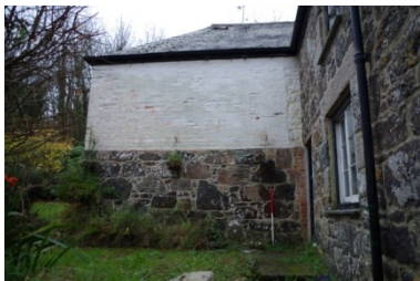
Fig 22 North elevation of east wing
