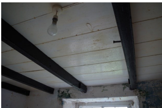
Fig 43 Interior kitchen showing early joists
