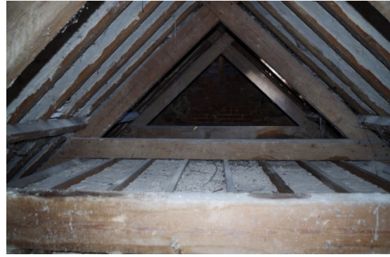
Fig 84 Roof timbers looking north to brick wall at north end
