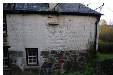
Fig 29 South elevation of east wing
