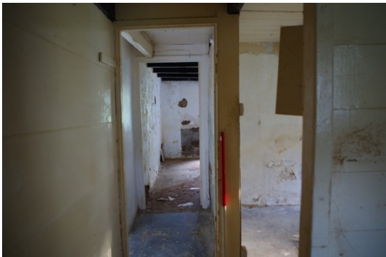
Fig 49 Interior hall south of stairs looking east
