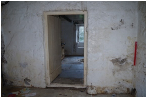
Fig 34 Interior wash house looking east
