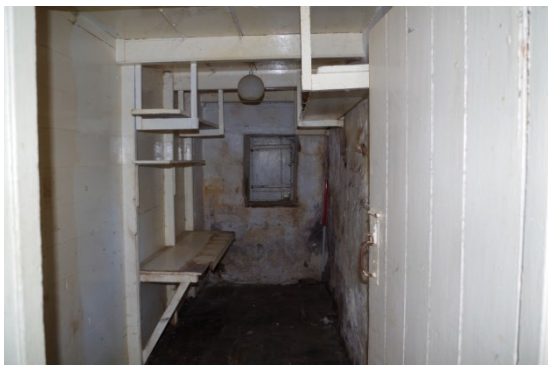
Fig 59 Interior store room looking south with original window opening
