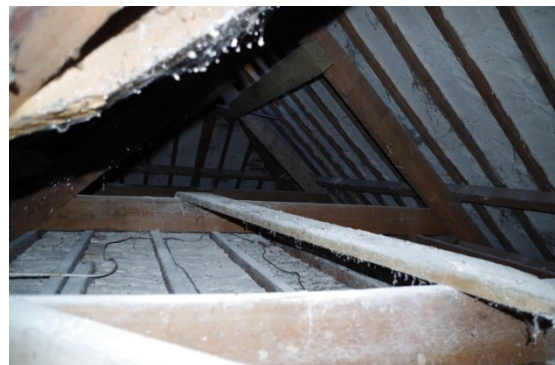
Fig 86 Roof timbers looking east into east wing
