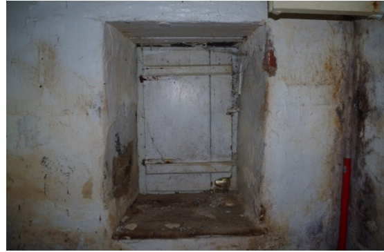
Fig 60 Interior store room original window opening in south wall
