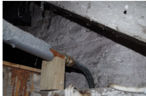
Fig 37 wash house roof space looking east
