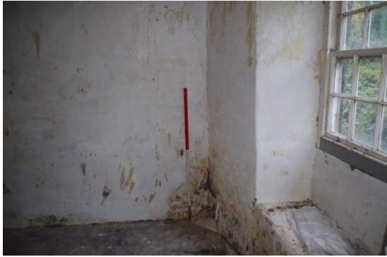
Fig 56 Interior study showing remaining base of demolished front wall
