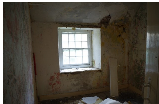
Fig 78 Interior bedroom 3 looking south
