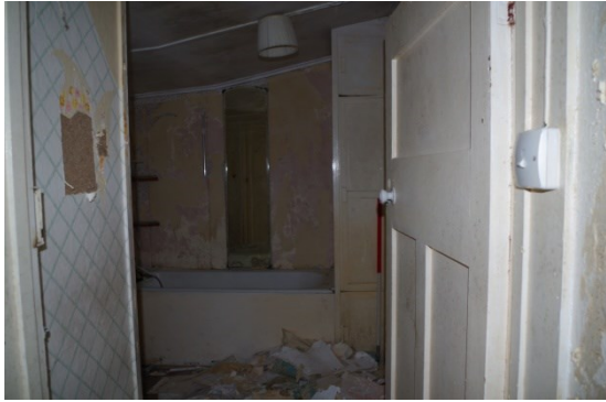
Fig 64 Interior bathroom looking west
