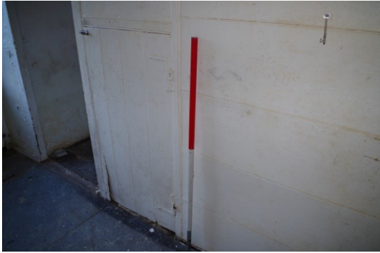
Fig 48 Interior below-stairs cupboard in hall
