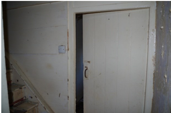
Fig 65 Interior base of stairs looking south
