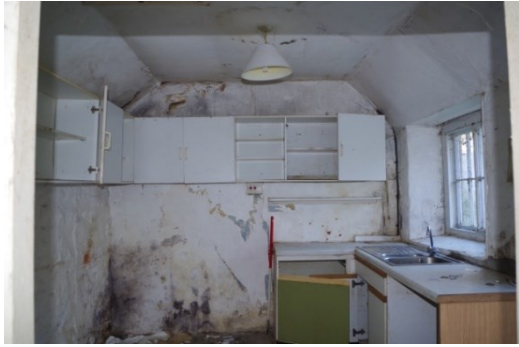
Fig 32 Interior wash house looking west
