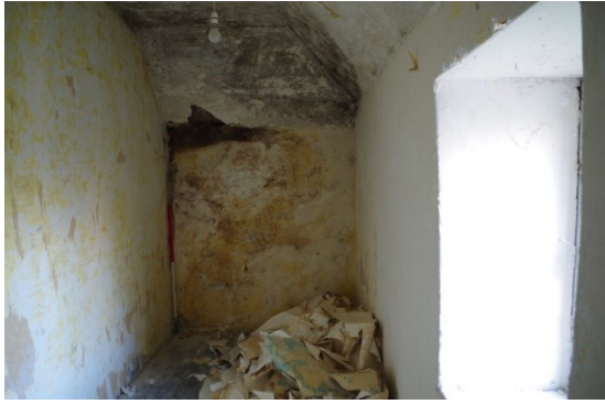
Fig 80 Interior bedroom 4 looking south
