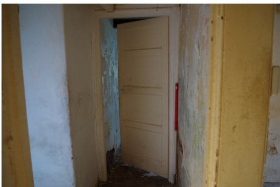
Fig 50 Interior hall south of stairs looking east
