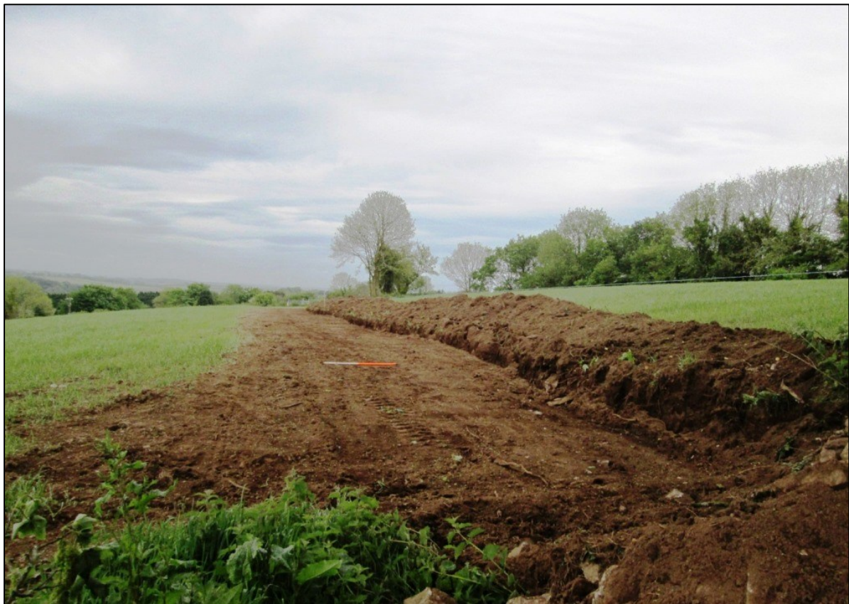
Fig 8 View from the west after excavation track remediation works (28/5/2014) © CAU.
