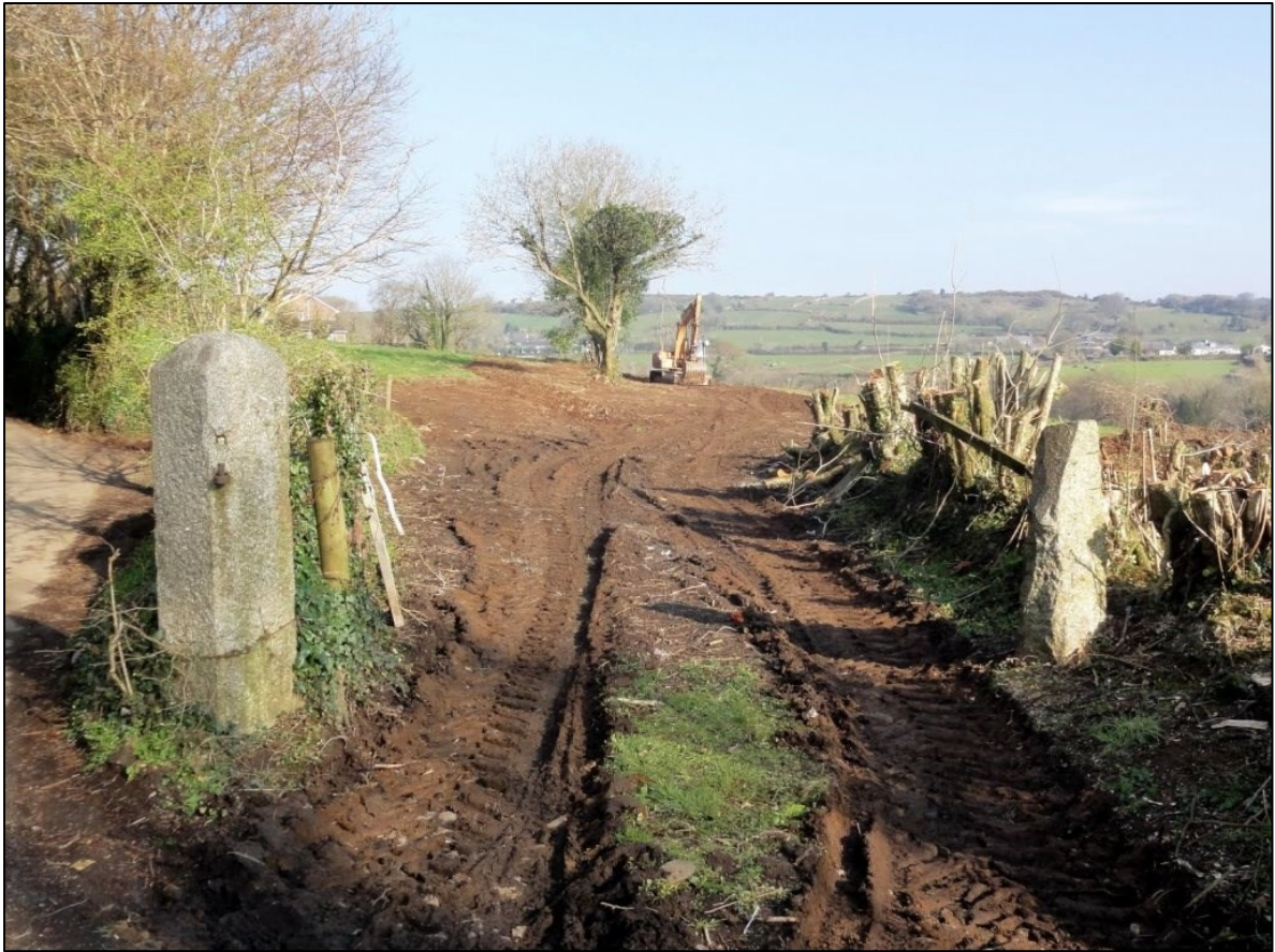
Fig 5 View from the east of the former LCR hedge after removal (10/4/2012) © WHS.
