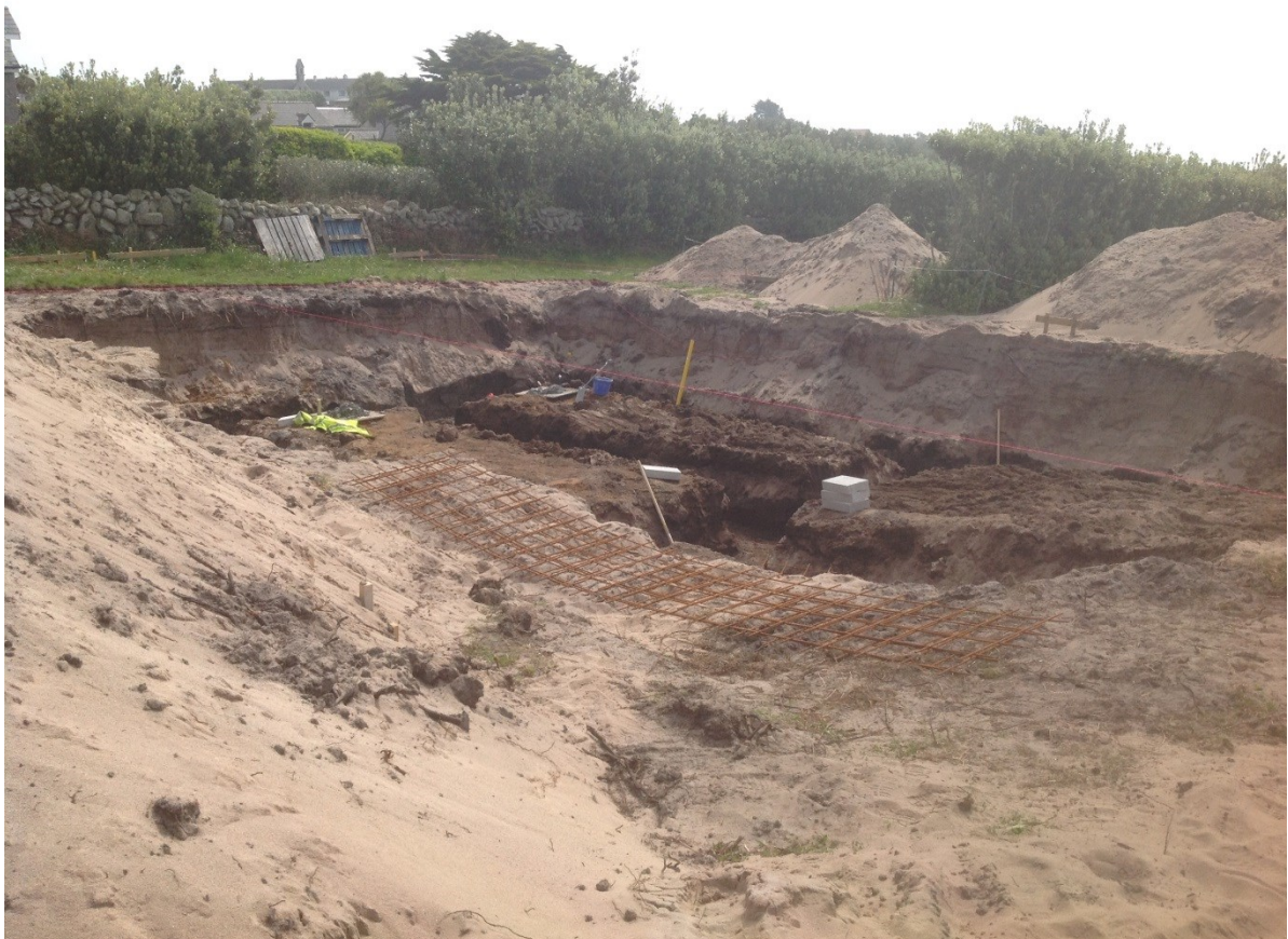
Fig 4 Overview of the building site.
