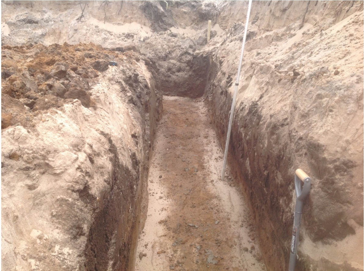
Fig 3 One of the foundation trenches, showing the depth of sand.
