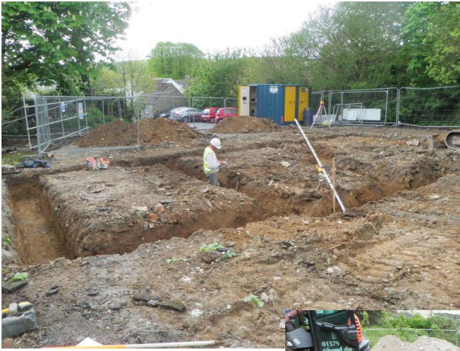
Fig 14 Looking south across the southern house foundation trenches.
