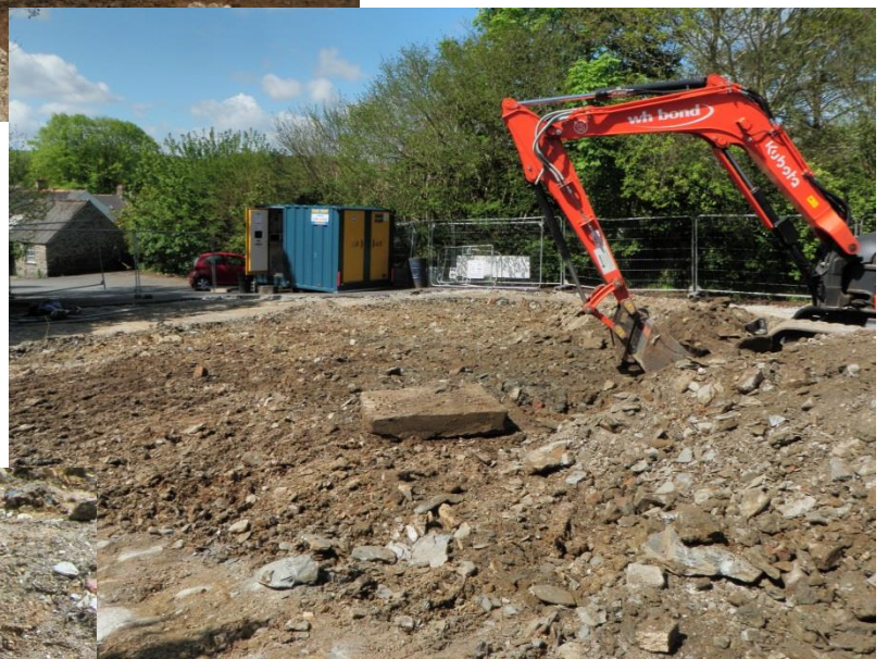
Fig 11 Looking south-west across the southern area showing layer (2) demolition layer.
