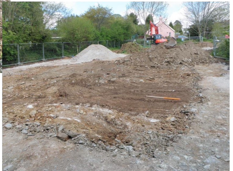
Fig 13 Looking north, showing drain (3) and soil (6) – right.
