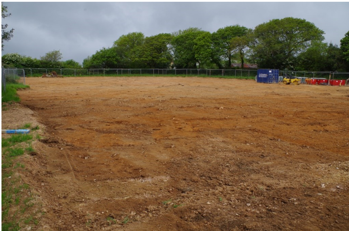
Fig 6 The completed topsoil strip of the development area at Lower Hugus.
