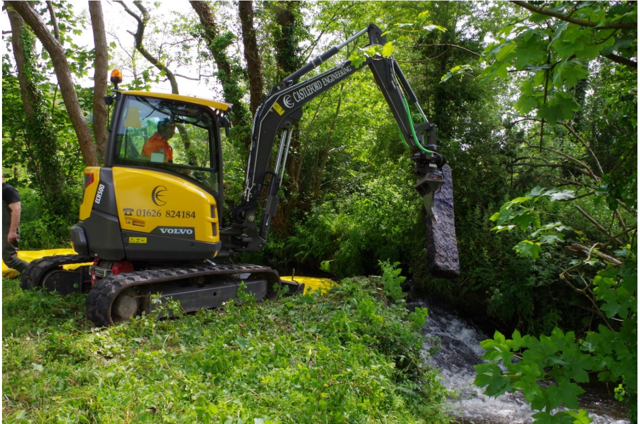
Fig 13 Removal of one of the granite capstones
