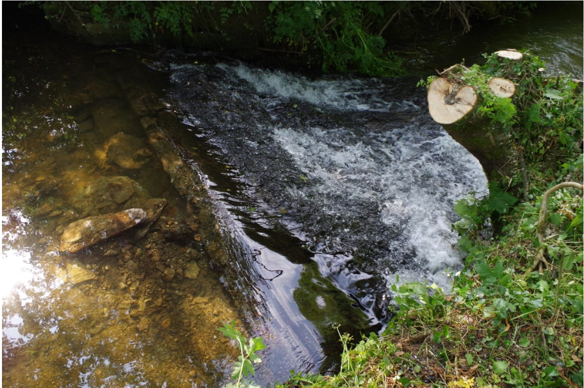
Fig 9 Weir before deconstruction looking east
