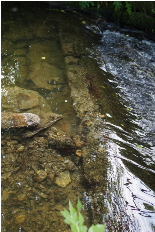
Fig 10 Capstones looking east prior to deconstruction
