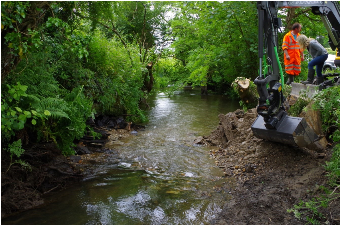
Fig 16 River looking south following the removal of the weir
