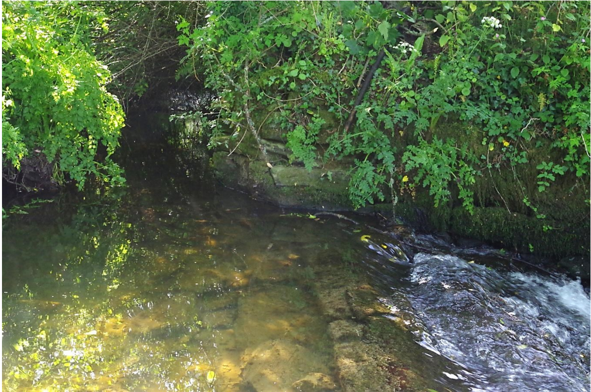
Fig 11 Eastern riverbank retaining wall
