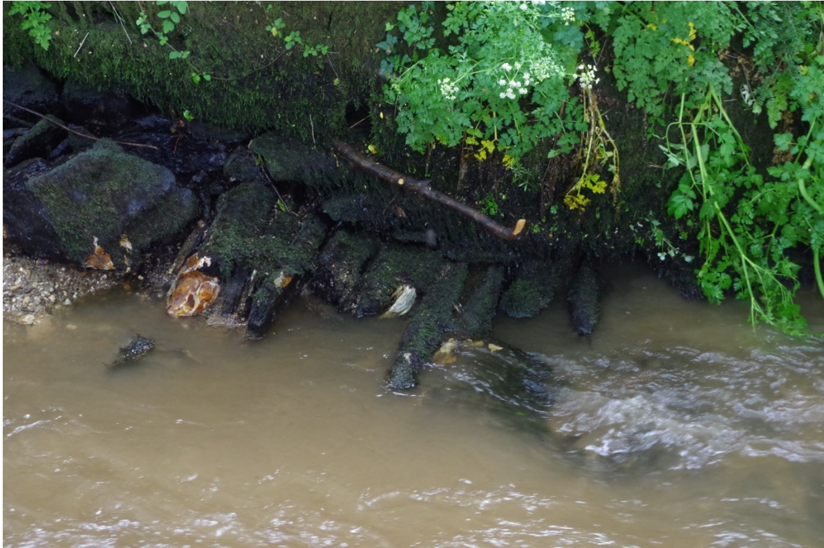
Fig 15 Remnants of the vertically set stones forming the sloping part of the weir secured below the retaining wall along the eastern bank
