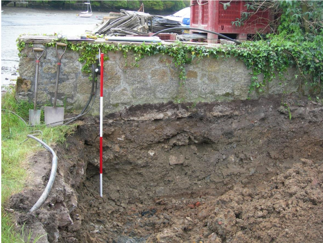
Fig 10 North east end of the landward face of the wall on the historic quay, used to define the Listing, (sited on the clay body of the quay, cut by the works)
