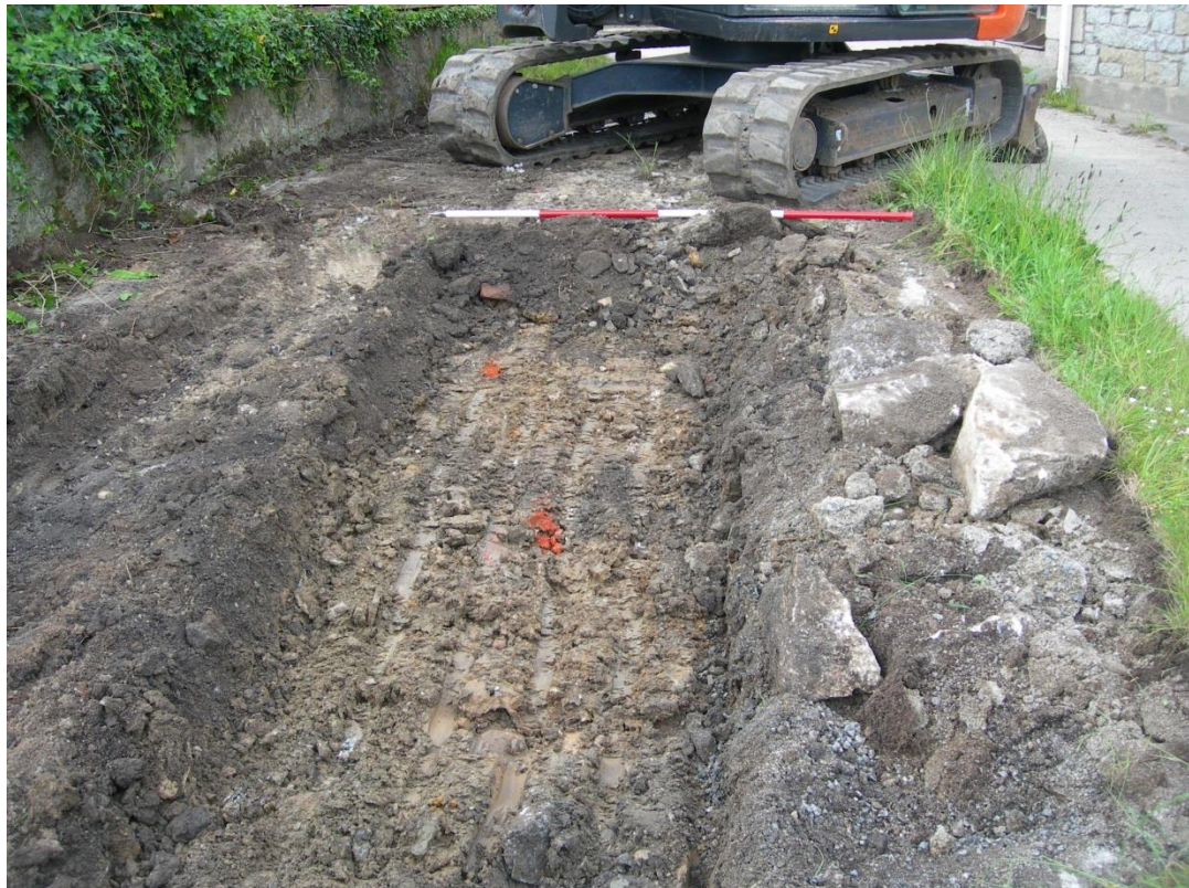
Fig 7 Layer 4, the yellowy clay with occasional brick laid to form the body of the historic quay behind its stone facing, in the centre of the works, seen from the north east The concrete to the right is from layer 2, broken and shifted to the edge of the trench.
