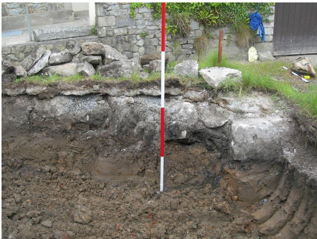
Fig 11 North corner of the works, with large granites bedded on the clay of the quay
