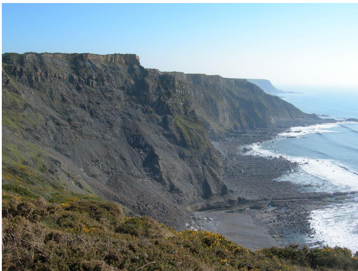
Fig 3 Cliffs showing the prominent, vulnerable, pale cap of sandstone at Embury Beacon
