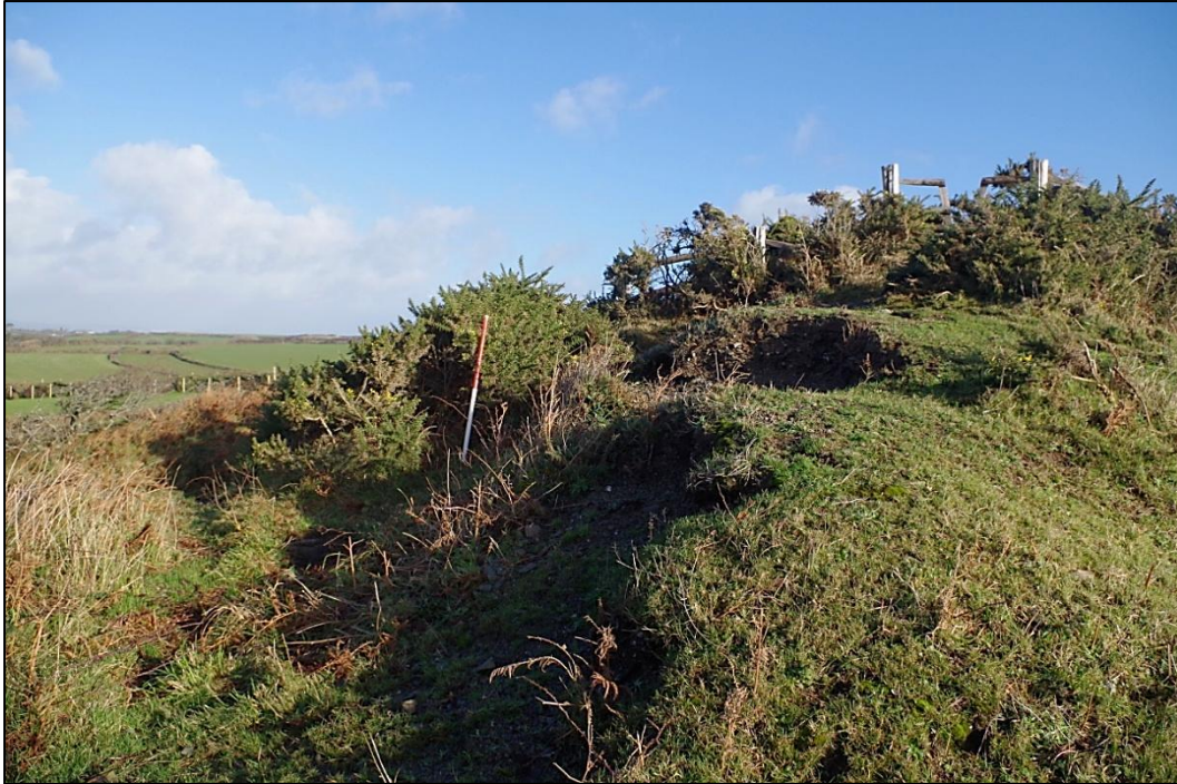
Fig 11 Looking northeast across the western section of The Bulwarks on the west side of Dodman Point. The coastal path crosses the ramparts here and walkers and stock movement have caused severe erosion to the profile of the ramparts in this area
