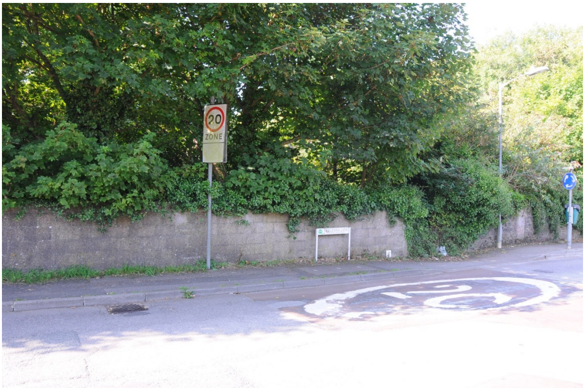
Fig 28. The blockwork and stone walls forming the northern boundary of the proposed development site.
