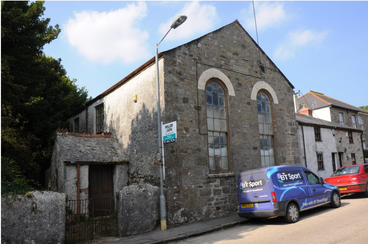
Fig 37. The Grade II Listed former Methodist chapel in Penponds.
