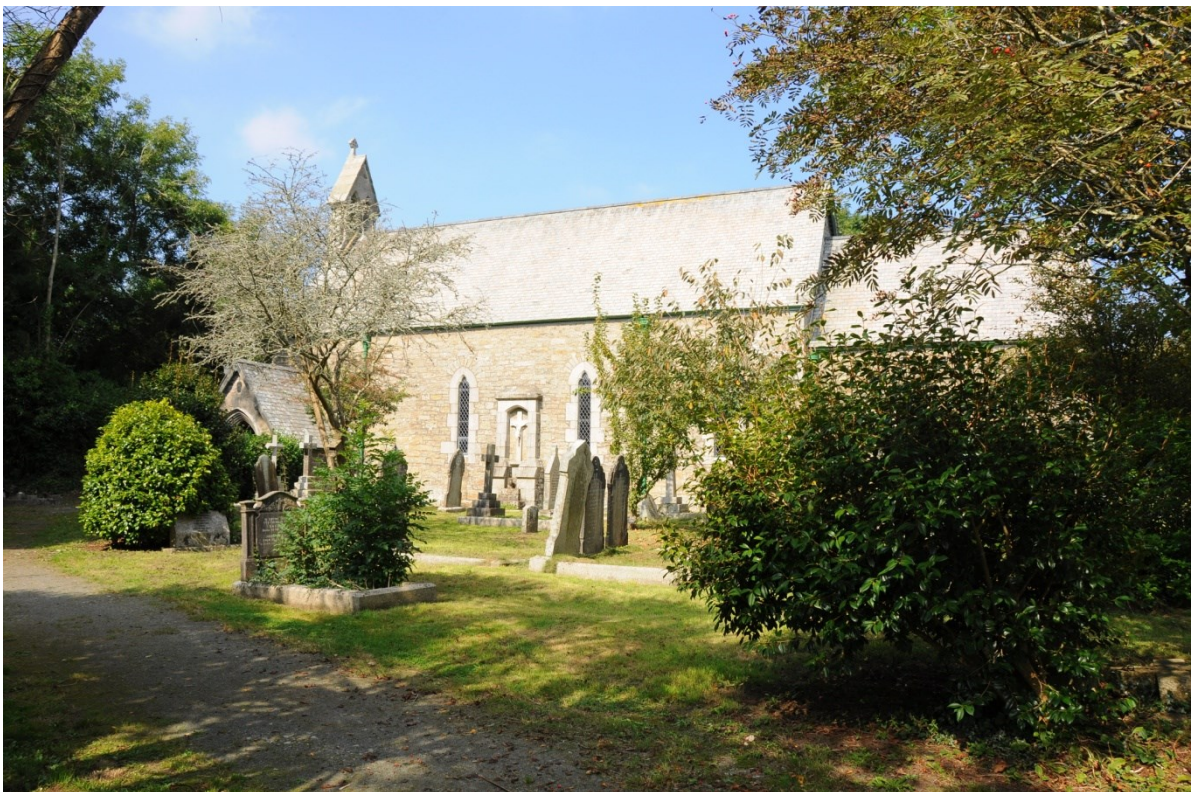
Fig 38. The Grade II Listed early 20 th century church at Penponds.
