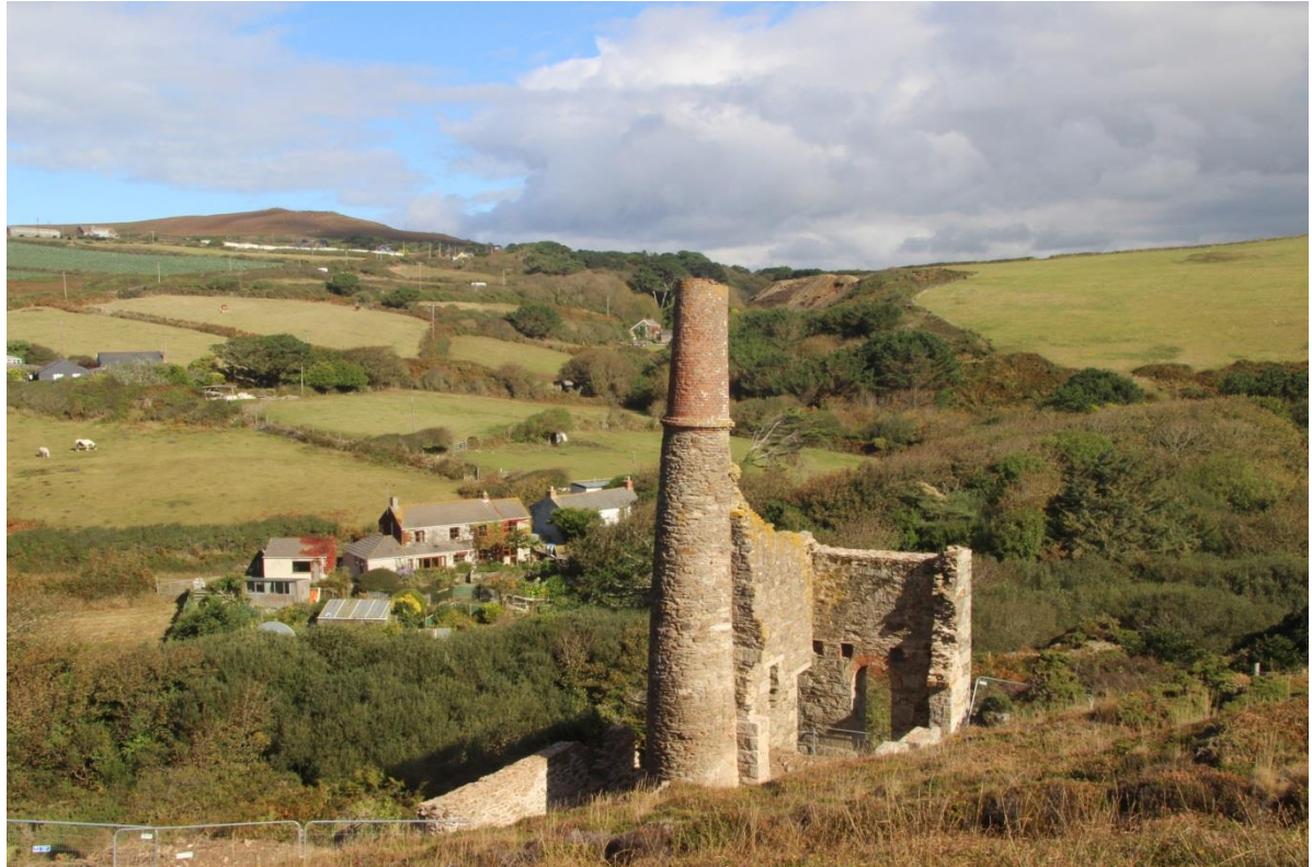
Fig 59. The engine house and boiler house at Charlotte United on completion of the conservation works undertaken to them.
