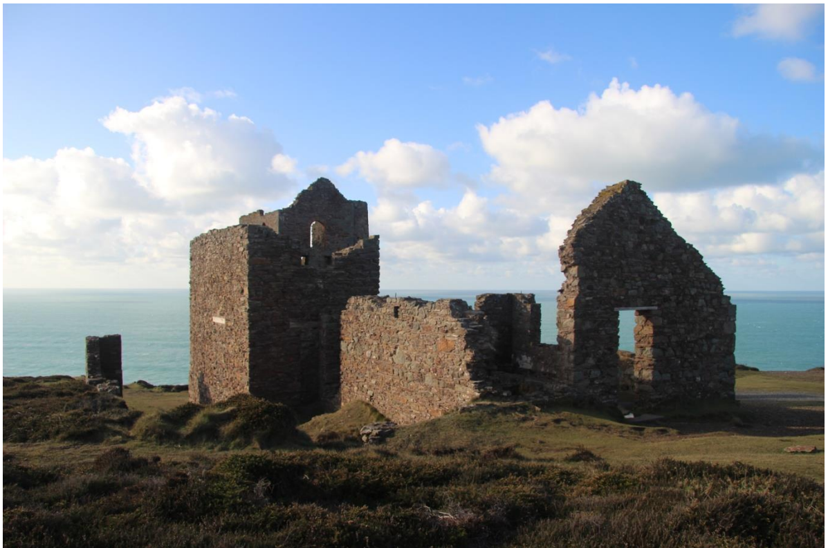
Fig 14. The horizontal whim engine house (right), boiler house (centre) and beam whim engine house (left), with the stamps engine house in the background.
