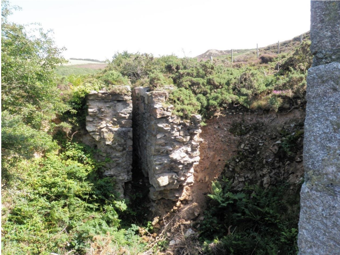
Fig 56. The balance bob mounting adjacent to the coned out shaft at Charlotte United.
