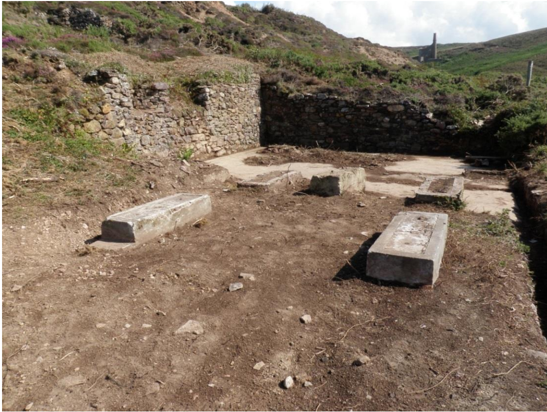
Fig 48. The eastern end of the Old Century Works dressing floors following the clearance of scrub and rubble. The concrete plinths would have supported vanning tables.
