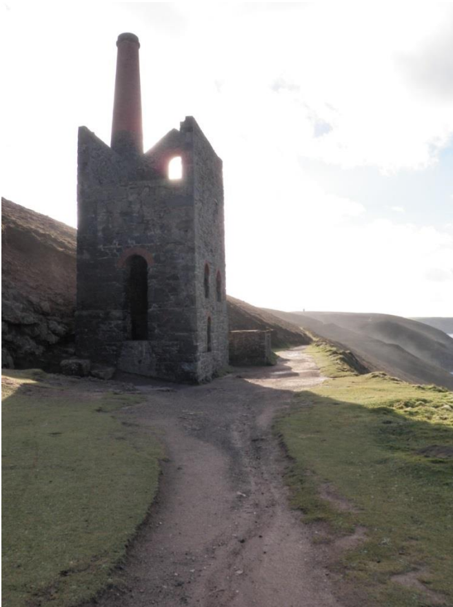
Fig 34. Towanroath engine house and the remains of the later horizontal engine house (foreground). The boiler house is in the shadowed area to their right.
