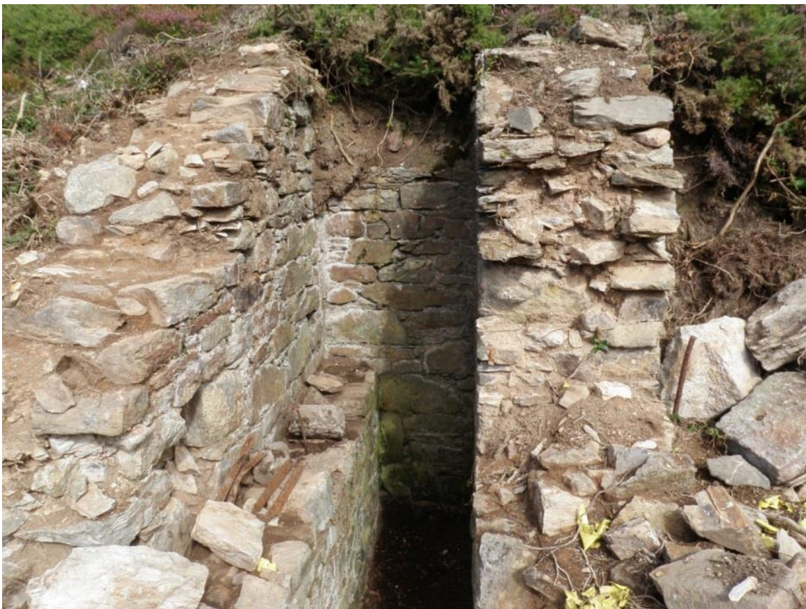
Fig 47. The Old Century Works stamps wheelpit following vegetation clearance but prior to its stabilisation.
