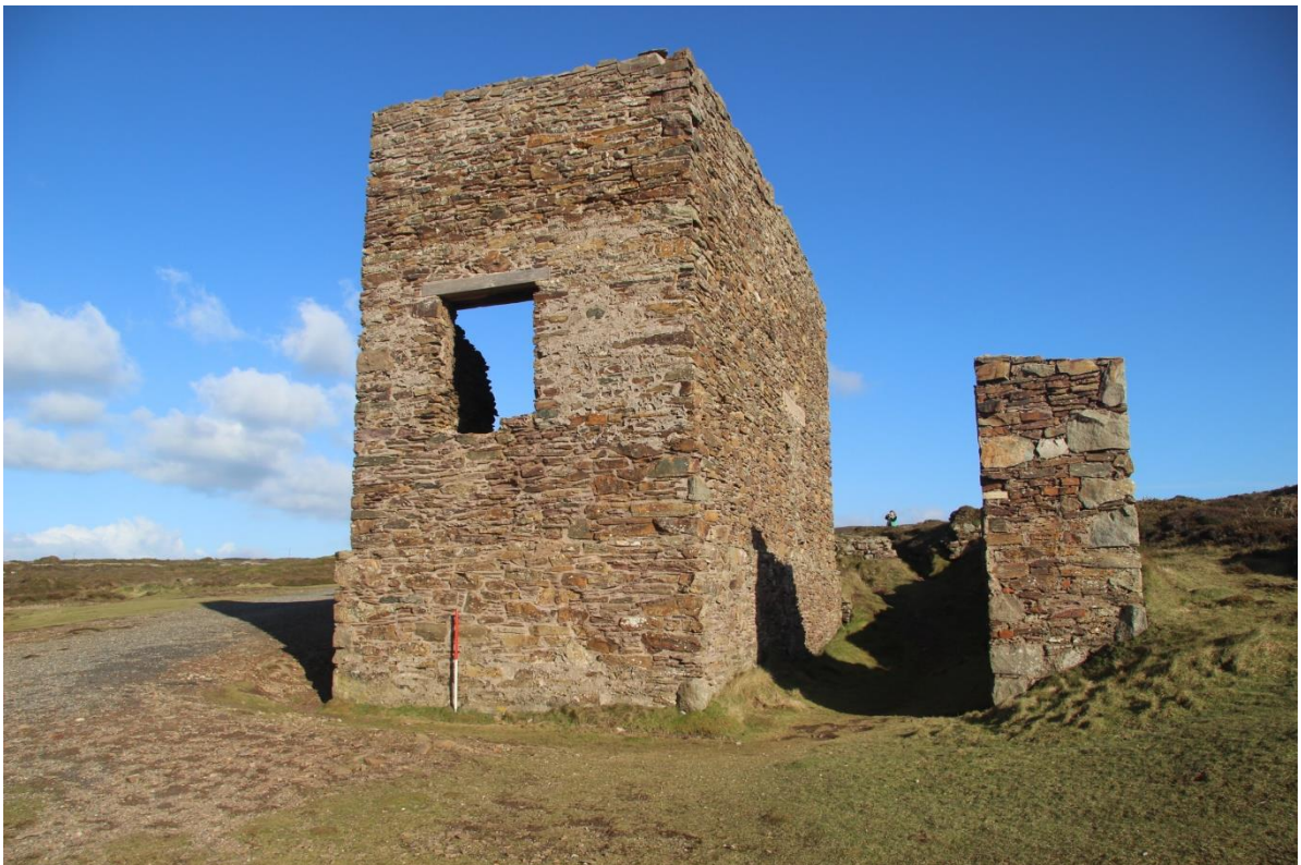
Fig 16. The Western elevations of the all-indoor beam whim engine house (left) and its boiler house (right).
