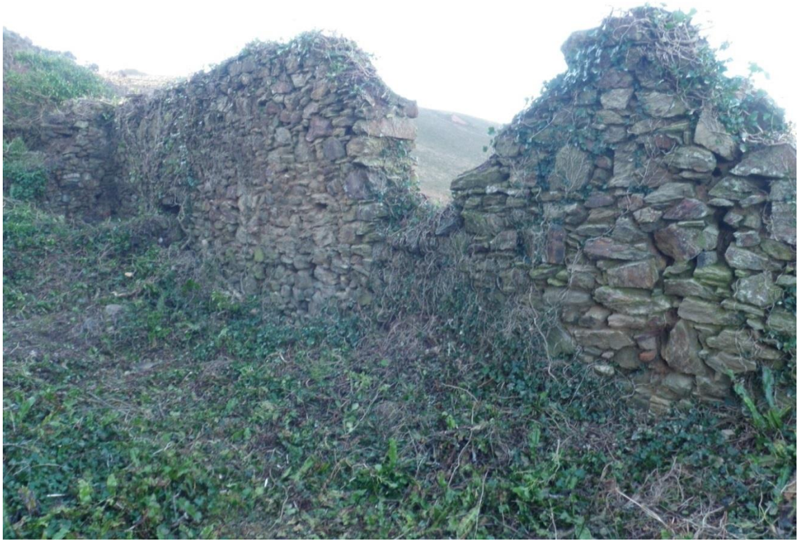
Fig 54. The boiler house at Charlotte United prior to its conservation.
