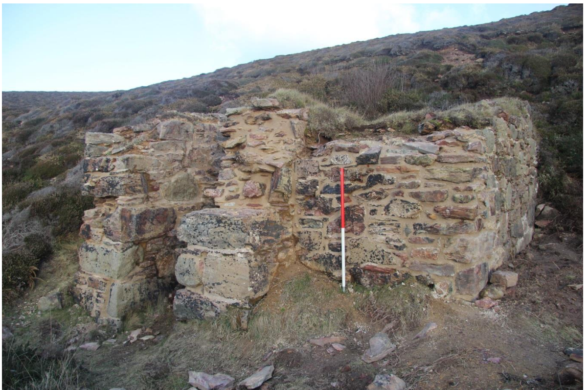
Fig 33. The wheelpit and stamps gear plat following repointing and limited re-building.
