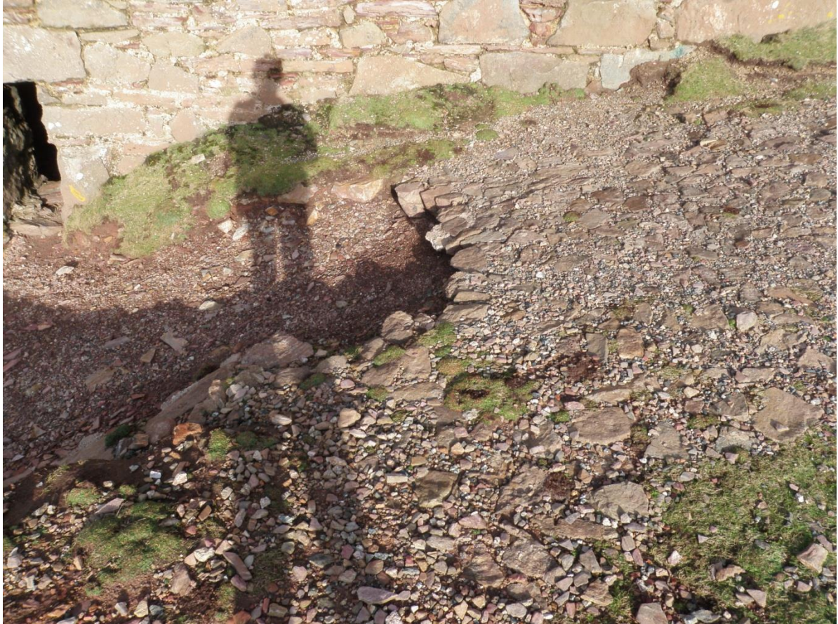
Fig 22. The damaged cobbling at the head of the former tramway from Towanroath Shaft to the whim engine house where it abuts the southern side of the stamps engine house.
