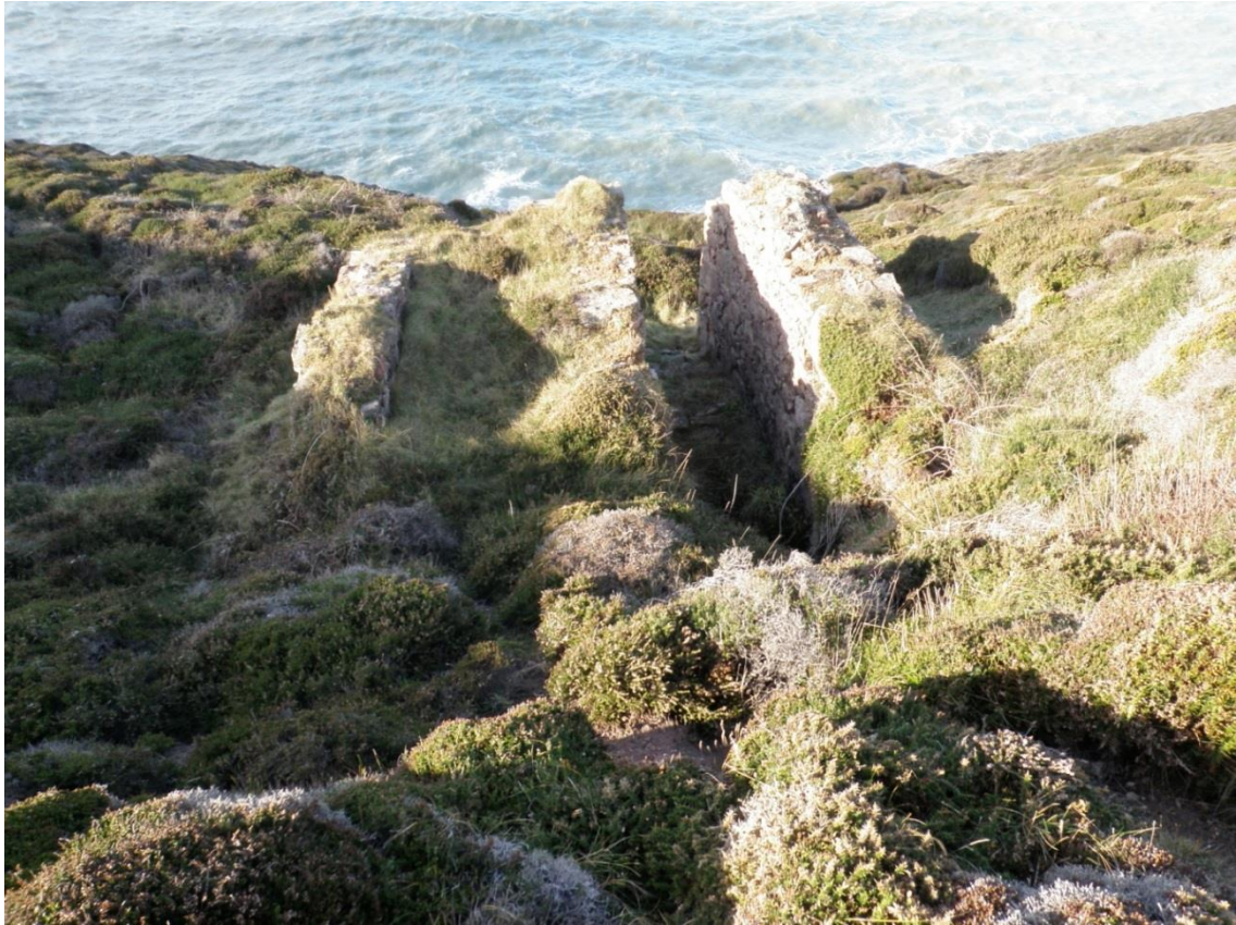
Fig 30. The tributers' stamps wheelpit (right) and gearing platform (left) prior to works.
