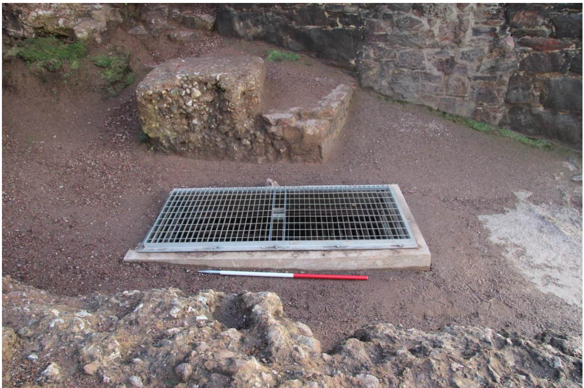
Fig 37. The replacement grille over Towanroath Shaft.
