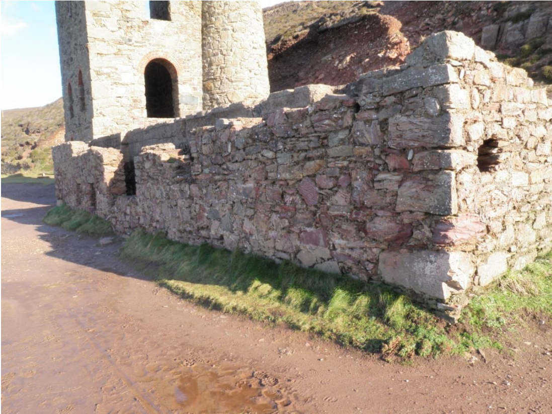
Fig 38. The remains of the 20 th century horizontal engine house constructed to the south of Towanroath engine house.
