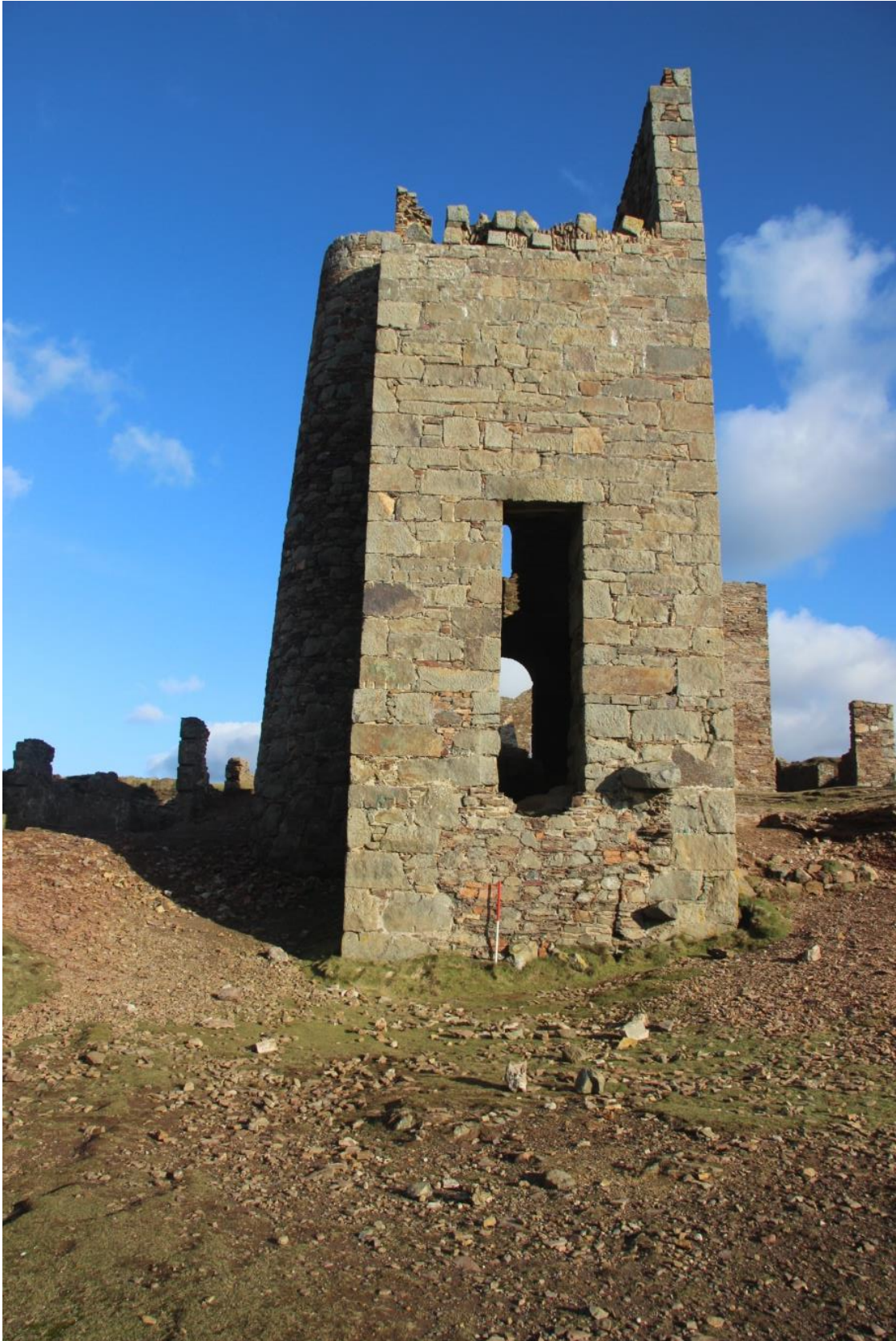
Fig 21. The western elevation of the stamps engine house showing the infill of the scar left when the flywheel loadings were removed and the consolidated collapsed wing way masonry on the head of the bob wall.
