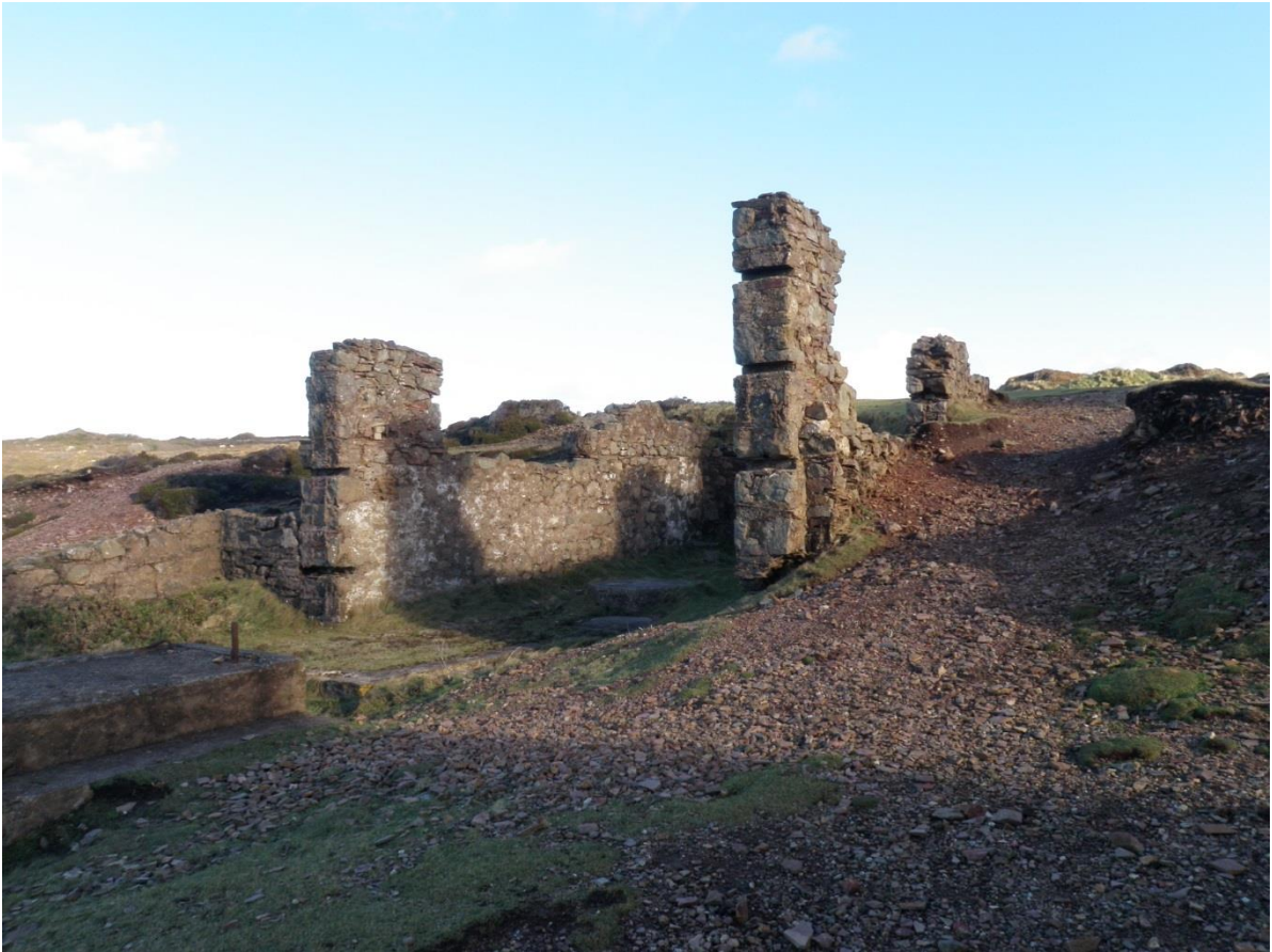
Fig 42. The 20 th century gas engine house at Wheal Coates.
