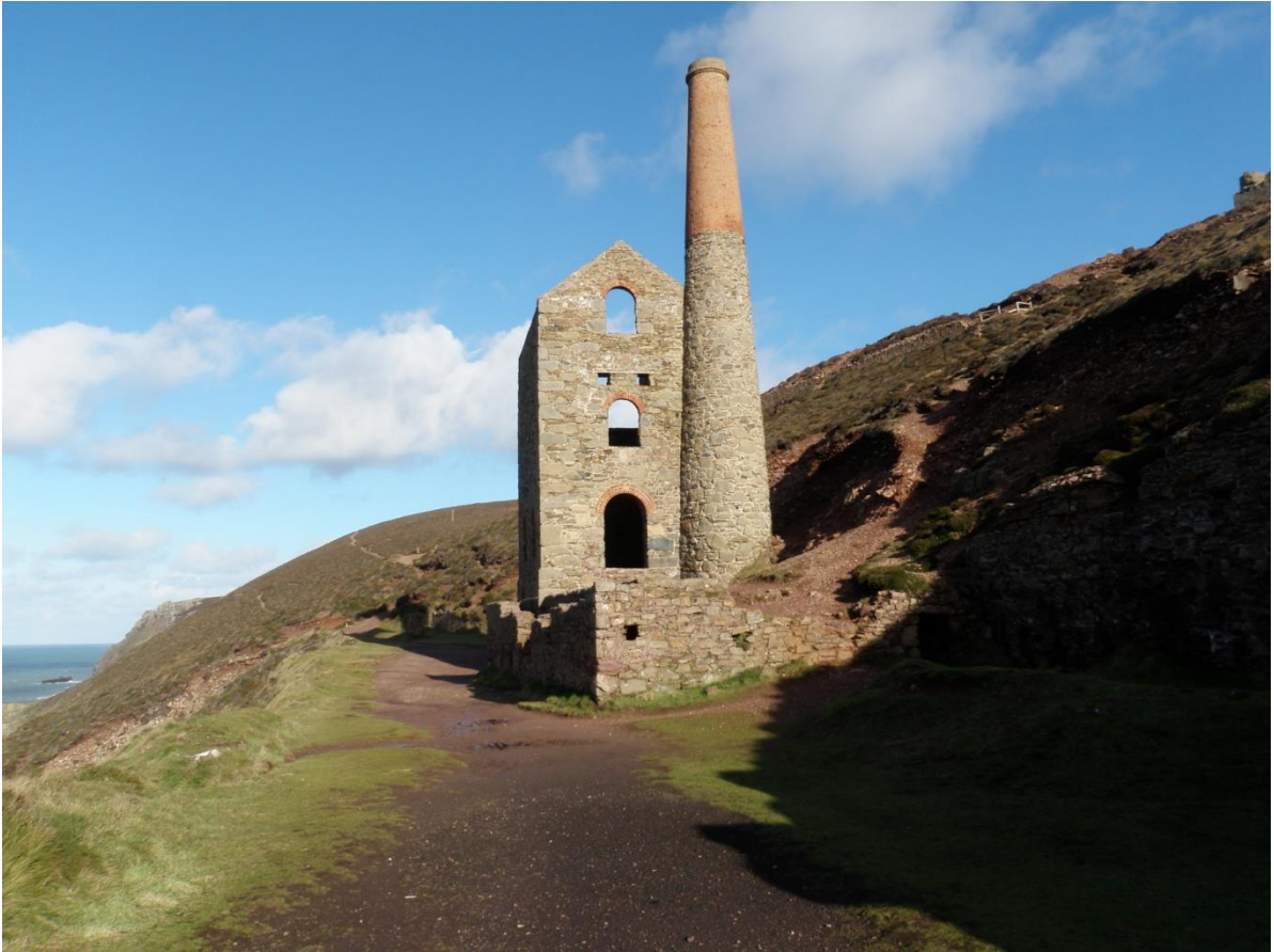
Fig 34. Towanroath engine house and the remains of the later horizontal engine house (foreground). The boiler house is in the shadowed area to their right.
