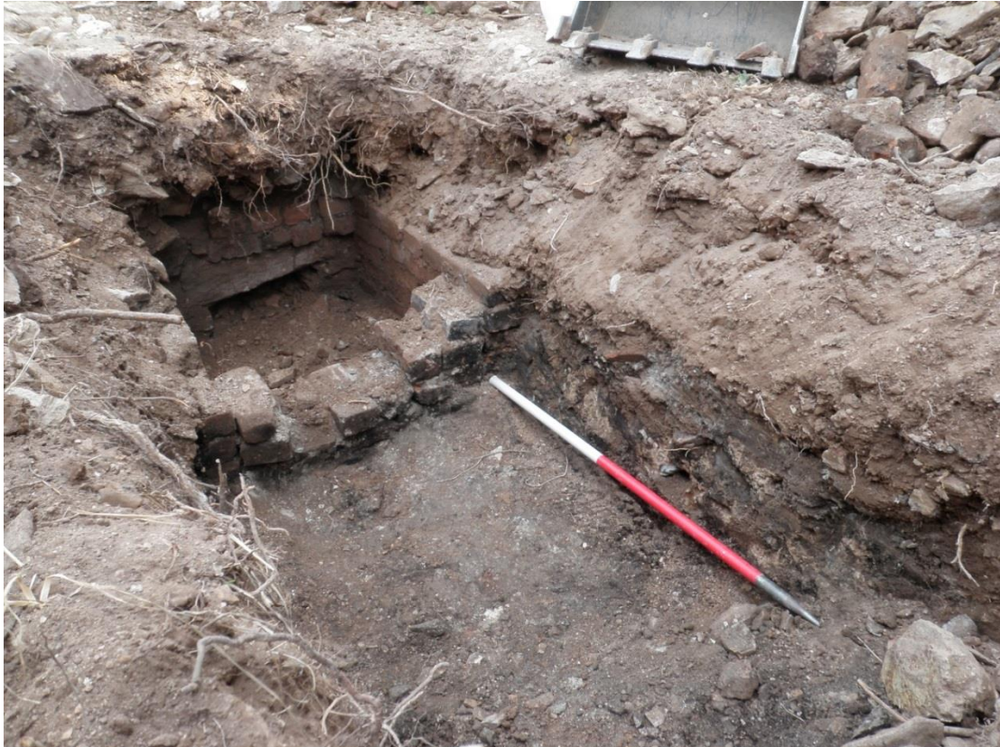
Fig 57. The under-flue for the single boiler revealed during the excavation of the interior of the boiler house at Charlotte United.
