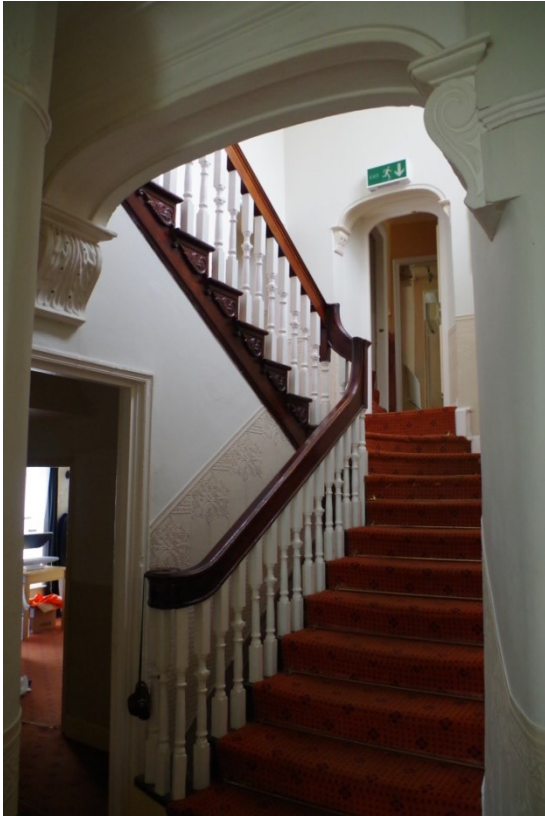
Fig 15 Staircase in projection to rear.
