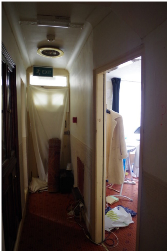
Fig 16 Hallway to east of dining room leading to door onto Church Street.
