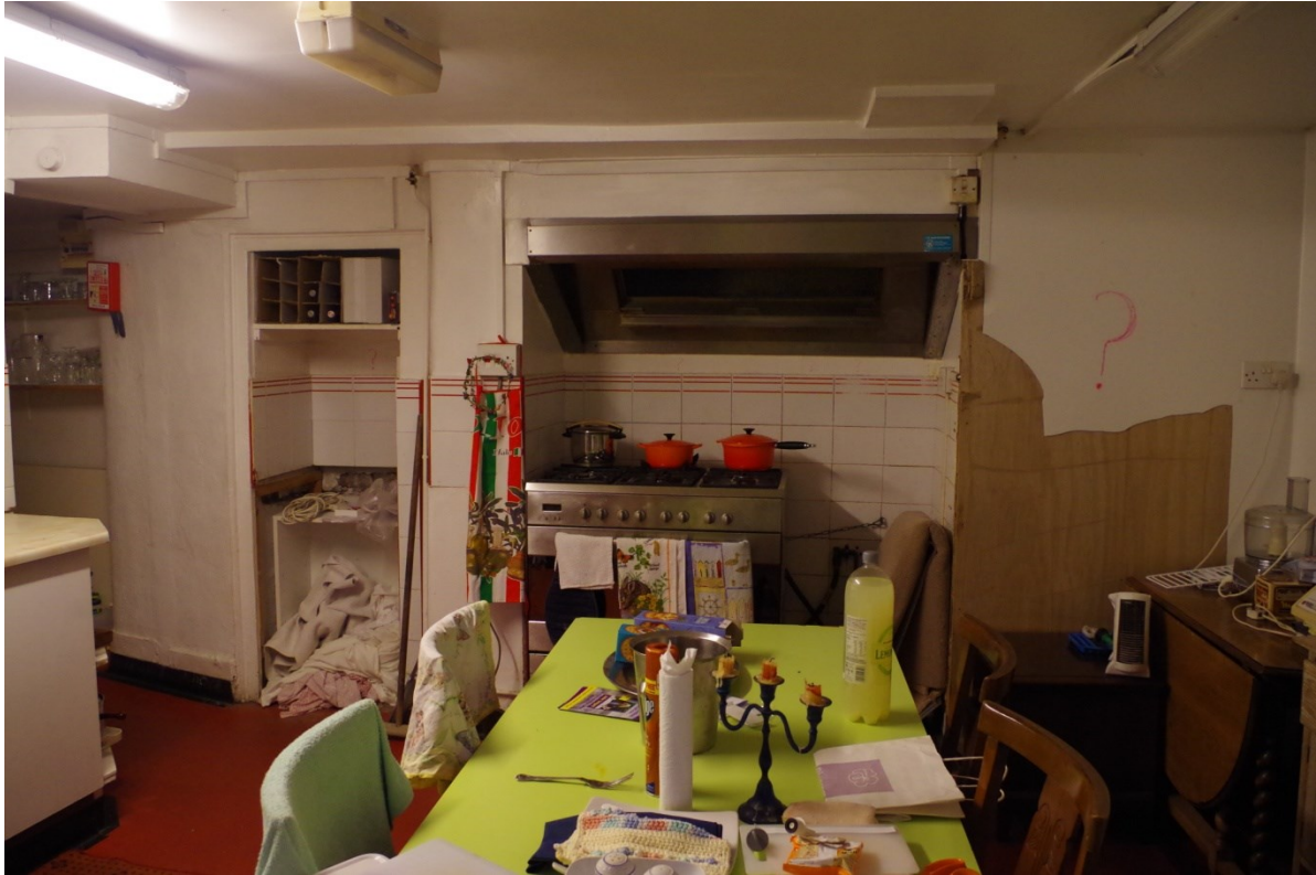
Fig 17 Kitchen looking south, showing rear wall of former cottage.
