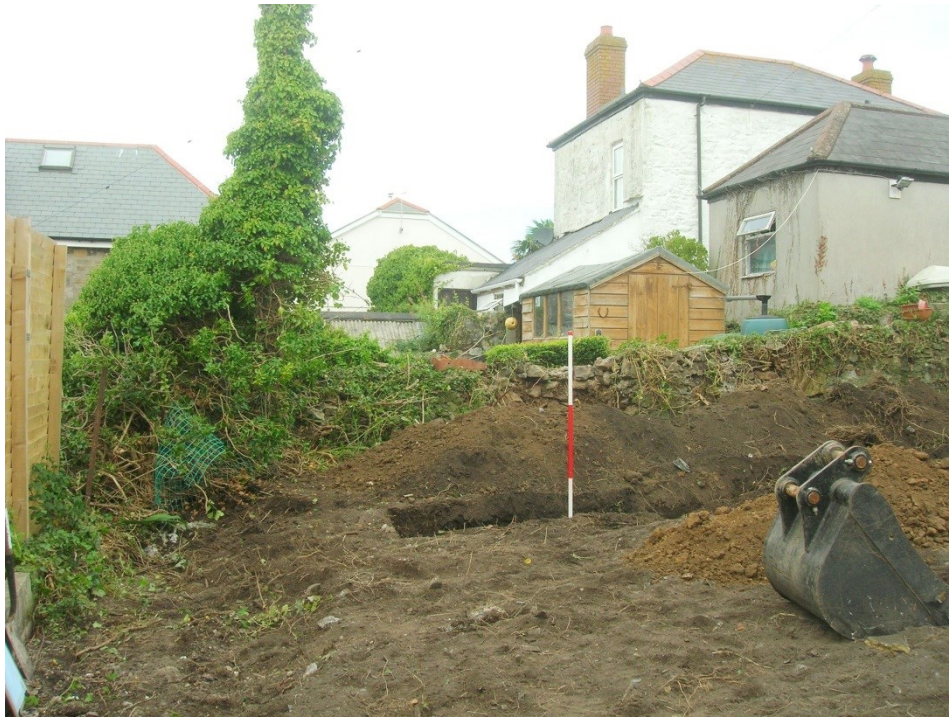
Figure 5. Location of drainage trench looking west.
