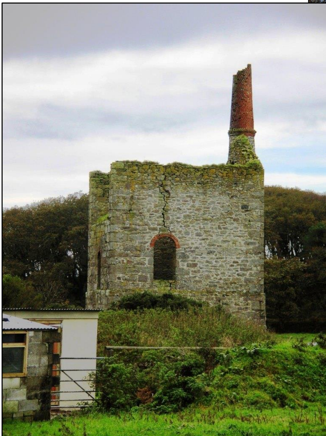
Figure 8 Engine house from South (© CAU 2014).
