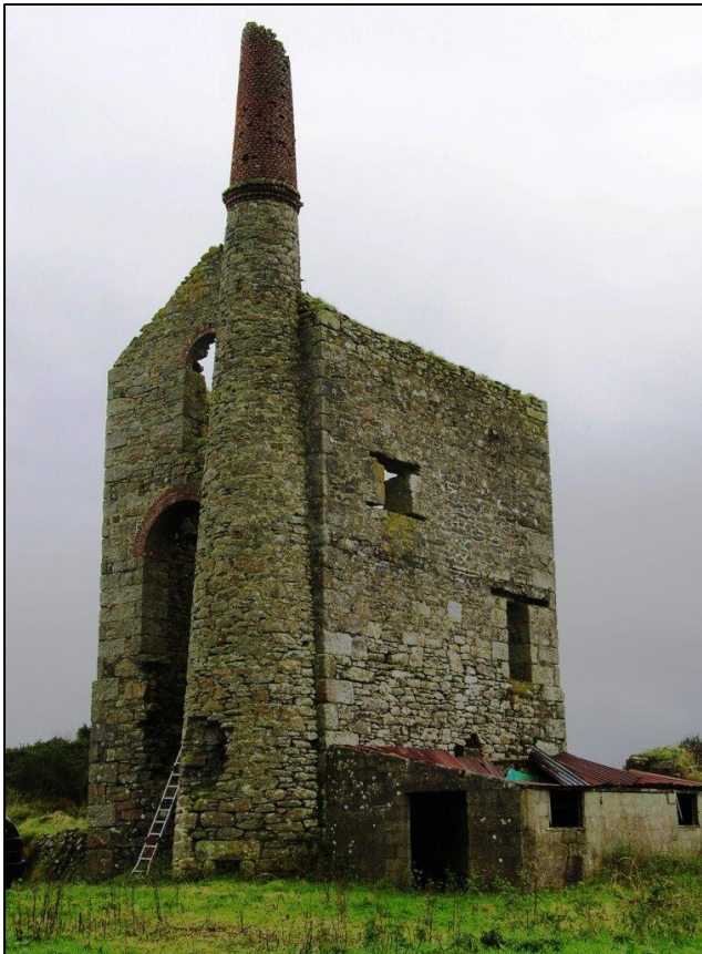
Figure 7 Engine house from North-west (© CAU 2014)
