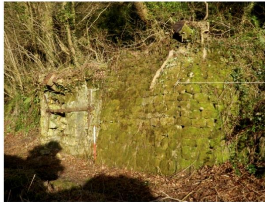
Retaining wall adjoining tank
