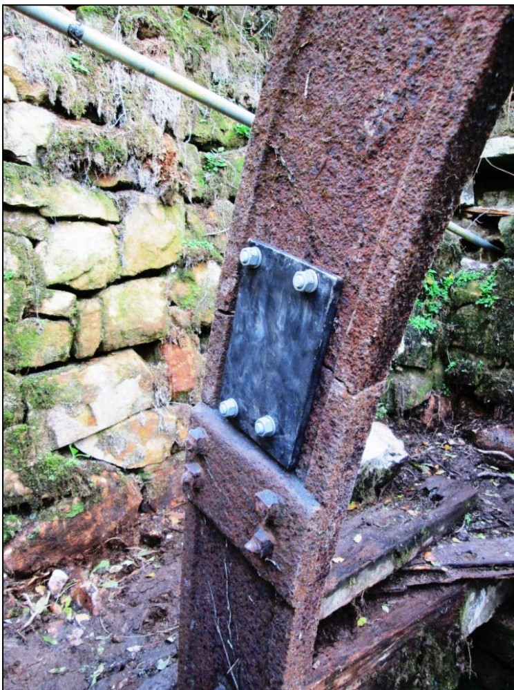
Figure 10 Detail view of the Wheal Arthur water wheel new cross rod steel replacements and new oak timber struts after works © CAU CC 14/5/2015.
