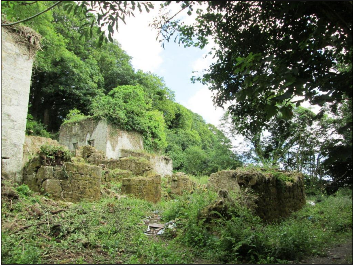
Figure 37 View of the pan kiln, linhay and cottage before works © CAU, CC 15/7/2014.
