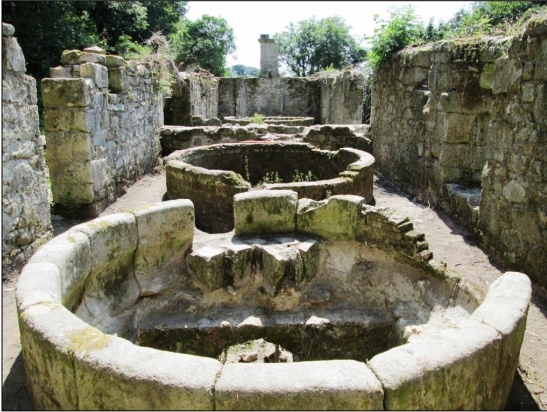
Figure 32 View of the first floor grinding pans and walls before works (looking south) © CAU, CC 23/7/2014.
