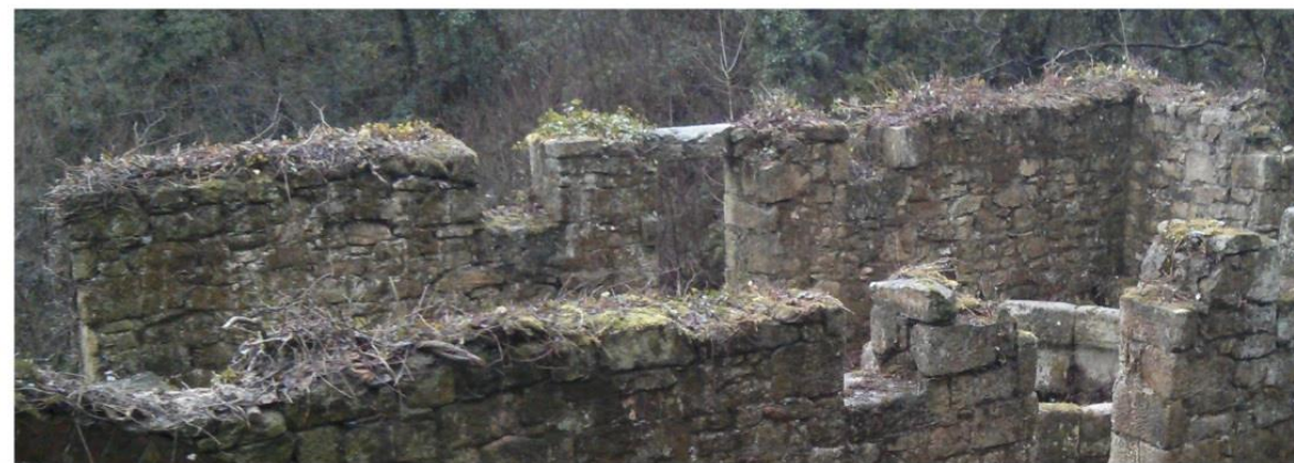
View of internal face of west elevation (north side)
