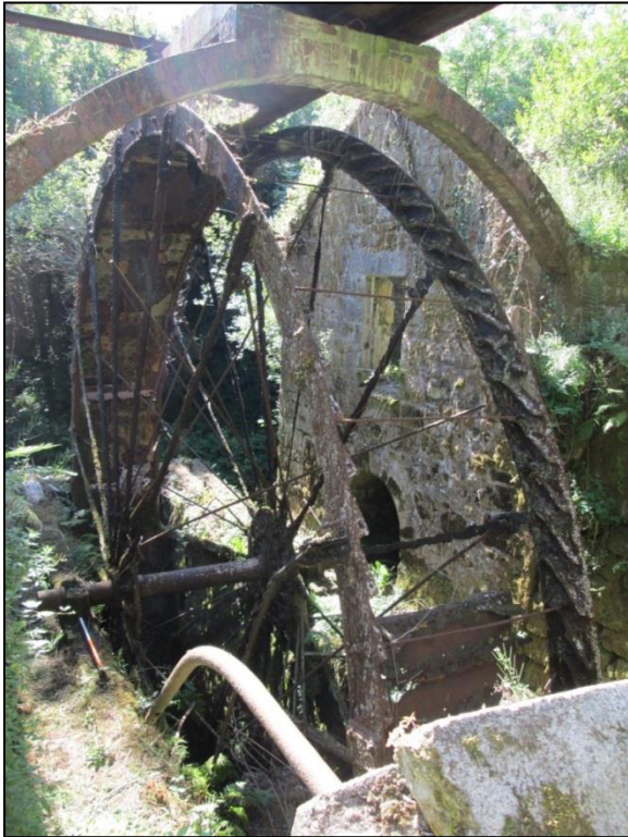
Figure 16 View of the Big Wheel china stone mill 'intact' water wheel from the north west after clearance works © CAU, CC 21/10/2014.
