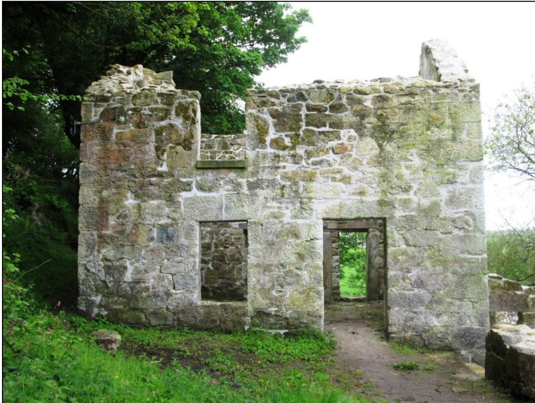
Figure 43 North view of Trevear cottage after works © CAU, CC 14/5/2015.
