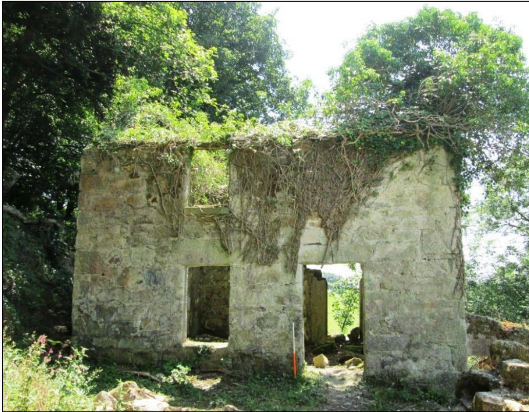
Figure 42 North view of Trevear cottage before works © CAU, CC 23/7/2014.
