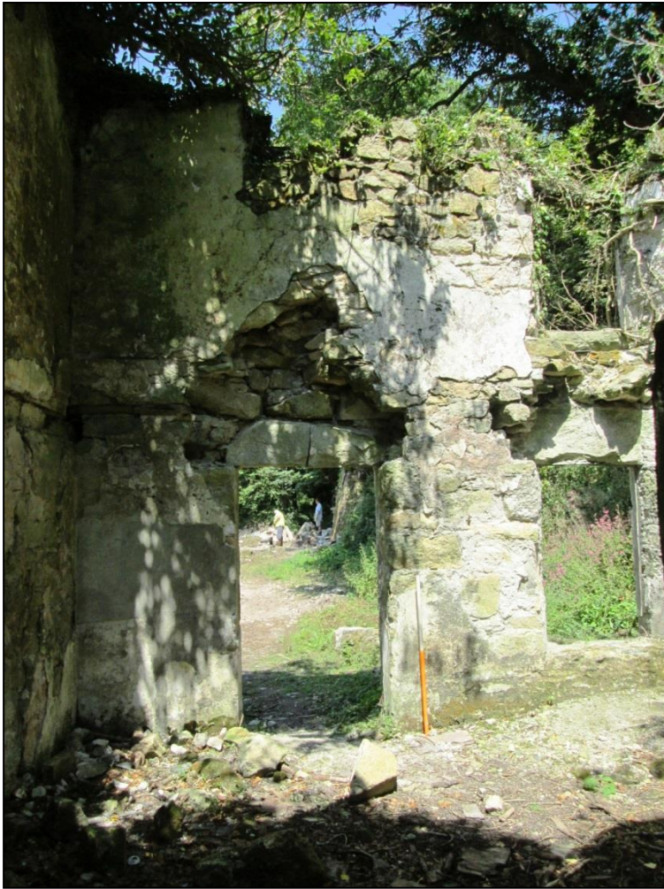
Figure 48 View of Trevear cottage internal north elevation before works © CAU, CC 30/7/2014.
