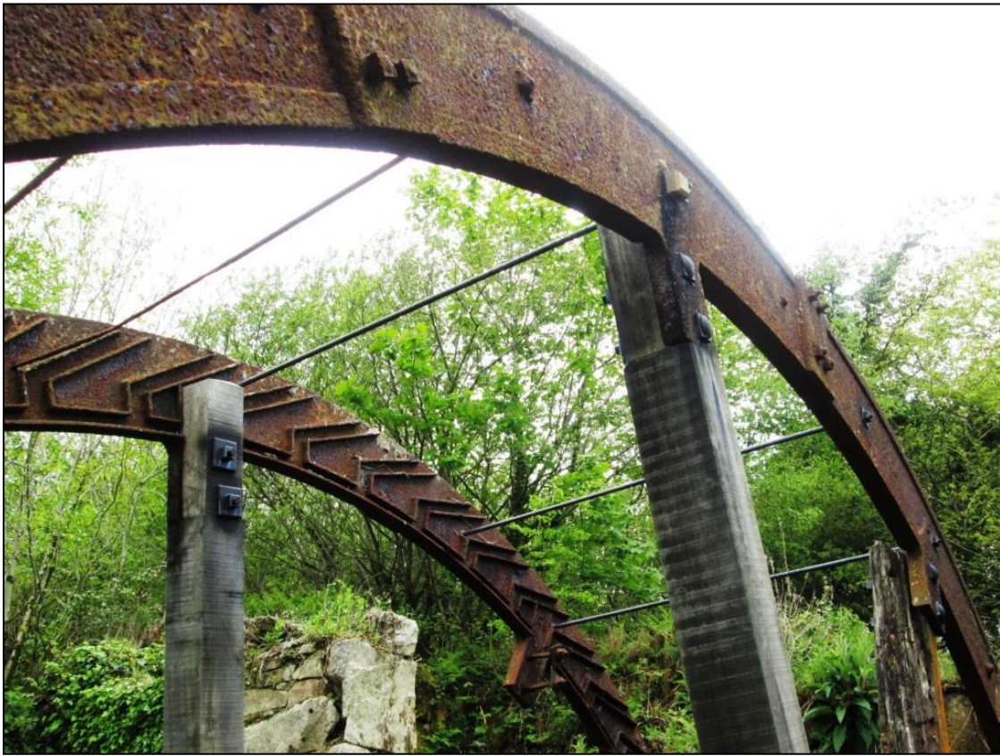
Figure 10 Detail view of the Wheal Arthur water wheel new cross rod steel replacements and new oak timber struts after works © CAU CC 14/5/2015.
