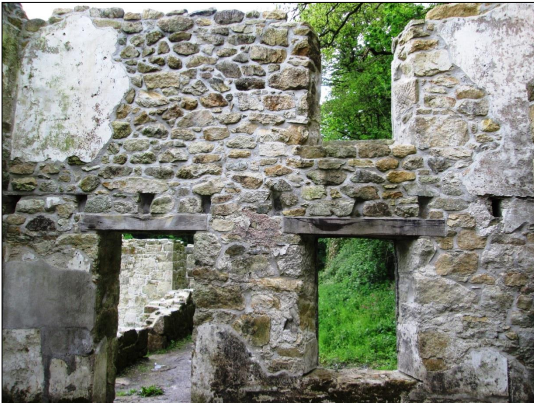
Figure 49 View of Trevear cottage internal north elevation after works © CAU, CC 15/5/2015.
