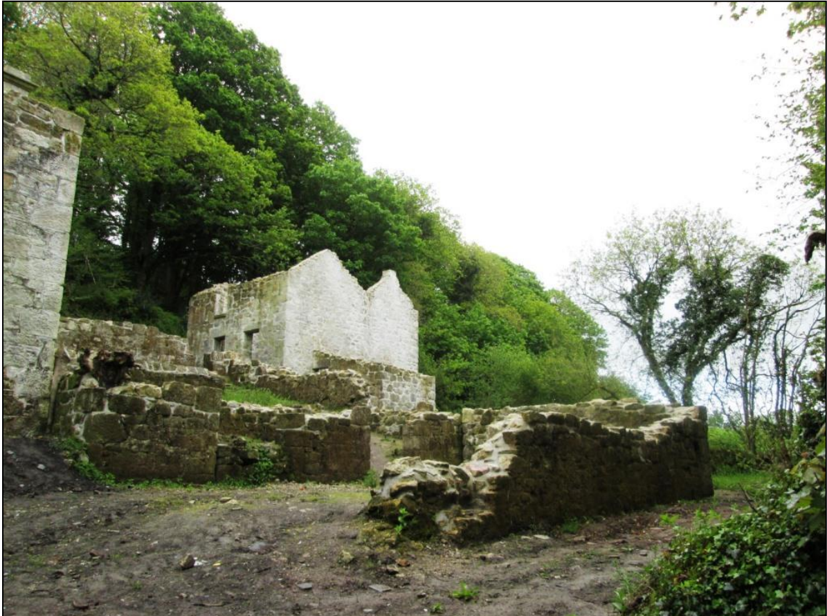
Figure 38 View of the pan kiln, linhay and cottage after works © CAU, CC 14/5/2015.
