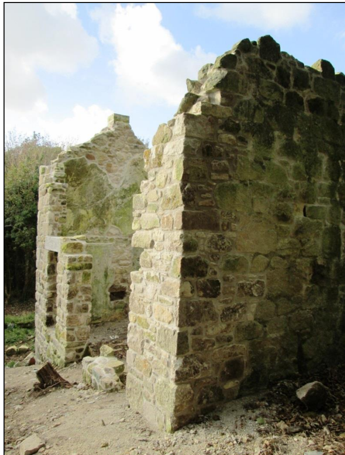
Figure 45 View of Trevear cottage south external elevation after works © CAU, CC 25/11/2014.
