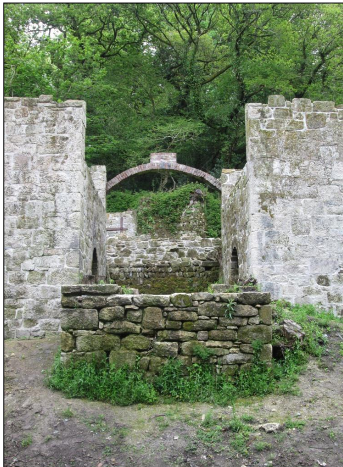
Figure 29 View of the west side of the Trevear wheelpit after works © CAU, CC 14/5/2015.
