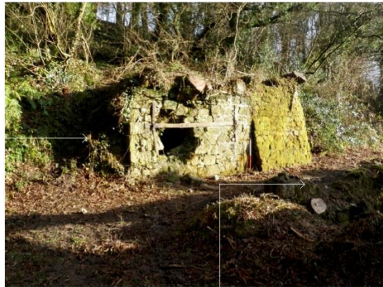
General view of tank
