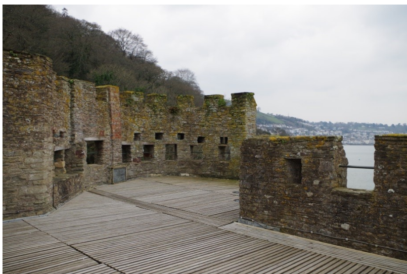
Gun Tower, roof.
