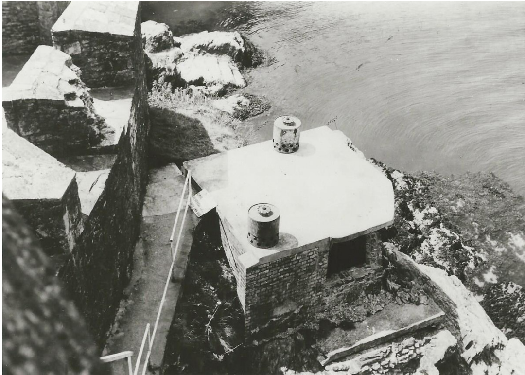
Fig 22. The pillbox for the heavy machine gun covering the harbour boom during WW2. It has been suggested that the two features on its roof might have housed smoke generators. The pillbox, which was sited next to the northern gun platform, was demolished a few years ago.
