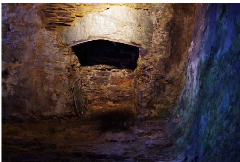
Fireplace in the basement of the Square Tower.
