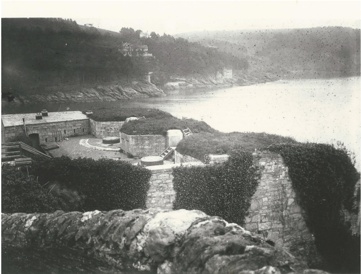
Fig 18. Dartmouth Point Battery during the inter-war period in the 20 th Century showing the mountings for the pair of QF guns which had been mounted there during WWI.
