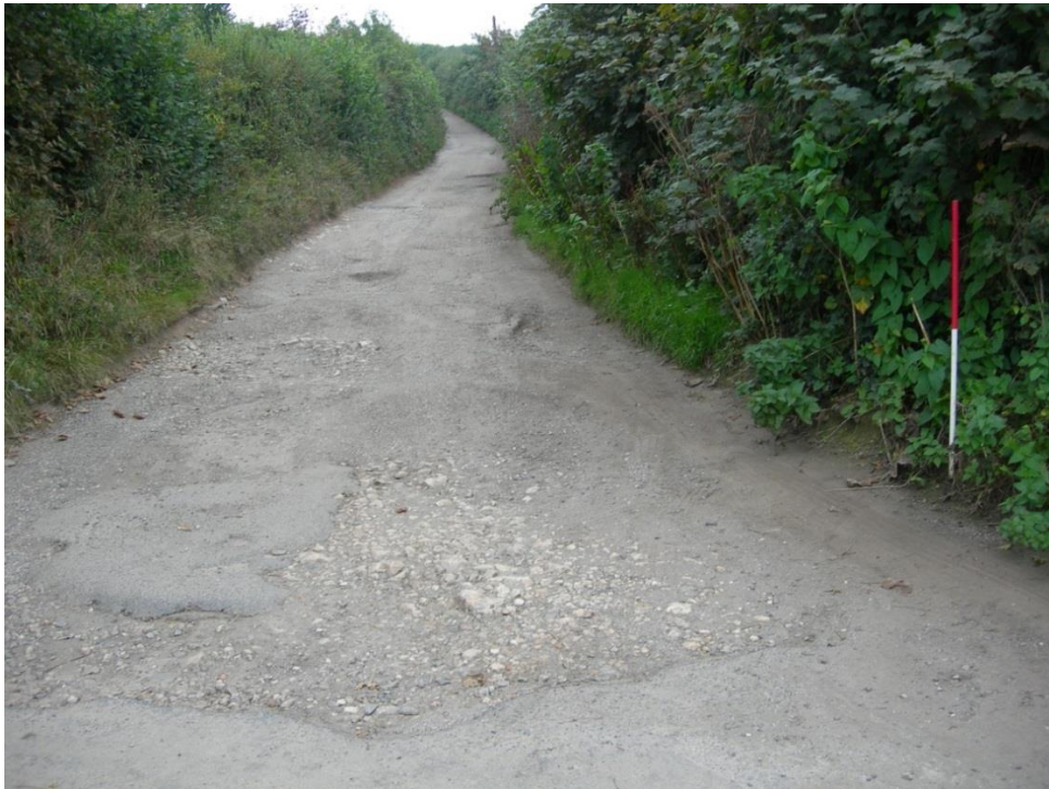
Fig 5 West end of the byway, with quartz metalling visible in the mouth of the lane, though largely obscured by previous resurfacing on the ascent in the rear ground (NGR SW 82857 40425, looking east).
