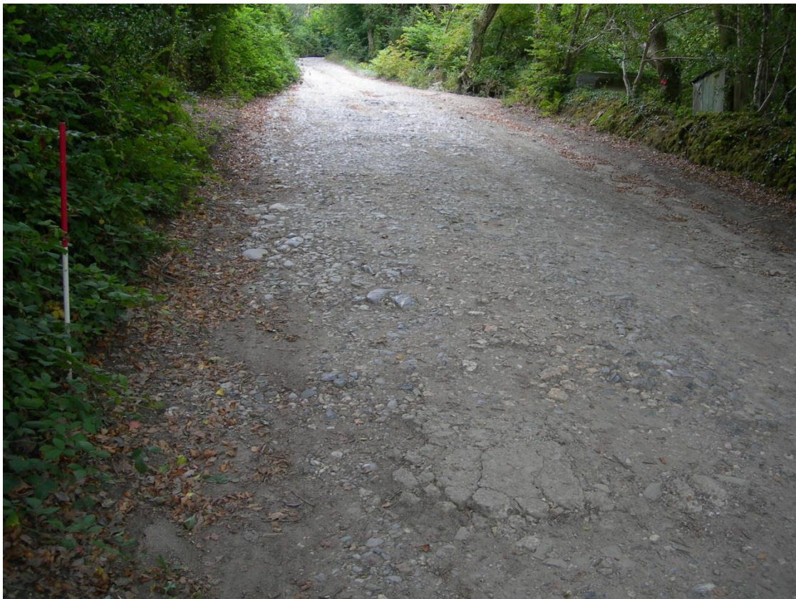
Fig 22 Surface between caravan and Quay Cottage with concrete patch (foreground) (NGR SW 83755 40466, looking SW).
