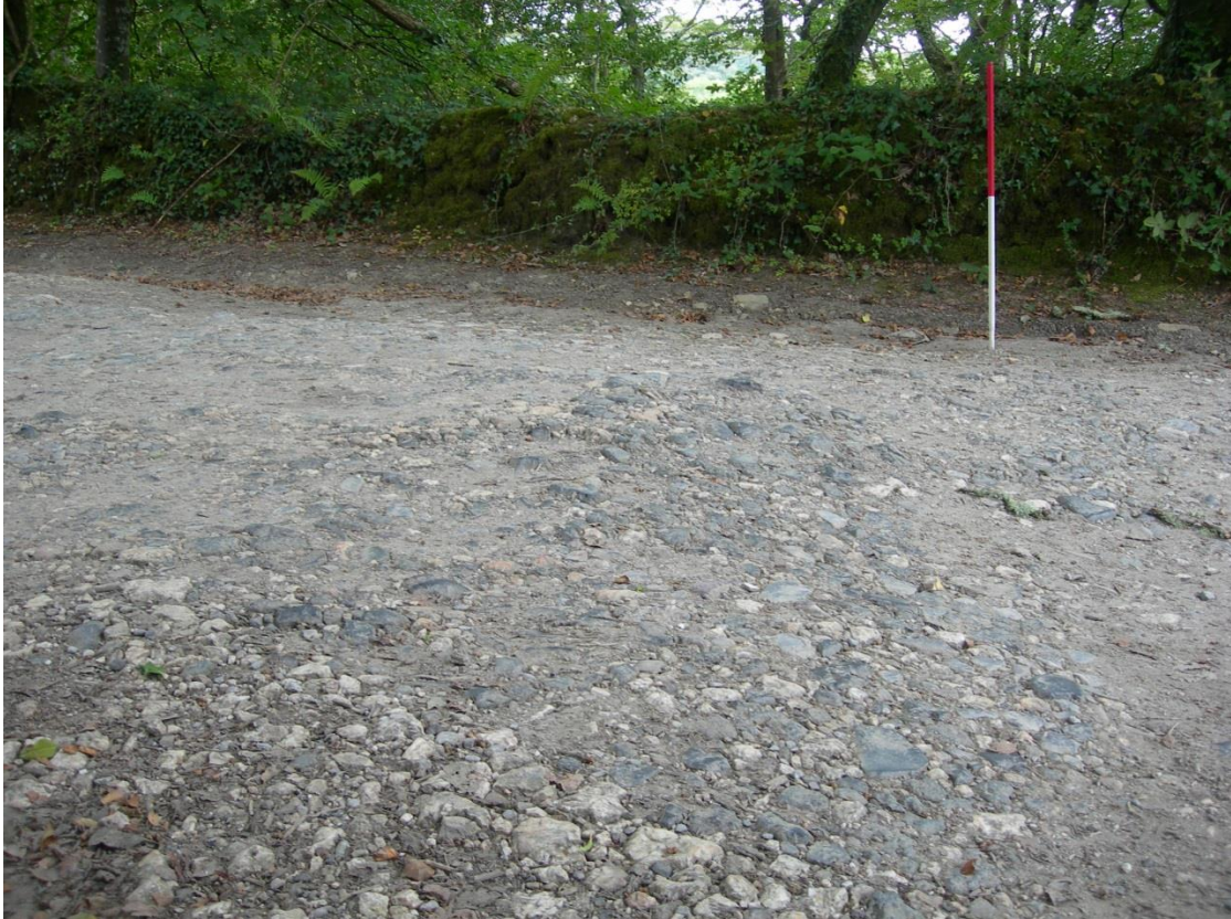
Fig 23 Lane showing mixed metalling fabric, and boundary bank, west of Quay Cottage (NGR SW 83756 40465, looking NW).
