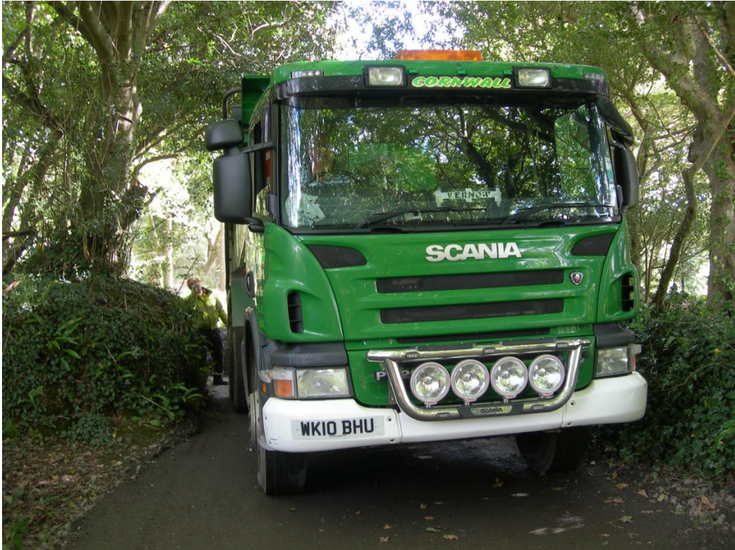
Fig 26 Truck delivering tarmac planings passing through the outer cross-rampart. Its front is on the causeway of the rampart's ditch, already made up with aggregate.
