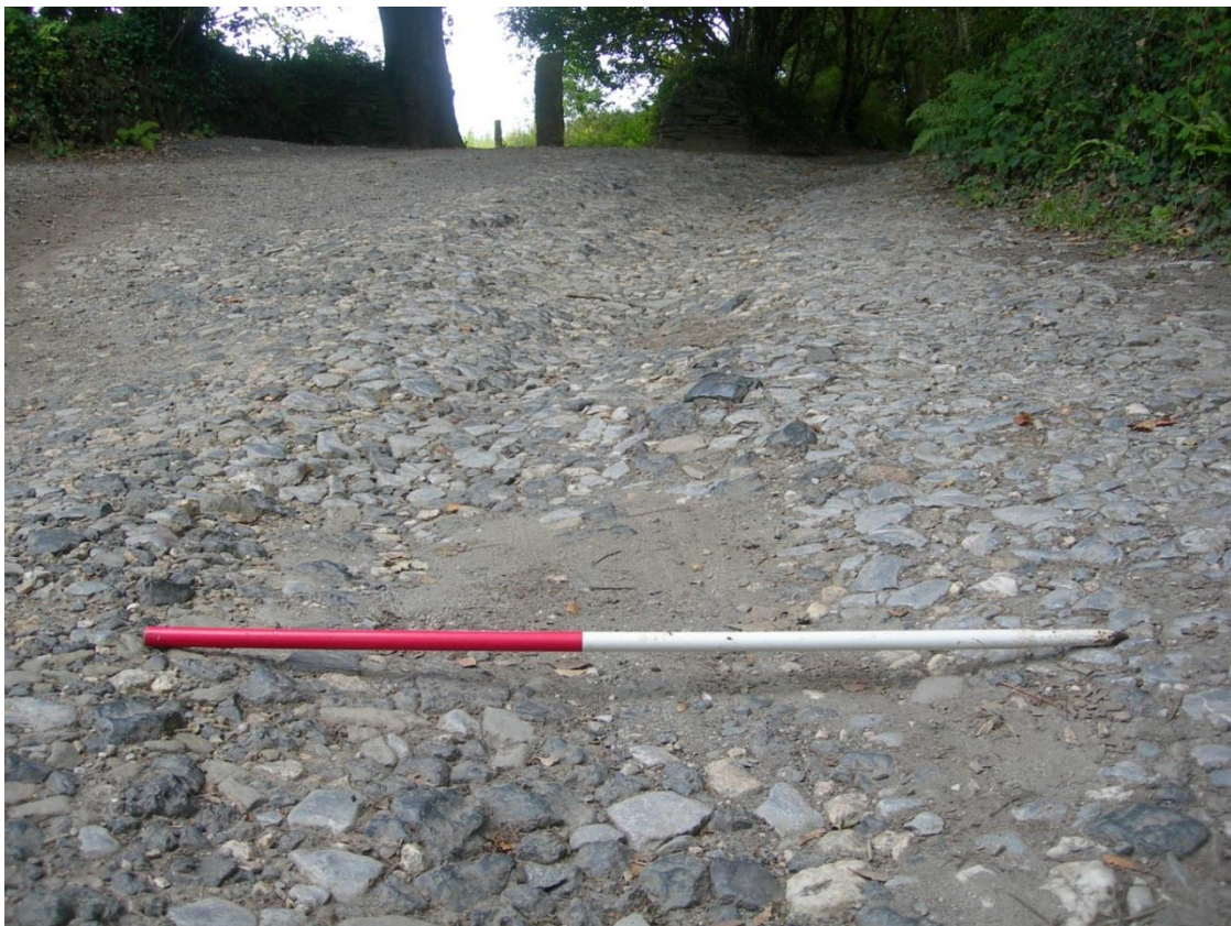
Fig 12 Limestone and slag metalling with linear hollow curving through fort entrance (NGR SW 83595 40391, looking west).
