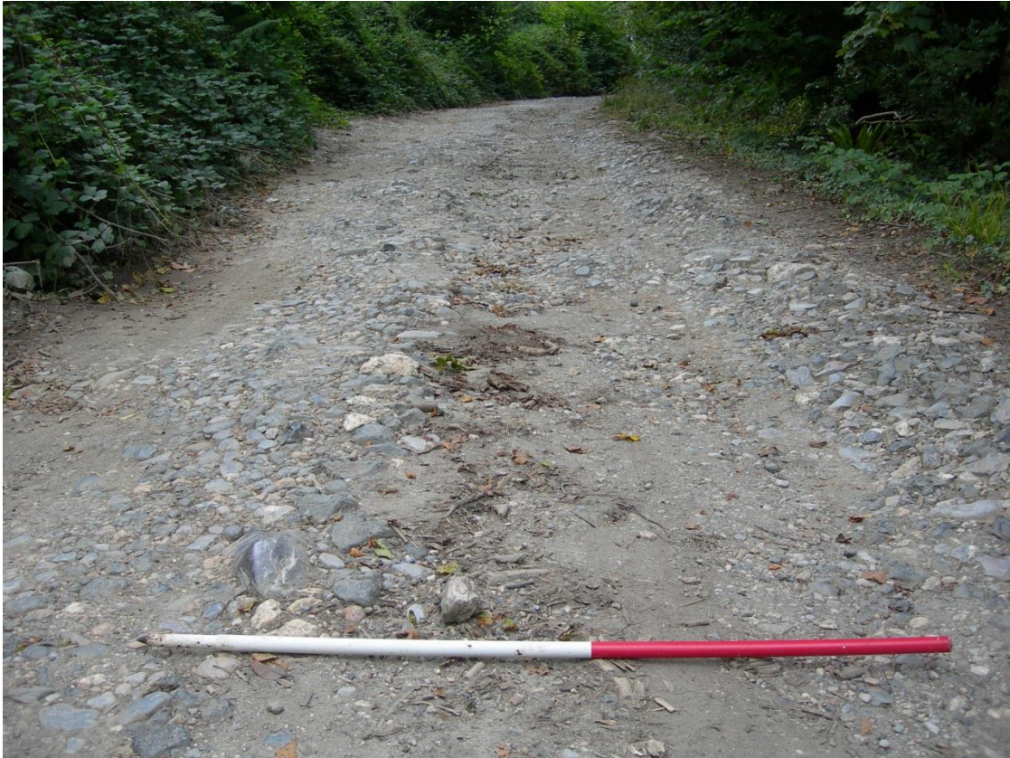
Fig 19 Metalling worn NW of centre, half way from inner cross-rampart to Quay Cottage (NGR SW 83725 40443, looking SW).
