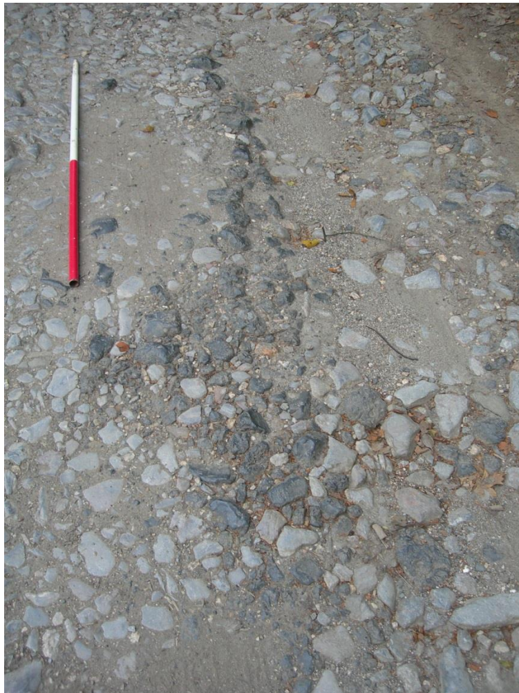
Fig 14 Metalling half way between the cross-ramparts with ridge of slag in limestone (NGR SW 83635 40405, looking south west).
