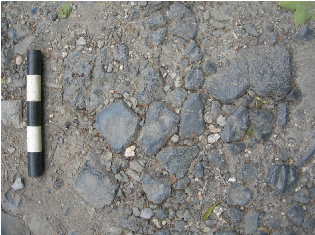
Fig 18 Detail of metalling at Profile A with bubbled slag and some paler grey limestone (NGR SW 83699 40426. Scale is 25cm).
