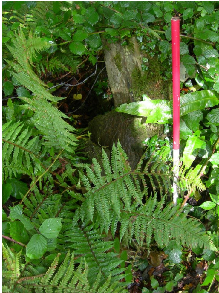
Fig 33 Slab facing to bank NW of lane by inner cross-rampart, with gap used as drain
