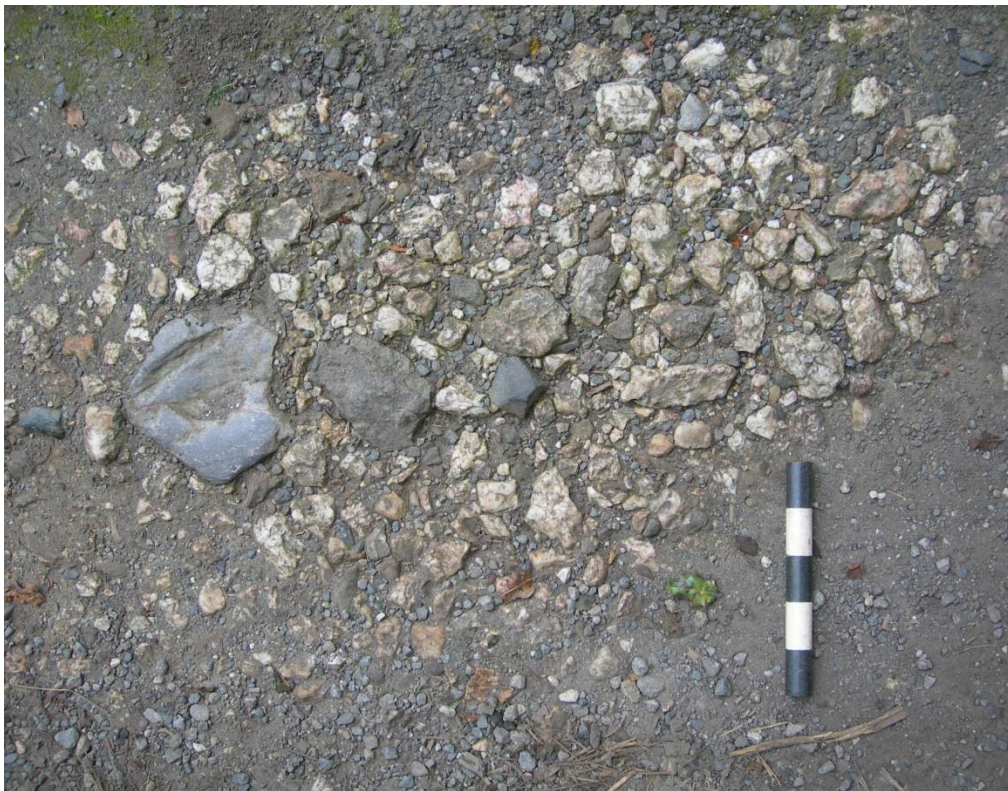
Fig 8 Quartz metalling with bluey-grey limestone to left and copper slag to right of that (NGR 83447 40420. Scale is 25cm).
