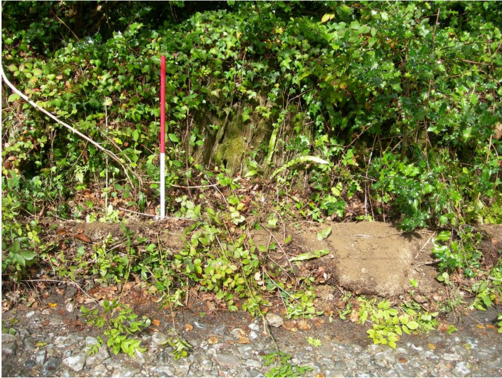
Fig 32 View NW over the south west drain, with its spoil in front, to the lane boundary
