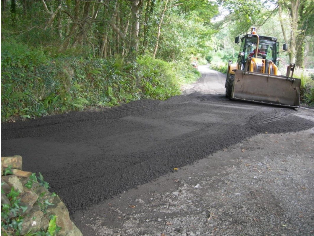
Fig 28 Planings spread on aggregate by and immediately within the outer cross-rampart This is the point where the metalled lane branches NE to the quay from the ridgeway.
