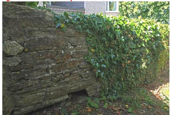
Fig A20 SE boundary wall with horizontally-bedded slatestone
