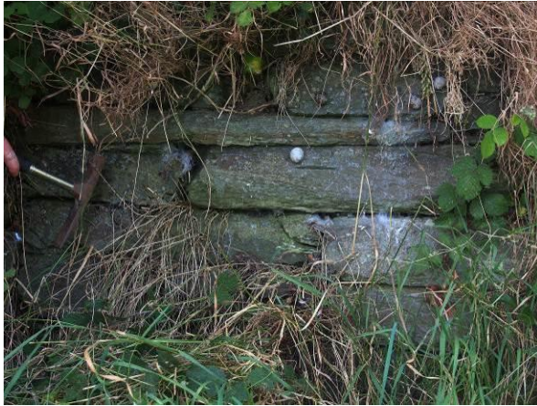
Fig A33 NE wall showing horizontally-bedded pier
