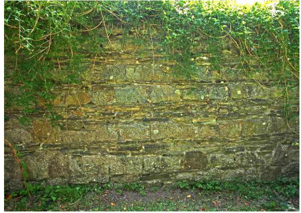
Fig A22 SE boundary wall with alternating slate and granite courses
