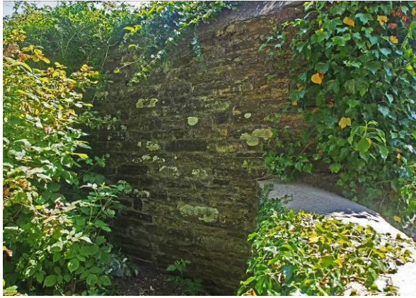
Fig A21 SE boundary wall with horizontally-bedded slatestone
