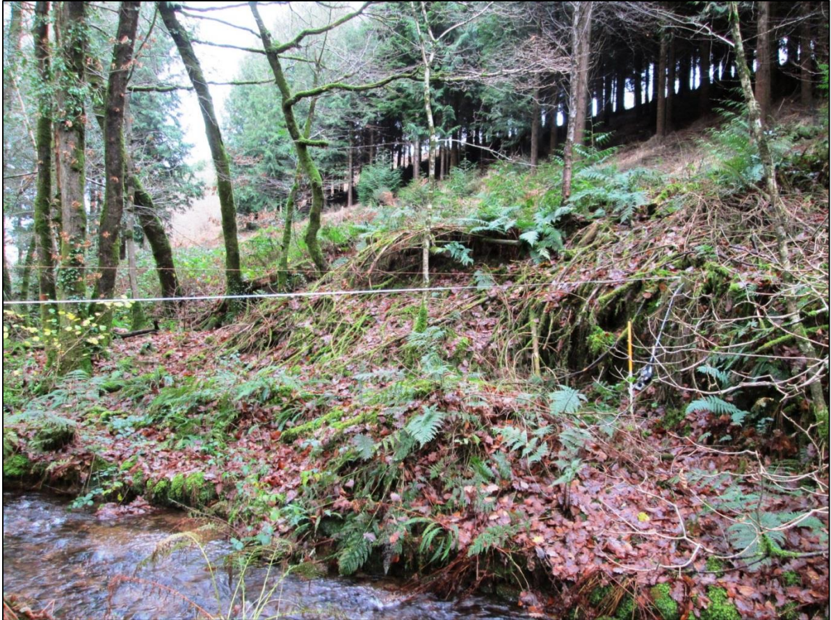
Figure 7: View looking north east across the stream (showing the remains of the leat and wall).
