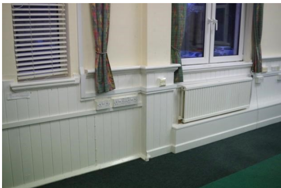
Fig 23 Site 20 interior panelling and moulded sills.
