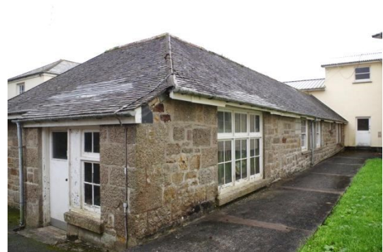
Fig 34 Site 35 late 19 th century stable block looking south-west.
