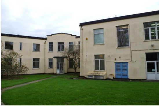
Fig 20 Site 20 looking south-east in quadrangle.
