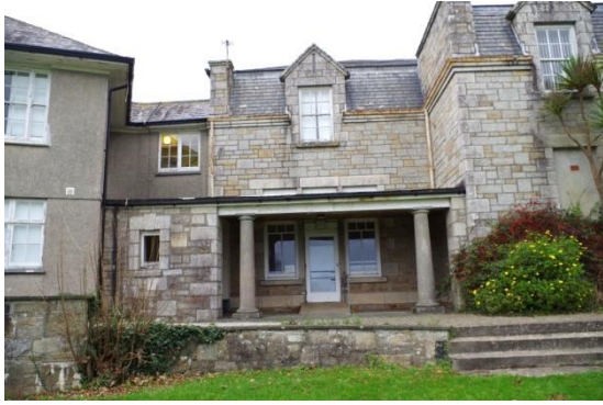
Fig 36 Site 39 looking north.
