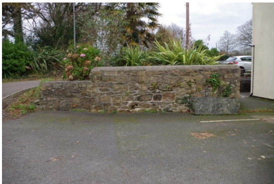
Fig 15 Site 11 looking north.
