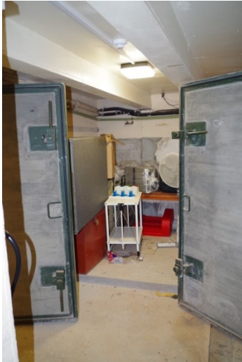
Fig 28 Site 29 looking north.
