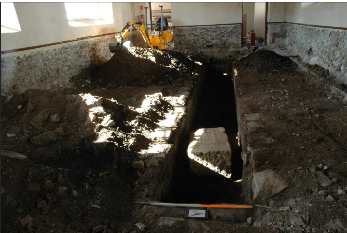
Figure 13: View of inspection pit after excavation.
