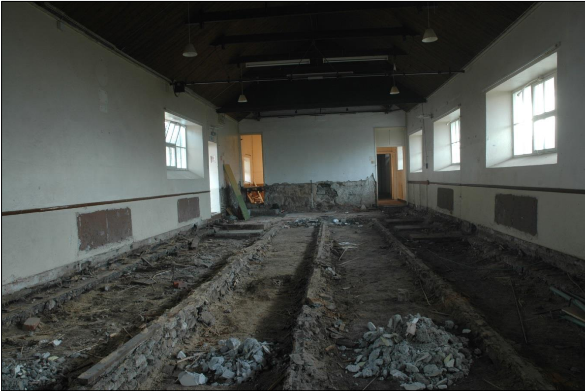
Figure 9: View of the interior of Devoran Village Hall looking east showing floor joists.
