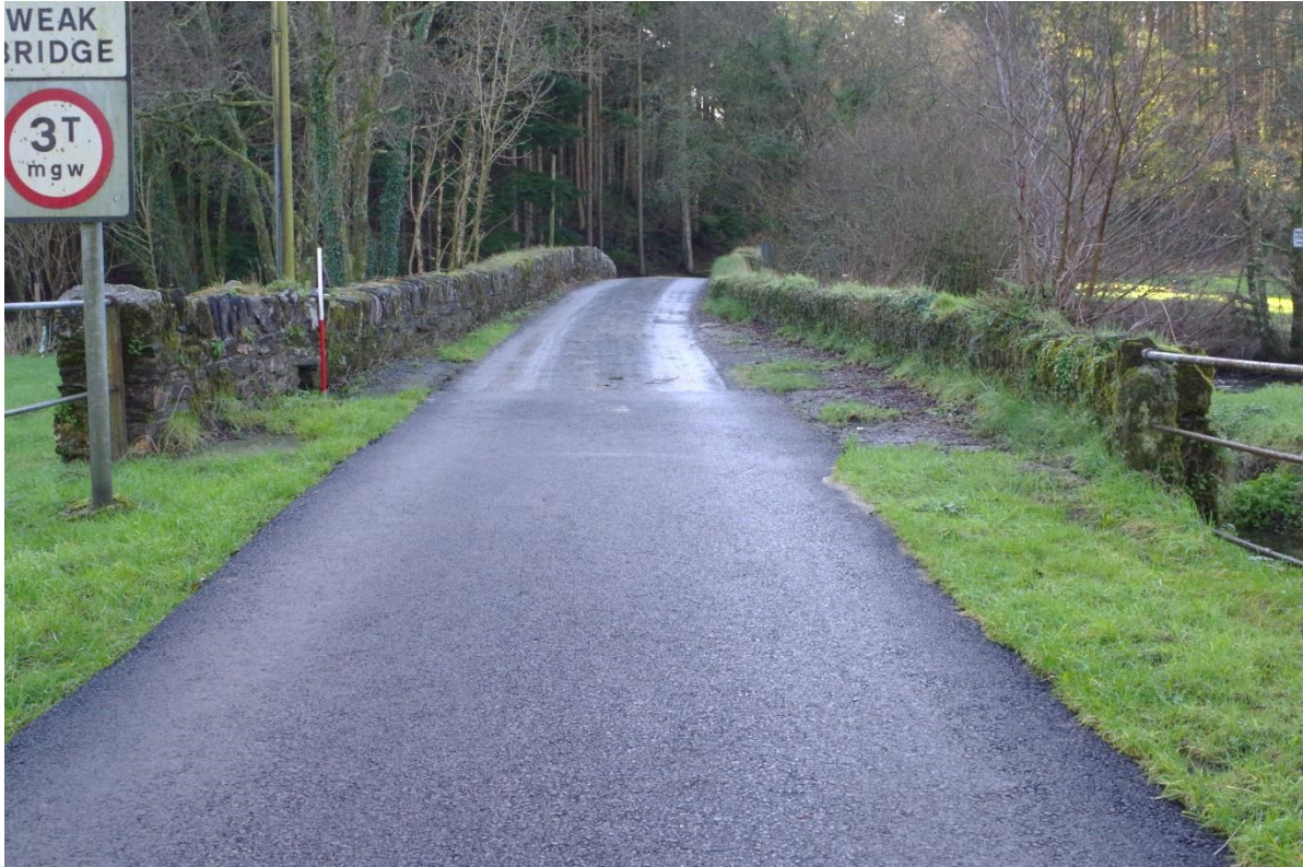
Fig 2 Looking south to the bridge from the direction of Trekener Mill.
