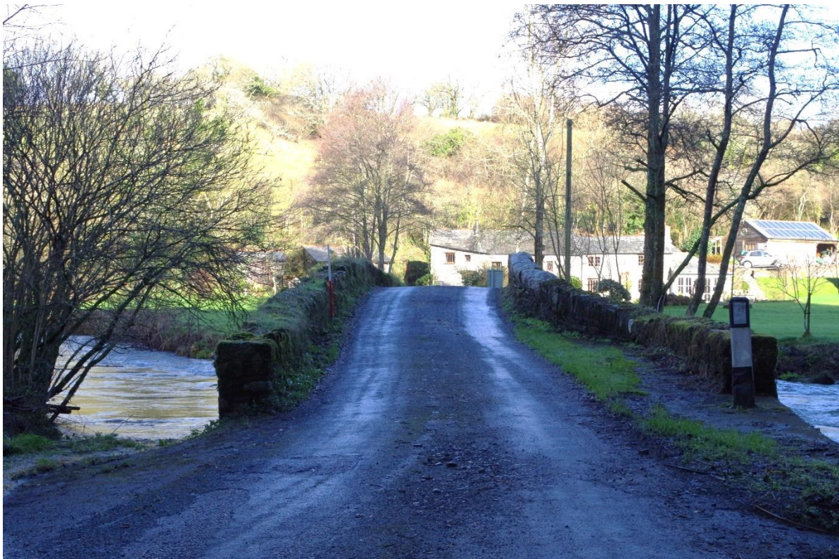
Fig 3 Looking north to the bridge. Note, the access way to the left (the right hand side one is not visible on this photograph)
