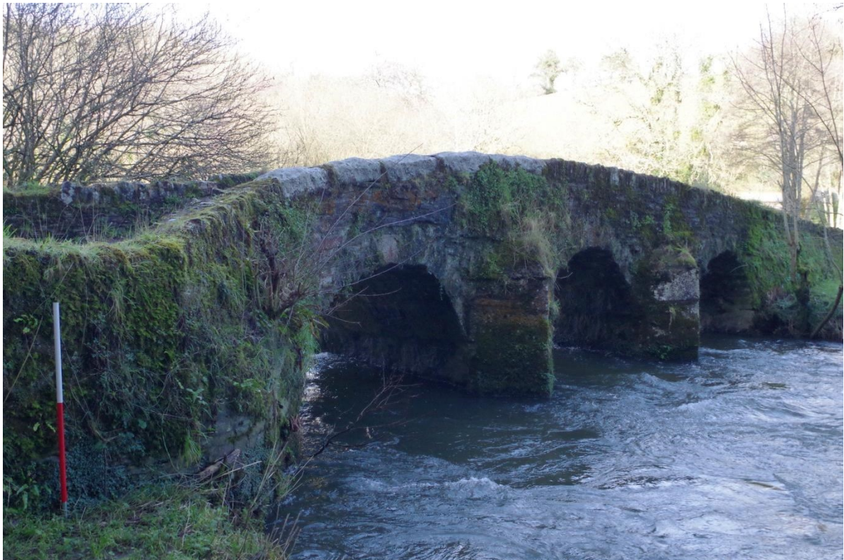
Fig 4 East elevation from the southern side.
