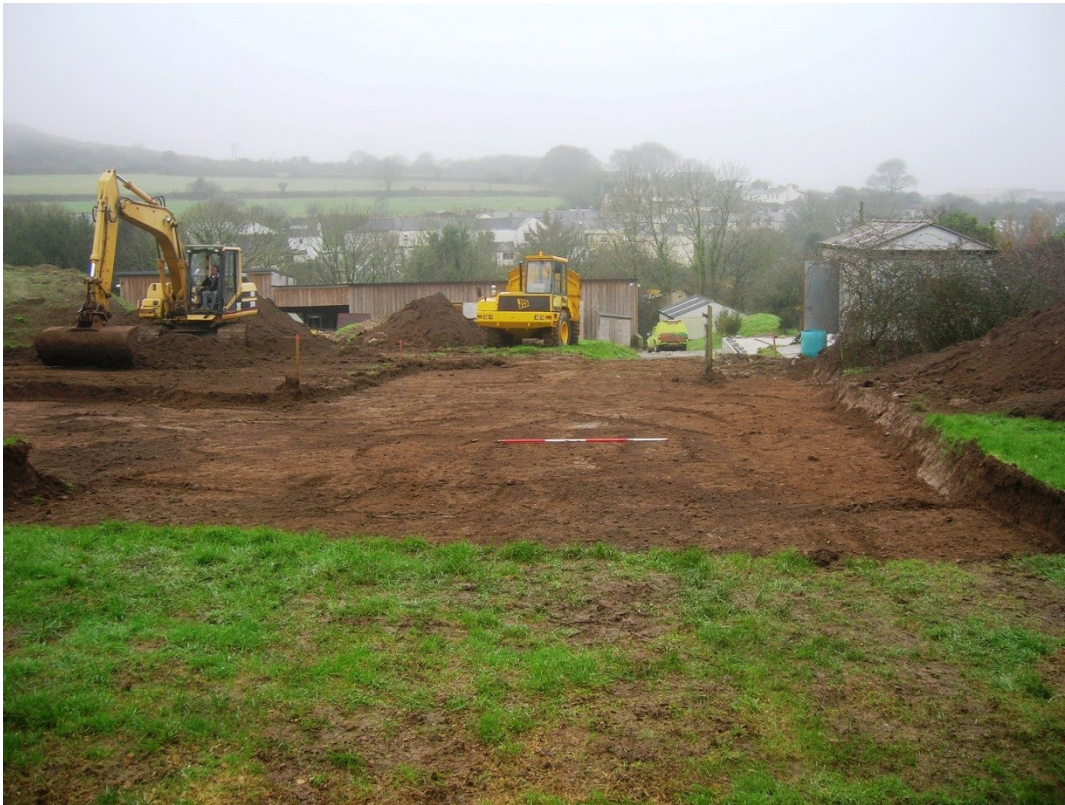
Figure 8. Northern part of site looking west.
