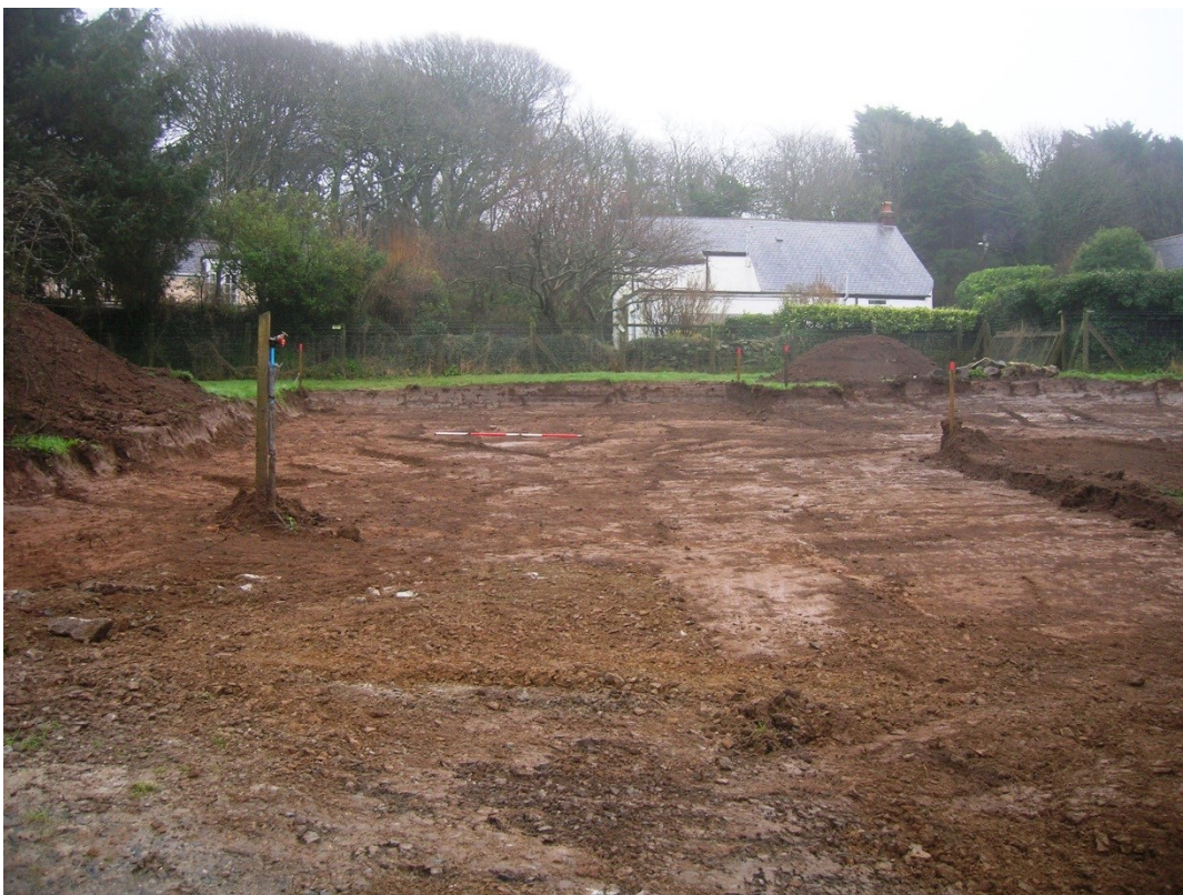
Figure 9. Northern part of site looking east towards Trelowen Cottage.
