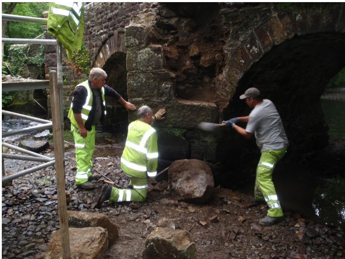
Fig 13 Pivoting the cutwater back to its original position.
