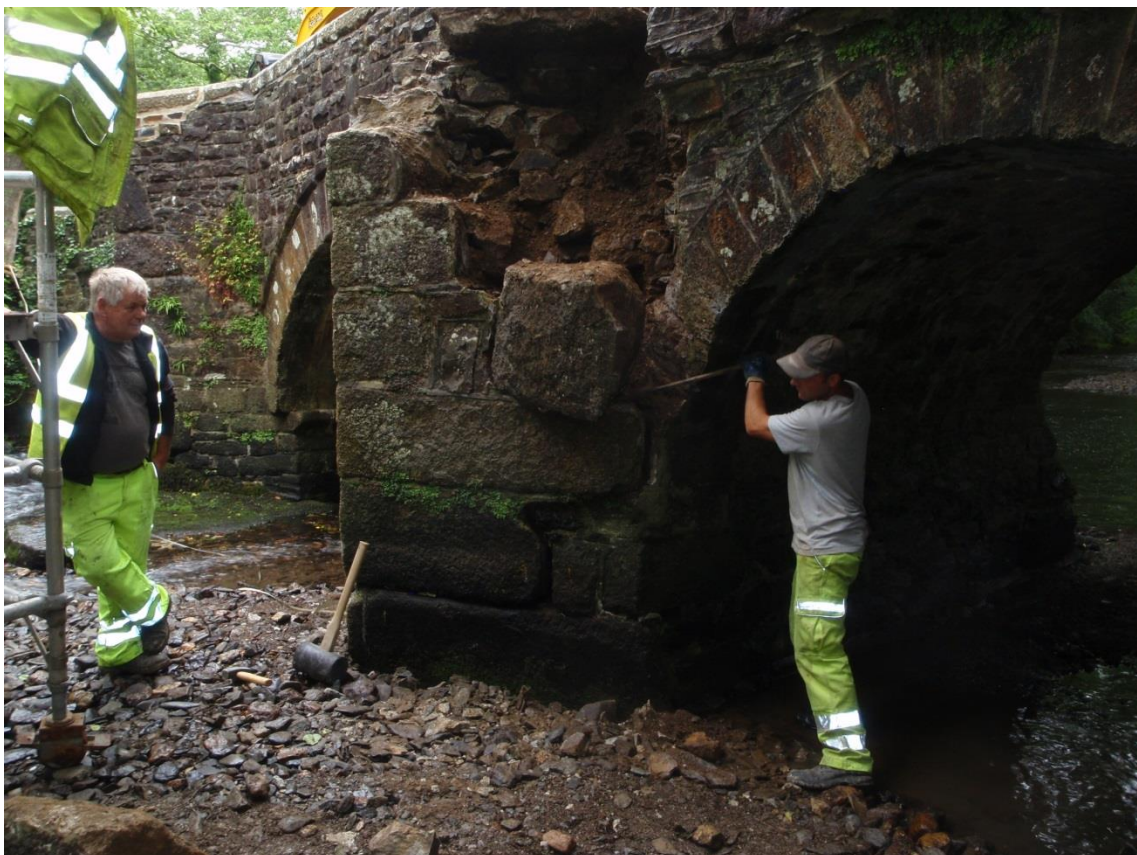
Fig 11 Removing the damaged section of cutwater.
