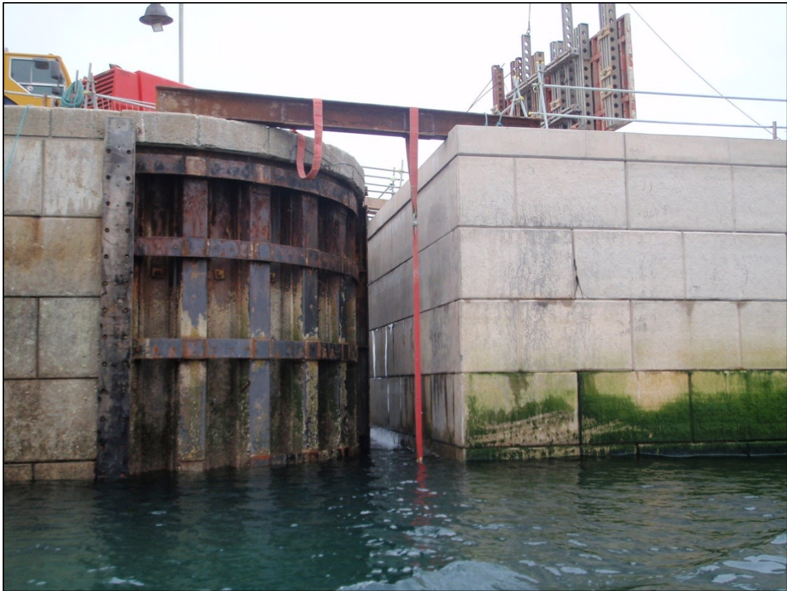
Fig 17 The new pre-cast concrete sections in place, 20 September 2015 (photo: CAU)
