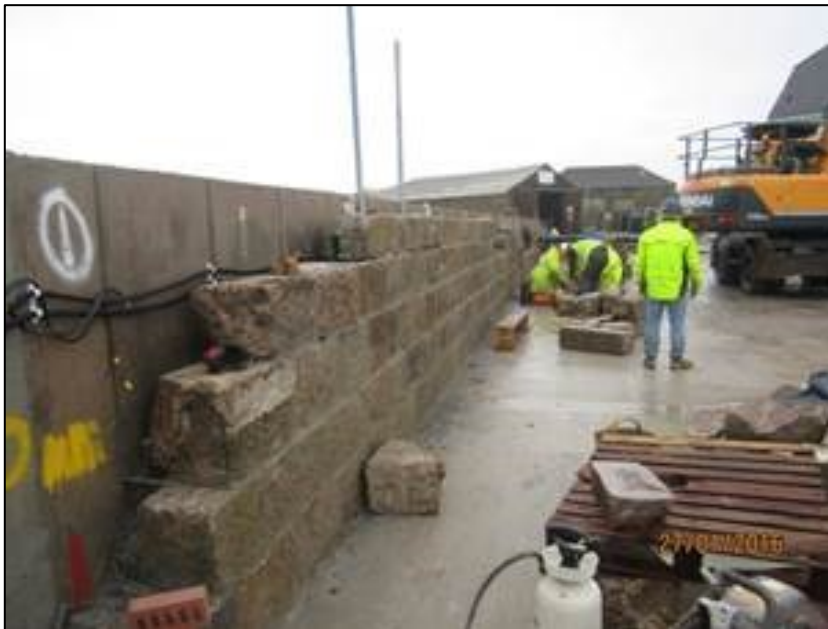
Fig 24 Rebuilding the quay wall (photo: Rients Jan Veldkamp).
