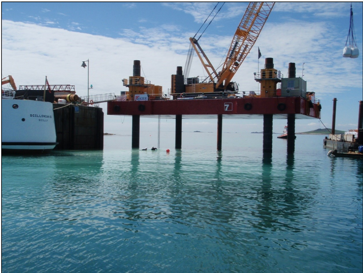
Fig 16 The jack-up barge and large Liebherr crane at the end of the quay on 19 July 2015, almost ready for the pre-cast concrete sections to be put in place (photo: CAU).
