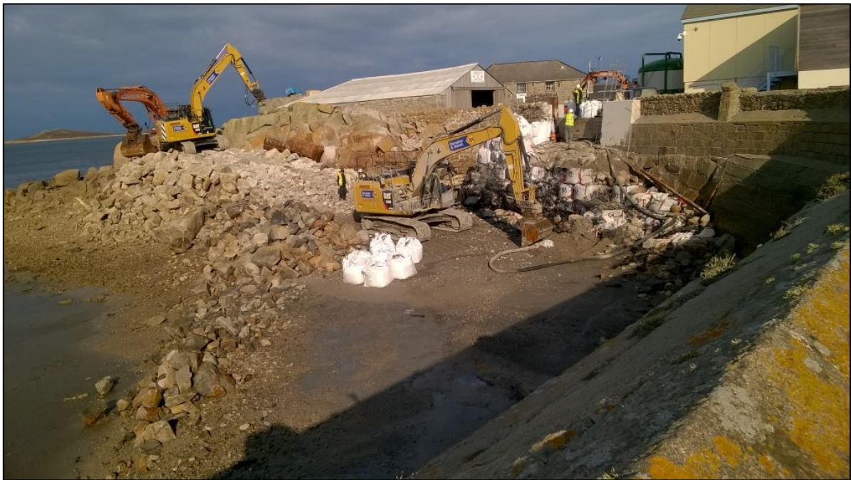
Fig 22 Backfilling of the quay widening area (photo: Rients Jan Veldkamp).
