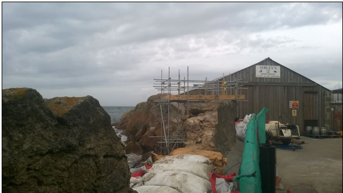
Fig 20 Breach in the quay wall, showing the wall structure (photo: Rients Jan Veldkamp).
