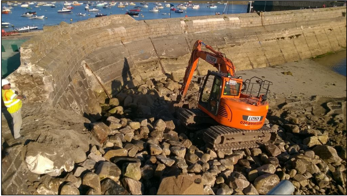
Fig 21 Ramp construction underway (photo: Rients Jan Veldkamp).
