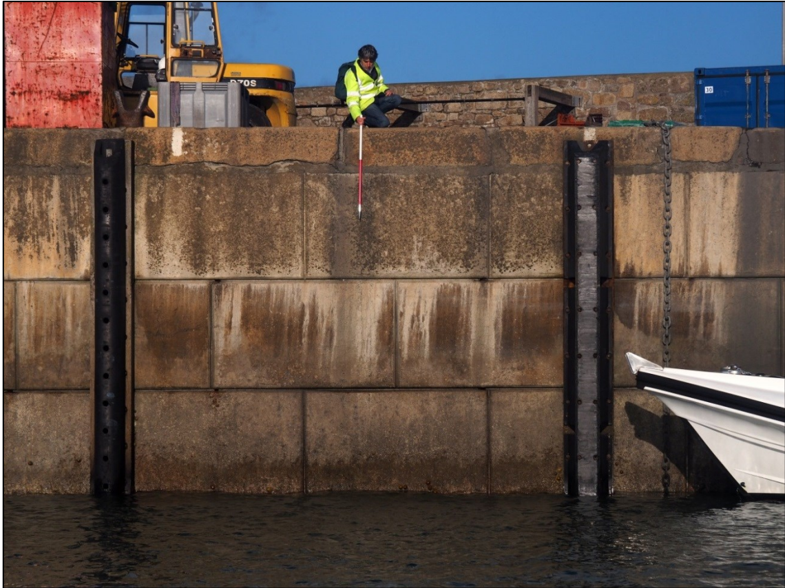
Fig 9 Detail of pre-cast concrete blocks facing the inner side of the quay (photo: Eric Berry).
