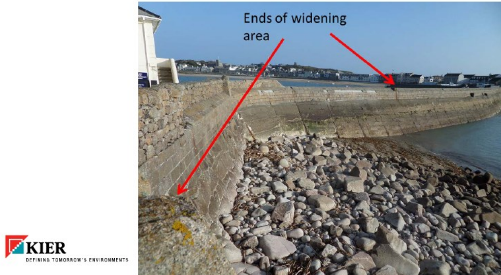
Fig 19 Quay widening scope (Kier).
