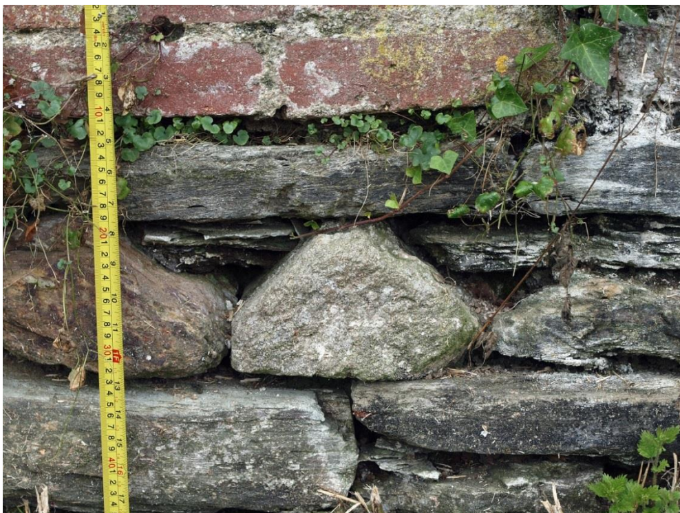
Fig 5 Stone of 17 th century type in the rear wall of the south garden (photo; Eric Berry)
