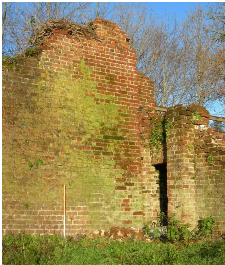
Fig 9 West wall of the south garden ramped up to the ruined summer house Note the ivy-filled feature at the highest surviving point of the wall (see below)
