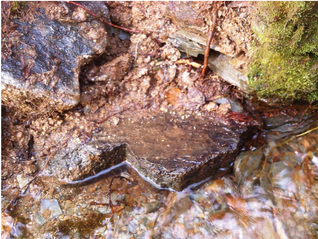
Fig 14 Detail of the lower part of the south east side of the doorway, looking south
