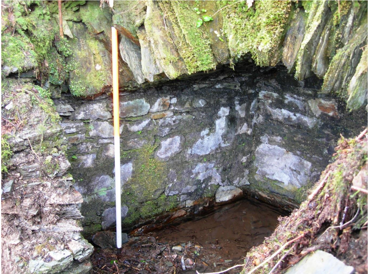
Fig 3 South-east corner of the well, from the doorway. This shows the roughly coursed, mortared stone of the interior, the vaulted roof, and collapse in the doorway (on the left)
