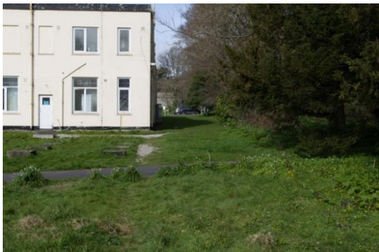
Fig 8 The north eastern corner of the Quadrangle Building (site 20) with the plantation to the right.
